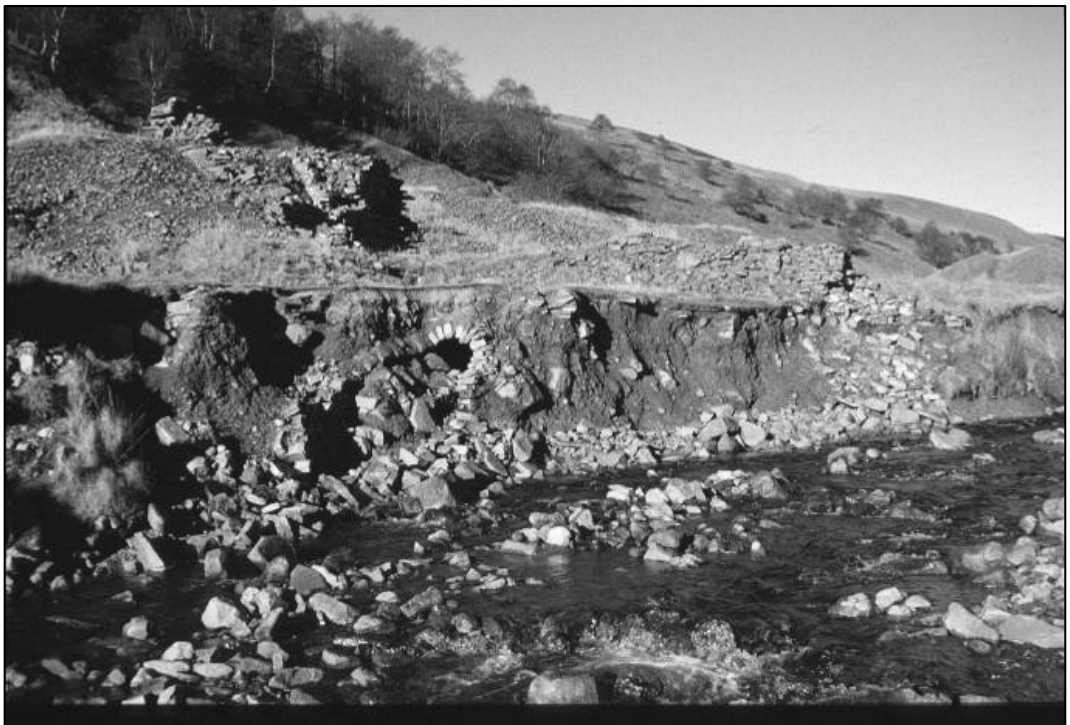
Plate 2: General view of eroding structures on Sir Francis Mine dressing floor, looking NW, January 2000 (YDNPA GG554).
