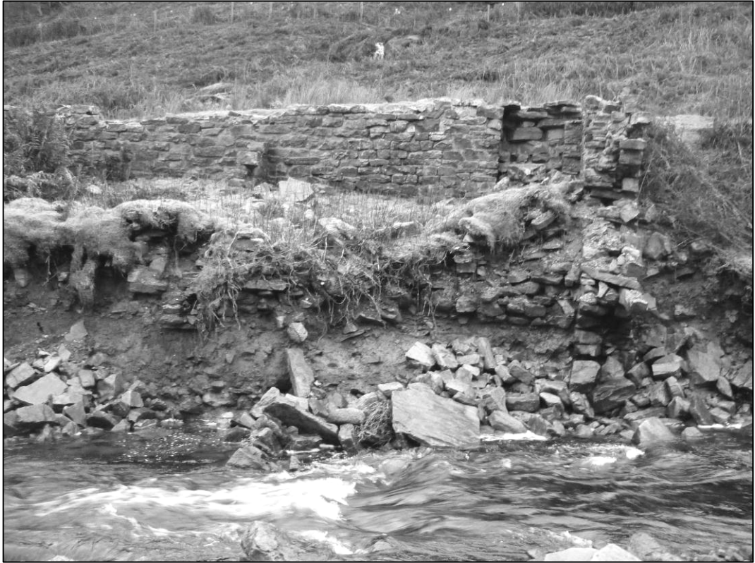
Plate 7: Area 1 Mineshop, looking W, December 2009 (photo 2/804).
