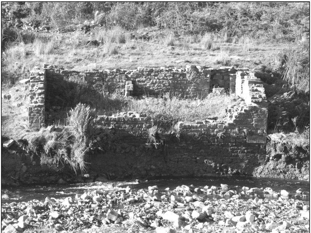
Plate 8: Area 1 Mineshop, after consolidation and prior to erosion, looking E, October 2005 (YDNP IMG 4462).
