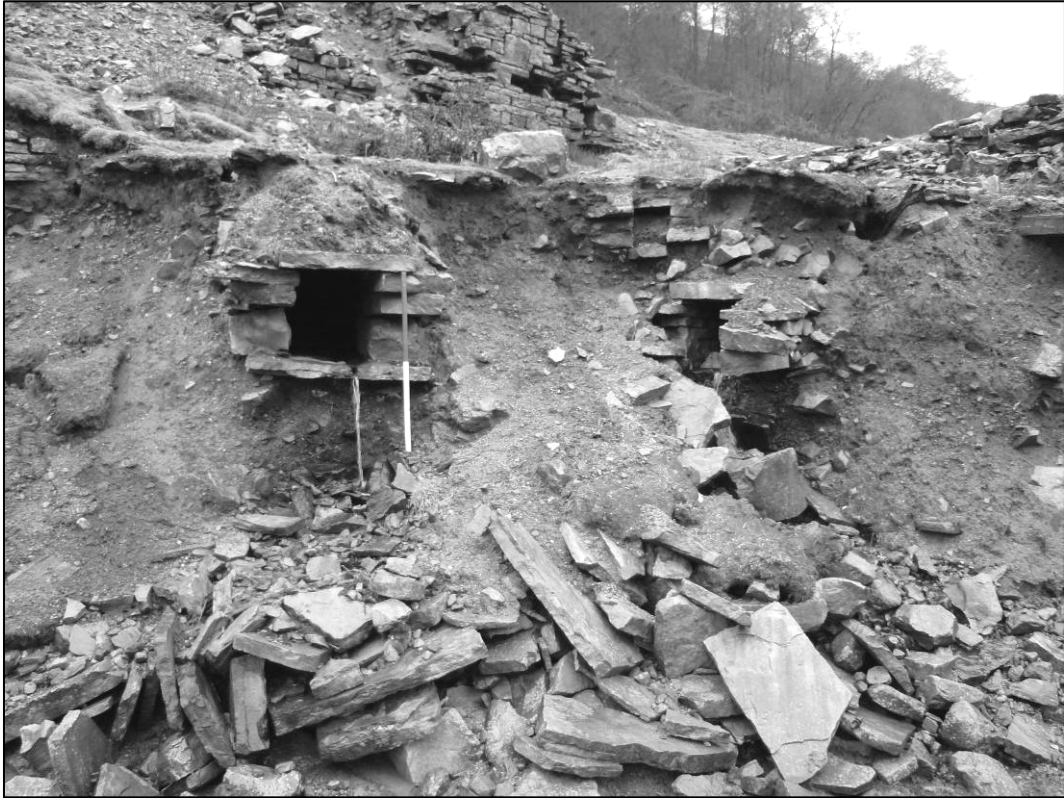
Plate 5: Culverts exposed in eroding bank of Sir Francis Mine dressing floor, looking NW, December 2009 (photo 2/776).
