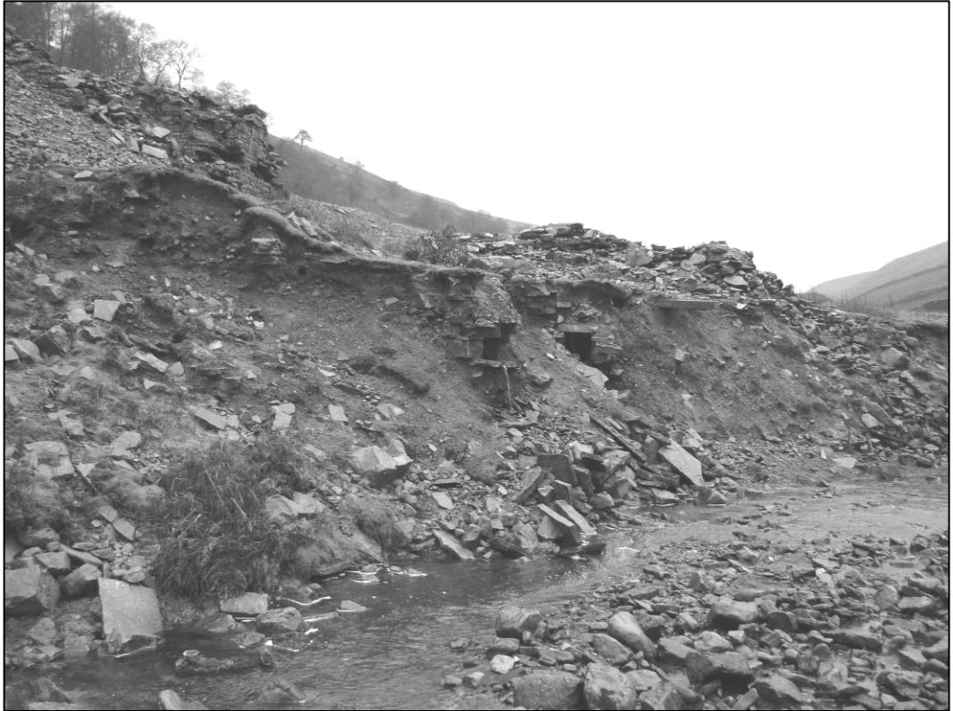
Plate 3: General view of eroding structures on Sir Francis Mine dressing floor, looking NW, December 2009 (photo 2/770).
