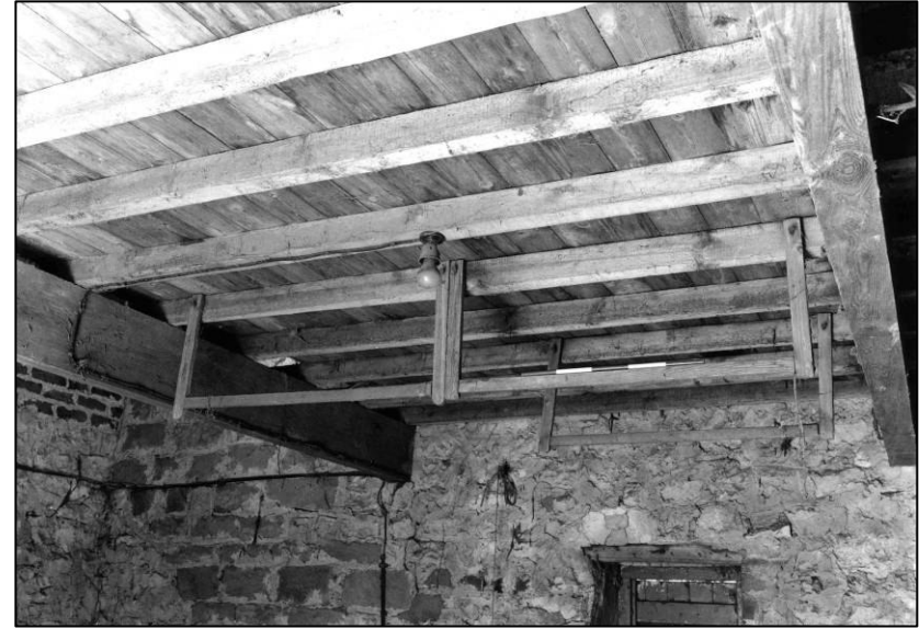
Plate 38: Granary: central bay of 1F N cell, frames in joists, looking SE (photo 3/5).
