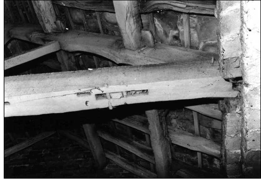
Plate 42: Granary: 2F pigeon loft, roof truss soffit, looking E (photo 4/18).
