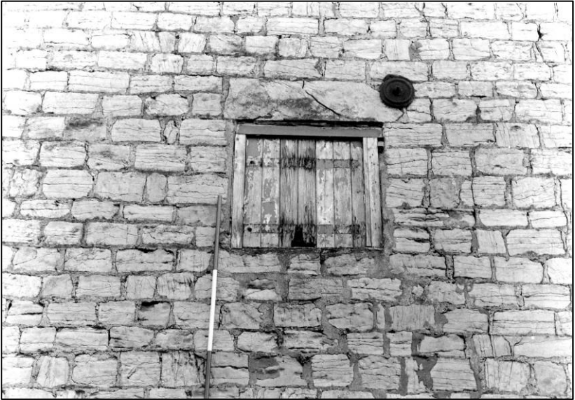
Plate 6: Granary: W elevation, typical 1F window with shutter, looking S (photo 1/13).
