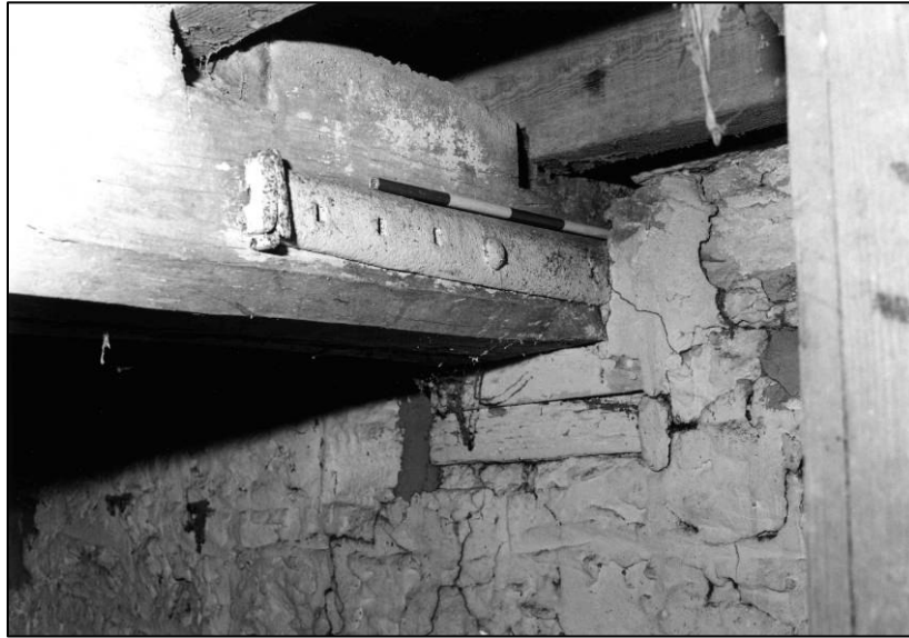
Plate 17: Granary: GF S cell, brace to ceiling beam, looking S (photo 1/8).
