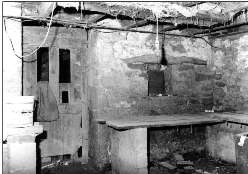
Plate 79: Barn: interior of W end, looking SW (photo 6/13).
