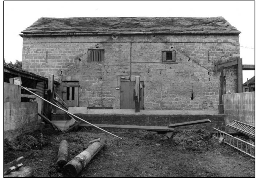
Plate 76: Barn: S elevation after demolition of adjoining shed, looking N (photo 9/3).
