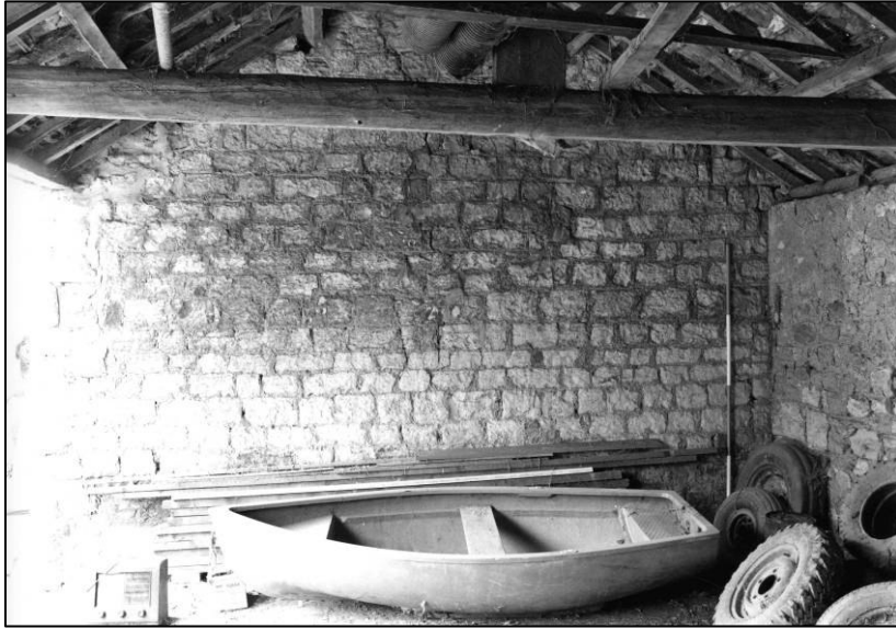
Plate 65: Cart shed: interior, looking SW (photo 5/11).
