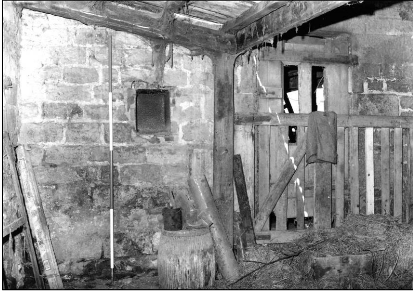
Plate 73: Barn: W end of S elevation, looking NE (photo 6/1).
