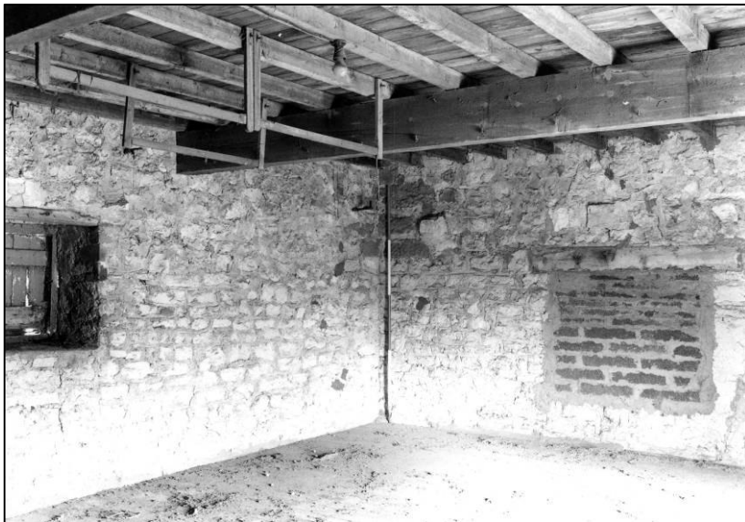
Plate 35: Granary: 1F N cell, looking N (photo 2/18).
