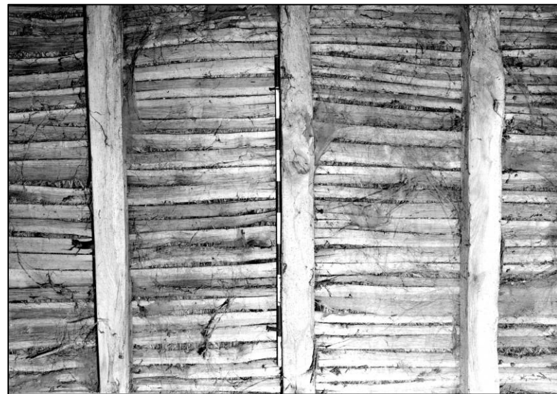
Plate 31: Granary: 1F S cell, detail of split lath and lime-ash floor to pigeon loft, looking SE (photo 2/8).
