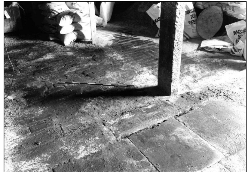
Plate 80: Barn: flagged and brick flooring, looking NW (photo 6/15).
