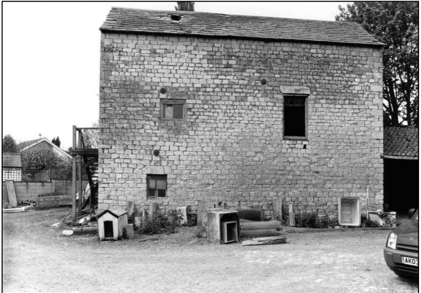
Plate 8: Granary: E elevation, looking NW (photo 5/6).
