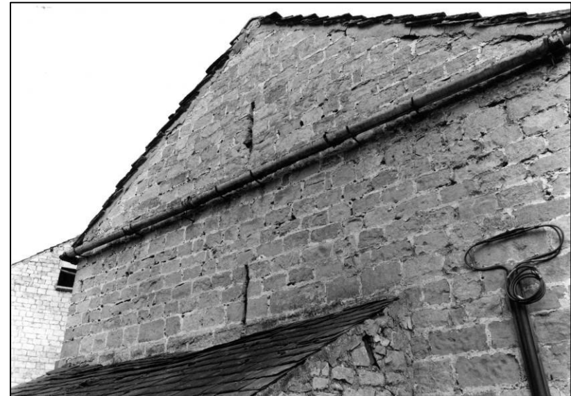
Plate 72: Barn: W gable over lean-to, looking NE (photo 7/11).
