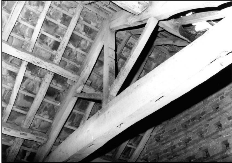
Plate 41: Granary: 2F pigeon loft, roof truss, looking W (photo 4/17).
