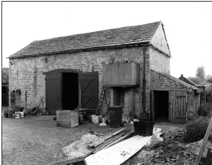
Plate 71: Barn: N elevation, looking S (photo 7/7).
