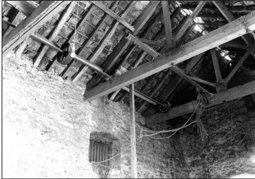
Plate 89: Barn: line shaft between trusses, looking SW (photo 6/10).
