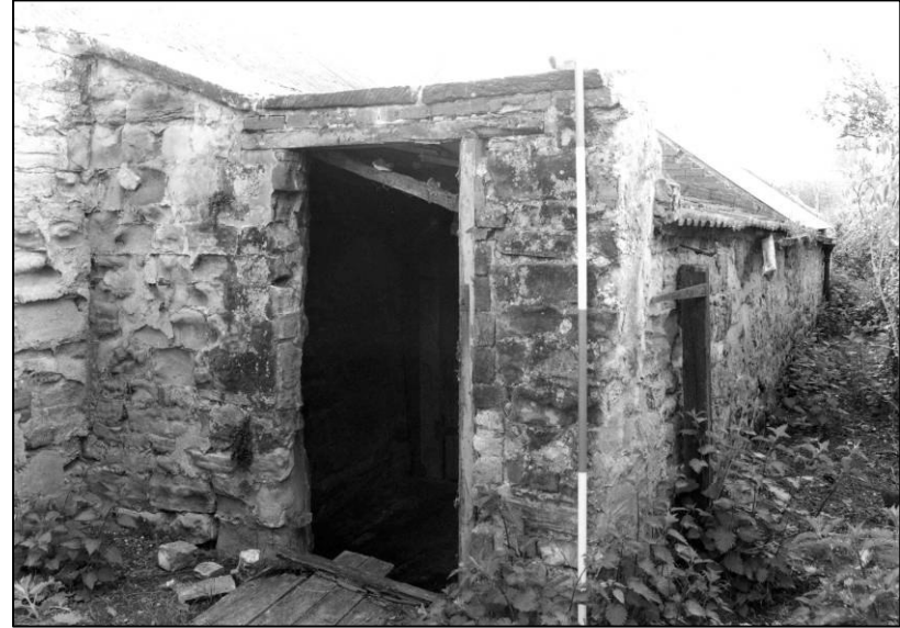
Plate 90: Workshop: door in N elevation, looking S (photo 7/9).
