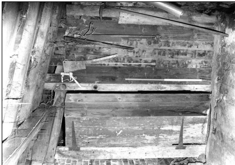
Plate 95: Workshop: interior of N cell, looking S (photo 5/16) (top to left).
