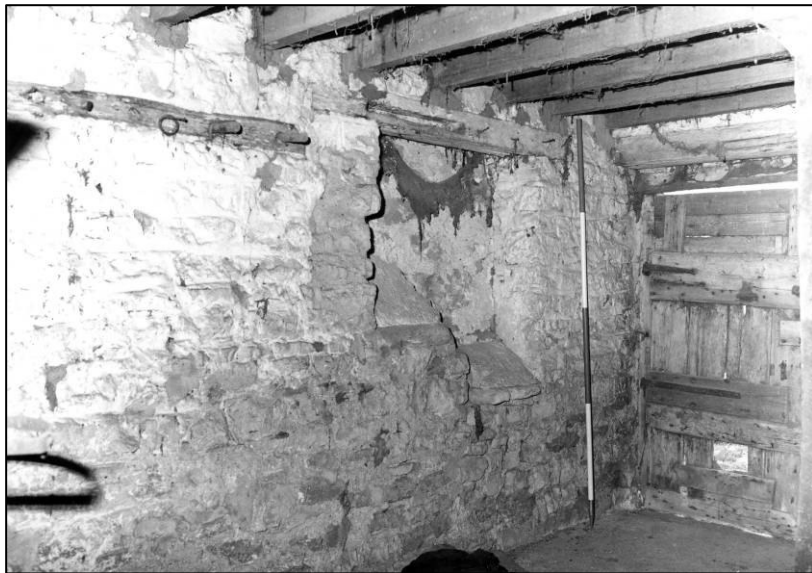
Plate 15: Granary: GF S cell, looking W (photo 1/2).
