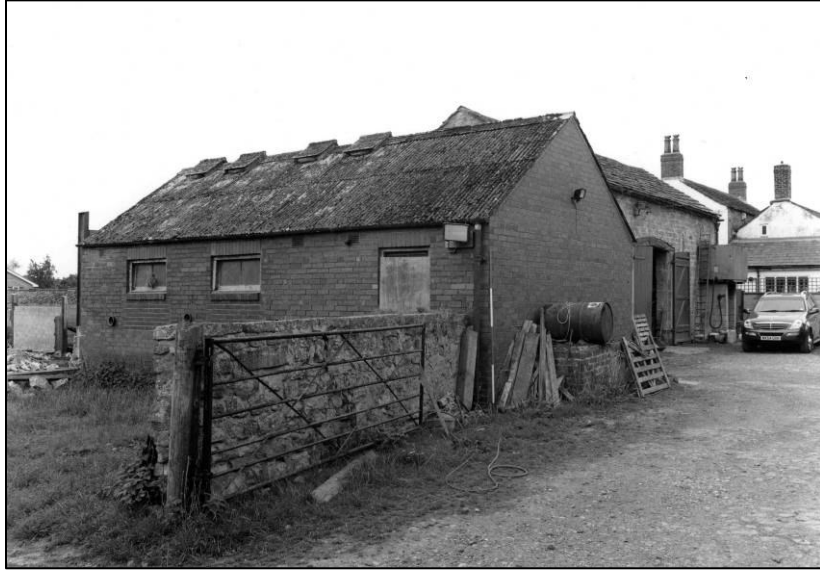
Plate 101: Dairy: E elevation & N gable, looking SW (photo 9/8).
