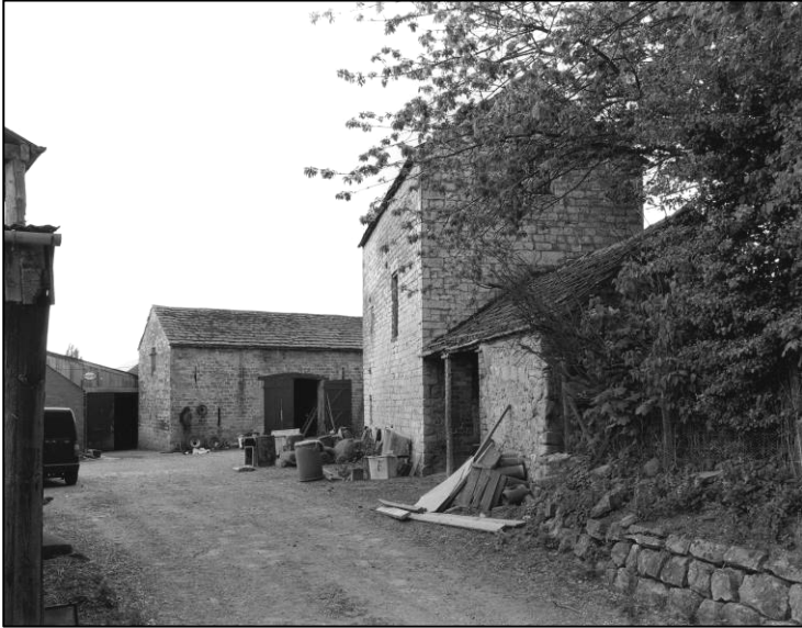
Plate 1: Granary and barn, looking S (photo 7/1).
