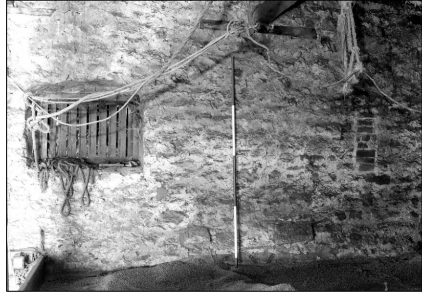
Plate 86: Barn: 1F at W end, looking S (photo 6/3).
