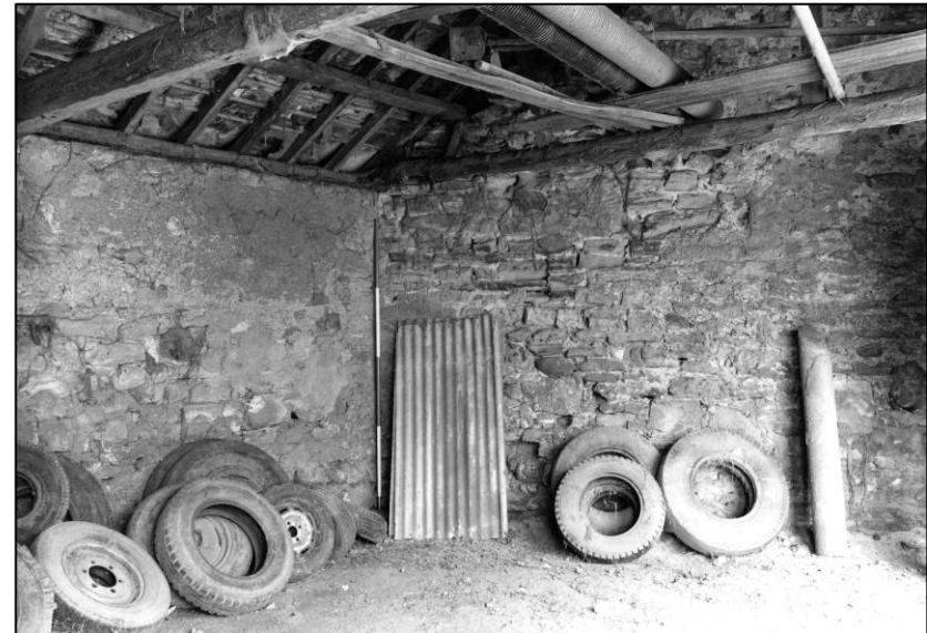
Plate 64: Cart shed: interior, looking NW (photo 5/10).
