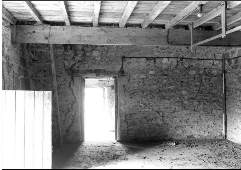
Plate 37: Granary: 1F N cell, looking SW (photo 3/1).
