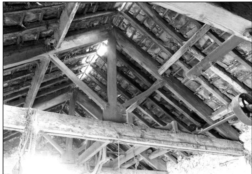
Plate 87: Barn: typical roof truss, looking SE (photo 6/6).
