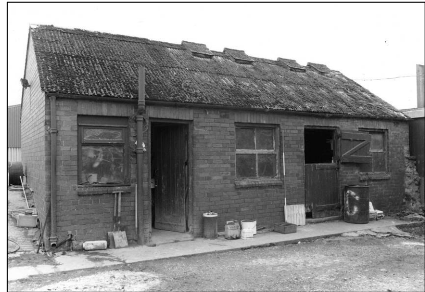
Plate 100: Dairy: W elevation, looking E (photo 9/10).
