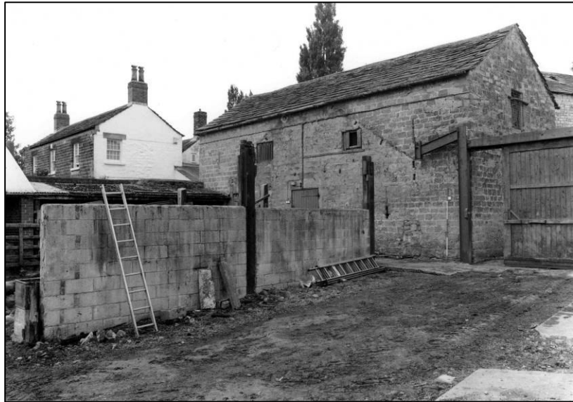
Plate 75: Barn: S elevation after demolition of adjoining shed, looking NW (photo 9/2).
