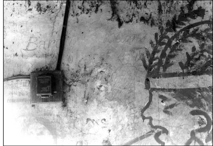
Plate 26: Granary: 1F S cell, graffiti to S wall, looking SW (photo 2/12).
