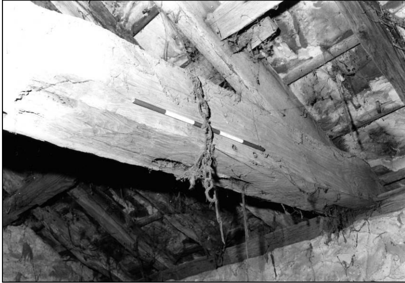
Plate 57: Granary: 2F N cell, soffit of N truss, looking E (photo 3/17).
