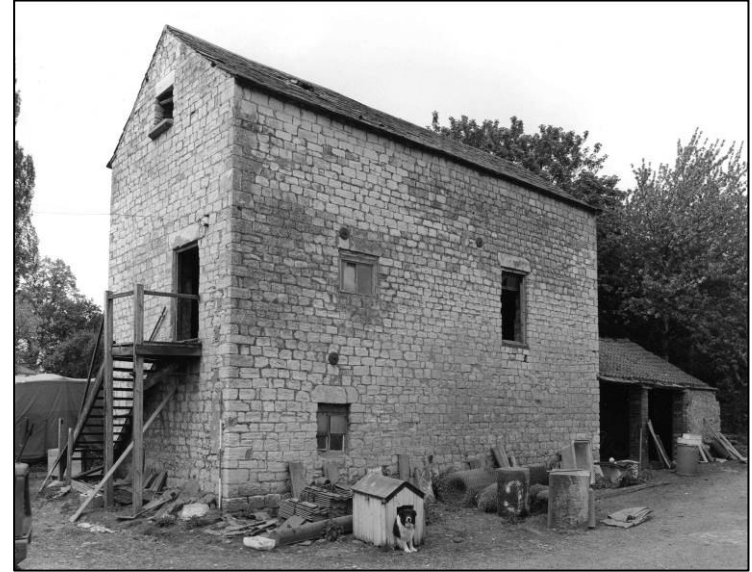
Plate 2: Granary: S & E elevations, looking N (photo 5/5).
