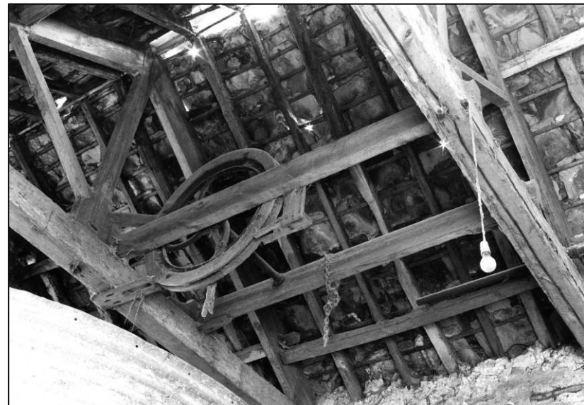
Plate 88: Barn: sack hoist over E part, looking SE (photo 6/9).
