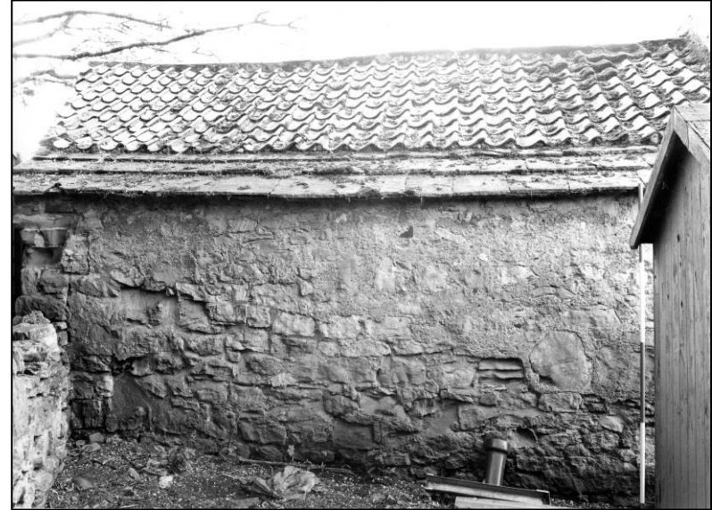
Plate 62: Cart shed: W elevation, looking SE (photo 5/3).
