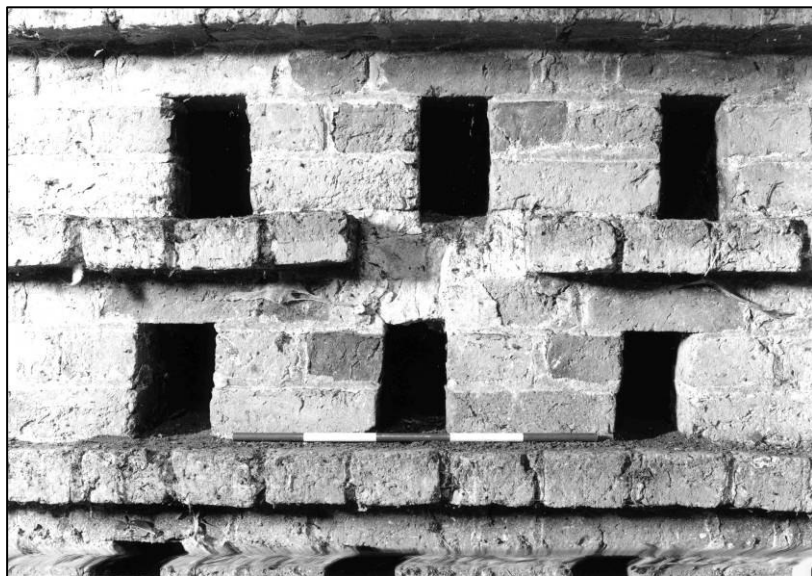
Plate 45: Granary: 2F pigeon loft, typical arrangement of boxes in S wall, looking W (photo 4/13).
