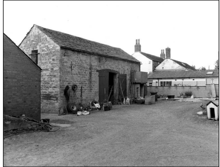
Plate 66: Barn: N elevation, looking SW (photo 7/3).
