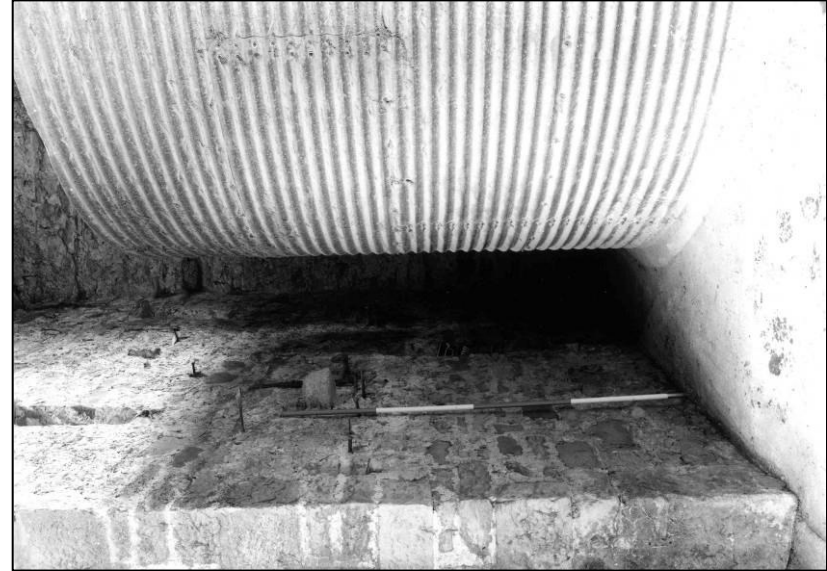
Plate 82: Barn: interior, looking E (photo 6/17) (top to left).
