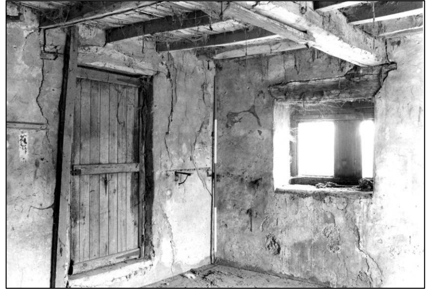
Plate 30: Granary: 1F S cell, looking E (photo 2/4).
