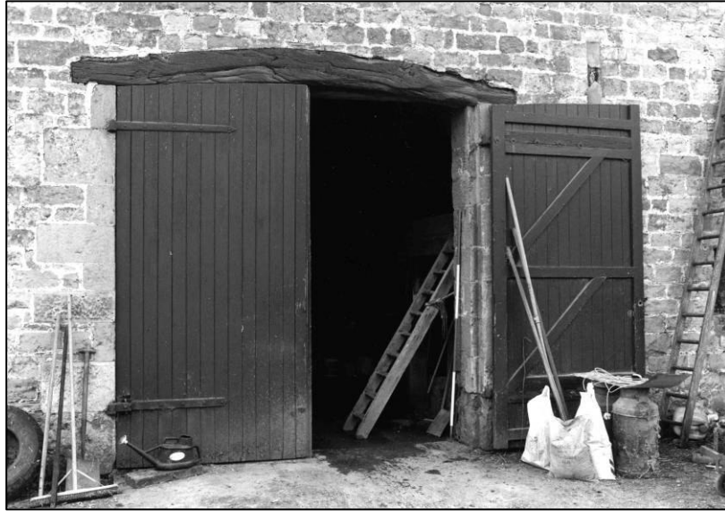
Plate 69: Barn: doorway in N elevation, looking S (photo 7/6).
