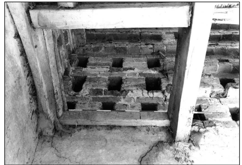
Plate 32: Granary: 1F S cell, former trap to pigeon loft, looking SW (photo 2/10).
