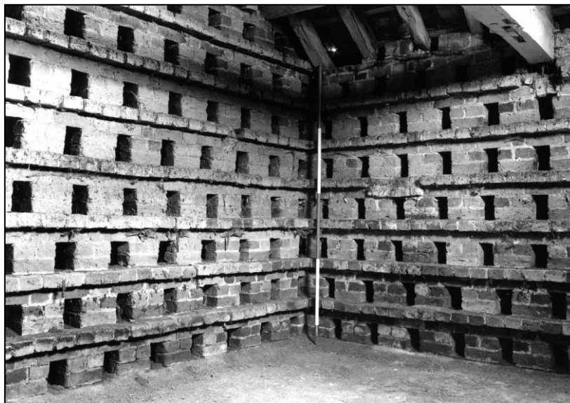
Plate 51: Granary: 2F pigeon loft, looking E (photo 4/5).
