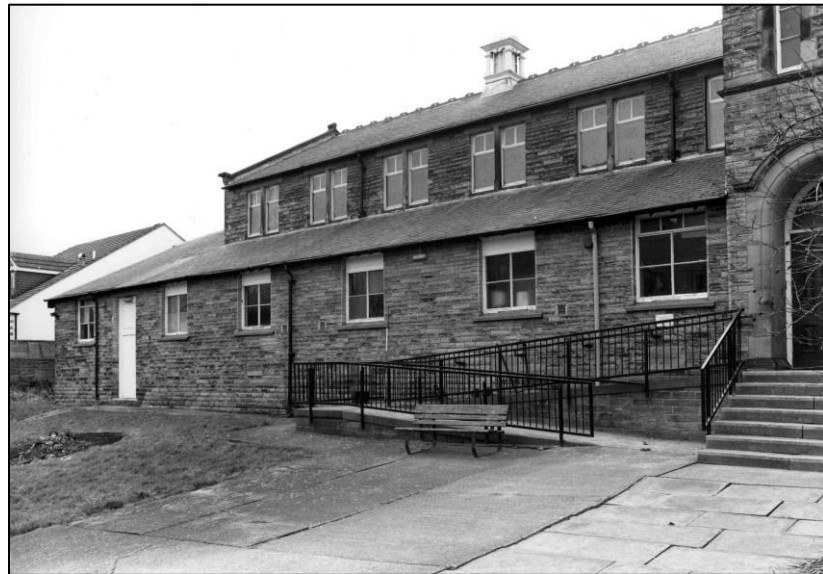
Plate 103: School: exterior, S side, looking NW (photo 8/12).
