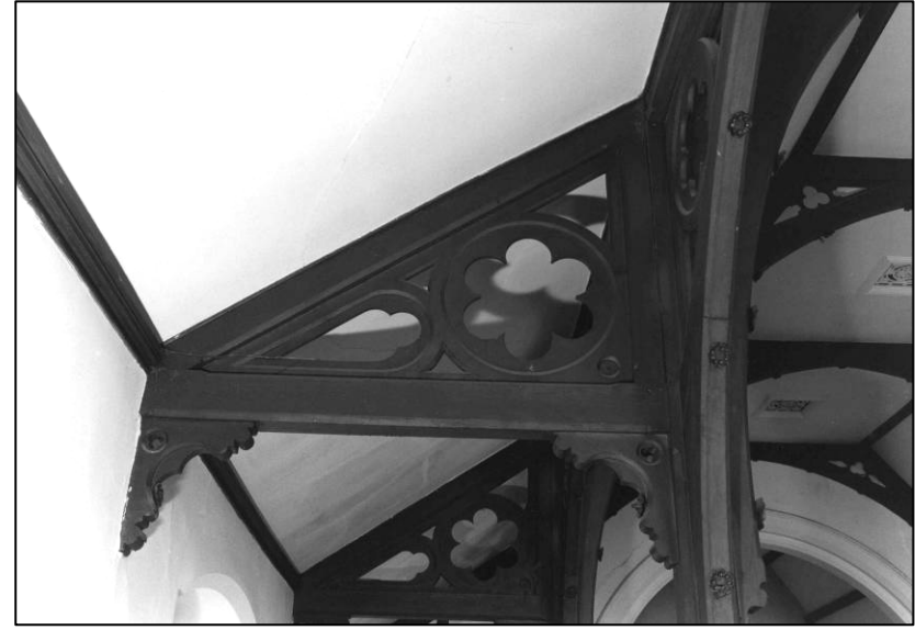
Plate 98: Church: 1F gallery, typical cusped half-truss to sides (W side), looking N (photo 4/12).
