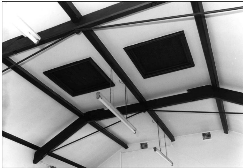
Plate 131: School: GF, band room ceiling, looking N (photo 12/15).
