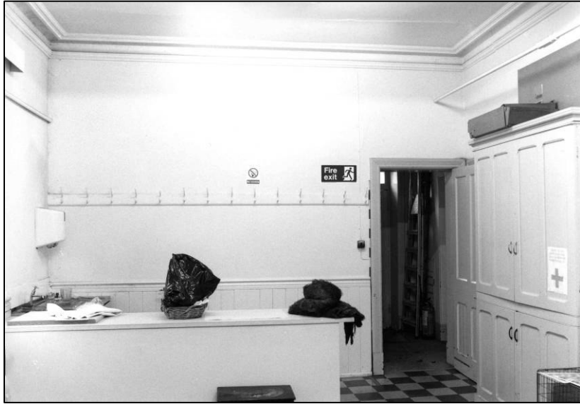
Plate 73: Church: meeting room (former band room), looking E (photo 9/18).
