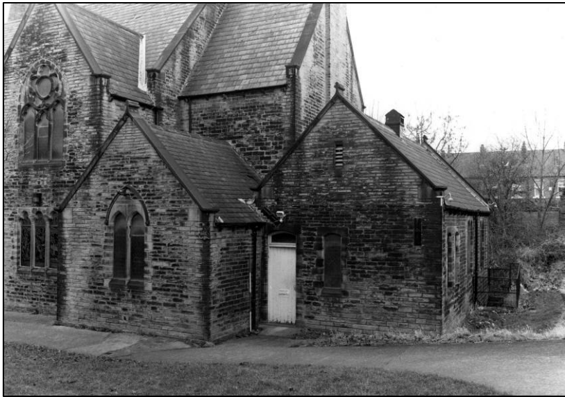
Plate 19: Church: exterior, NE corner, looking SW (photo 8/4).
