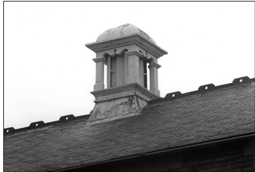
Plate 104: School: exterior, roof lantern/vent to main hall, looking N (photo 8/16).
