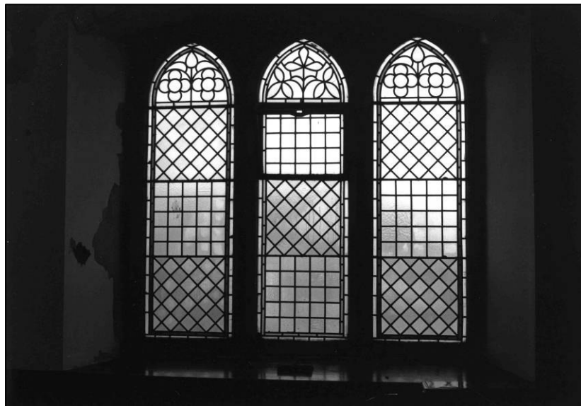
Plate 87: Church: 1F gallery, typical window on W side, looking W (photo 3/9).
