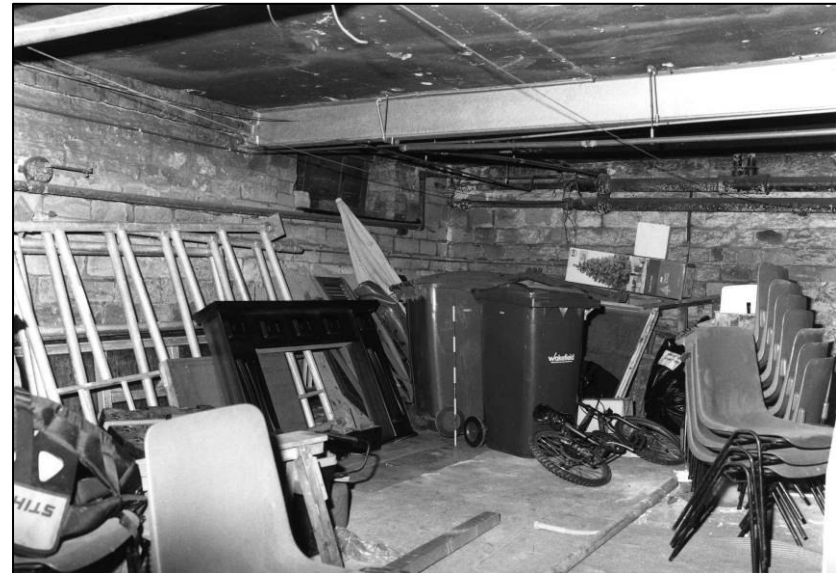
Plate 108: School: heating basement beneath SE end, looking N (photo 9/9).
