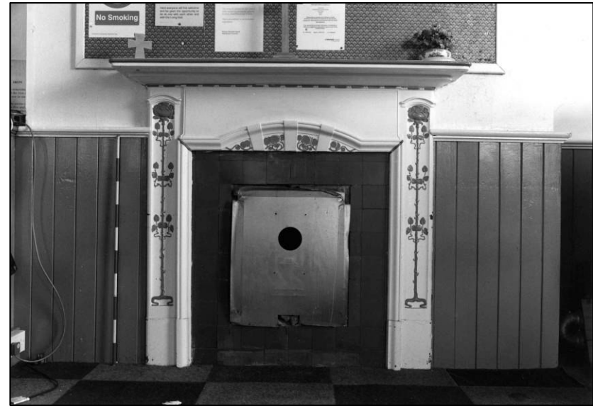
Plate 132: School: GF, band room, fireplace, looking E (photo 12/10).
