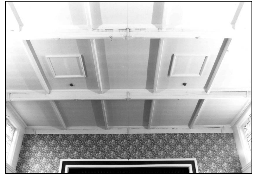
Plate 148: School: GF main hall, panelled ceiling, looking W (photo 11/7).
