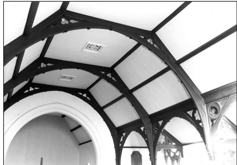
Plate 96: Church: roof trusses, looking NE (photo 4/15).
