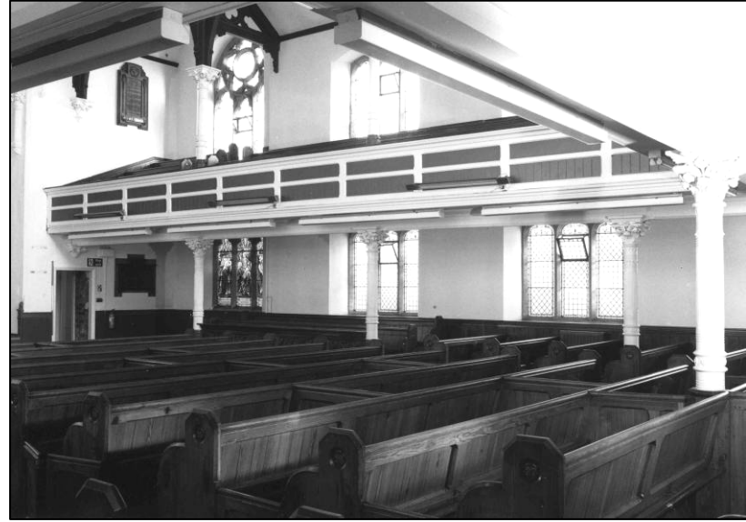
Plate 50: Church: GF and 1F gallery, looking NE (photo 2/8).
