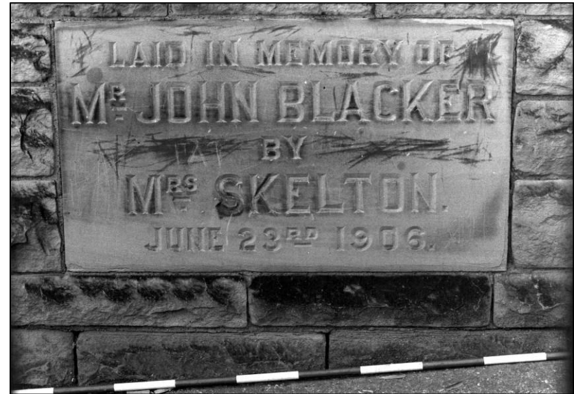
Plate 114: School: 'Blacker' foundation stone, S elevation of main hall, looking N (photo 13/11).
