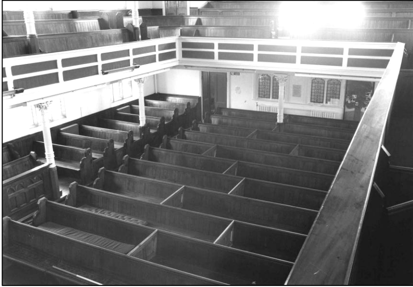
Plate 57: Church: GF and 1F gallery, looking SW (photo 6/3).
