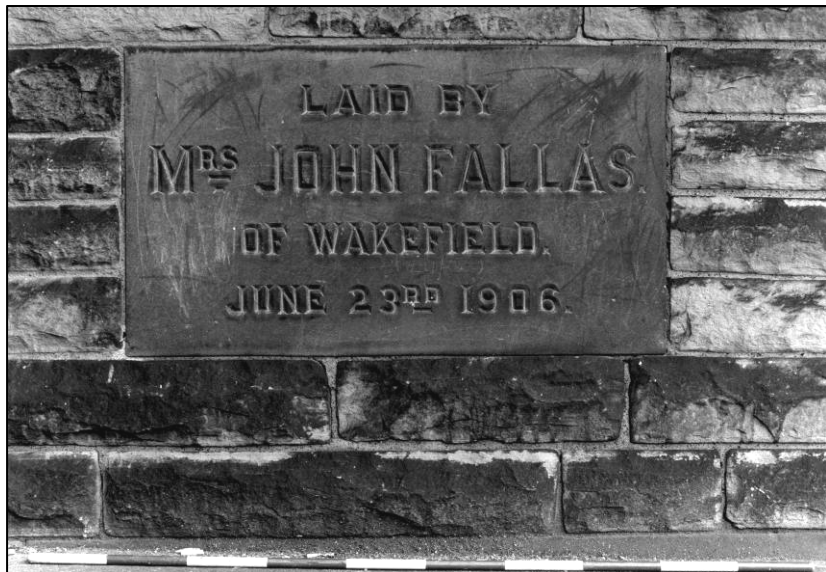
Plate 115: School: 'Fallas' foundation stone, W elevation of band room, looking E (photo 13/12).
