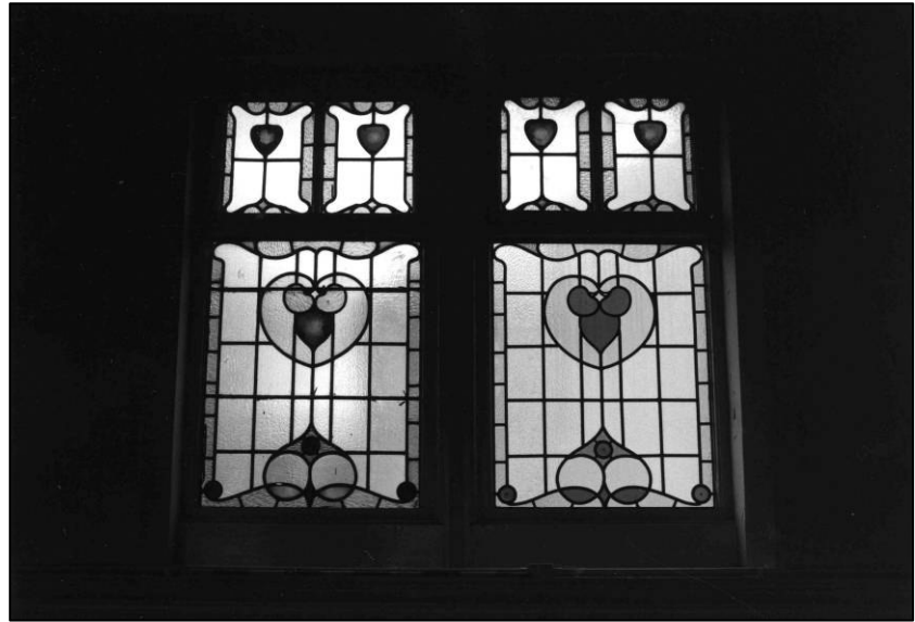
Plate 156: School: 1F gallery, typical window (NE corner), looking N (photo 11/12).
