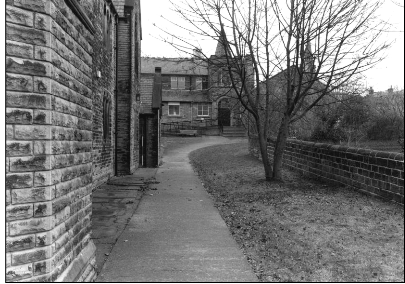
Plate 102: View to School along E side of church, looking N (photo 7/18).
