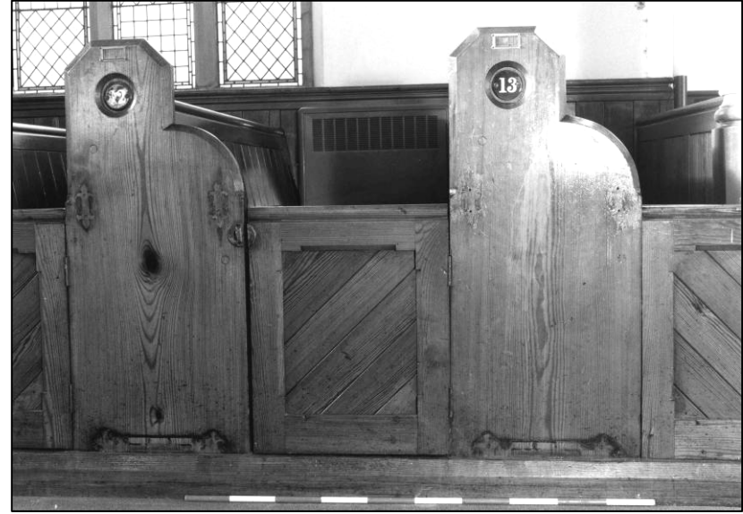
Plate 58: Church: GF, typical pew numbering in W aisle, looking W (photo 2/11).
