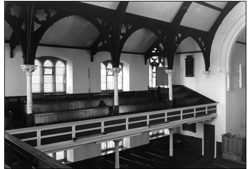
Plate 80: Church: 1F gallery, W side, looking NW (photo 3/17).
