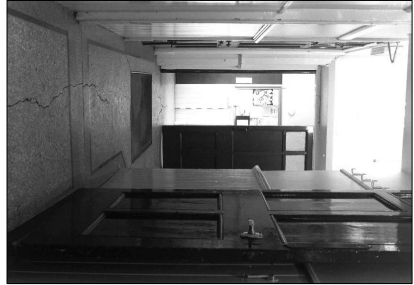
Plate 126: School: GF entrance lobby, looking W (photo 12/8) (top to right).
