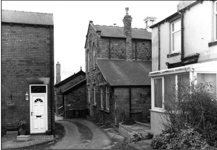
Plate 121: School: exterior, E side, looking S (photo 9/4).
