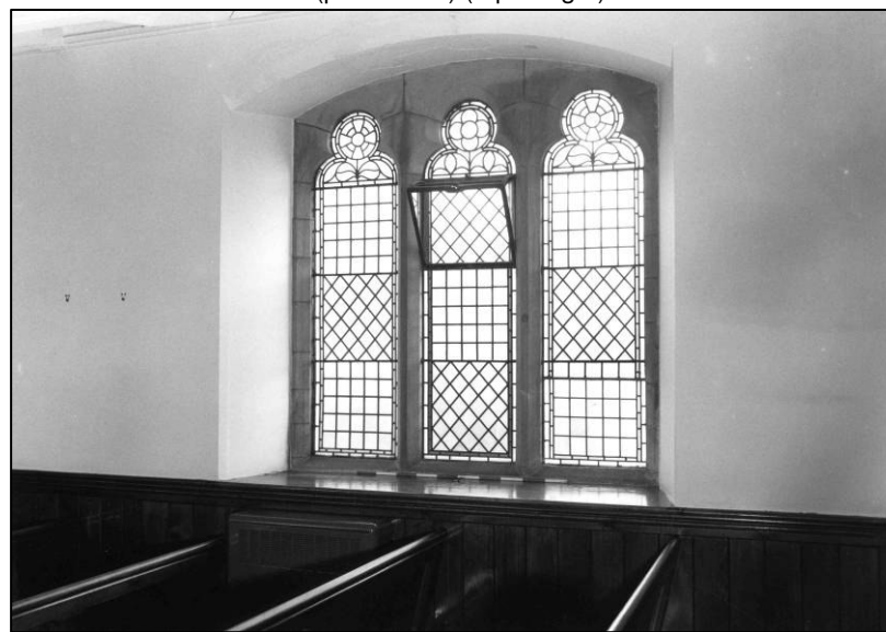
Plate 64: Church: GF, typical window in E aisle, looking E (photo 2/5).
