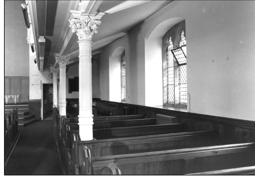
Plate 54: Church: GF, E aisle, looking N (photo 2/4).
