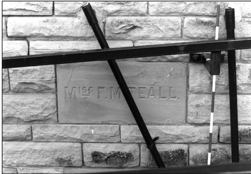
Plate 113: School: 'Teall' foundation stone, S elevation of main hall, looking N (photo 13/10).
