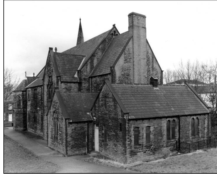
Plate 14: Church: exterior, NE corner, looking SW (photo 8/3).
