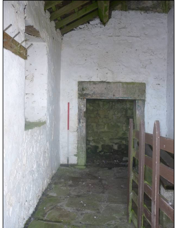
Plate 8: Fireplace in west wall of south cell, looking W.
