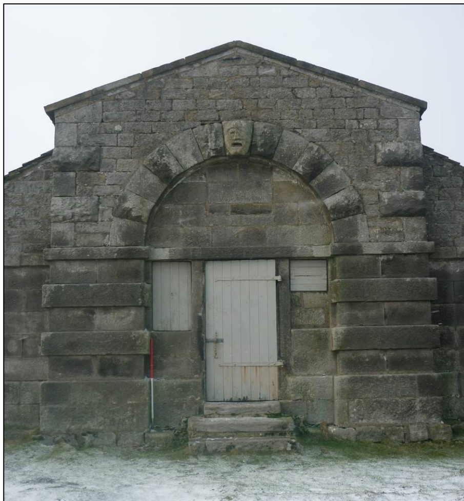
Plate 4: Detail of east elevation of central bay, looking W.
