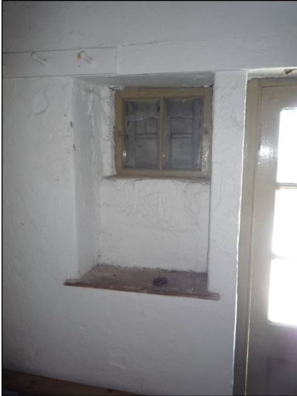
Plate 7: Partially blocked window in north-east corner of central cell, looking E.
