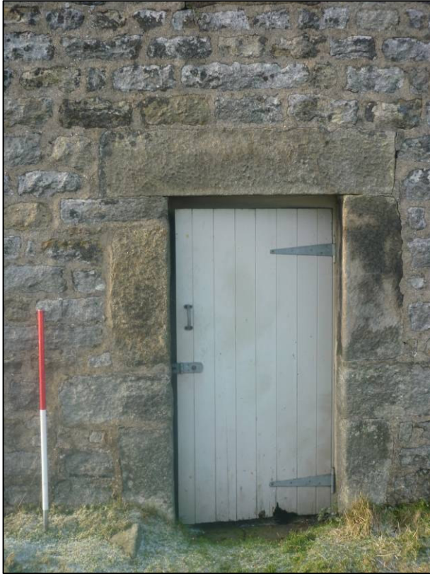
Plate 10: Door in east elevation of house, looking W.
