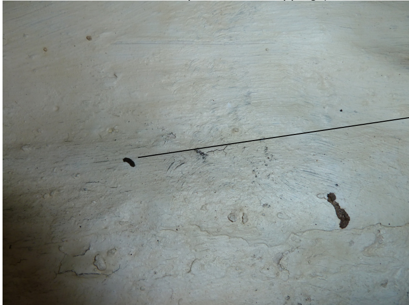
Plate 10 North room: close-up of the bat dropping (refer to Plate 9)
