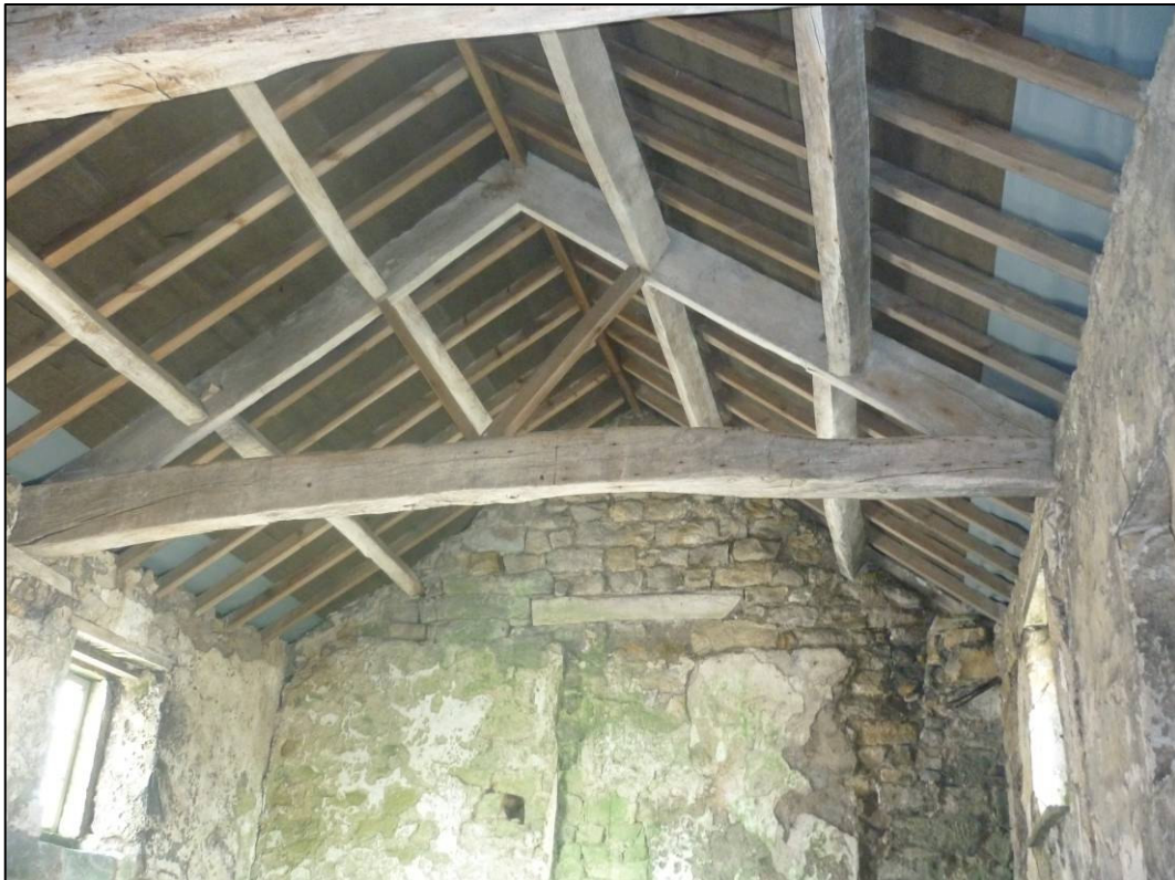
Plate 12: North roof truss in house, looking N.
