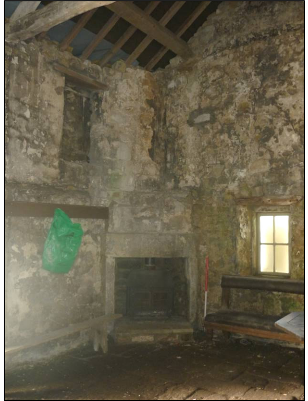
Plate 11: Fireplace in south-east corner of house, looking SE.
