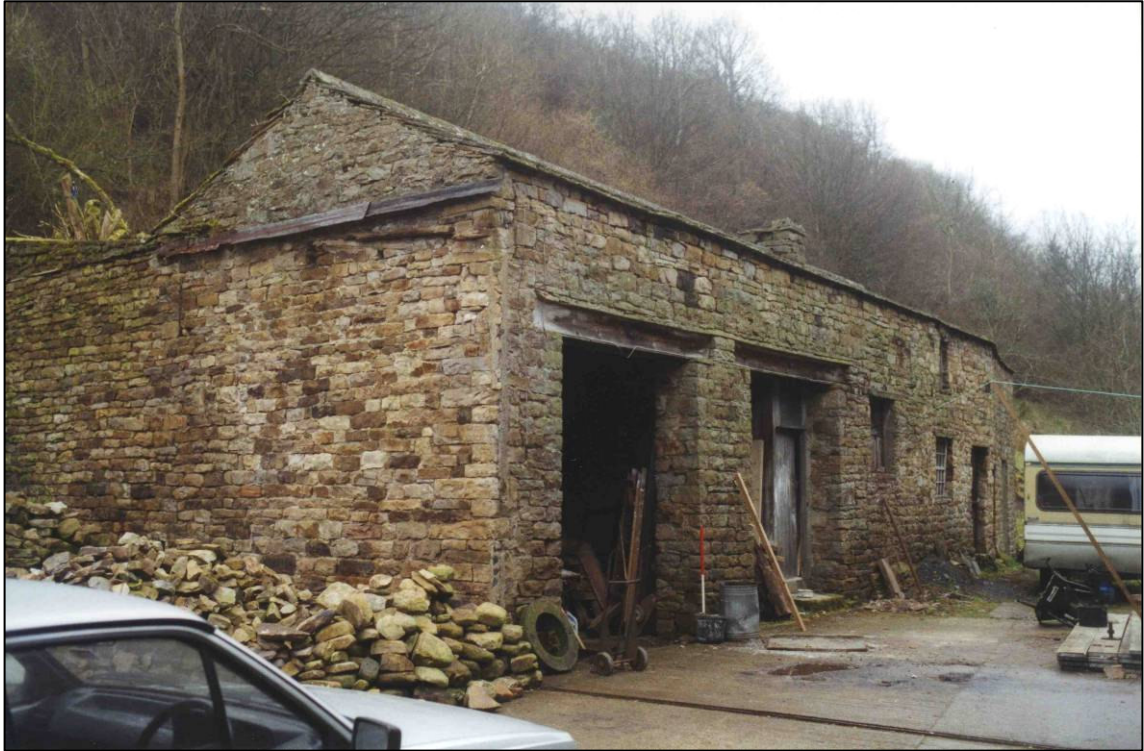
Plate 4: General view of west range, looking NW.
