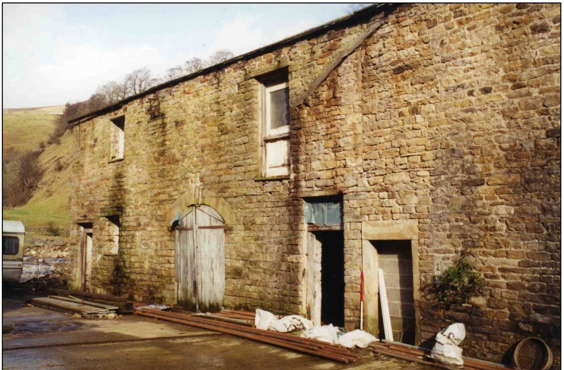
Plate 7: West elevation of east range (north end), looking E.
