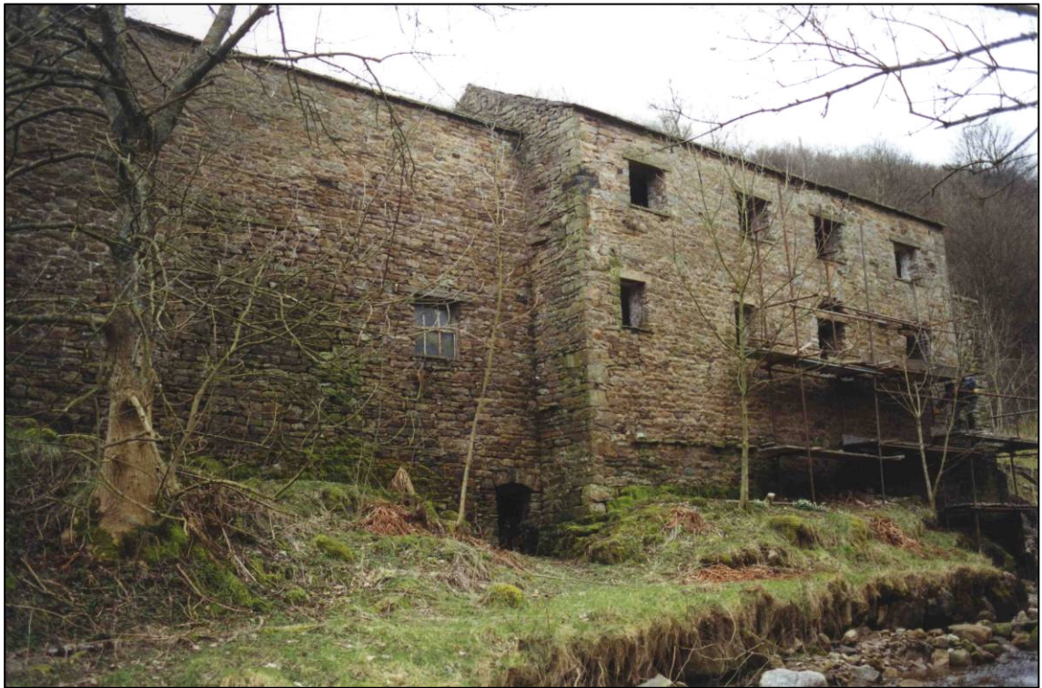
Plate 8: East elevation of east range, looking W.
