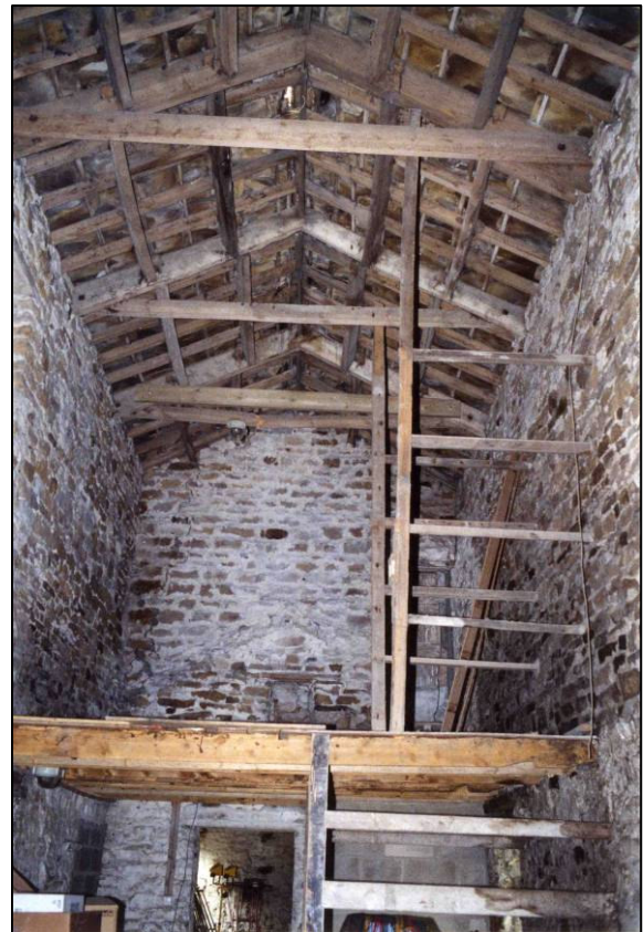
Plate 3: Interior of south end of east range, looking N.
