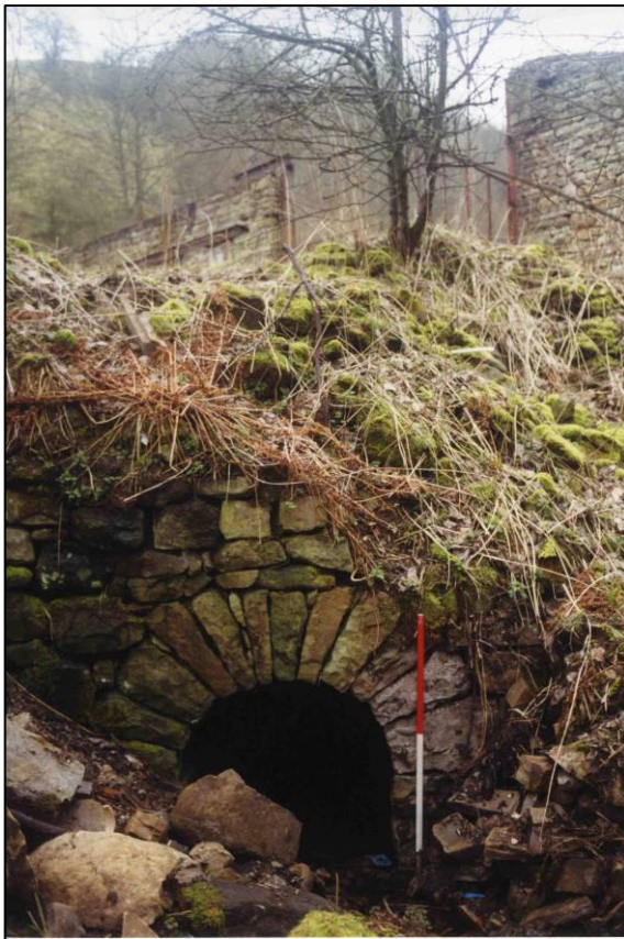
Plate 2: Culvert on east side of access track, looking NW.
