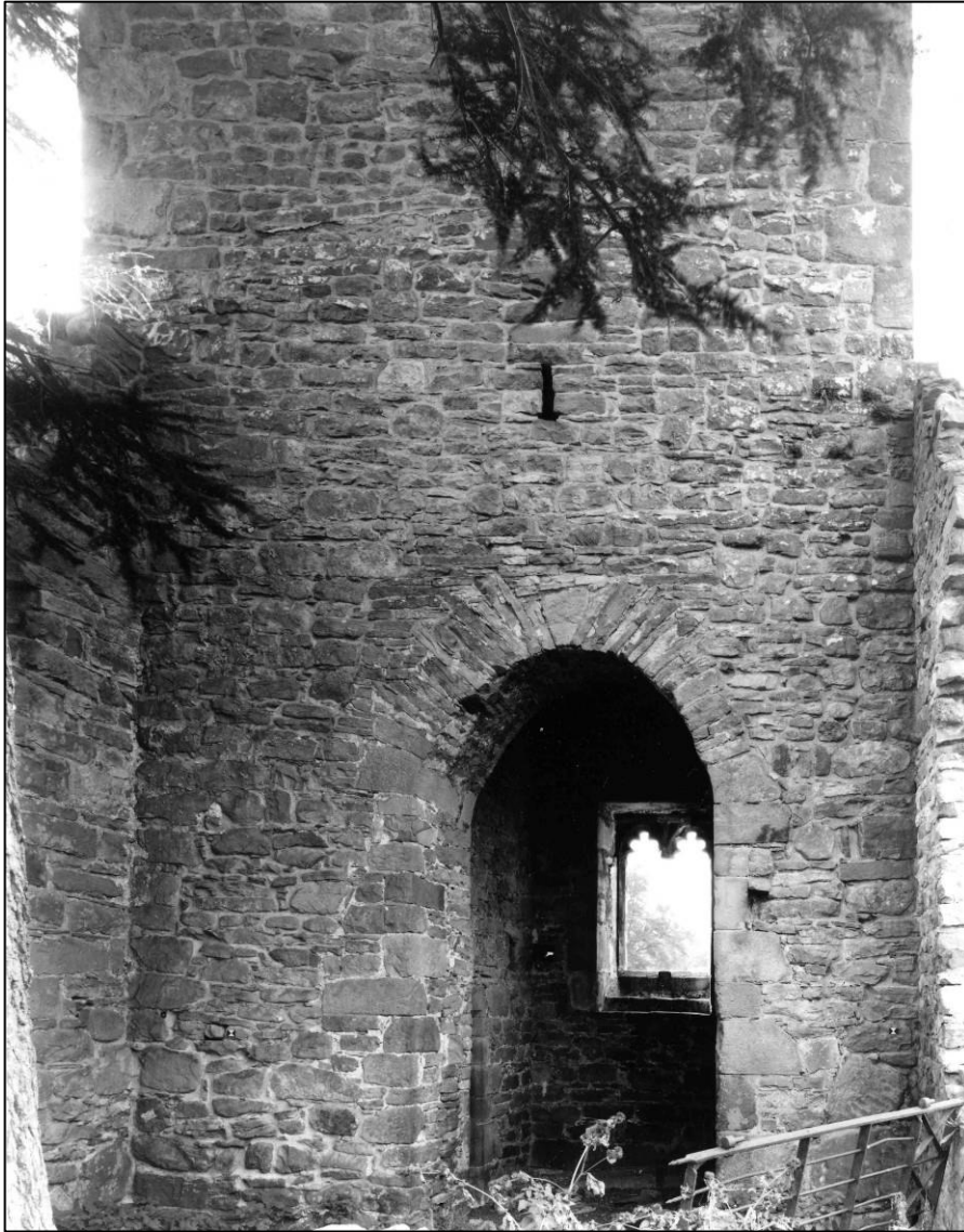
Plate 10: West external elevation of tower, looking W (photo 1/7 September 1996).
