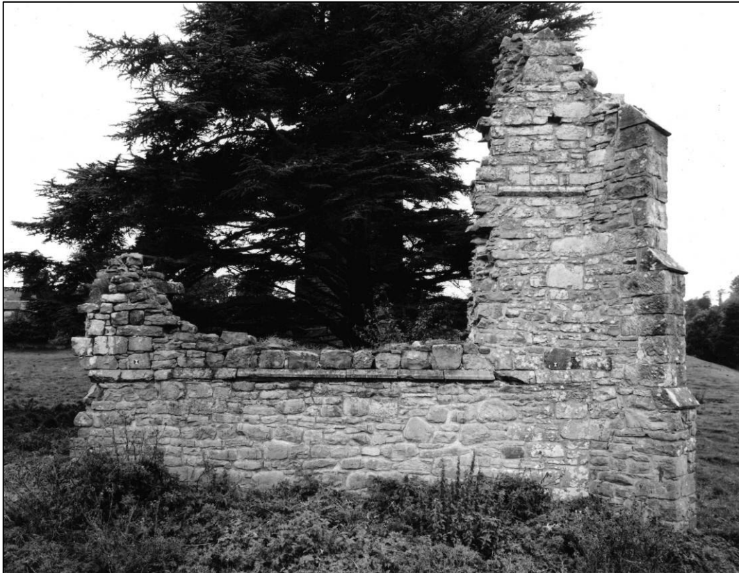
Plate 5: East external elevation of chancel, looking W (photo 2/7 September 1996).
