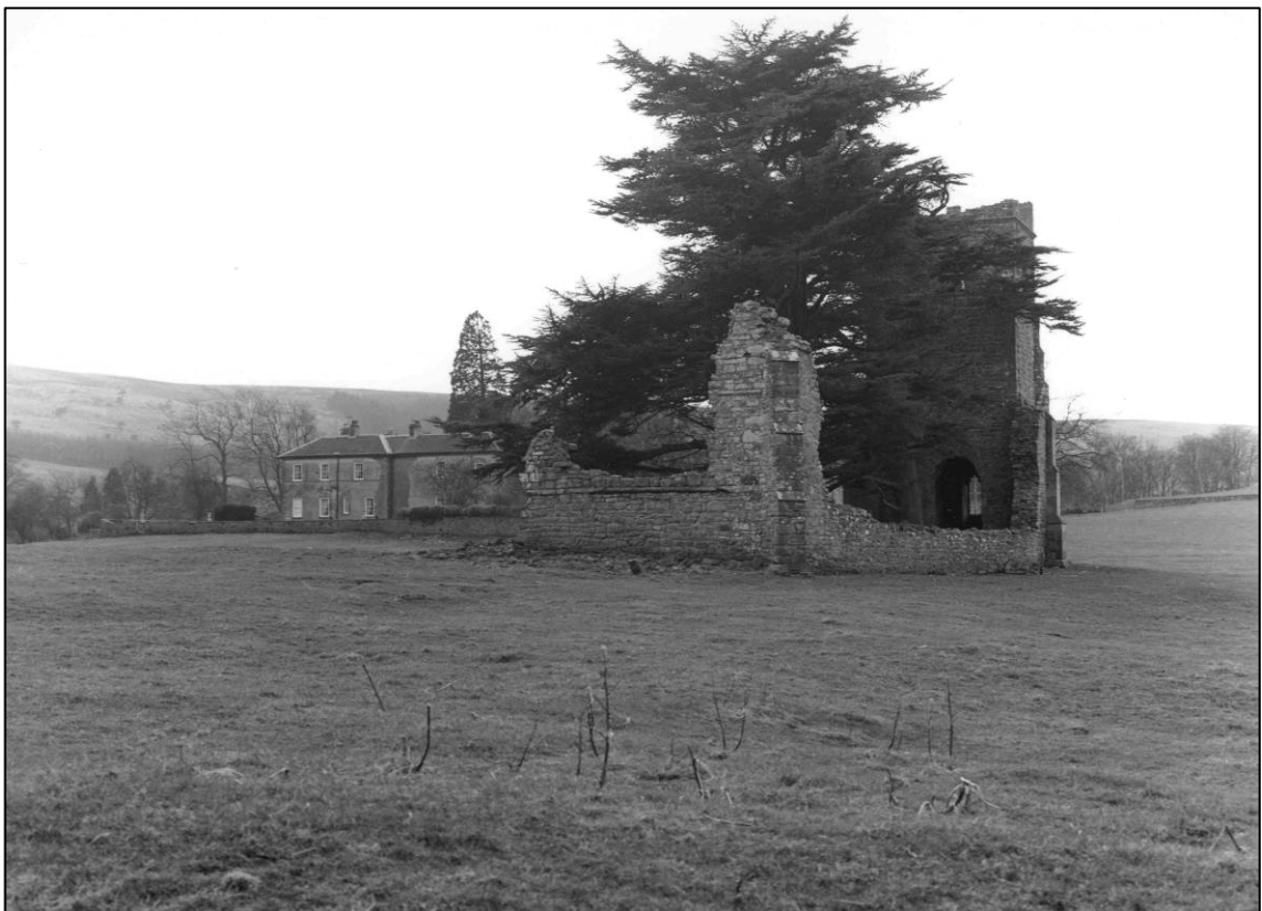
Plate 2: Ellerton Priory church, looking SW towards Ellerton Abbey (house) (February 1999).
