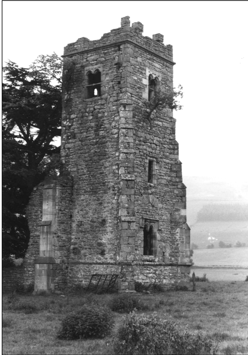
Plate 3: Church tower, looking SE (YDNP 643/15 March 1983).
