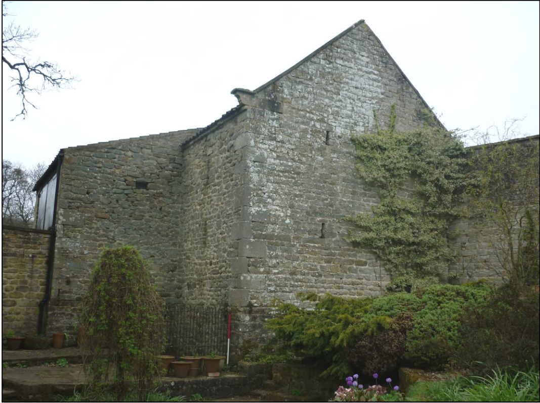
Plate 1: East end of mill range and outshot, looking NW (photo 1/85).
