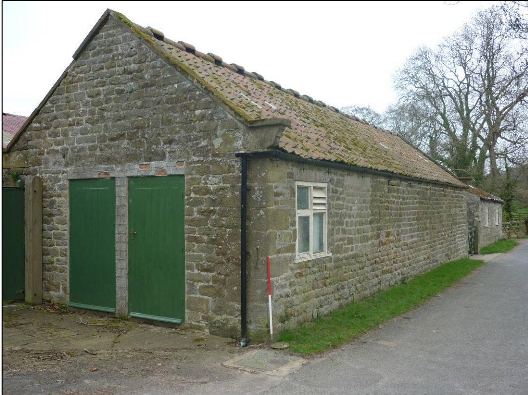
Plate 11: North gable and west elevation of byre/cow house, looking SE (photo 1/13).
