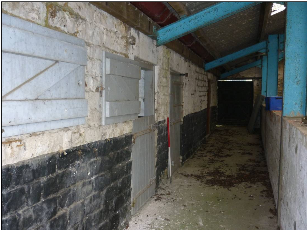
Plate 12: East elevation of byre/cow house, looking NW (photo 1/31).
