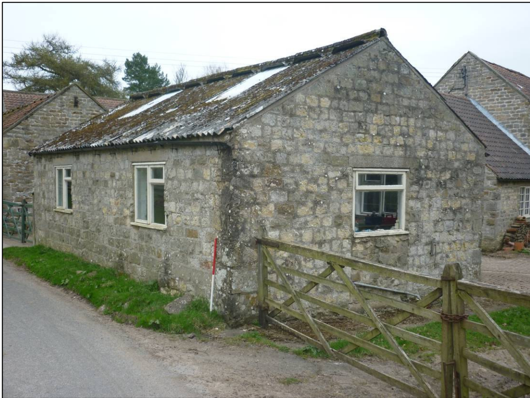
Plate 13: South gable and west elevation of dairy parlour, looking NE (1/09).
