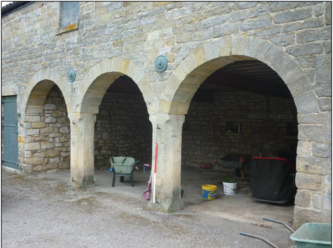
Plate 7: South elevation of cart shed, looking NW (photo 1/40).
