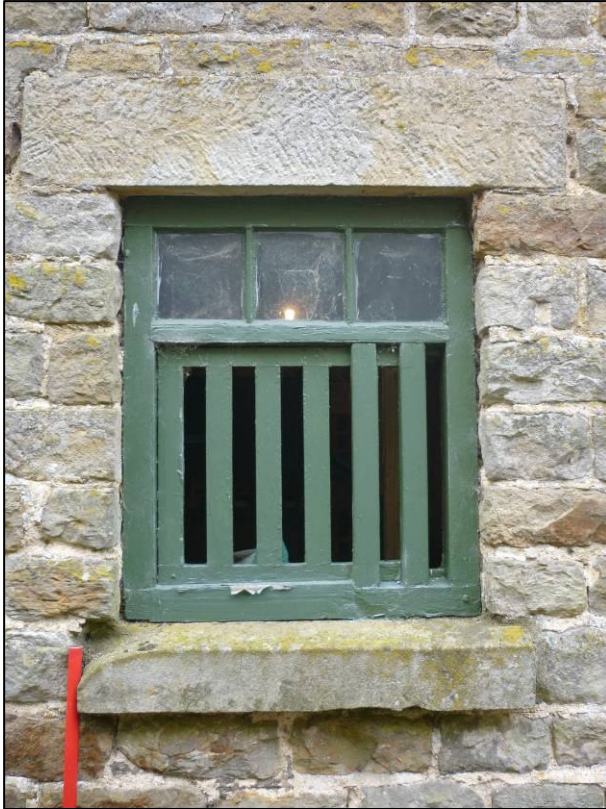
Plate 8: Open ventilated window in south elevation of stables, looking N (photo 1/54).
