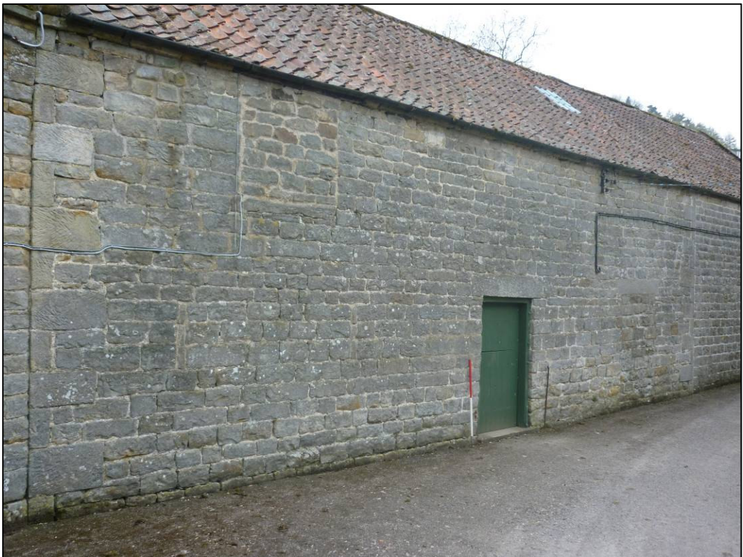
Plate 2: North elevation of east part of mill range, looking SW (photo 1/91).
