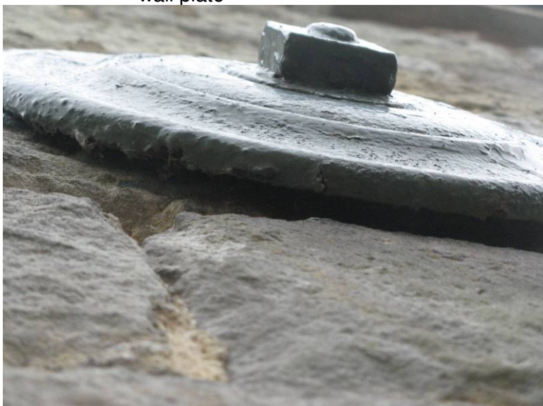
Plate 5 The Granary (south elevation) – bat recorded in the stone wall
