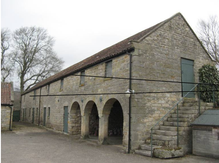
Plate 1 The Granary (south and east elevation) – bats recorded in the crevices between the fascia board and stone wall along the southern elevation
