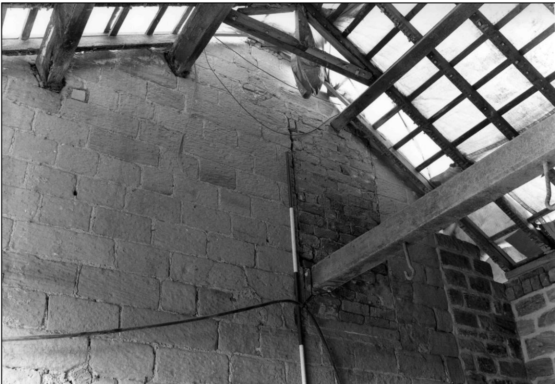
Plate 18: Upper part of north wall of north room, looking NE (photo 3/4).
