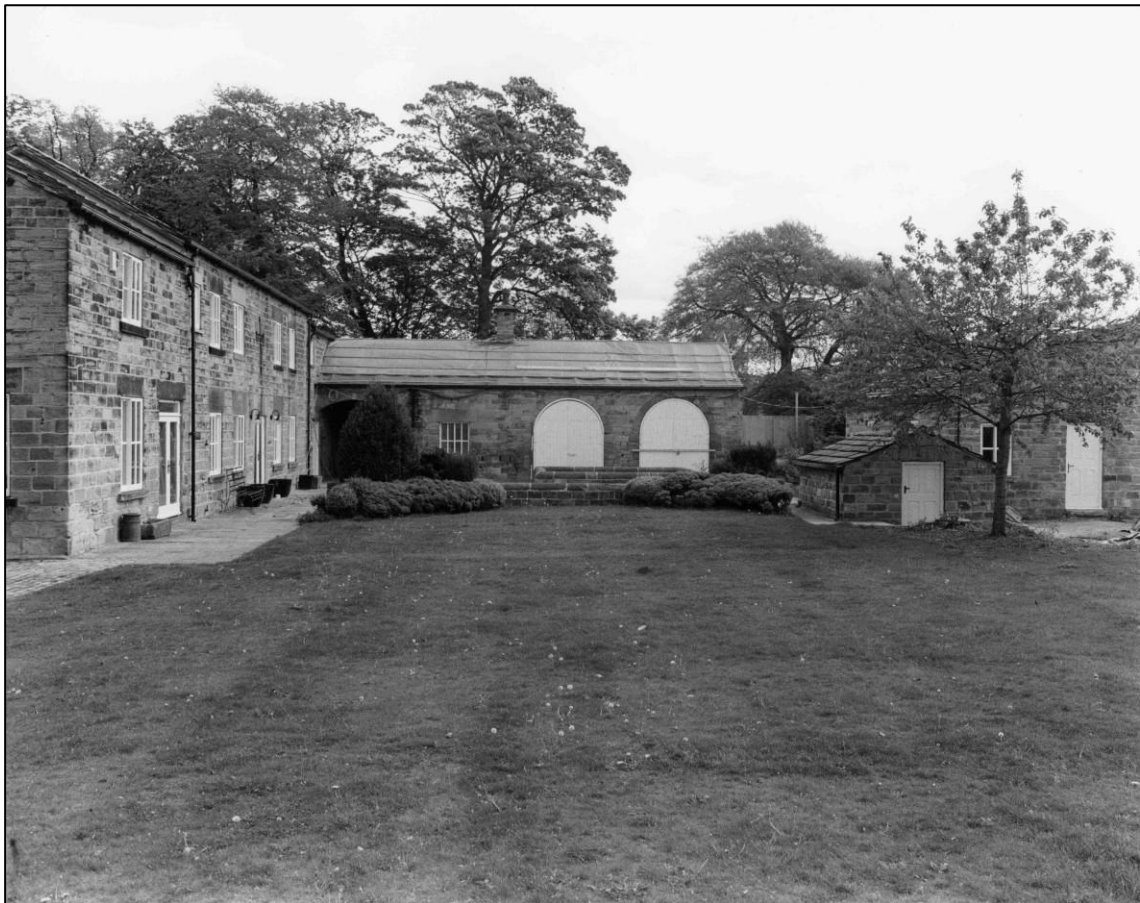
Plate 8: West external elevation, looking E (photo 4/3).
