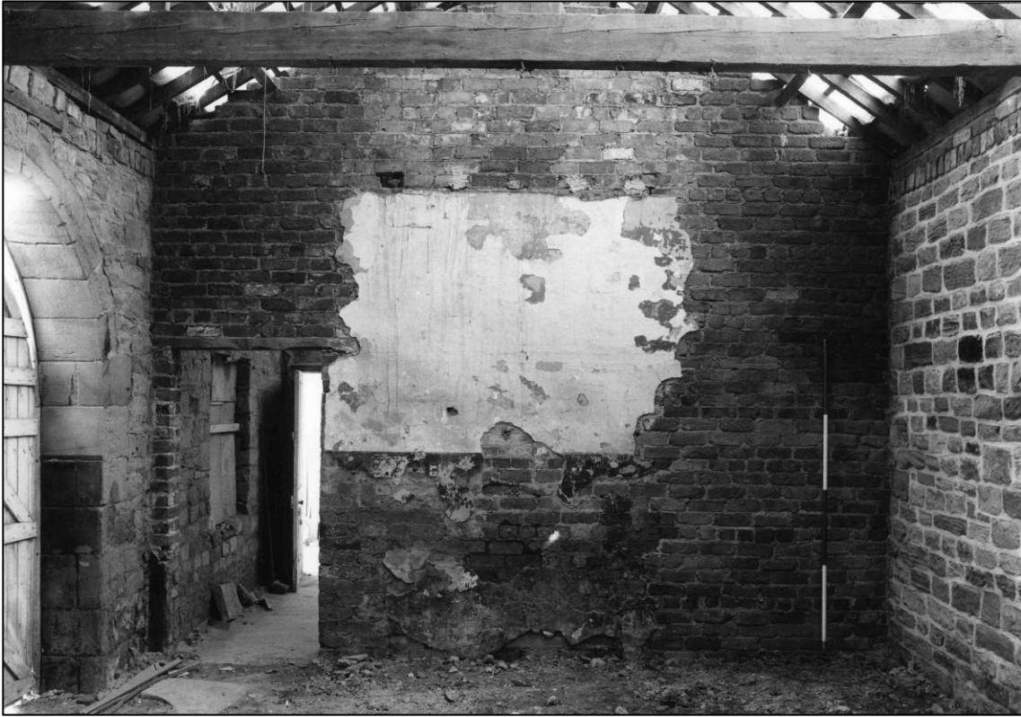
Plate 39: North wall of south room, looking N (photo 1/4).
