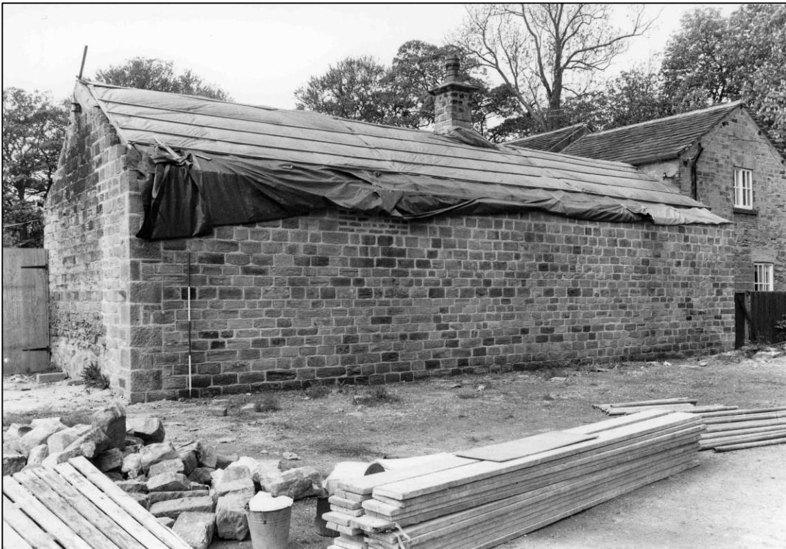
Plate 12: East external elevation, looking NW (photo 4/6).
