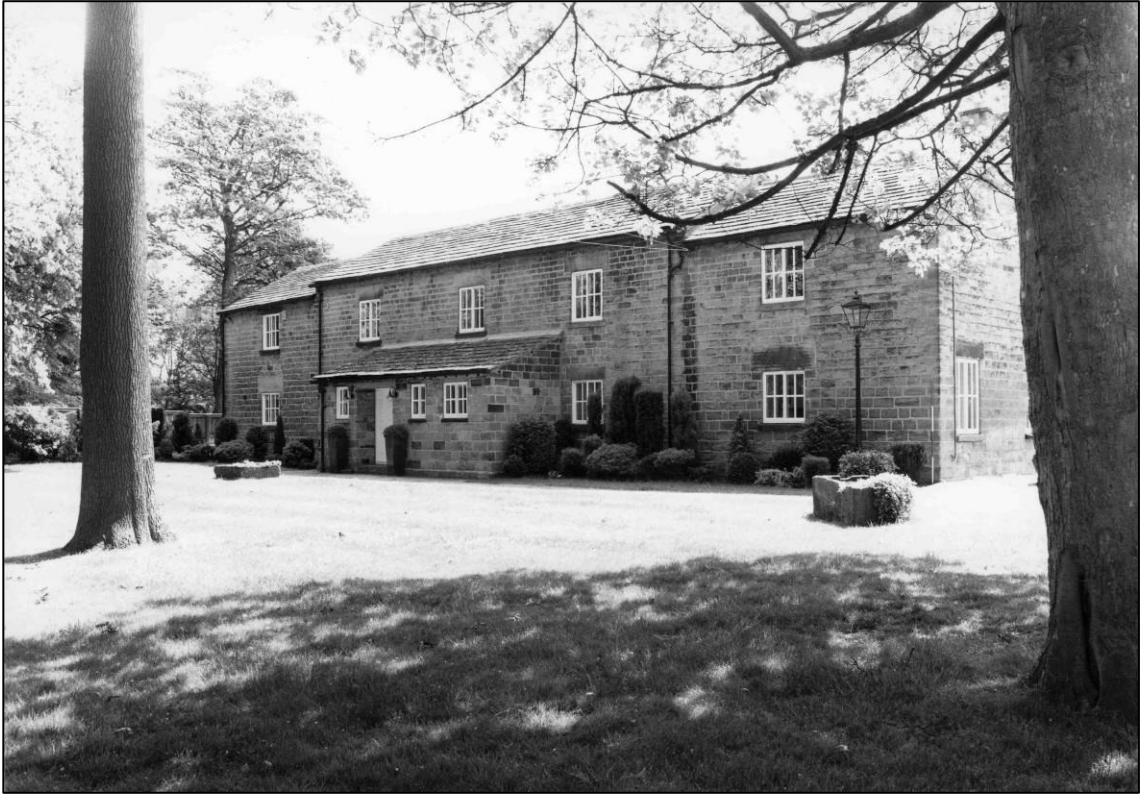
Plate 3: North elevation of north range, looking SE (photo 4/10).
