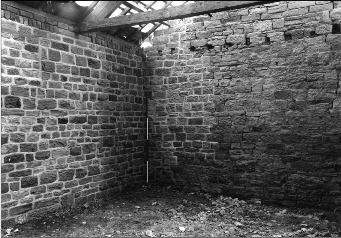
Plate 41: South-east corner of south room, looking SE (photo 1/6).
