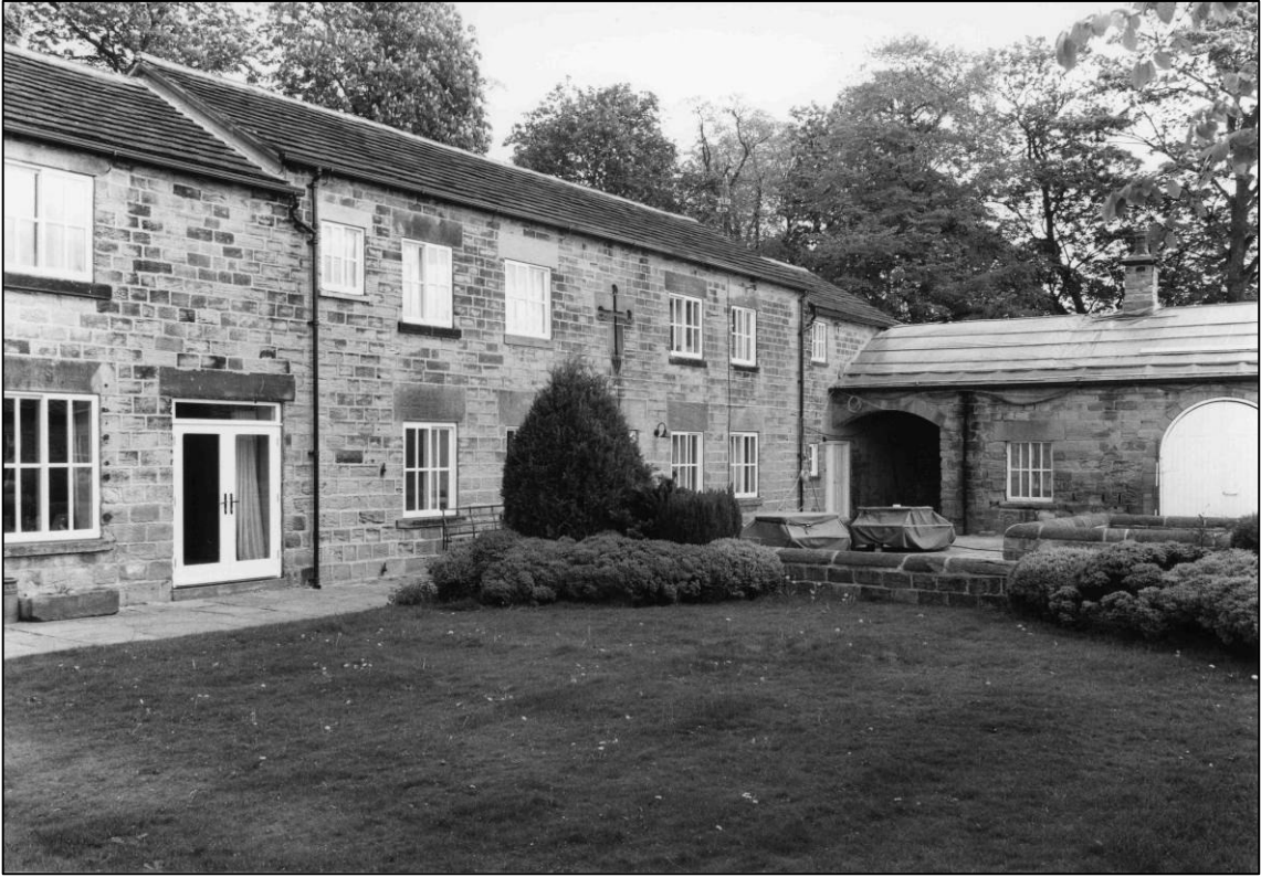
Plate 1: North range and coach house, looking NE (photo 4/1).
