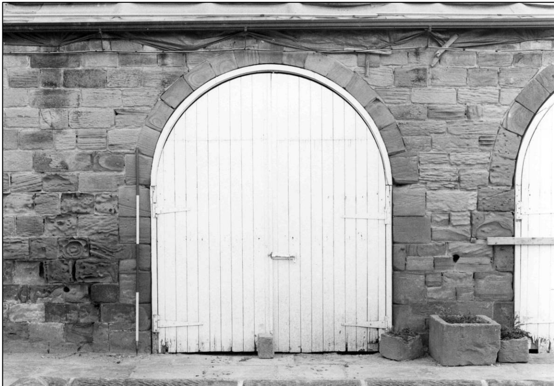
Plate 10: North coach opening, west external elevation, looking E (photo 3/16).
