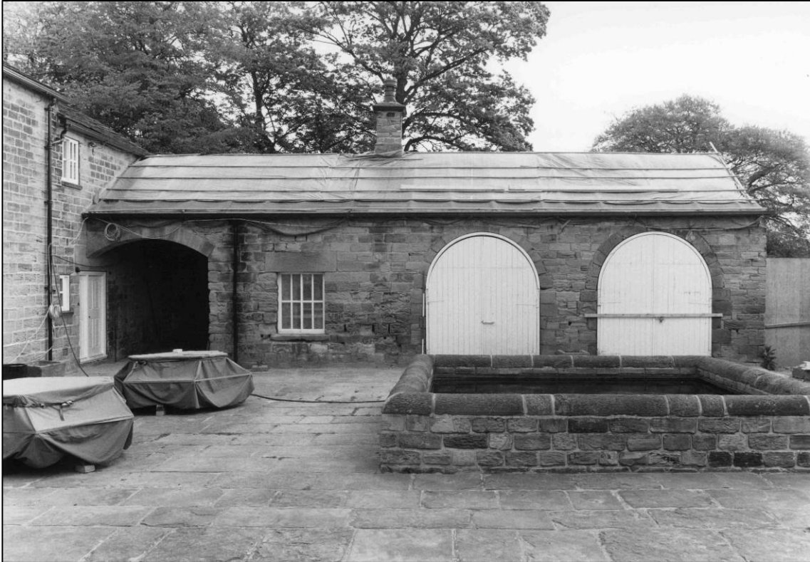
Plate 7: West external elevation, looking E (photo 3/17).
