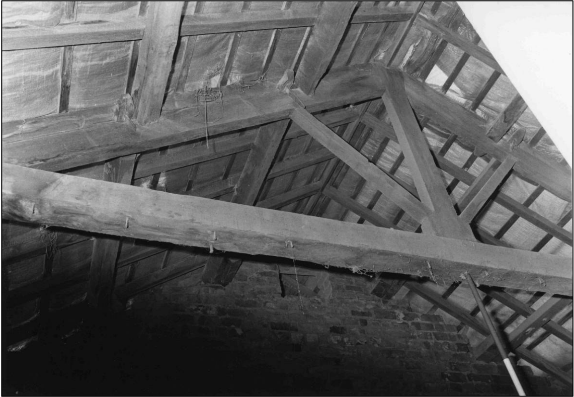
Plate 37: Truss of central room, looking NE (photo 2/9).
