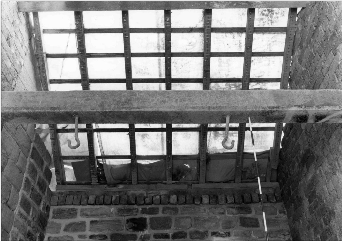
Plate 23: Beam crossing north room, looking E (photo 3/7).
