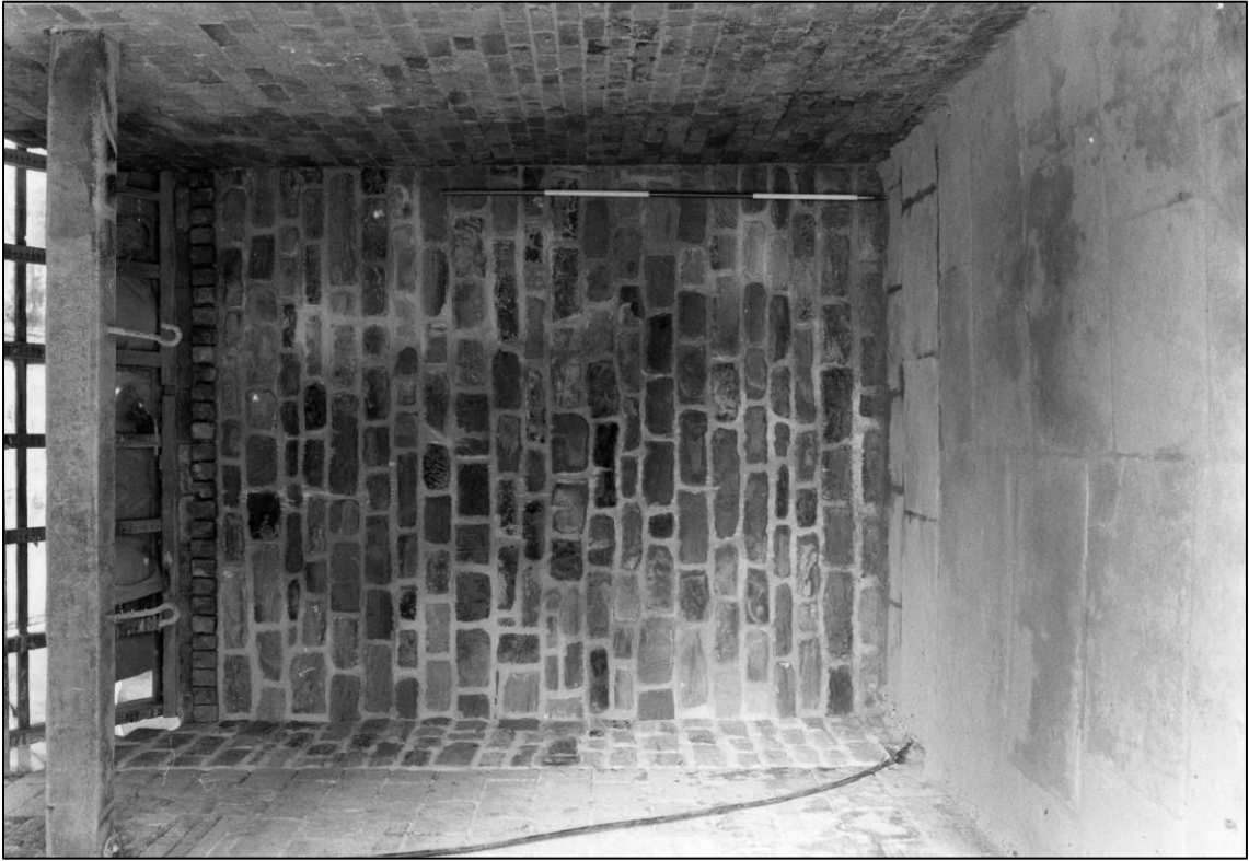
Plate 19: East wall of north room, looking E (photo 3/1) (top to left).
