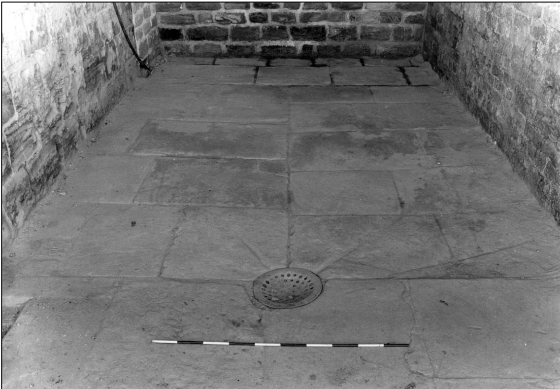
Plate 14: Drain and flagged floor in north room, looking E (photo 3/9).
