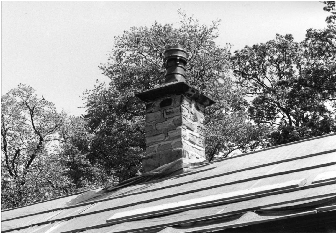
Plate 6: Coach house chimney, looking NE (photo 3/15).
