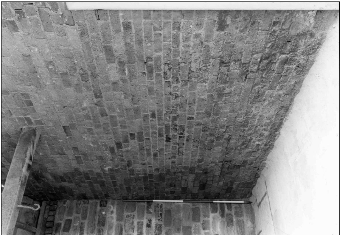
Plate 20: South wall of north room, looking SE (photo 3/5) (top to left).
