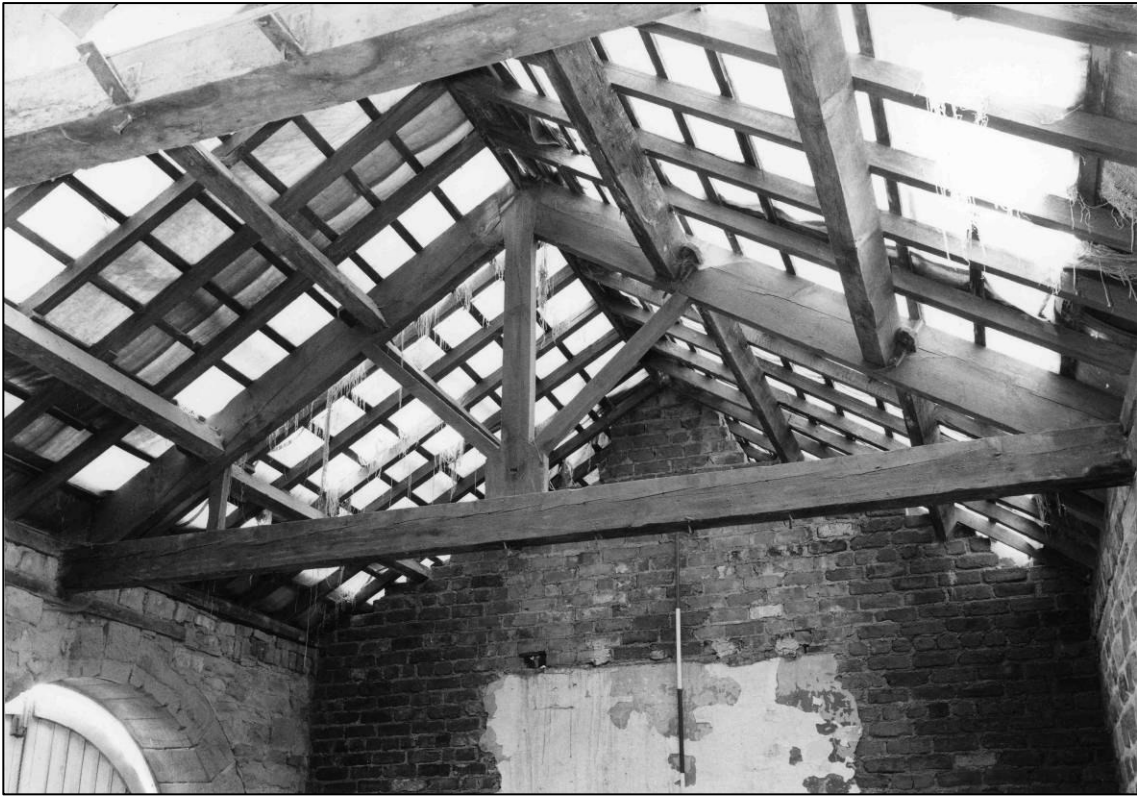
Plate 47: North truss of south room, looking NW (photo 1/9).
