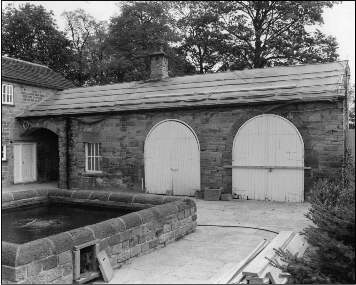
Plate 5: West external elevation, looking NE (photo 3/18).
