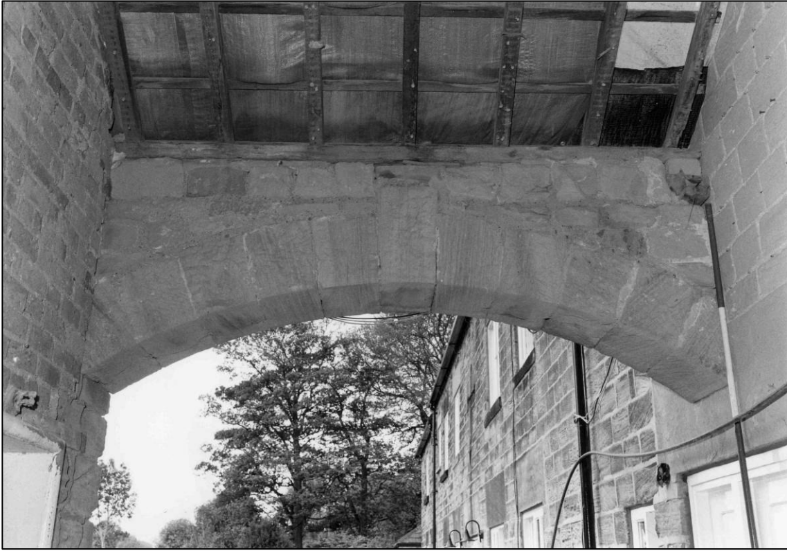
Plate 17: Entrance arch to north room, looking W (photo 3/12).
