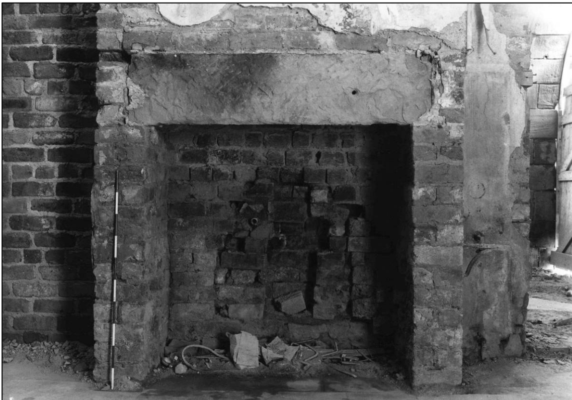
Plate 34: Fireplace in south wall of central room, looking S (photo 2/10).
