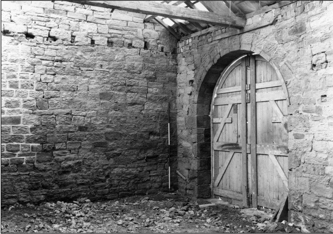
Plate 43: South-east corner of south room, looking SW (photo 1/1).
