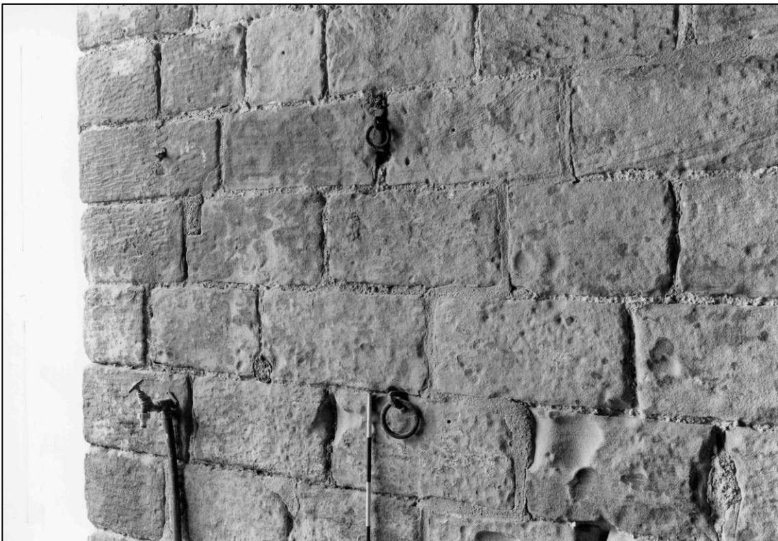
Plate 16: Tethering rings to north wall of north room, looking NW (photo 3/11).
