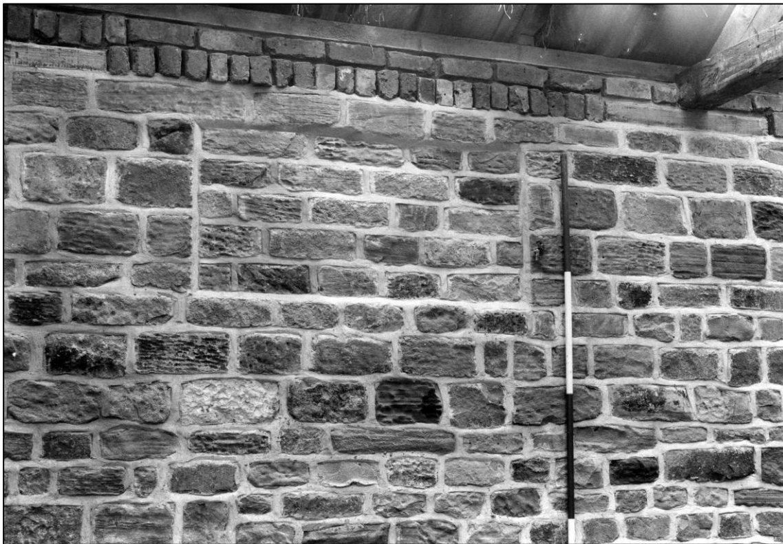
Plate 42: Blocked window in east wall of south room, looking E (photo 1/16).
