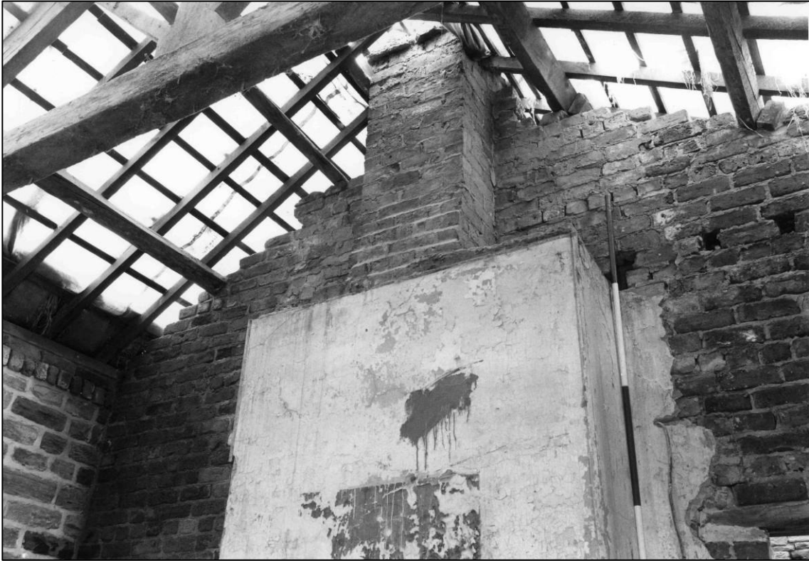
Plate 31: Upper part of south wall of central room, looking S (photo 2/15).
