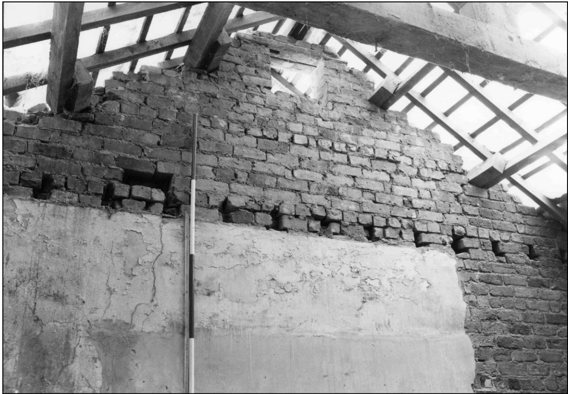
Plate 27: Upper part of north wall of central room, looking N (photo 2/7).
