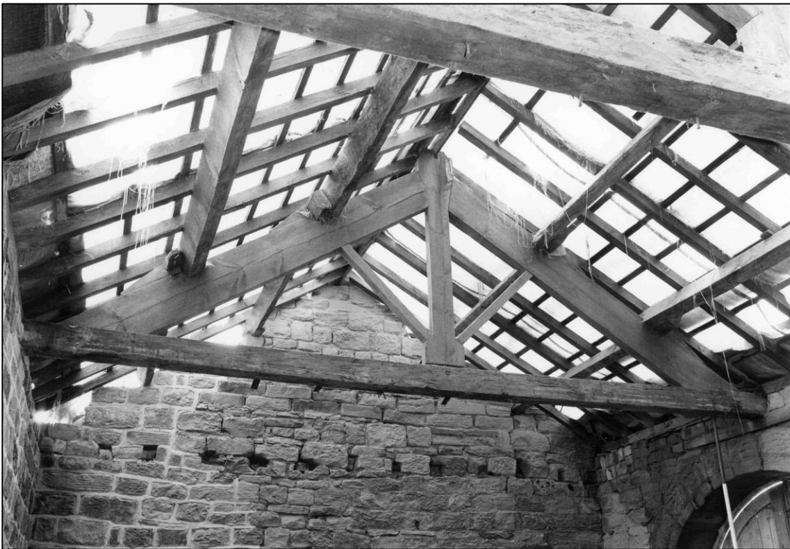
Plate 48: South truss of south room, looking SE (photo 1/11).
