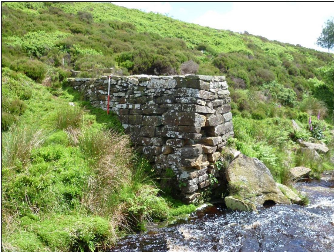
Plate 7: East pier, looking SE (photo 2/239).
