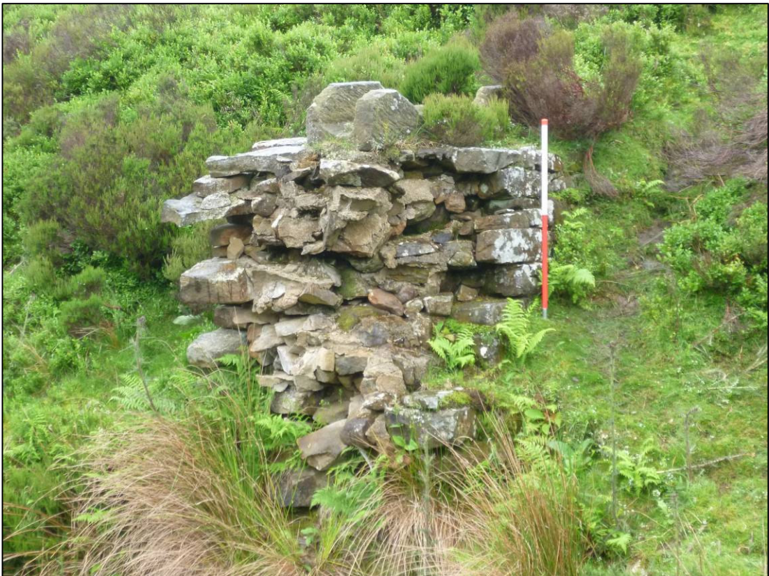
Plate 5: Exposed core in west end of west pier, looking W (photo 2/248).
