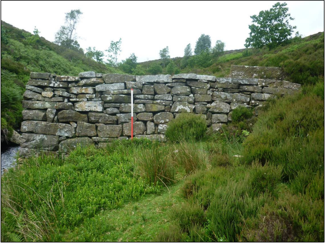
Plate 6: South face of east pier, looking N (photo 1/638).
