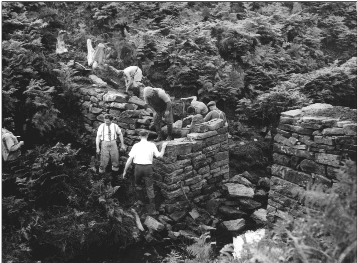
Photographs of repairs in progress (courtesy Helmsley Archive, HA 02455 & HA 02462).
