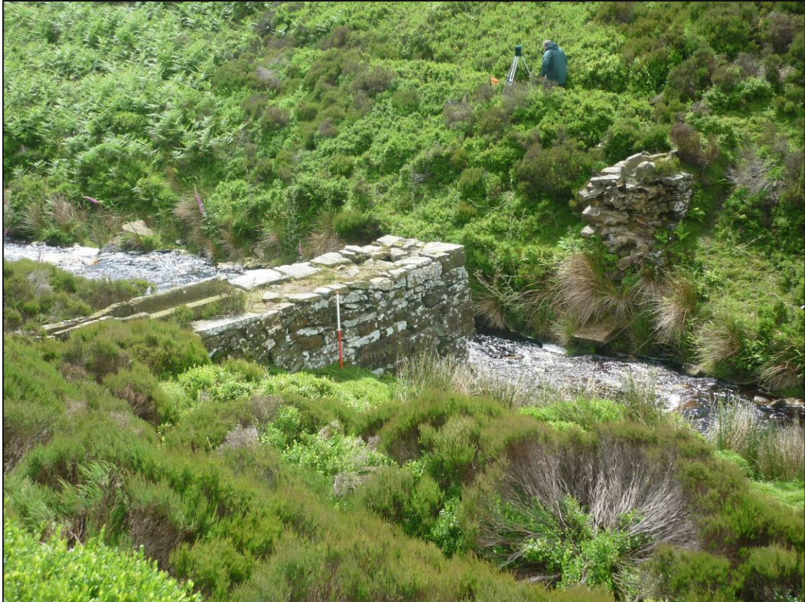
Plate 1: General view of aqueduct, looking SW (photo 1/628).
