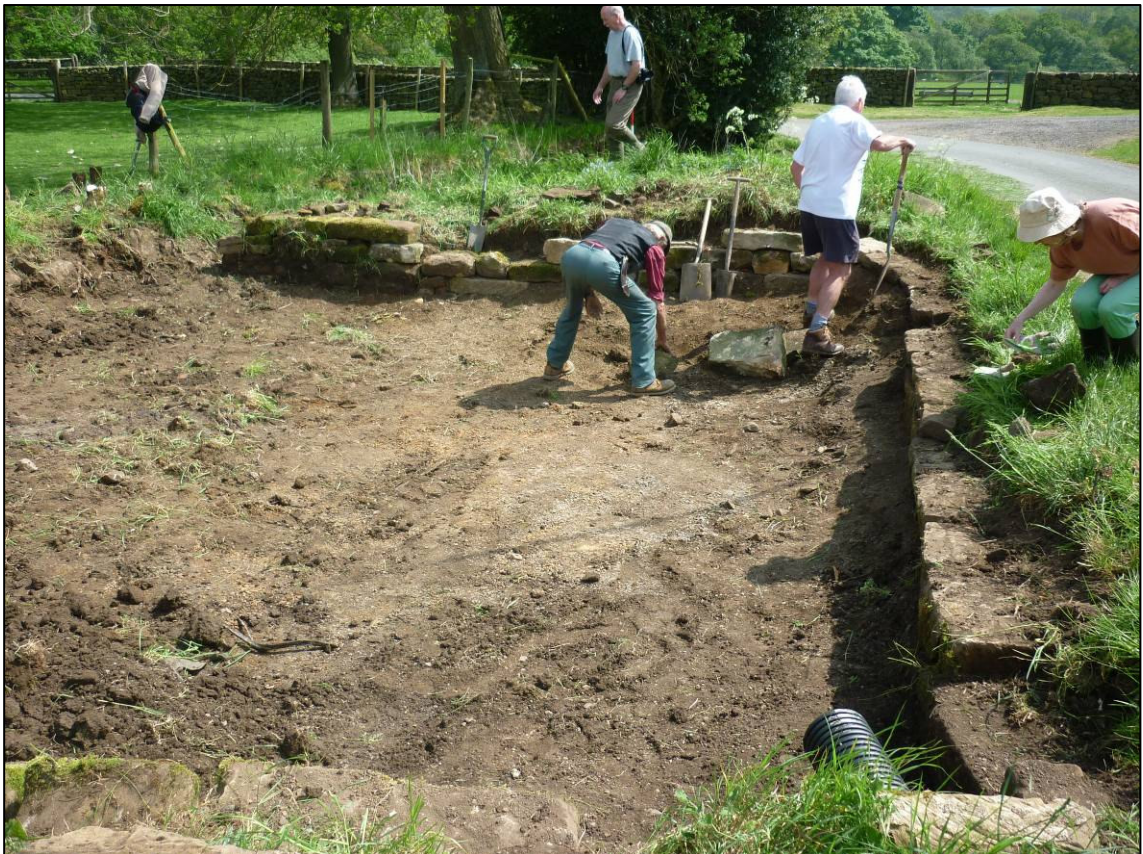
Plate 4: Pond under excavation and west wall partly rebuilt, looking S (photo 1/246).
