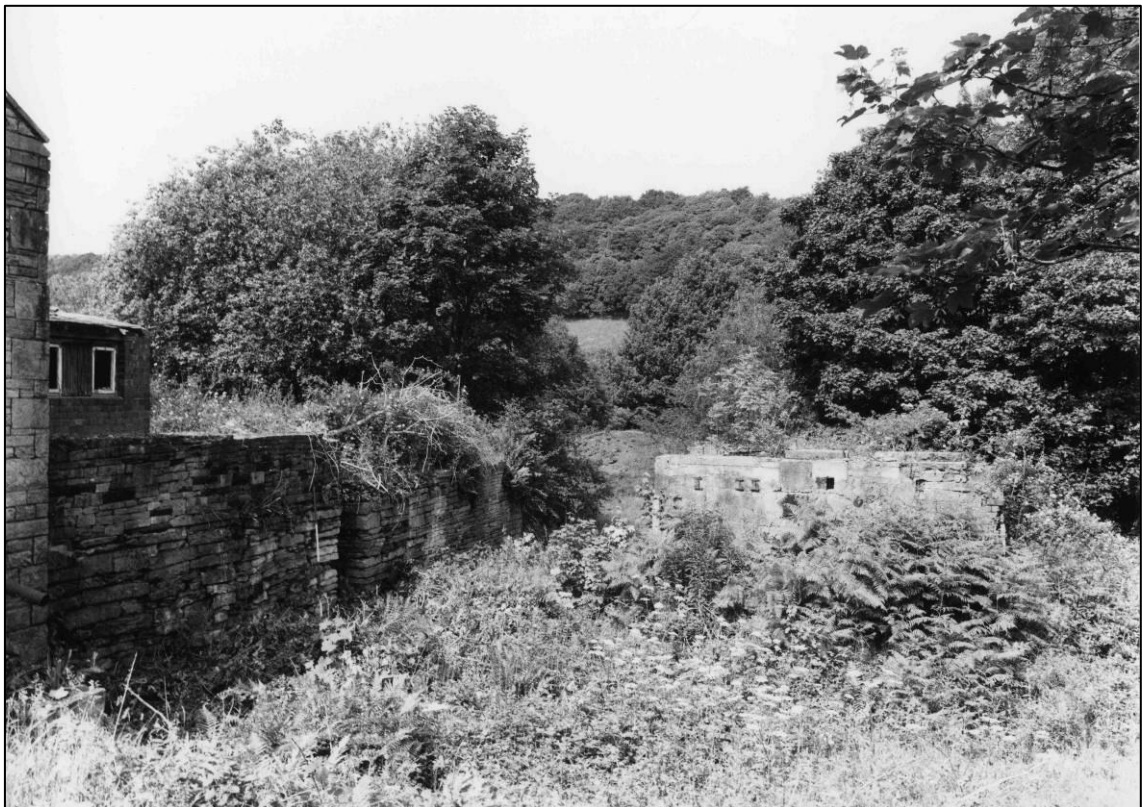
Plate 6: Building N2, revetment wall to north and base, looking NW (photo 6/6).
