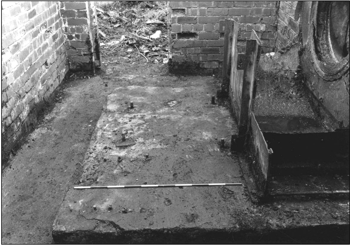
Plate 41: Building N3, fan case and base, looking E (photo 3/13).
