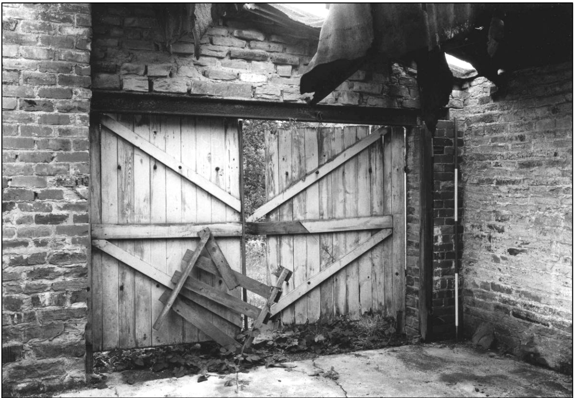
Plate 50: Building N4, interior, looking SE (photo 3/17).
