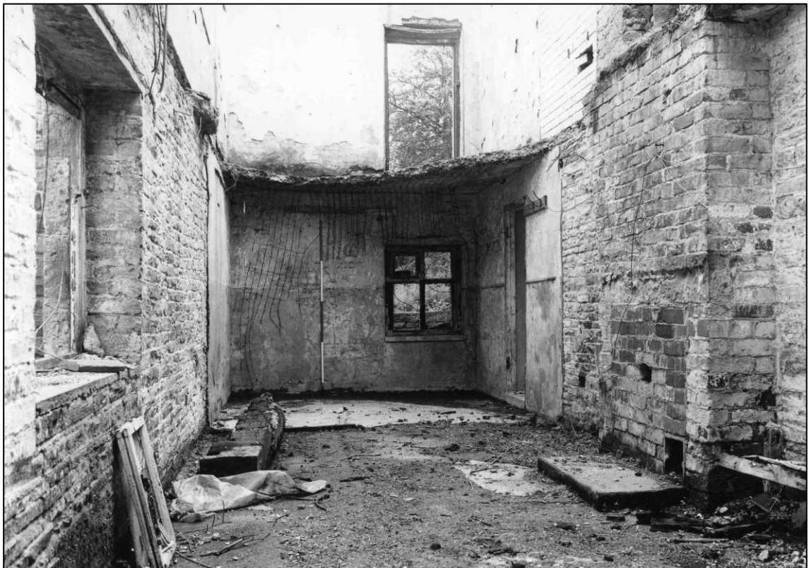
Plate 80: Building S1, ground floor interior, looking E (photo 2/16).
