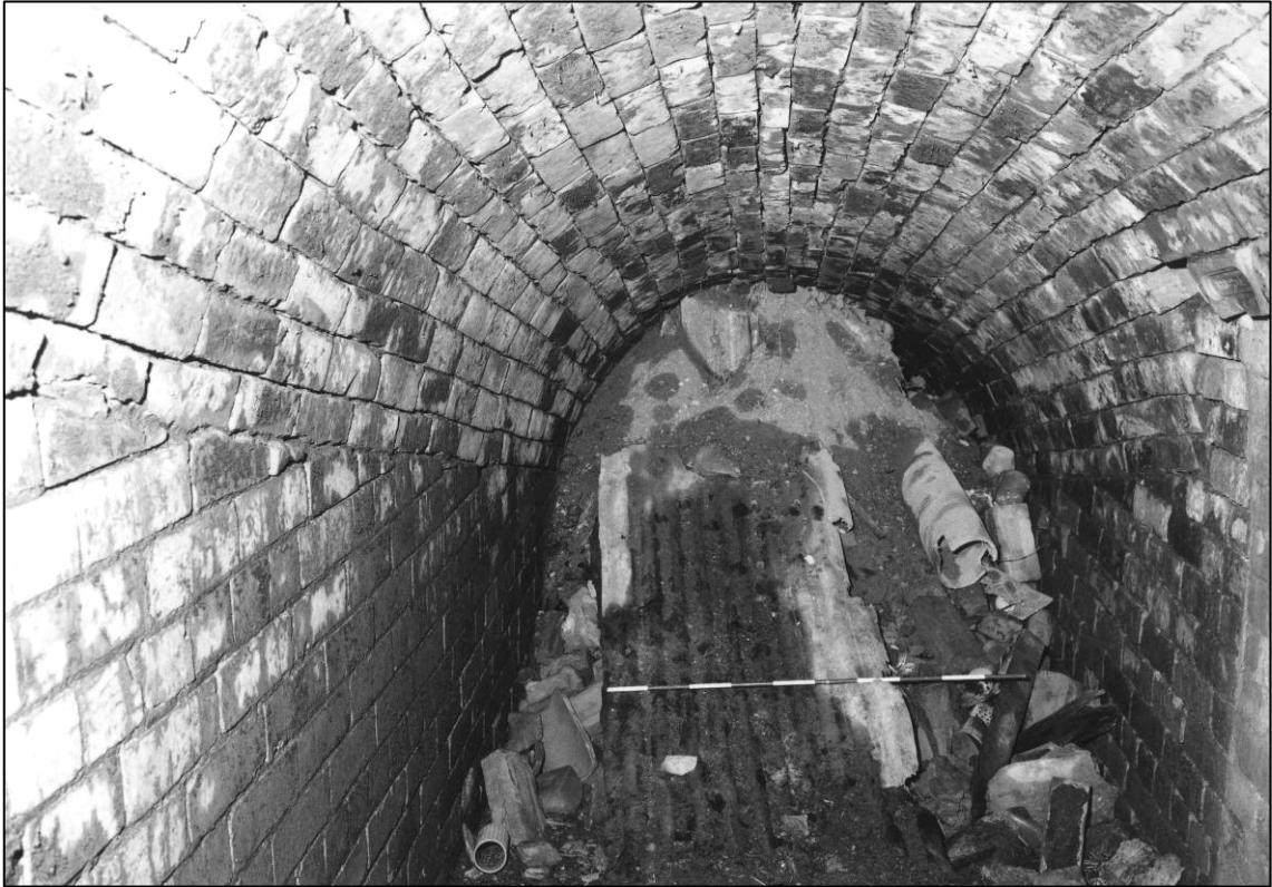
Plate 63: Building N4, interior of fan drift, looking W (photo 4/4).
