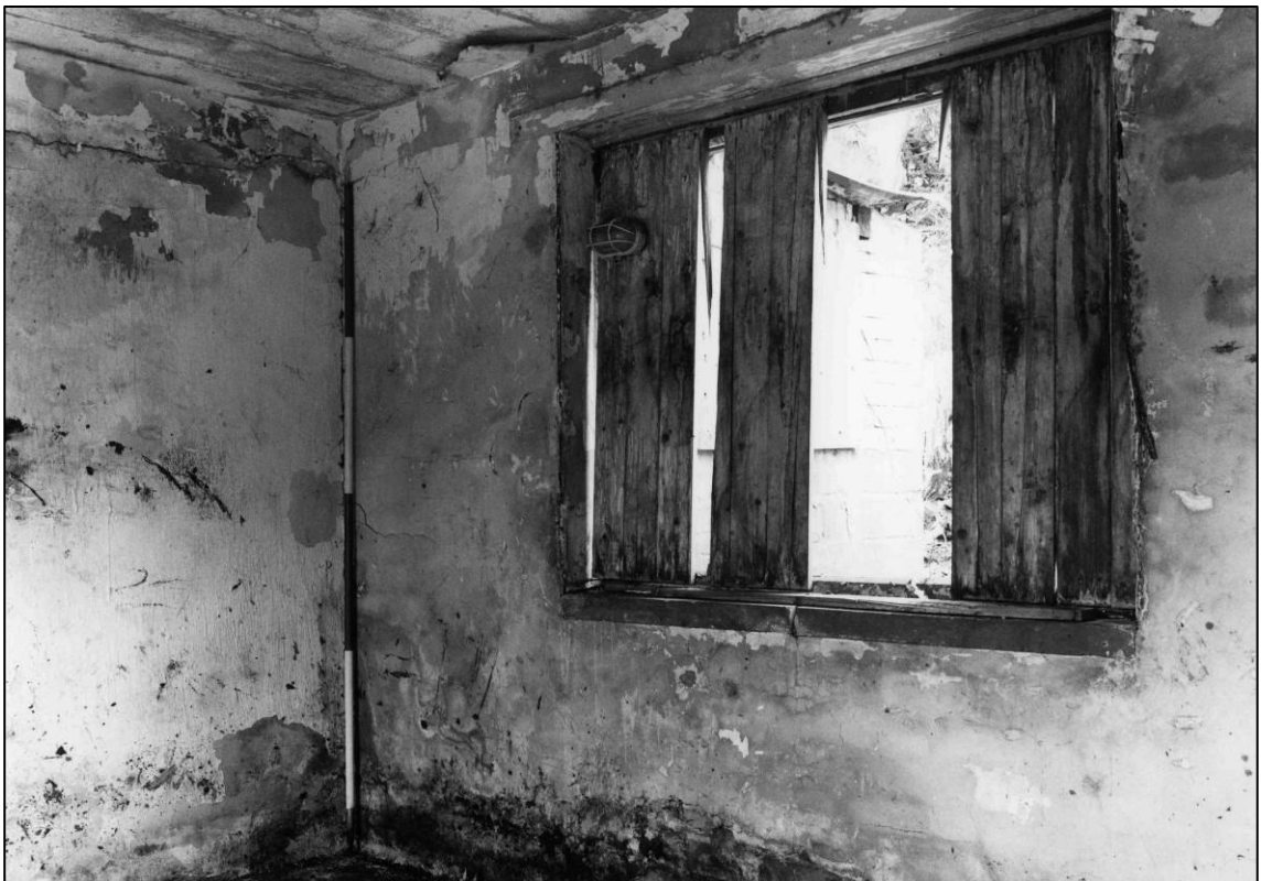
Plate 74: Building S3, interior, looking SE (photo 2/13).
