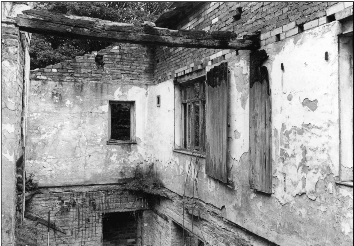
Plate 86: Building S1, first floor interior, looking NW (photo 3/1).
