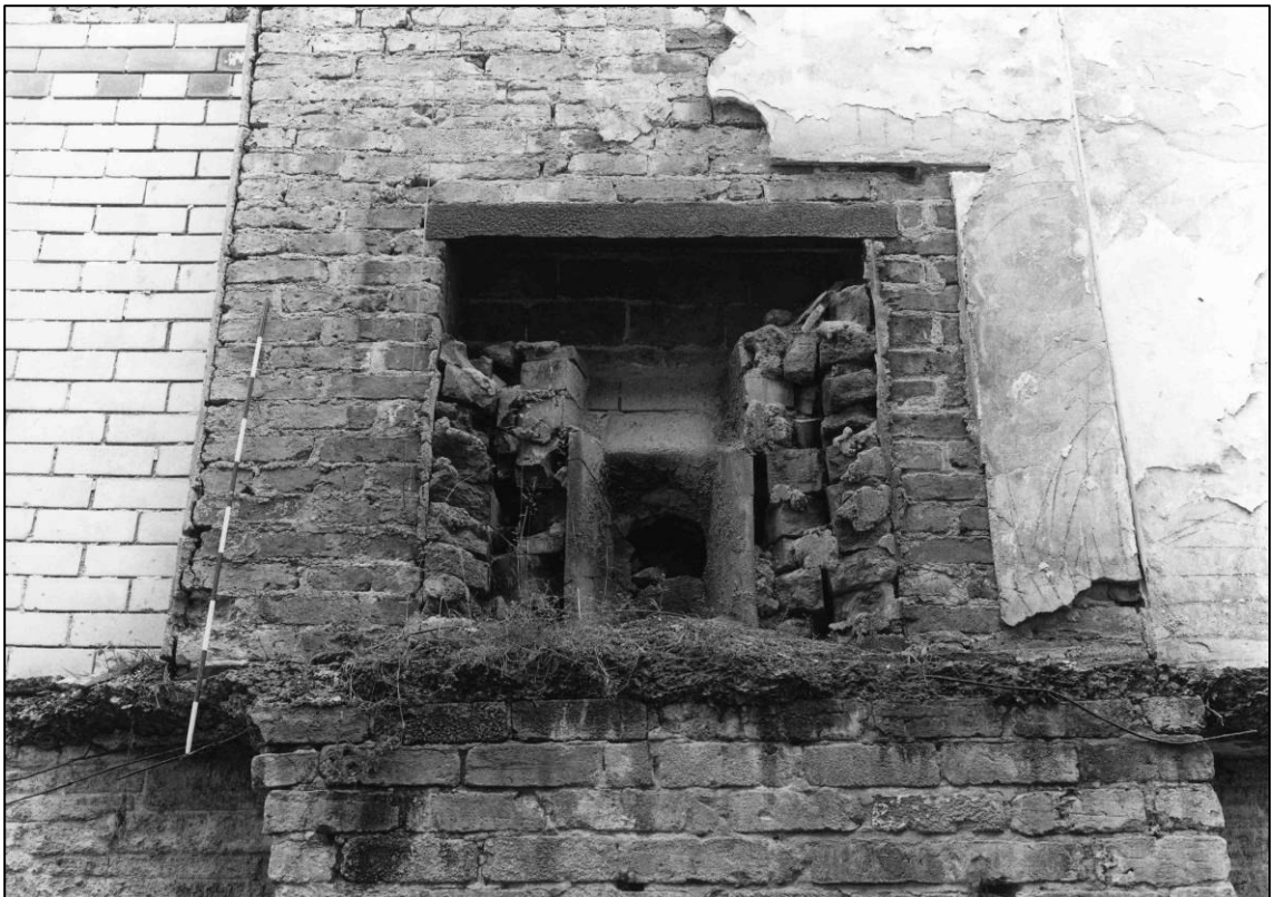
Plate 84: Building S1, first floor fireplace, looking S (photo 3/7).
