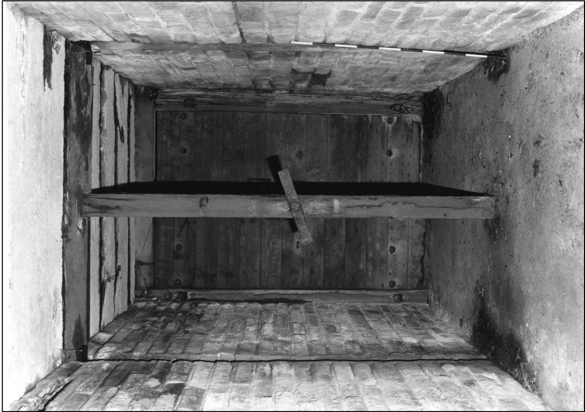
Plate 59: Building N4, interior of fan passage, looking W (photo 4/13).
