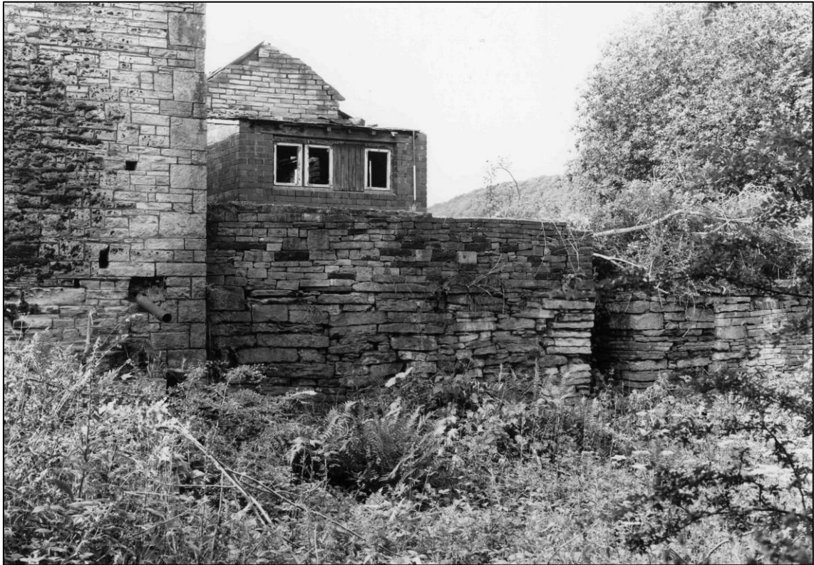
Plate 5: Building N2, revetment wall to north, looking W (photo 6/9).
