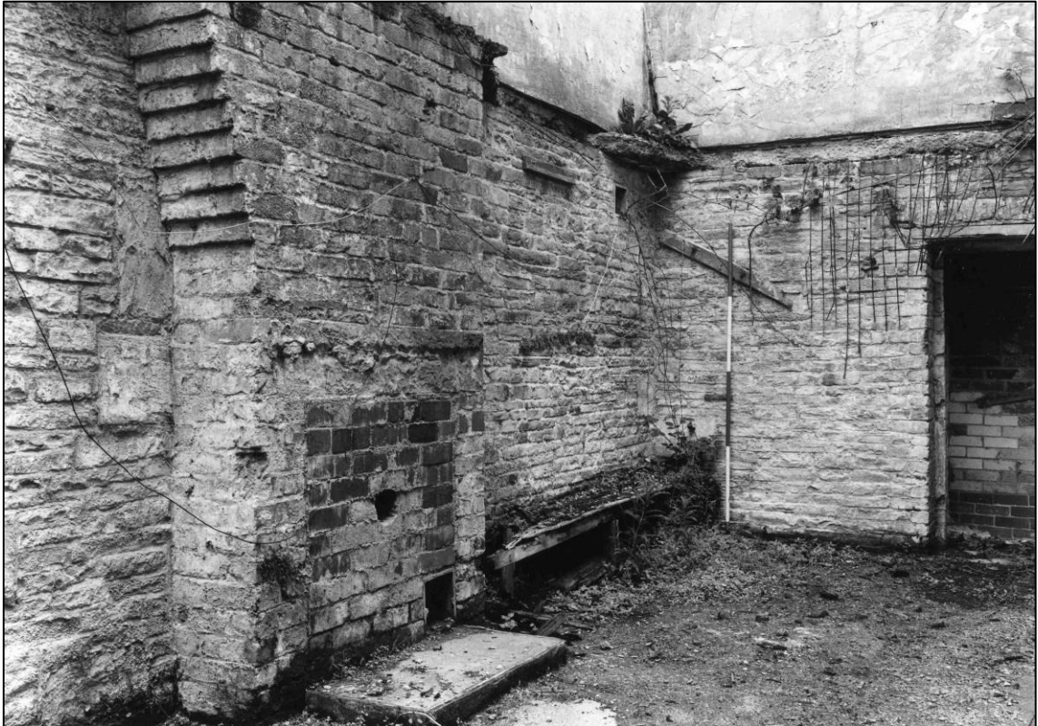
Plate 79: Building S1, ground floor interior, looking SW (photo 2/18).
