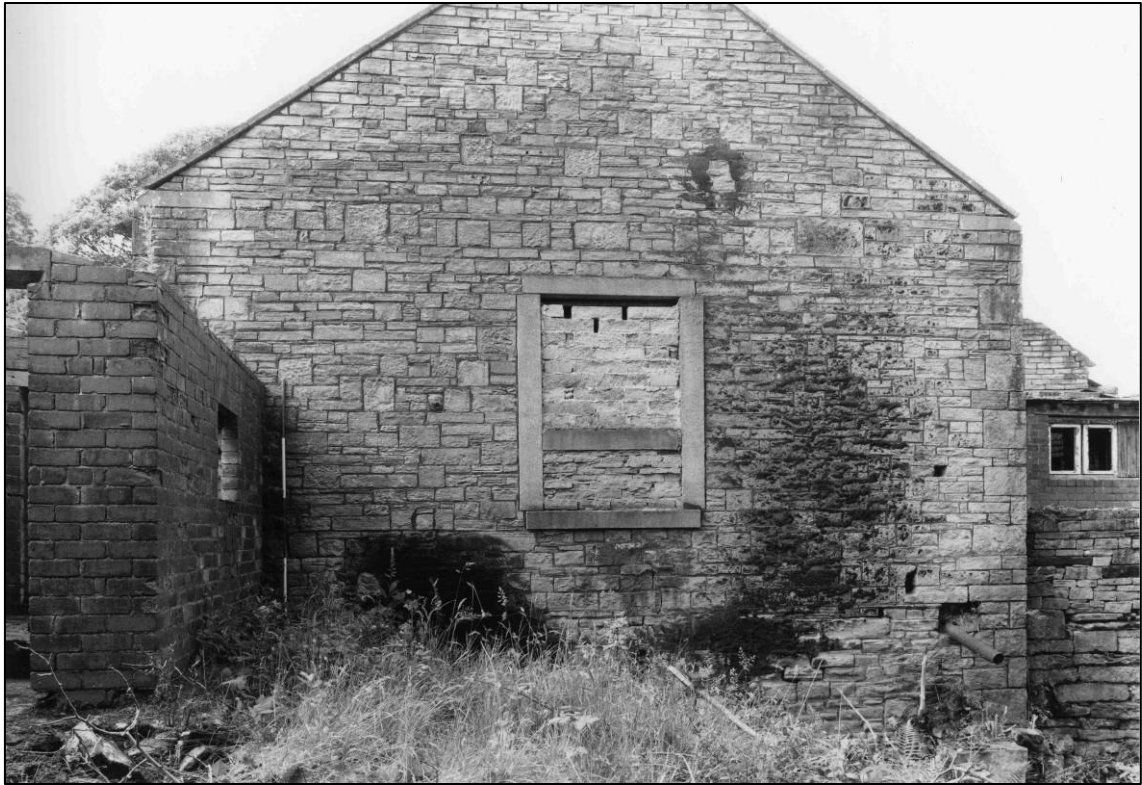
Plate 27: Building N2, east gable, looking W (photo 6/3).
