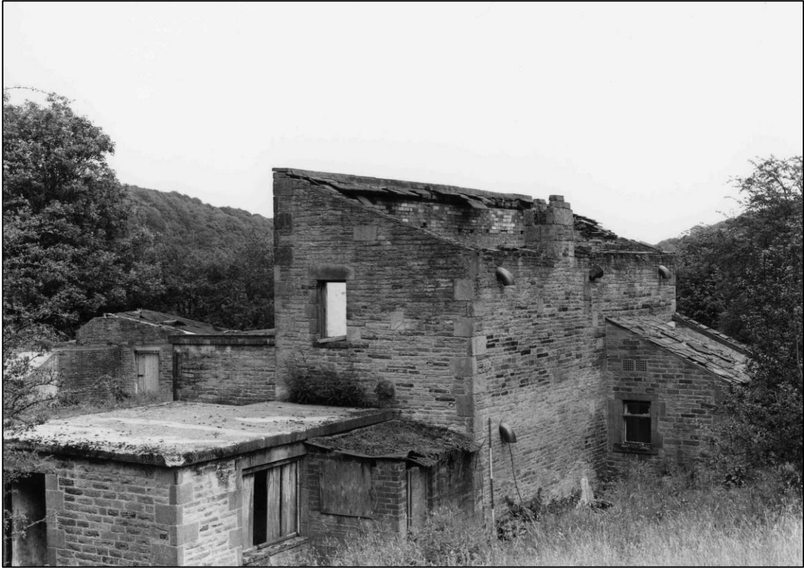
Plate 67: Mine offices (Buildings S1, S3, S4 and S5), looking NE (photo 6/12).
