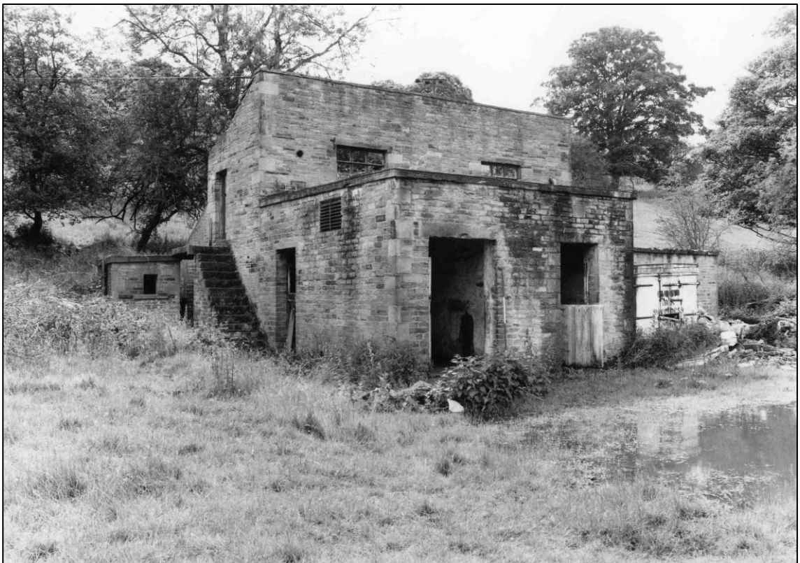
Plate 66: Mine offices (Buildings S1, S2 and S6), looking SW (photo 6/17).
