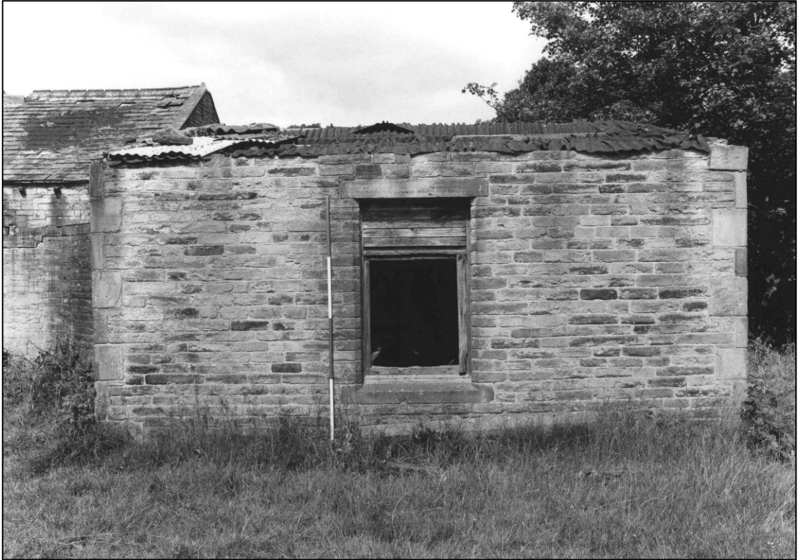
Plate 49: Building N4, external south elevation, looking N (photo 5/17).
