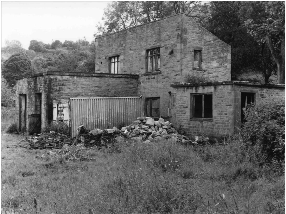
Plate 2: Mine offices (Buildings S1, S5 and S6), looking SE (photo 6/11).
