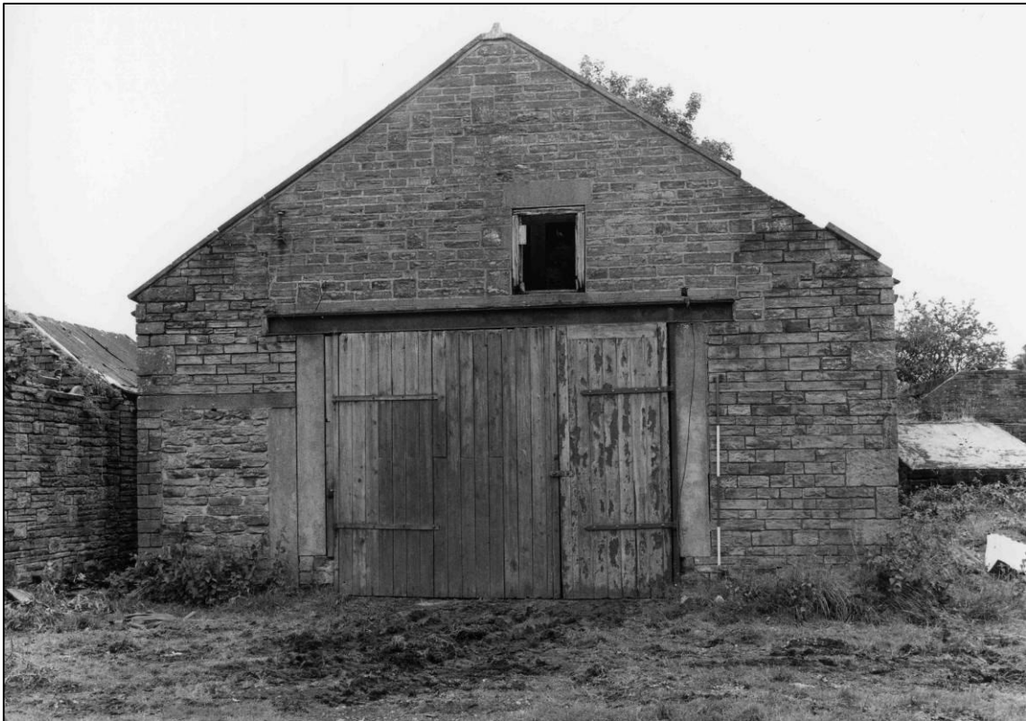
Plate 24: Building N2, west gable, looking E (photo 5/4).
