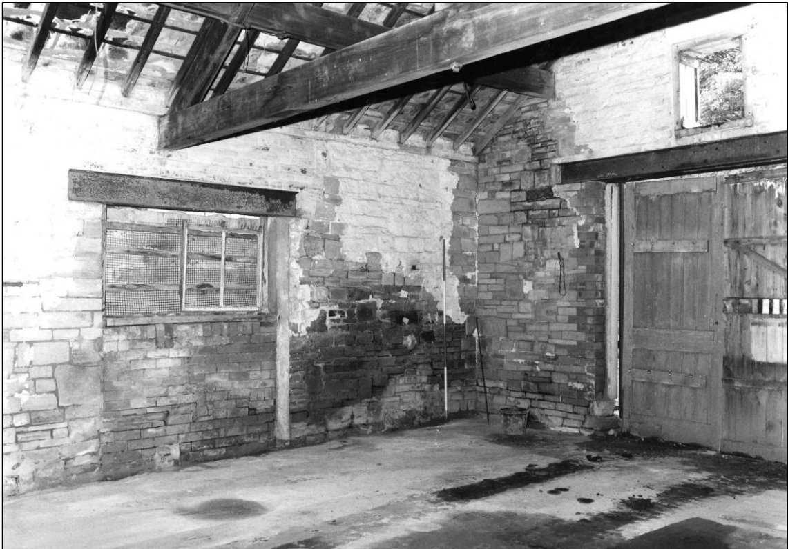
Plate 34: Building N2, interior, looking SW (photo 1/5).
