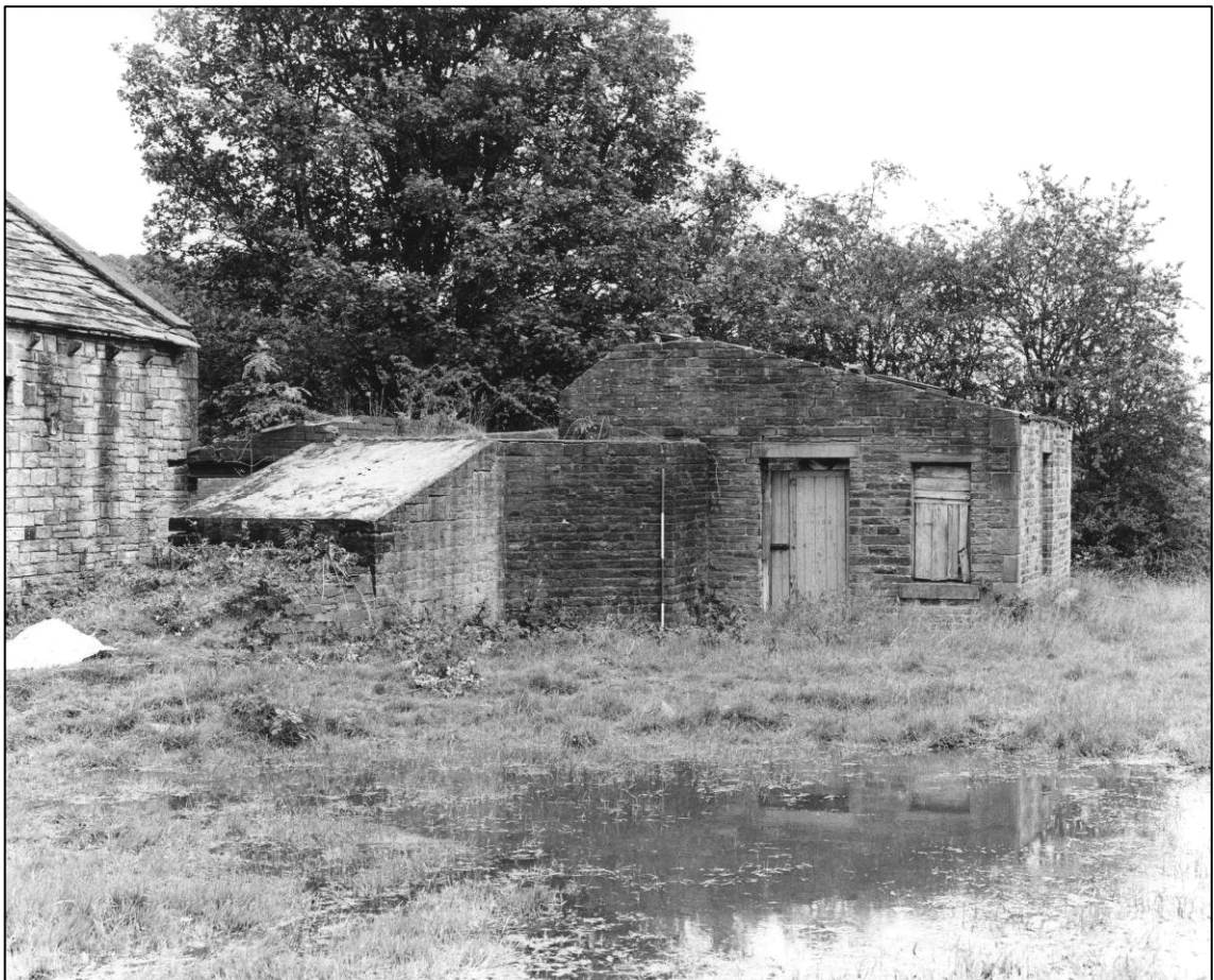
Plate 44: Building N4, looking E (photo 5/6).
