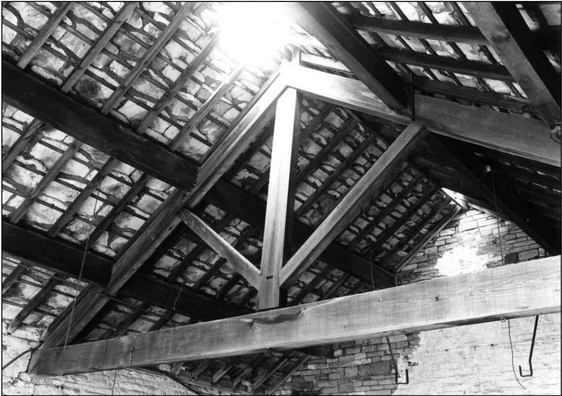
Plate 35: Building N2, truss, looking NE (photo 1/11).
