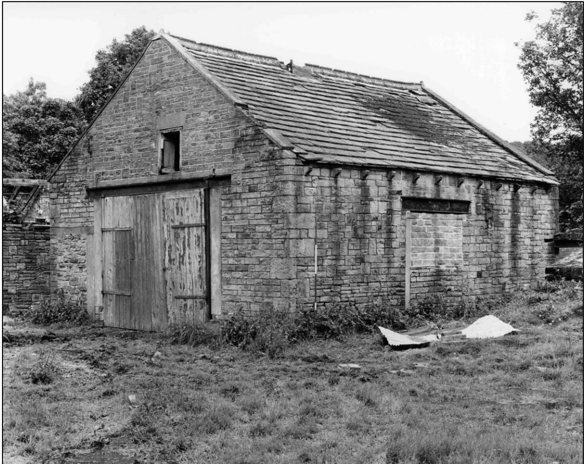
Plate 20: Building N2, exterior, looking NE (photo 5/5).
