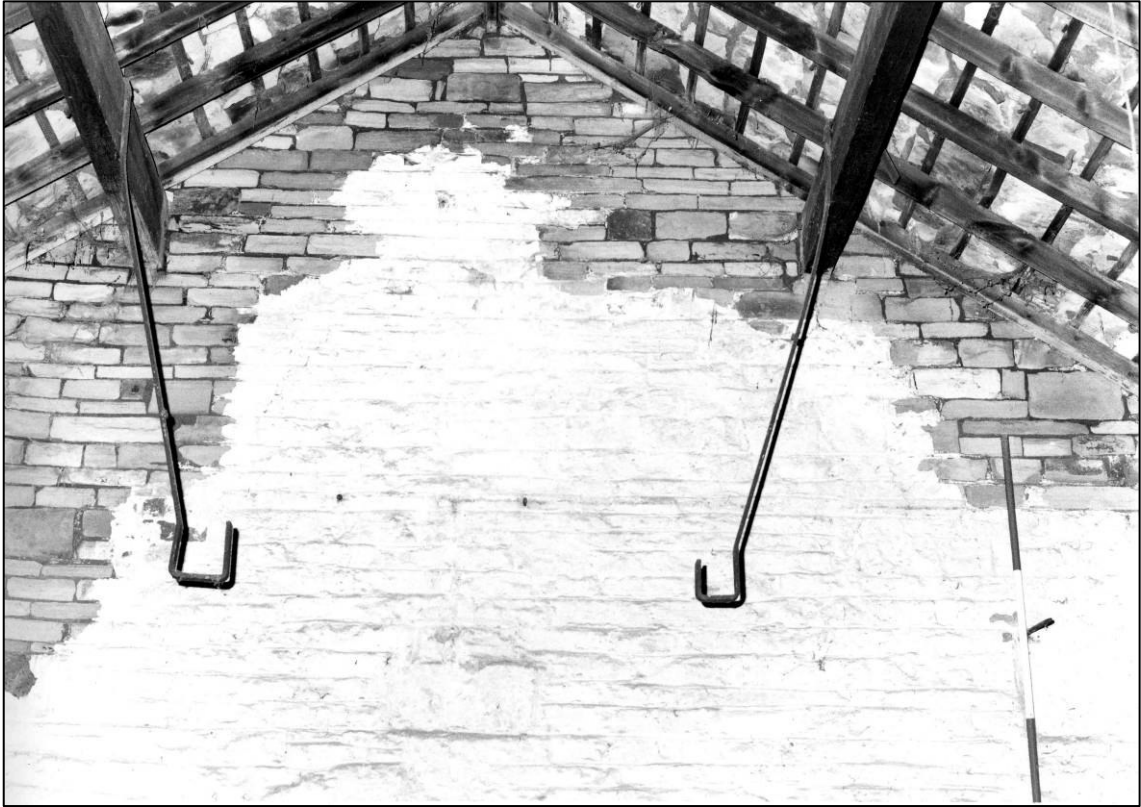
Plate 37: Building N2, brackets from truss, looking E (photo 1/7).
