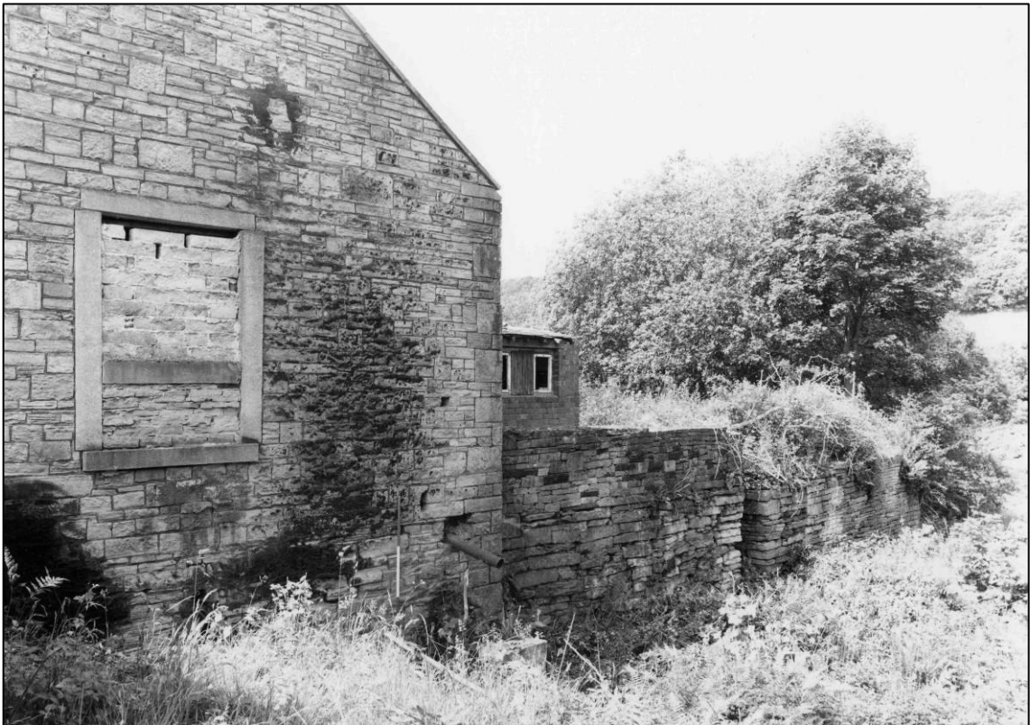
Plate 4: Building N2, revetment wall to north, looking NW (photo 6/5).
