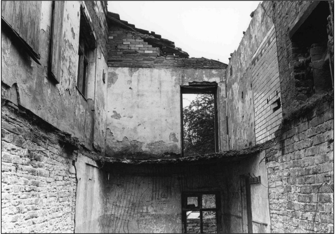
Plate 83: Building S1, first floor interior, looking E (photo 3/6).
