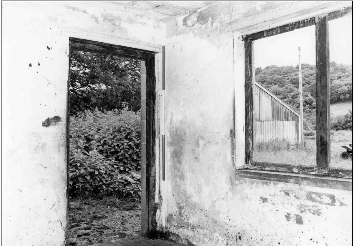
Plate 75: Building S3, interior, looking NW (photo 2/15).
