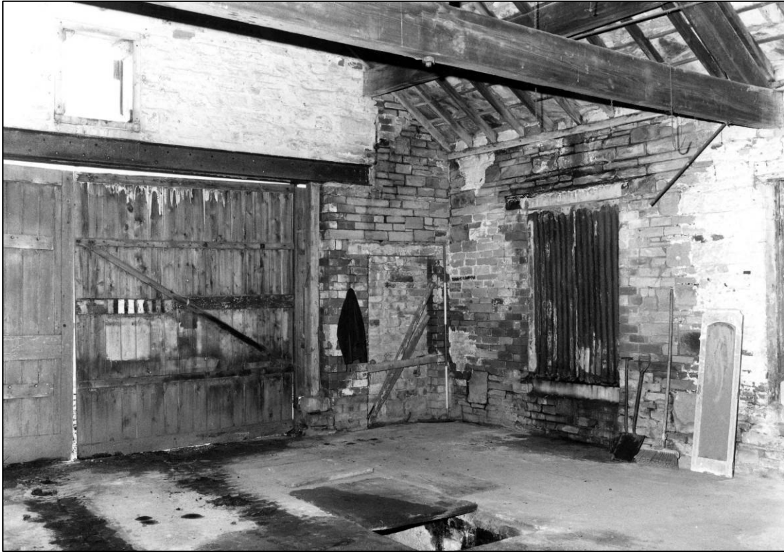
Plate 29: Building N2, interior, looking NW (photo 1/4).
