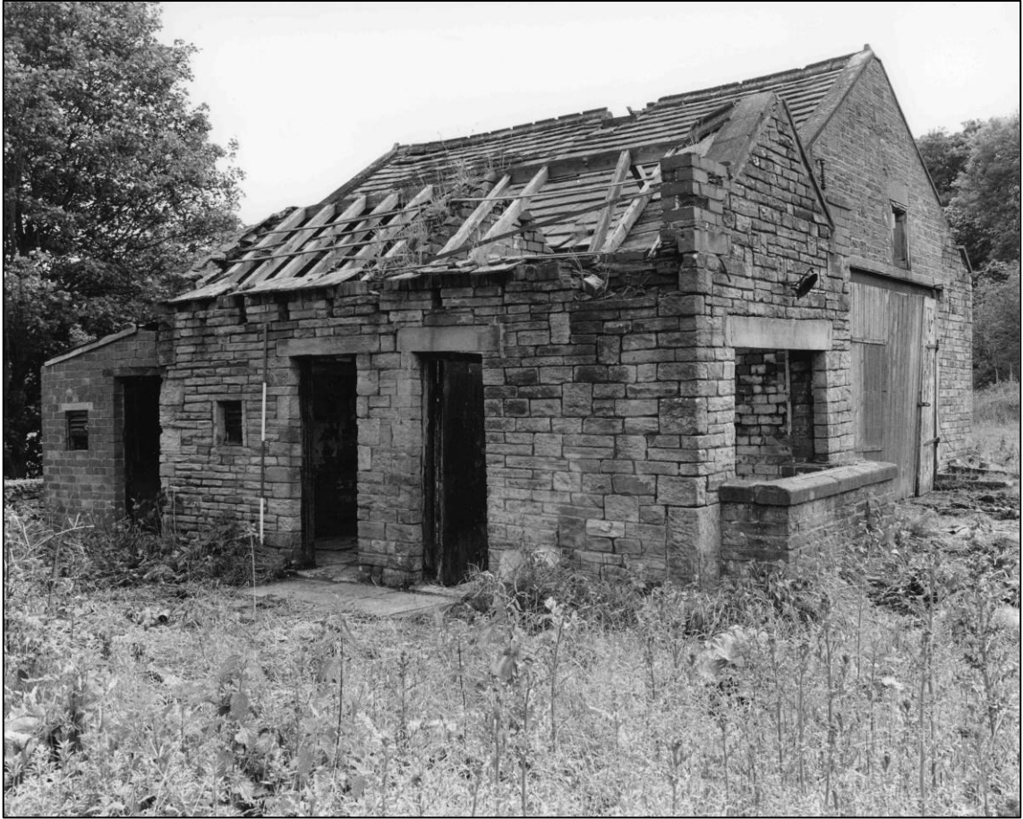
Plate 7: Building N1, exterior, looking SE (photo 5/11).
