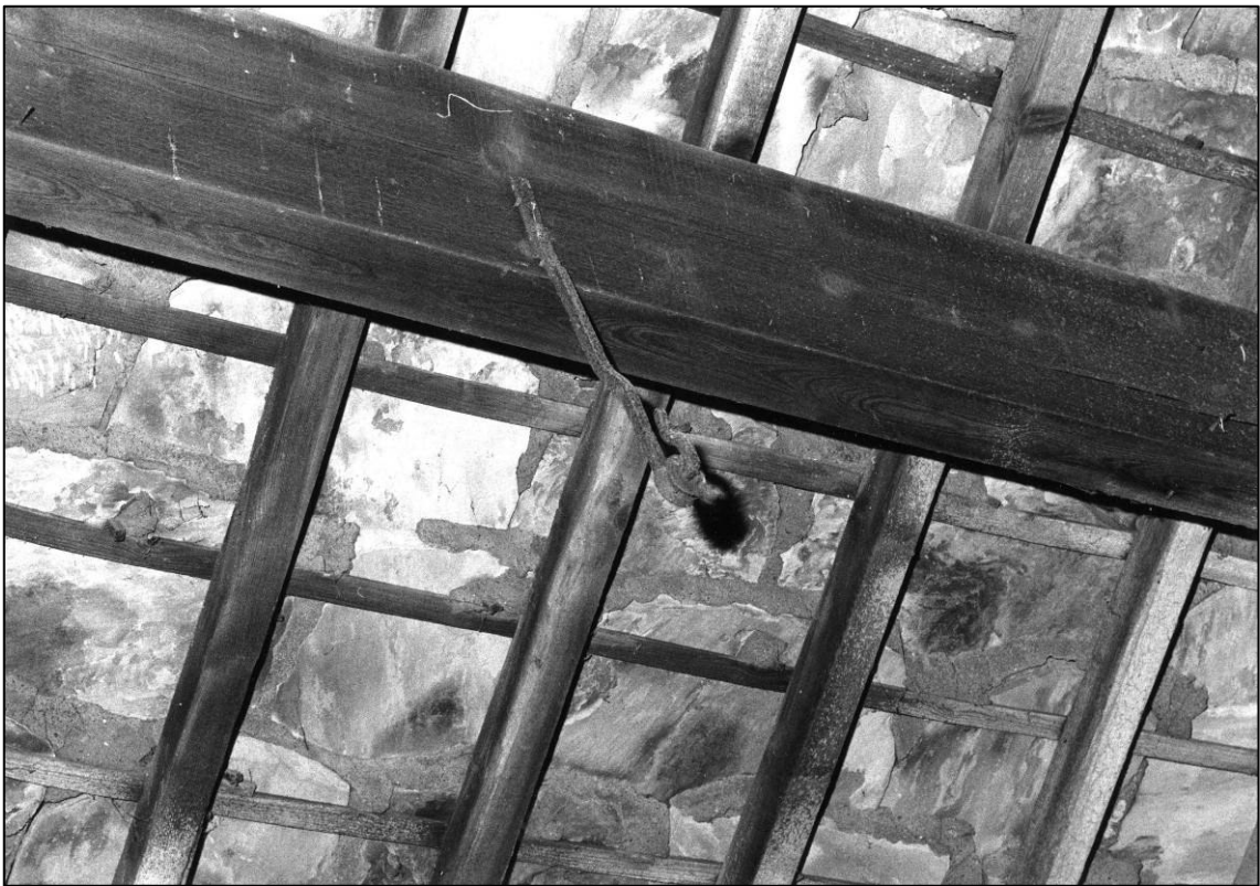
Plate 36: Building N2, guide pulley, looking SW (photo 1/9).
