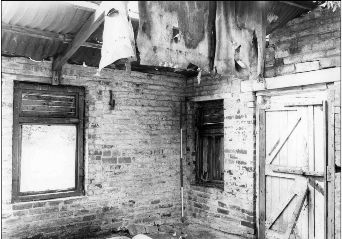
Plate 51: Building N4, interior, looking SW (photo 3/16).
