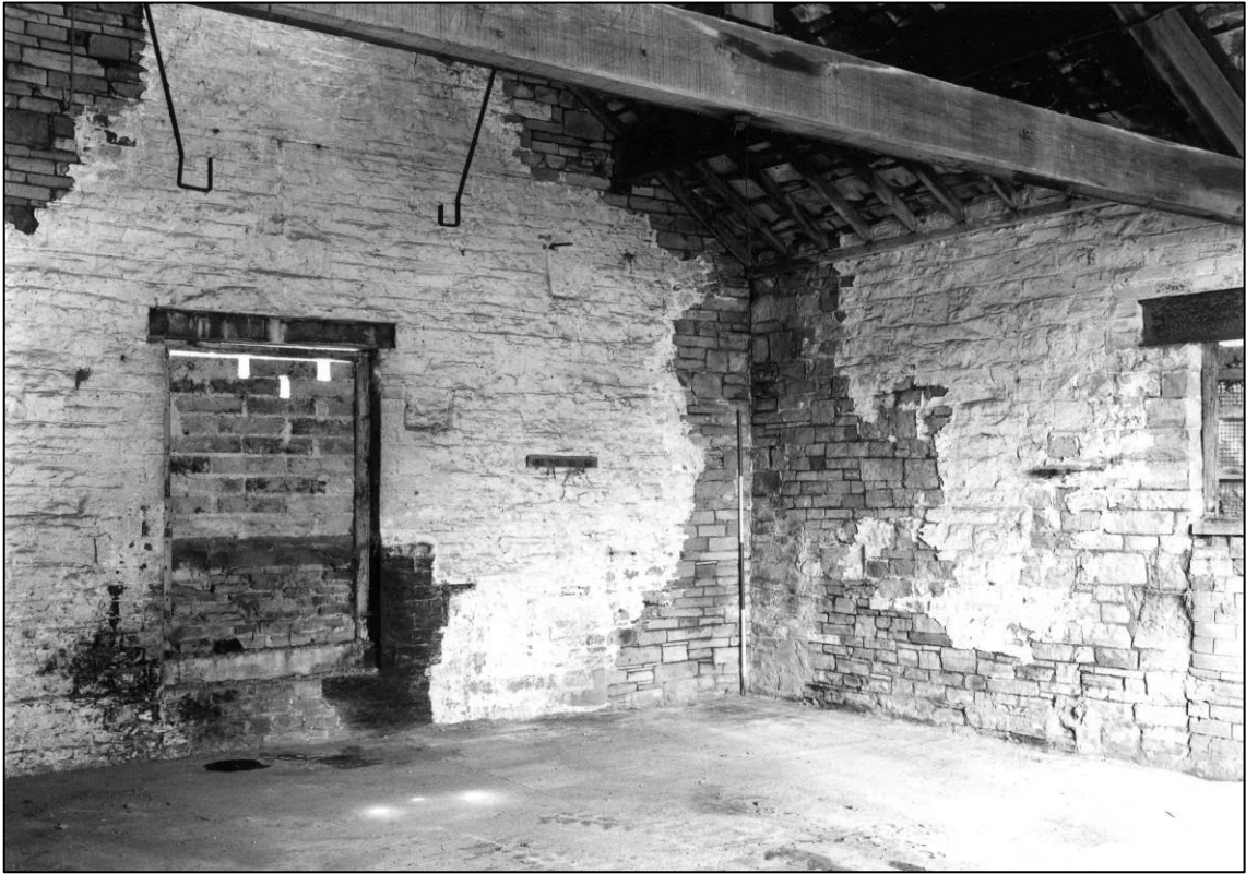
Plate 33: Building N2, interior, looking SE (photo 1/1).
