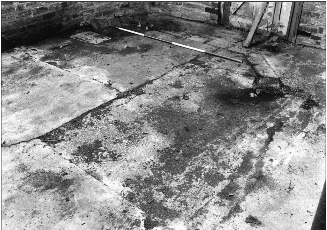
Plate 52: Building N4, former fan and engine base, looking SW (photo 4/16).
