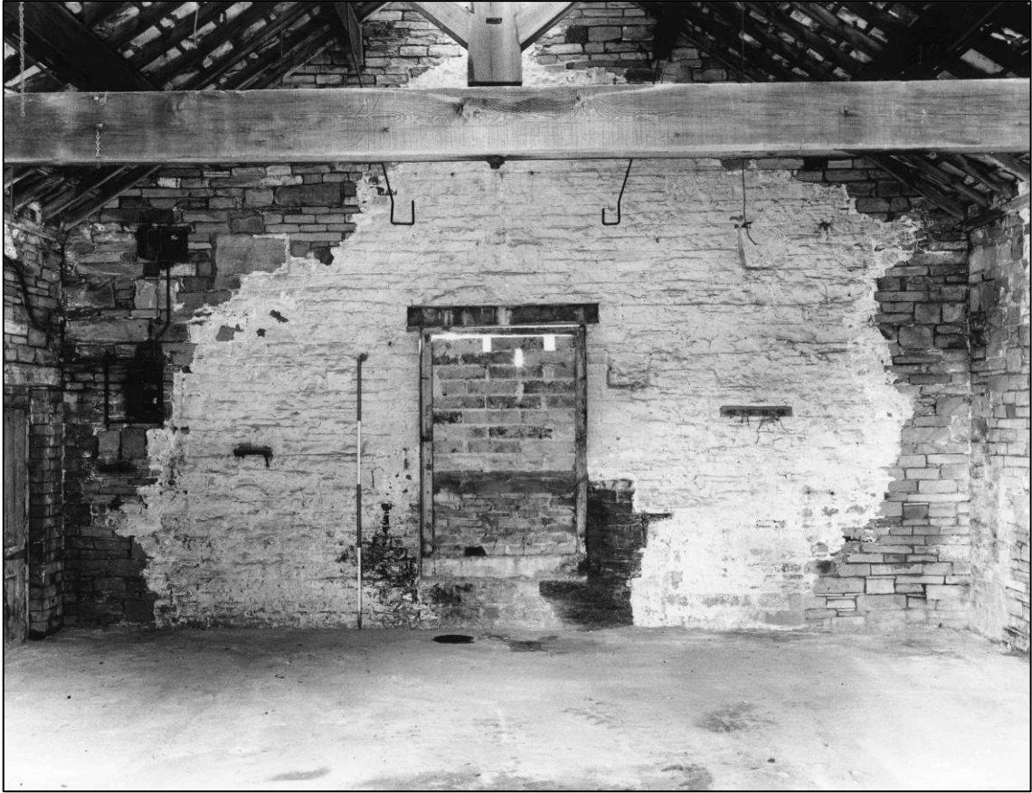
Plate 31: Building N2, interior east wall, looking E (photo 2/2).
