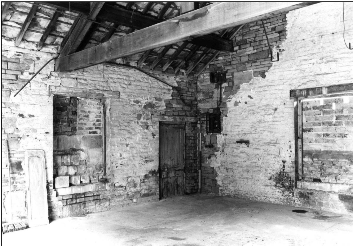
Plate 30: Building N2, interior, looking NE (photo 1/2).
