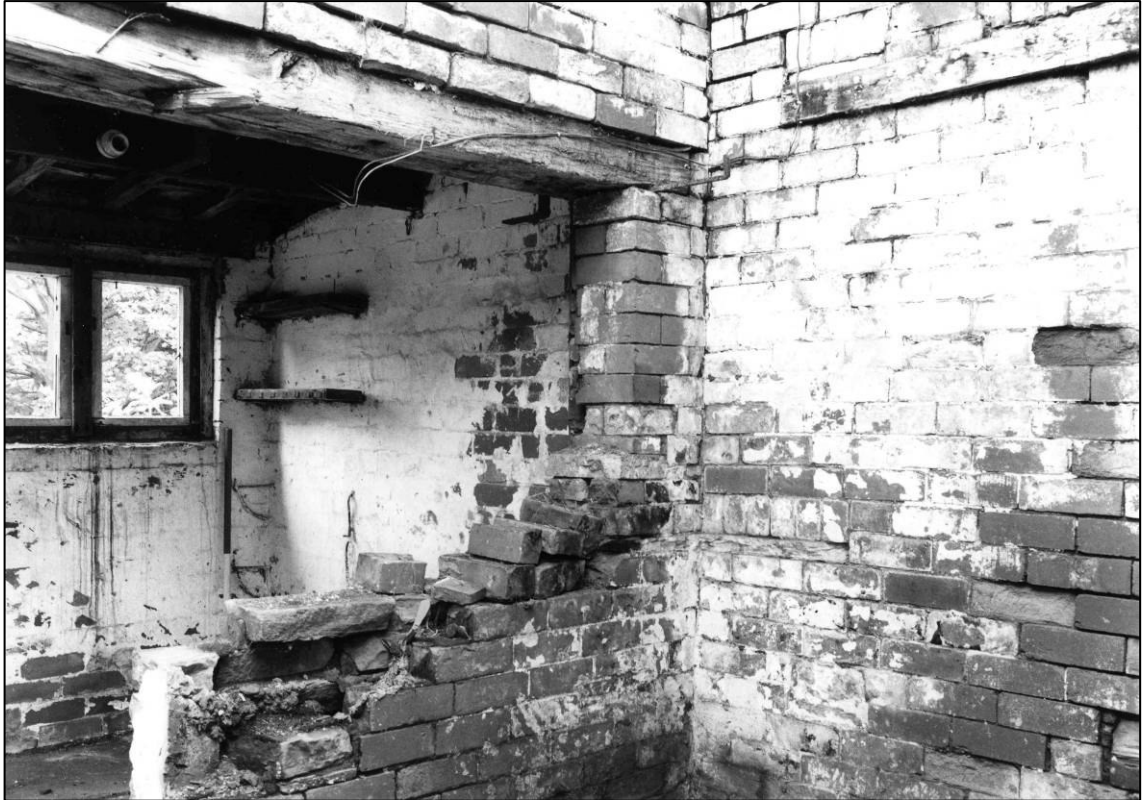
Plate 17: Building N1, interior central cell, looking SE (photo 2/11).
