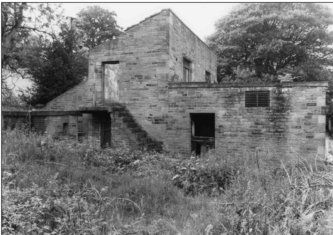
Plate 69: Mine offices (Buildings S1 and S2), looking SW (photo 6/16).
