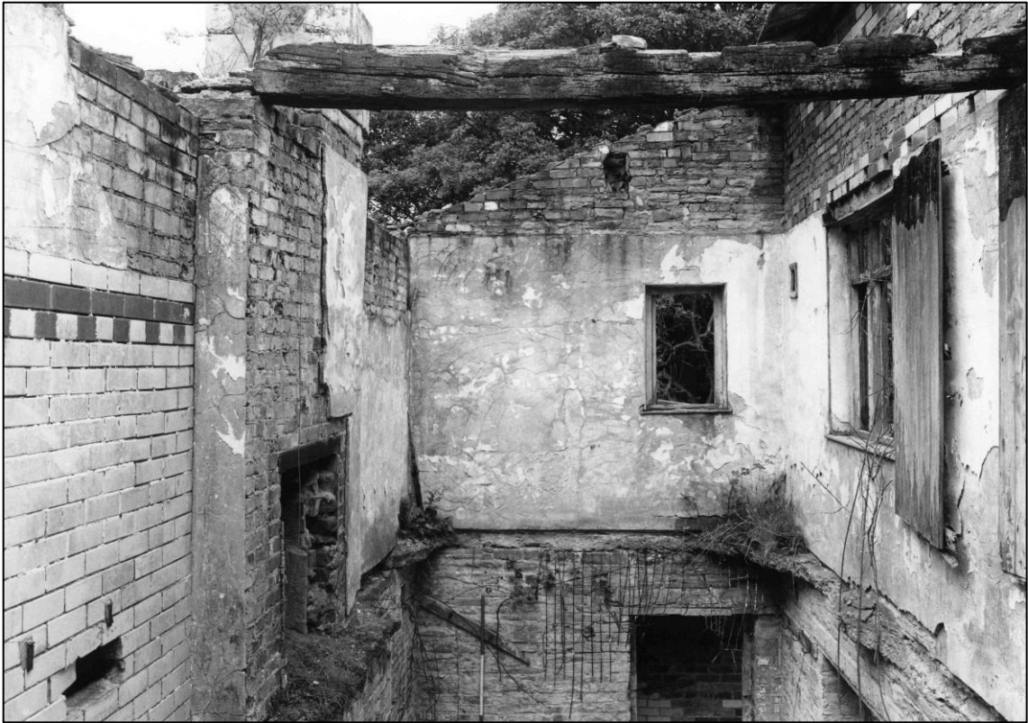
Plate 85: Building S1, first floor interior, looking W (photo 3/3).
