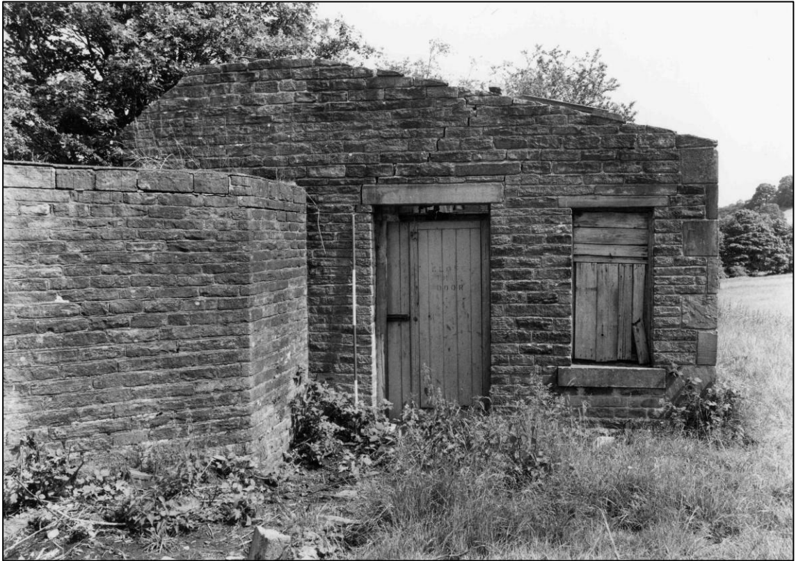
Plate 45: Building N4, external west elevation, looking E (photo 5/16).
