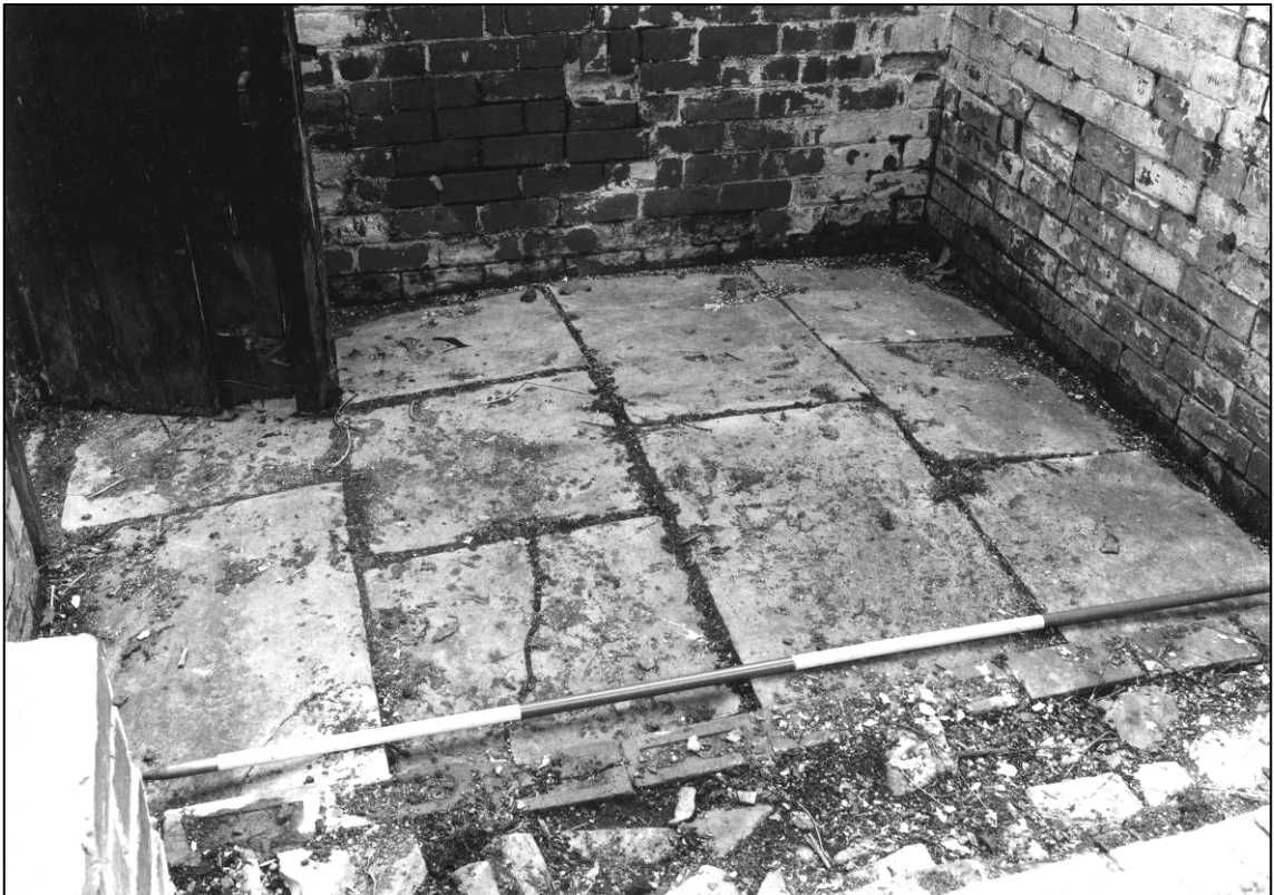
Plate 8: Building N1, floor to west cell, looking E (photo 1/12).
