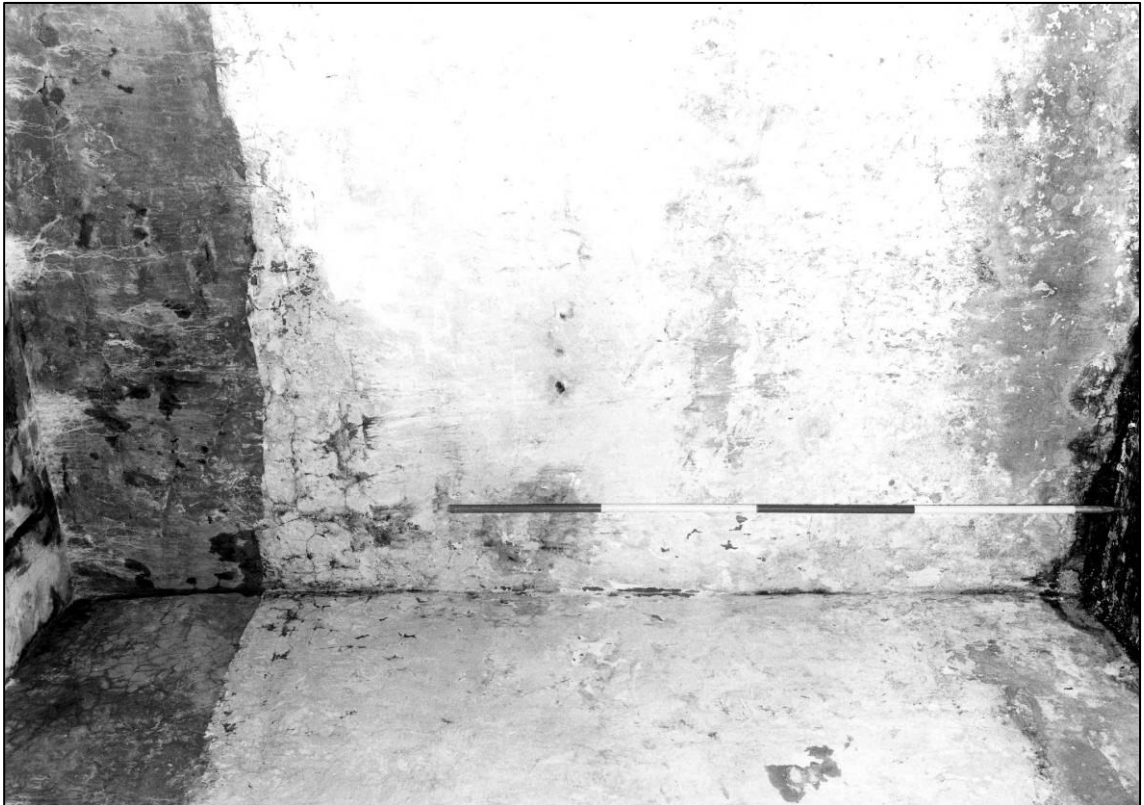
Plate 73: Building S3, interior, looking SW (photo 2/12) (top to left).
