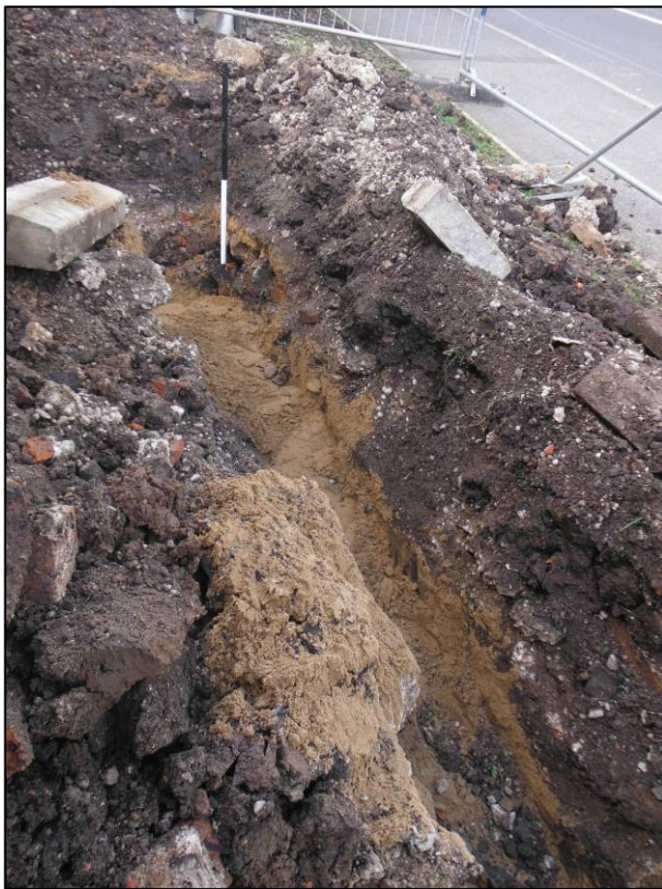
Plate 4: West end of north drainage trench, looking W.
