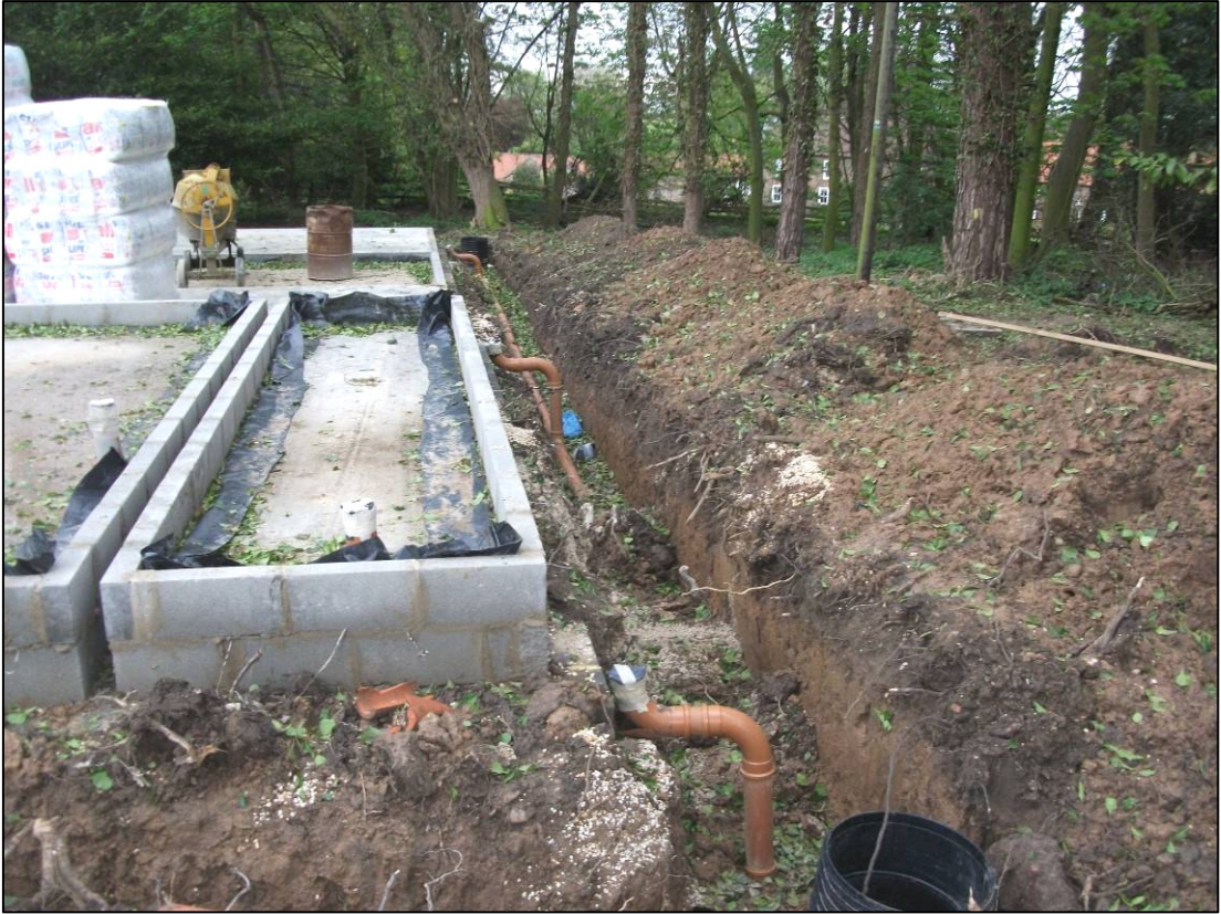
Plate 1: Previously excavated Trench 1, looking NE.
