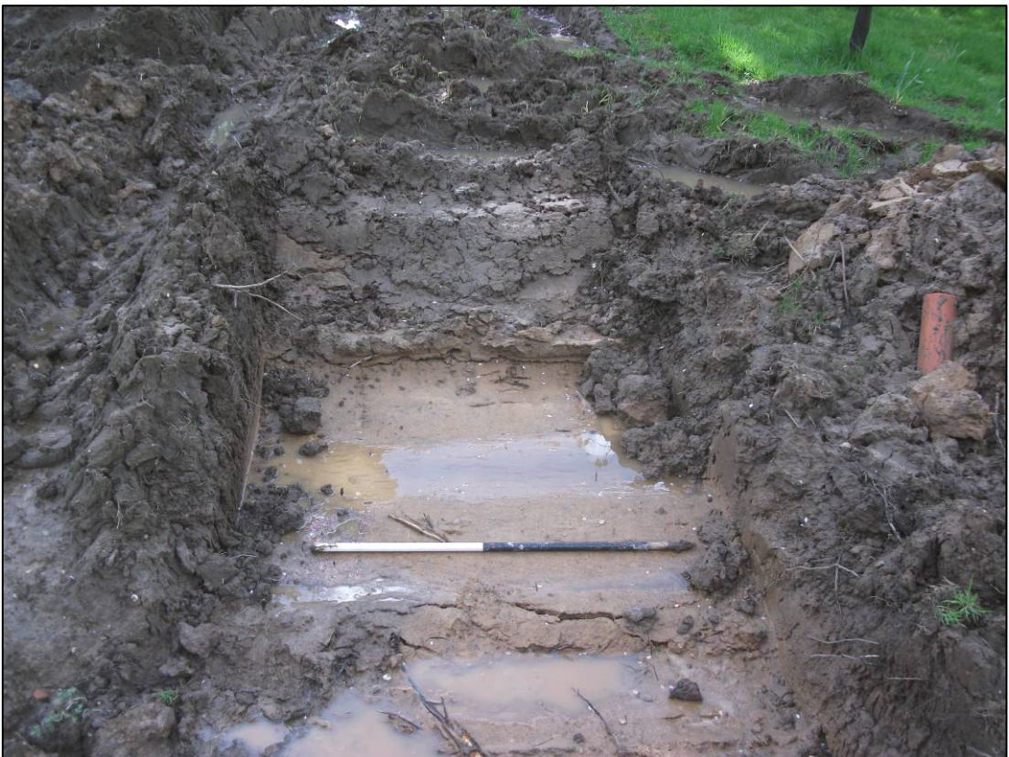
Plate 2: Pit 3, looking SE.
