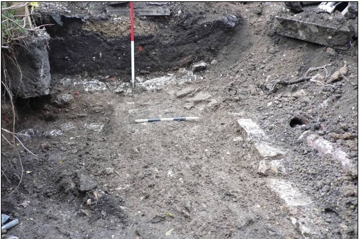
Plate 15: South side of chalk foundation (049) with central sewer pipe (052), with chalk foundation (048) to rear, looking W.
