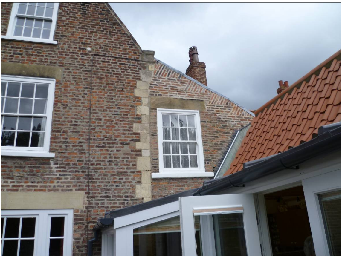
Plate 6: Restored tumbled brickwork of later kitchen extension, after development, looking E.
