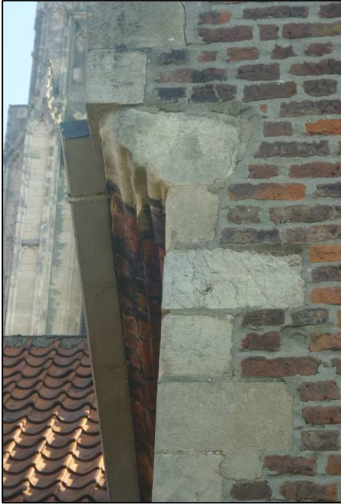
Plate 4: Moulded kneeler and eaves cornice to north side of rear gable, looking E.
