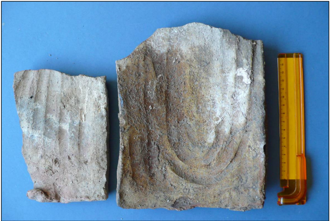
Plate 18: Handmade ceramic roofing tiles with finger marks on top (left) and bottom (right).
