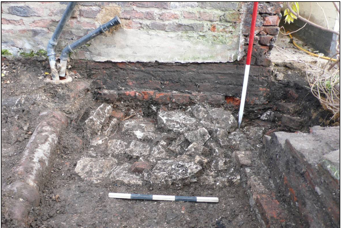
Plate 10: Chalk foundation (030) running beneath SW corner of mid 18th century extension (017) and brick wall (016) forming the southern boundary of the site, looking E.
