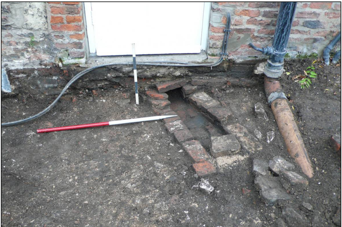
Plate 8: Brick gully (019) passing under wall of presumed mid 18th century kitchen extension (017), looking E.
