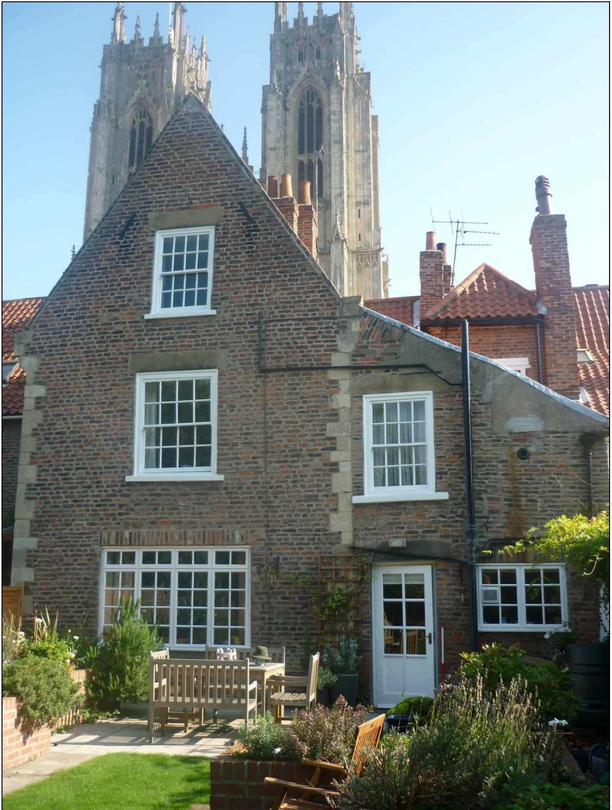
Plate 3: Rear of no. 8 showing west gable of Lambert's c.1700 rear wing to left, and later kitchen extension to right, prior to development, looking W.
