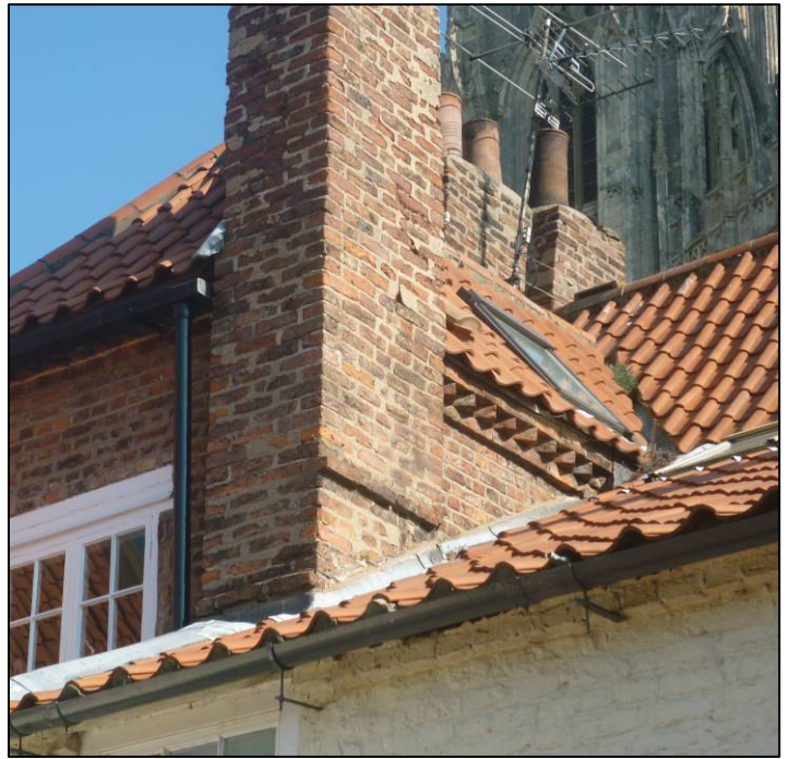
Plate 5: Top of small c.1700 staircase showing cogged brickwork, looking NE.
