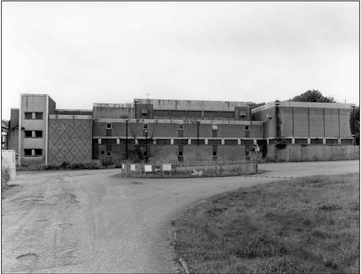
Plate 3: Control Centre complex, E elevation, looking SW (photo 7/4).
