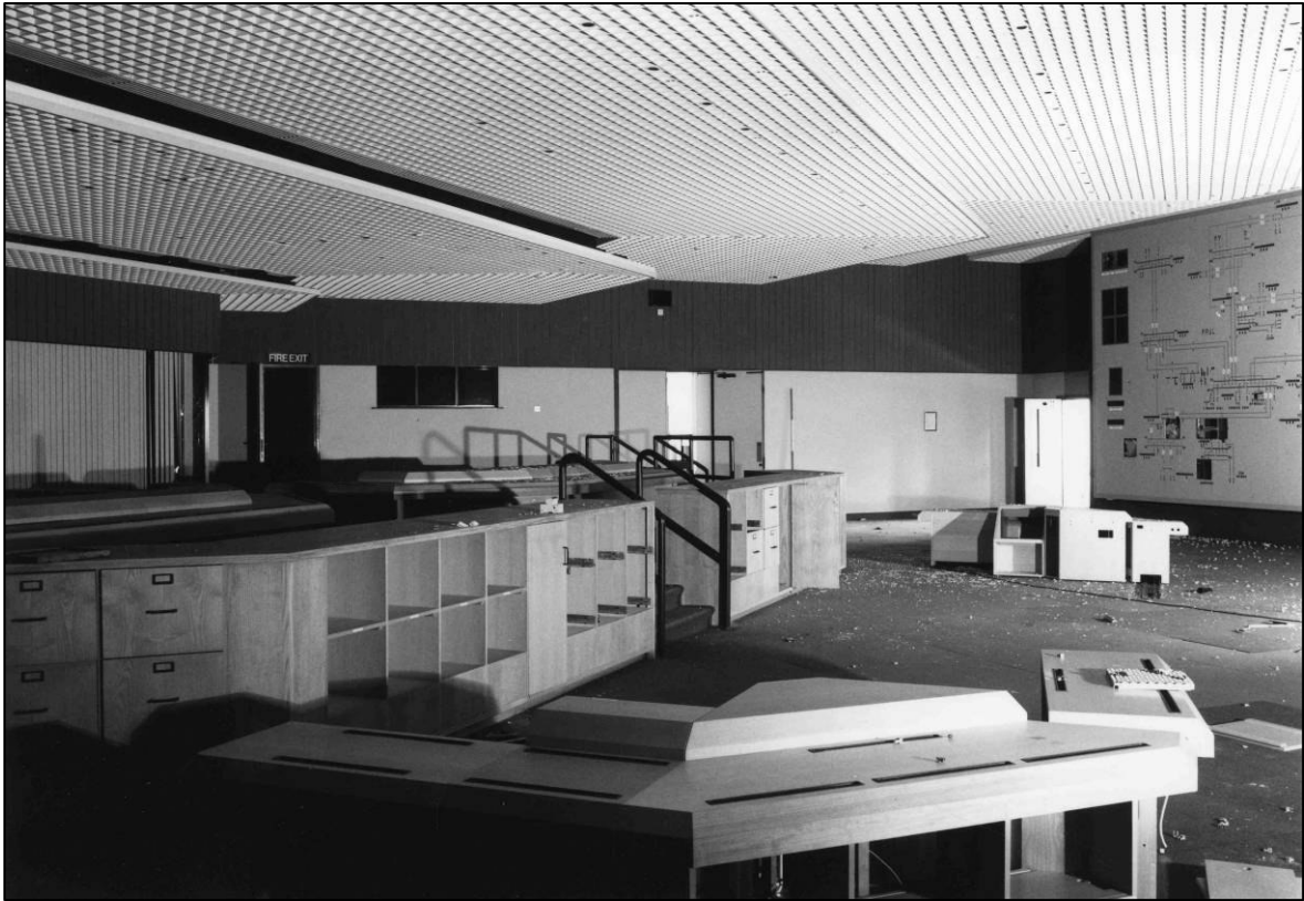
Plate 85: Control room (1F15), control desks, looking S (photo 1/15).
