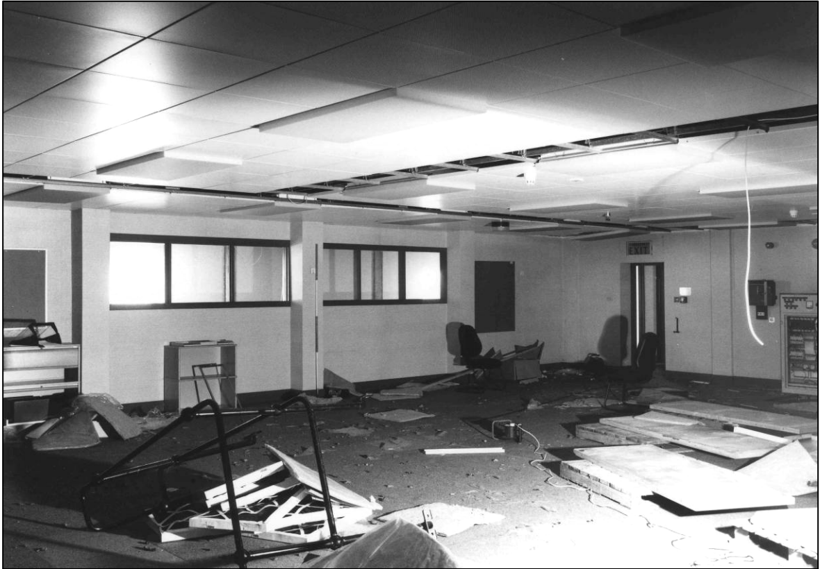
Plate 55: Apparatus Room 4 (GF16), looking E (photo 4/18).
