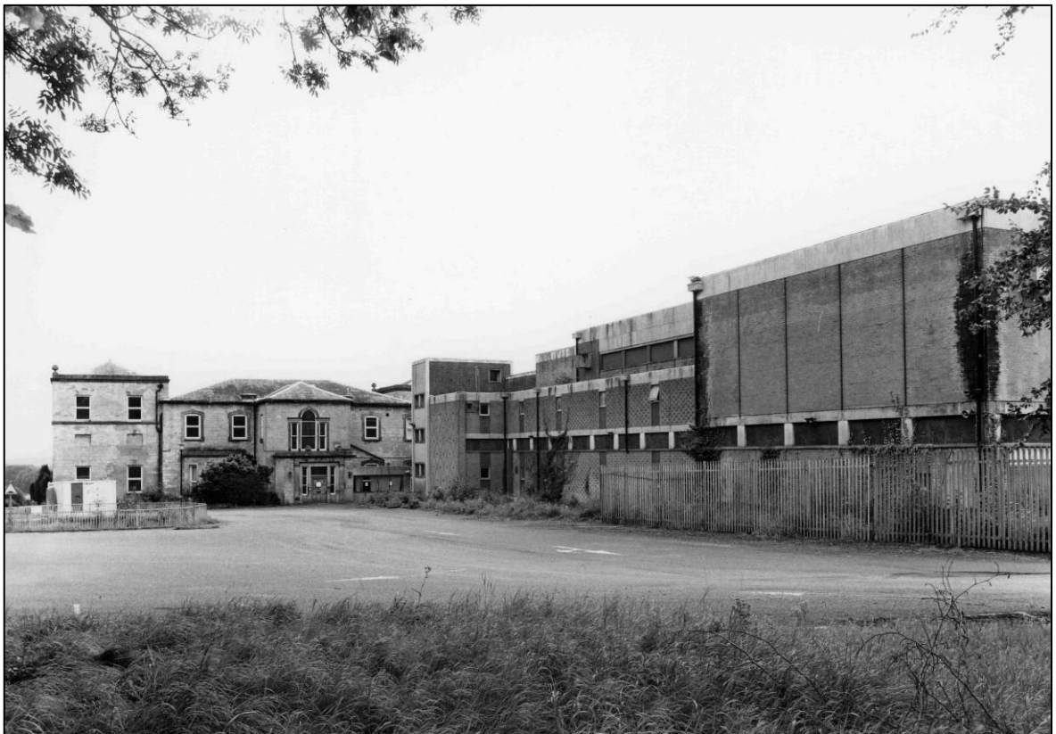
Plate 2: Becca Hall and Control Centre complex, looking S (photo 7/3).
