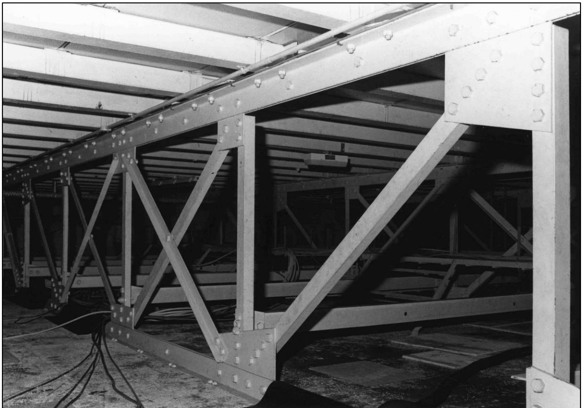
Plate 106: Cable loft area C below Asset Management (1F21), looking N (photo 9/8).
