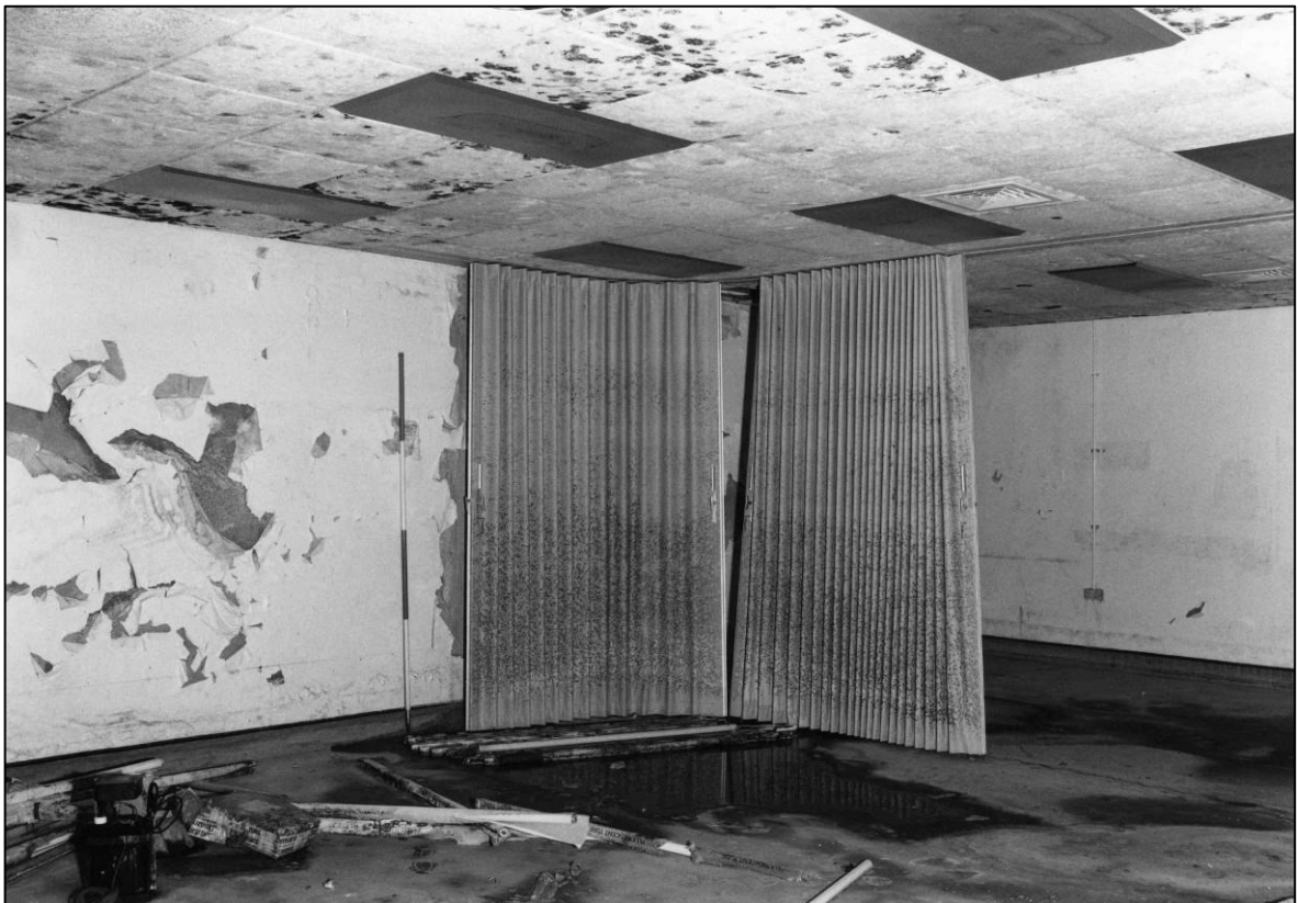
Plate 44: Former Apparatus Room 1 (B10), looking N (photo 6/1).
