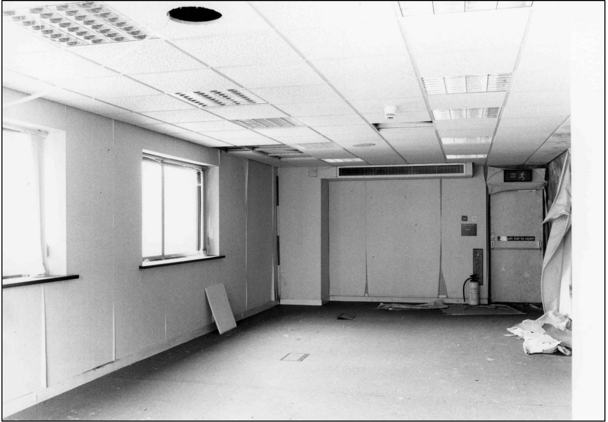
Plate 117: Room 2F1, looking NE (photo 2/15).
