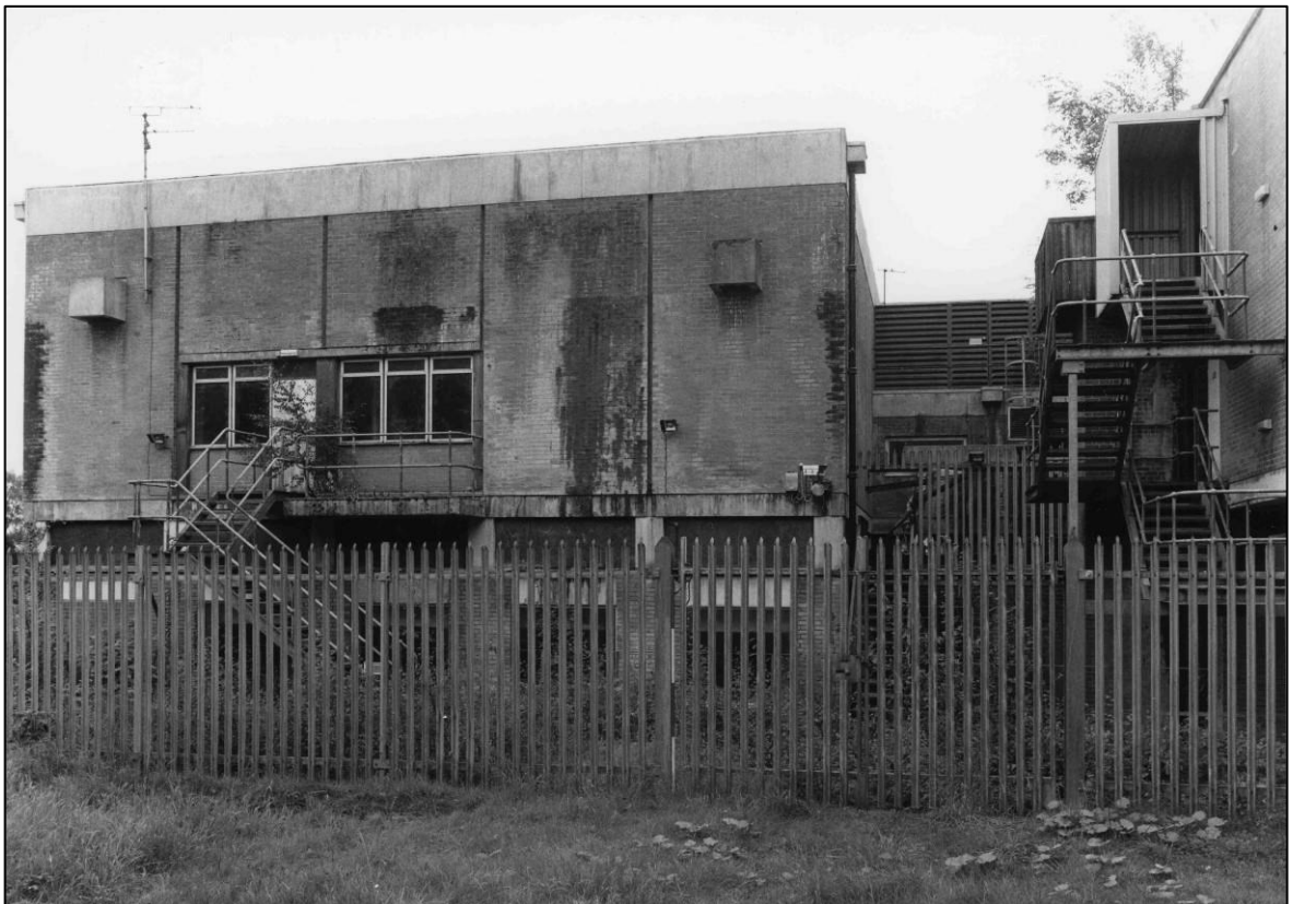
Plate 26: Control Centre complex, E end of N elevation, looking SE (photo 8/1).
