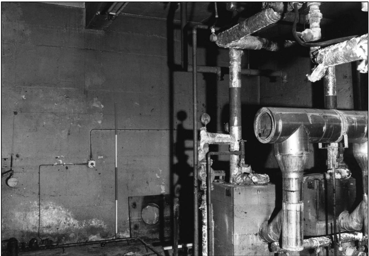
Plate 40: Boiler House (B2), looking N (photo 6/6).
