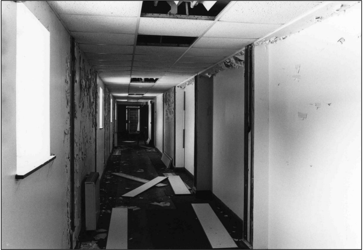
Plate 75: Corridor 1F6, looking SE (photo 3/15).
