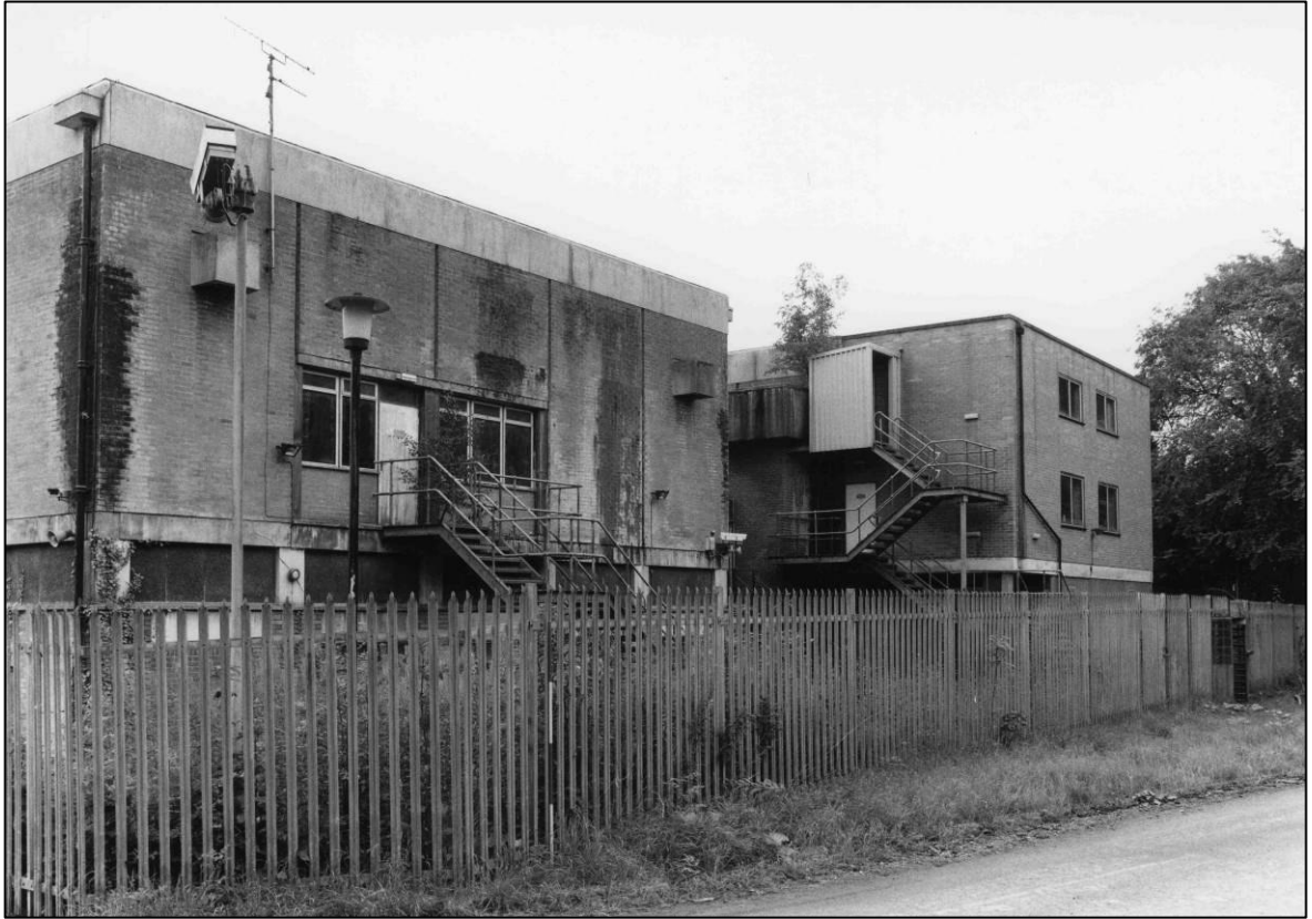
Plate 25: Control Centre complex, N elevation, looking S (photo 7/18).
