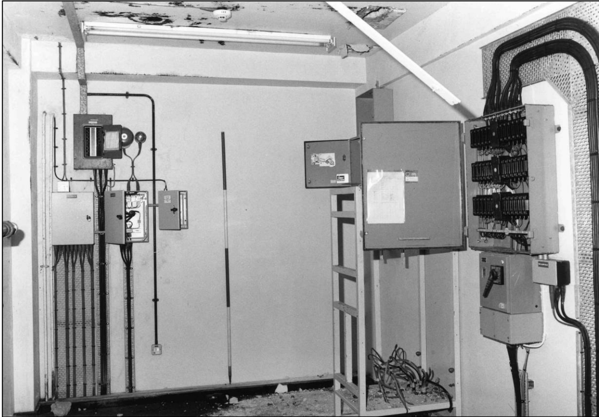
Plate 65: Halon Gas Store (GF29), looking SE (photo 5/11).
