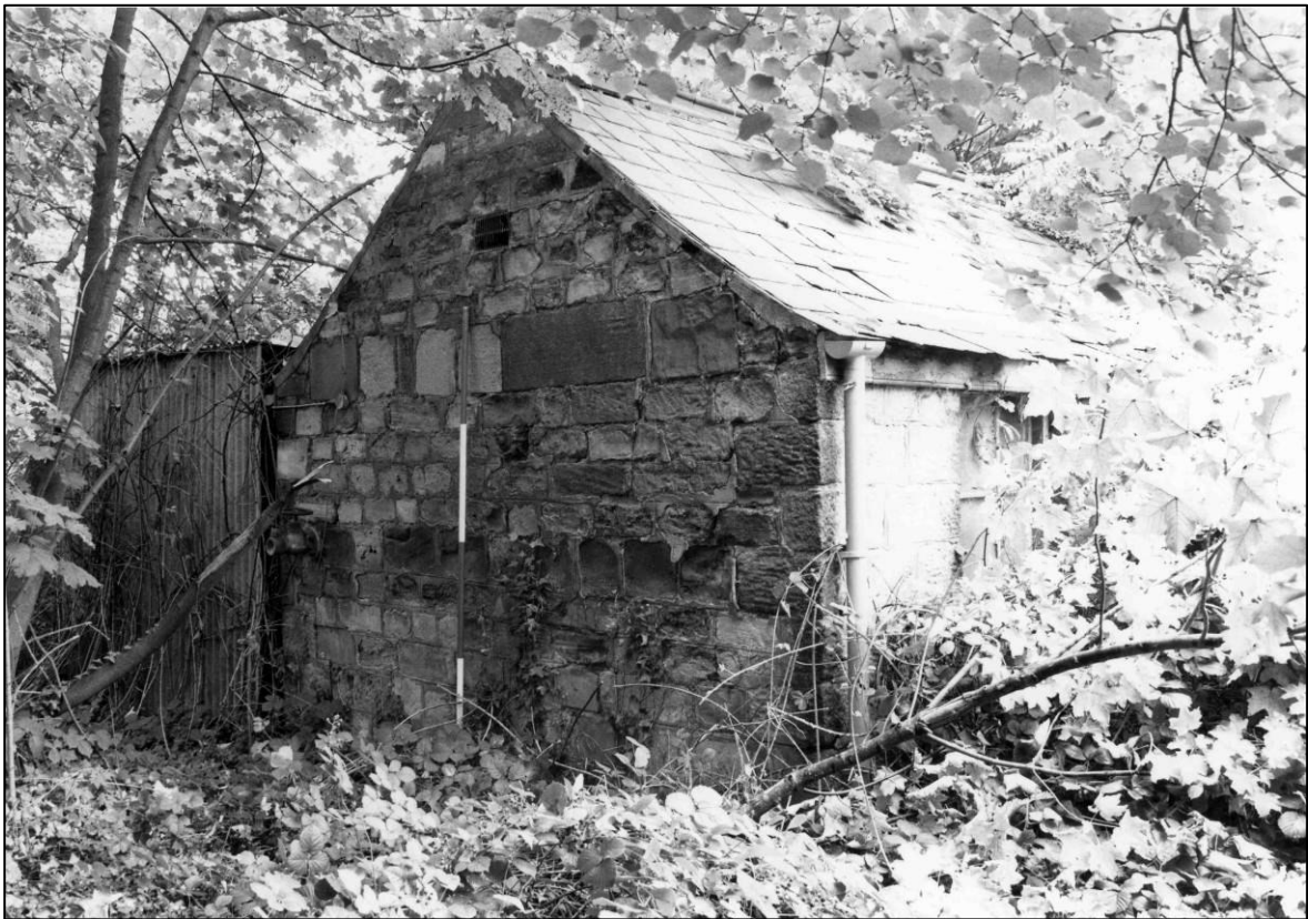
Plate 8: Pump house, looking NW (photo 8/6).
