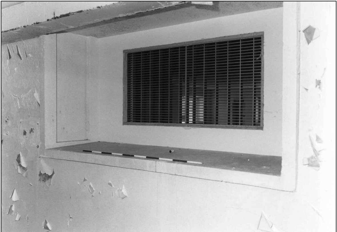
Plate 74: Corridor 1F6, blocked window at S end of W wall, looking S (photo 3/18).
