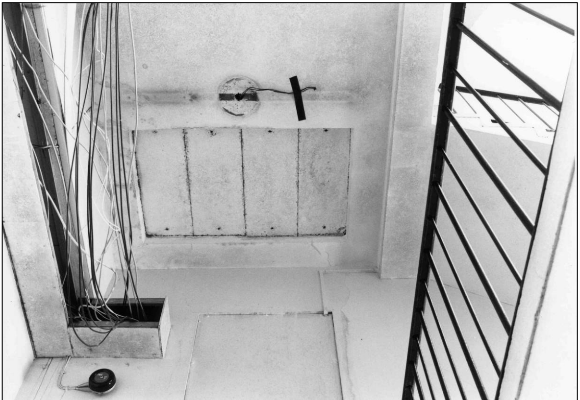
Plate 48: Staircase GF6, detail of ceiling trap, looking NW (photo 4/7).
