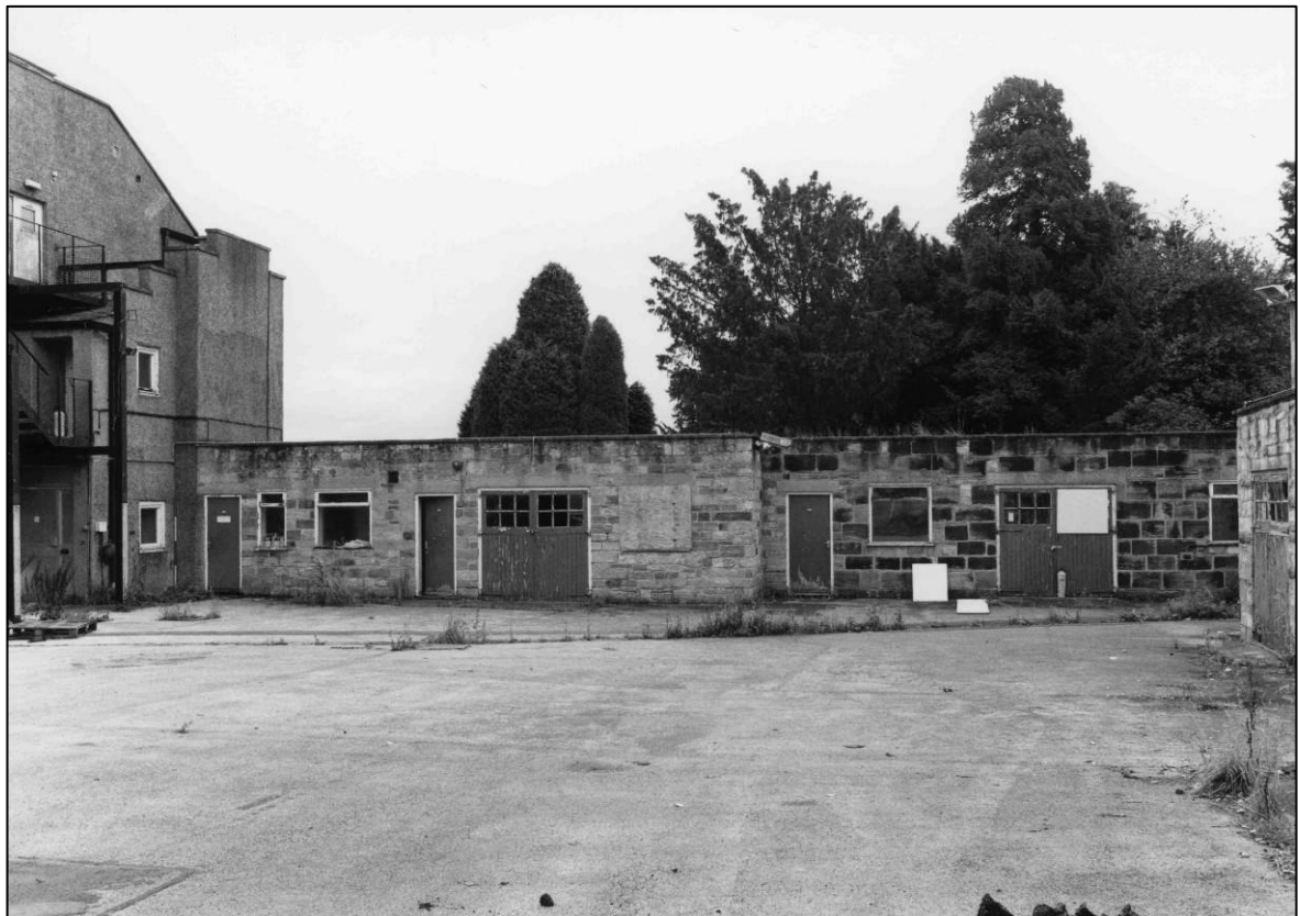
Plate 12: Courtyard buildings (H to J), looking SE (photo 8/17).
