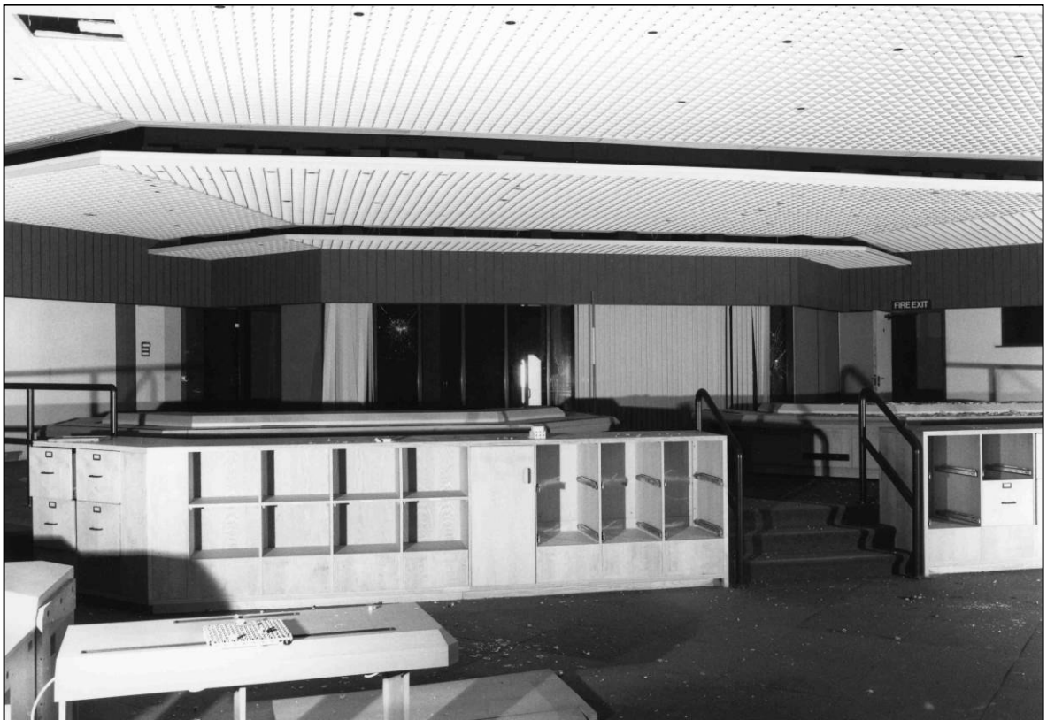
Plate 84: Control room (1F15), control desks, looking E (photo 1/13).
