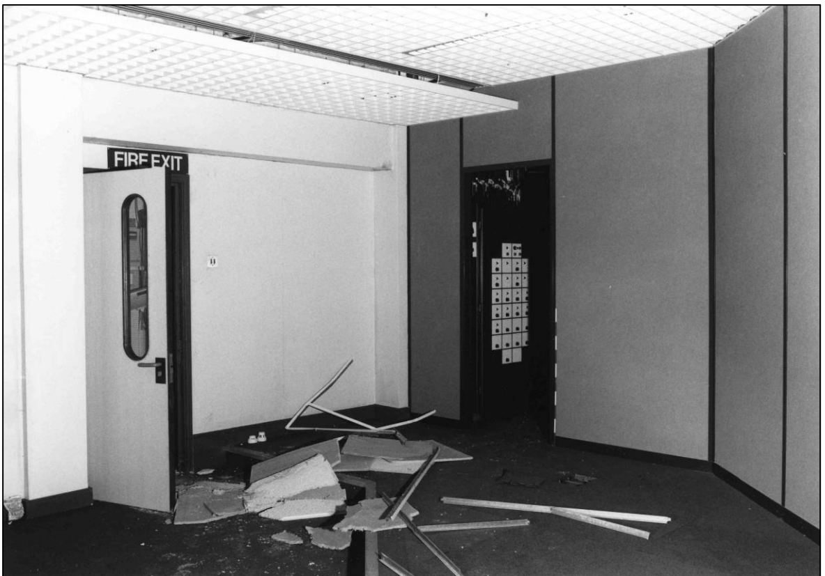
Plate 98: Triangular office (1F16), looking NE (photo 2/10).
