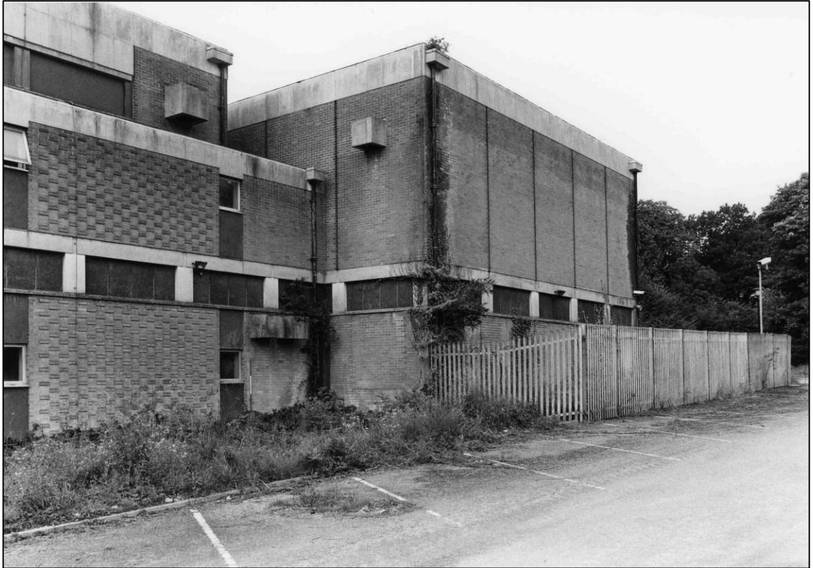
Plate 21: Control Centre complex, N end of E elevation, looking W (photo 7/12).
