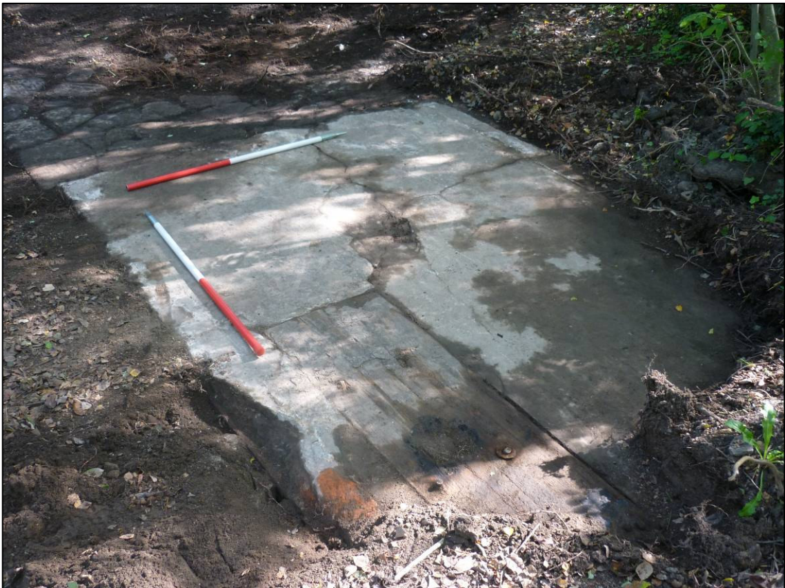
Plate 2: Exposed concrete base, looking E.
