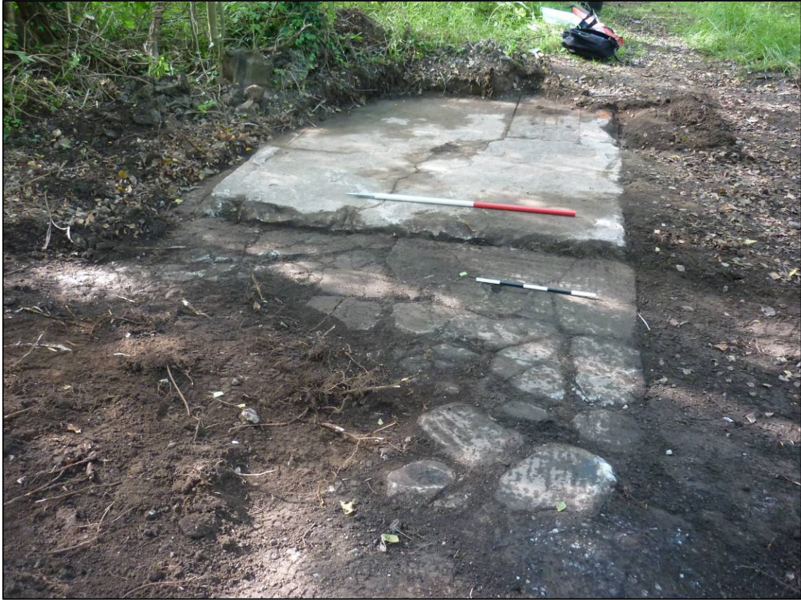
Plate 3: Exposed concrete base and fractured concrete surface, looking SW.
