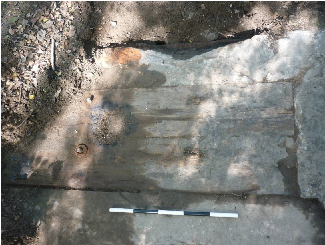
Plate 4: Timber in concrete base.
