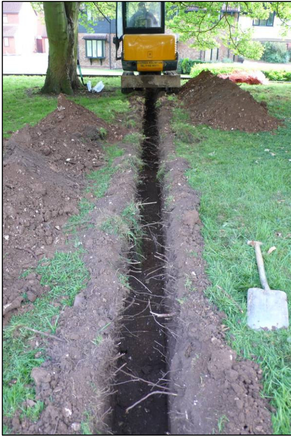
Plate 1: Excavations in progress, looking north-east.
