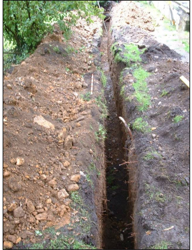
Plate 2: Trench 1 running south on east side of vestry, looking south.
