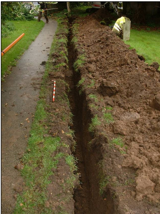
Plate 3: Trench 1 running south on west side of path, looking south.
