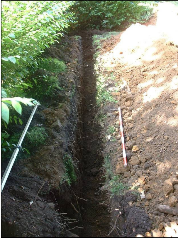
Plate 1: Trench 1 running north from vestry, looking north.
