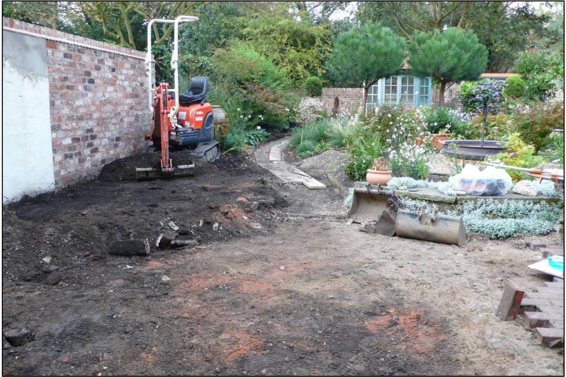
Plate 3: Topsoil strip in progress, looking W.
