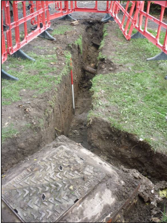
Plate 1: Trench 1, looking NE.
