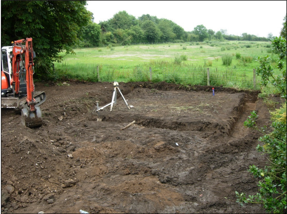
Plate 6: Phase 2 garage foundations, looking E.
