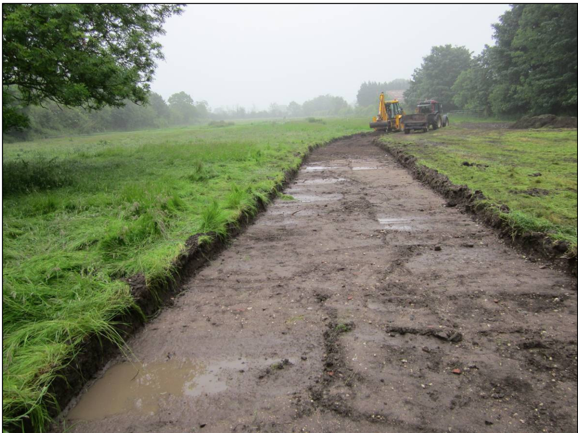
Plate 7: Phase 3 access road under excavation, looking E.
