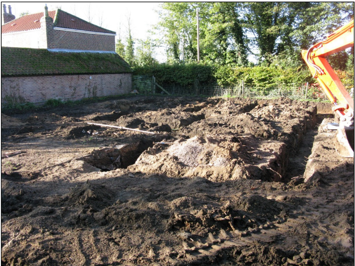
Plate 3: General view of Phase 2 house foundations under excavation, looking SW.
