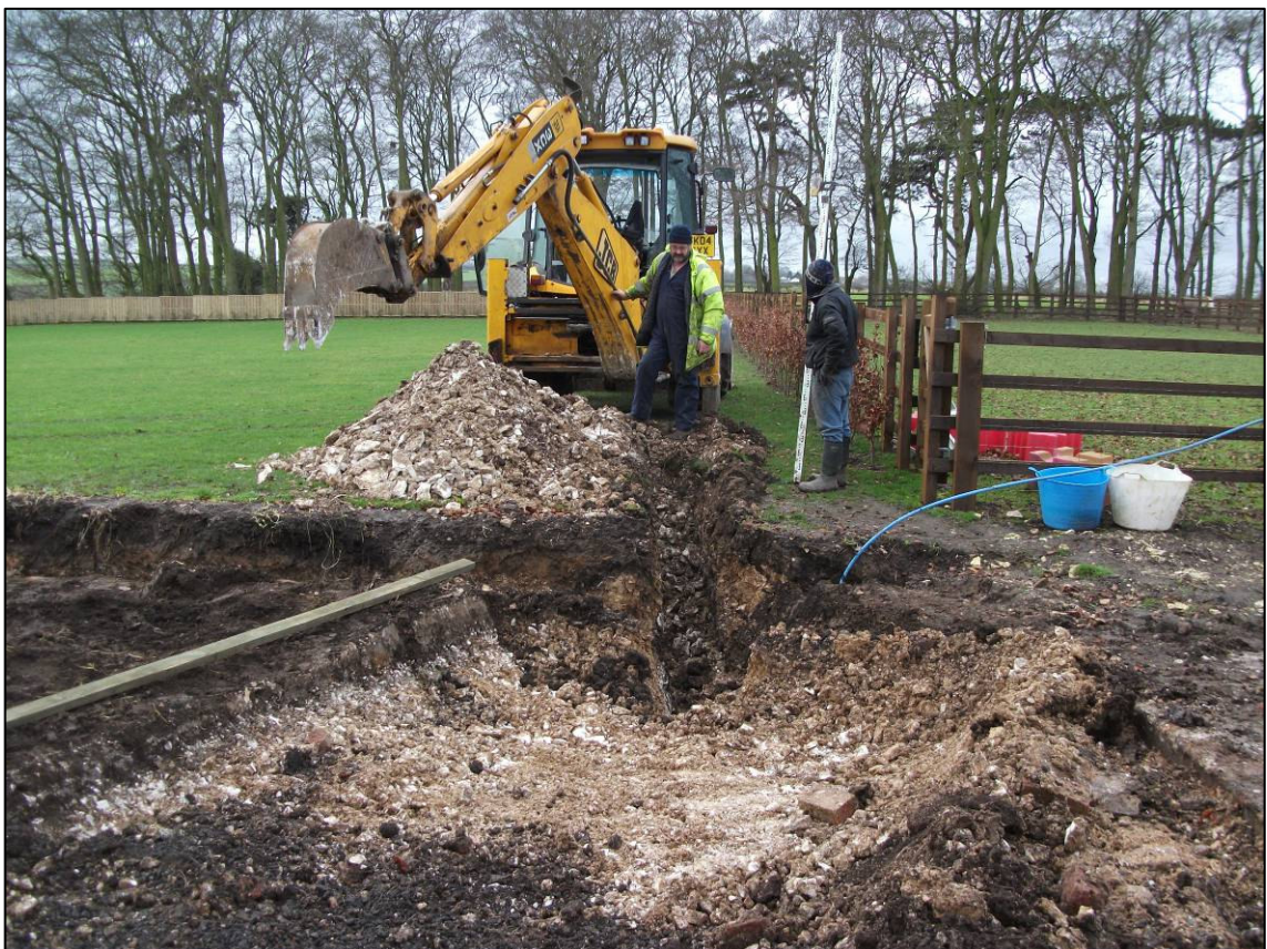
Plate 2: Start of excavations for drainage trench, looking W.
