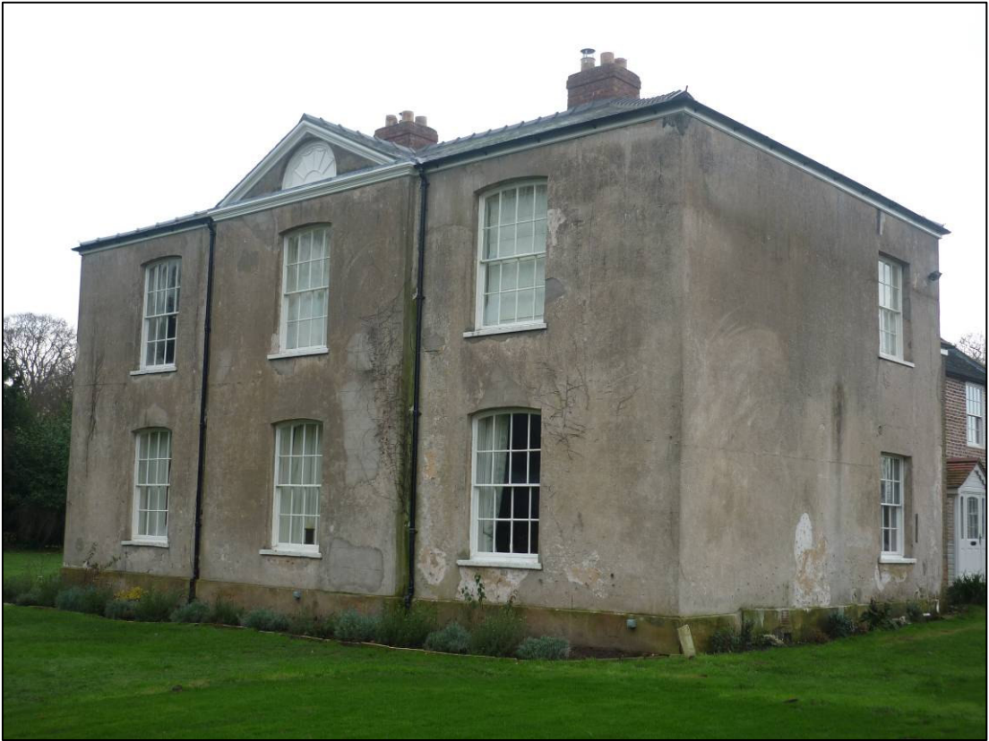
Plate 1: Principal (east) elevation of Sutton Hall, looking SW (photo 1/65).
