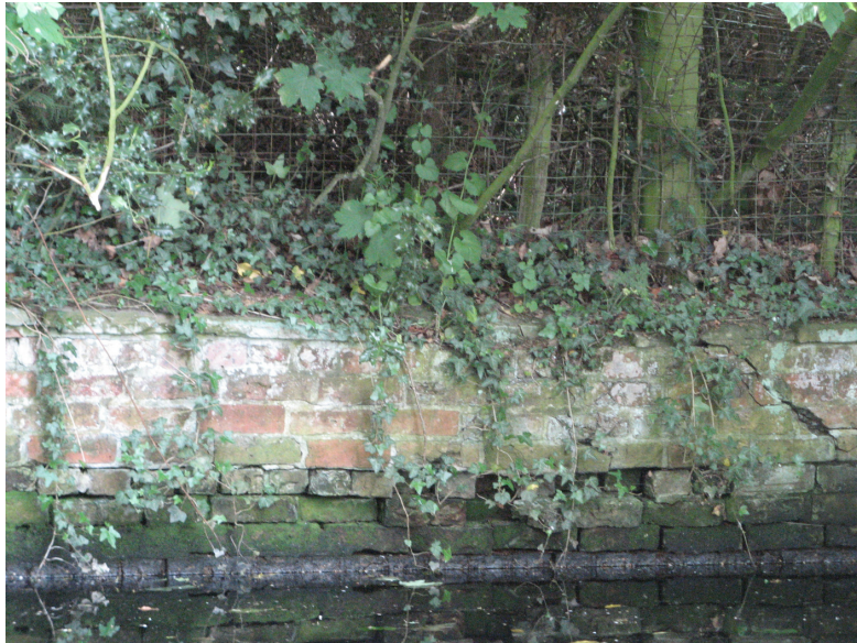
Plate 2 East wall (looking west to east)
