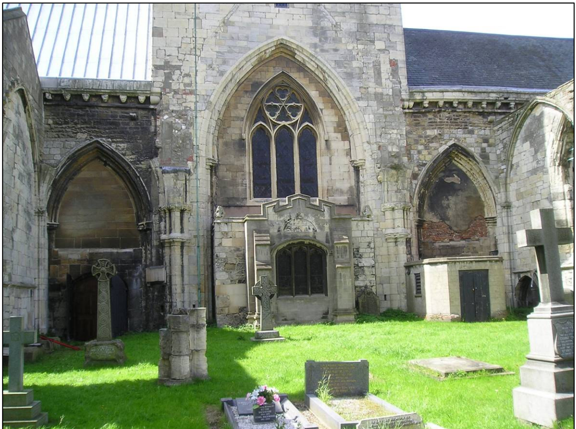
Plate 2: Interior of west end of ruined choir, looking north-west.
