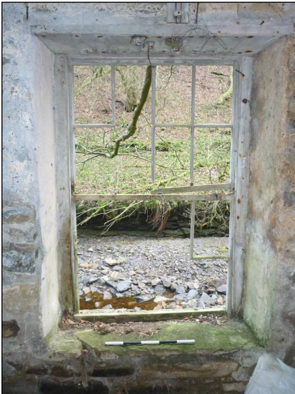
Plate 64: Power house (Site 32), west window in south elevation, looking S (photo 8/780).
