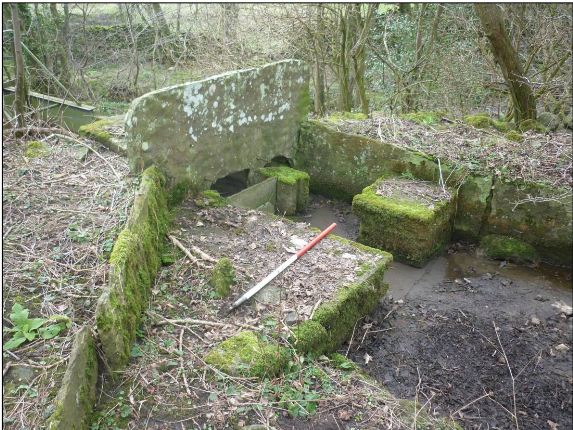
Plate 24: Mill Gill survey area, sluice arrangement at south end of header tank (Site 29f), looking S (photo 8/753).
