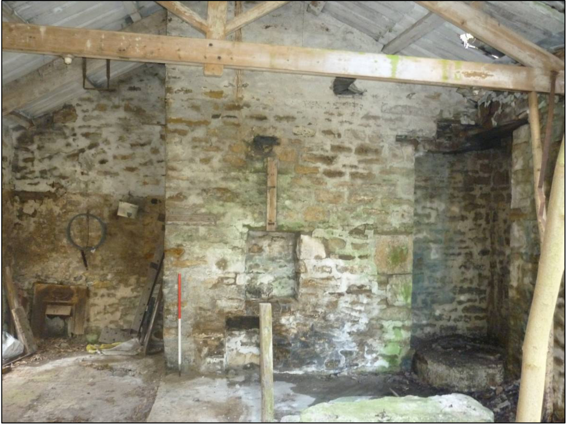
Plate 66: Power house (Site 32), west internal elevation, looking W (photo 8/784).
