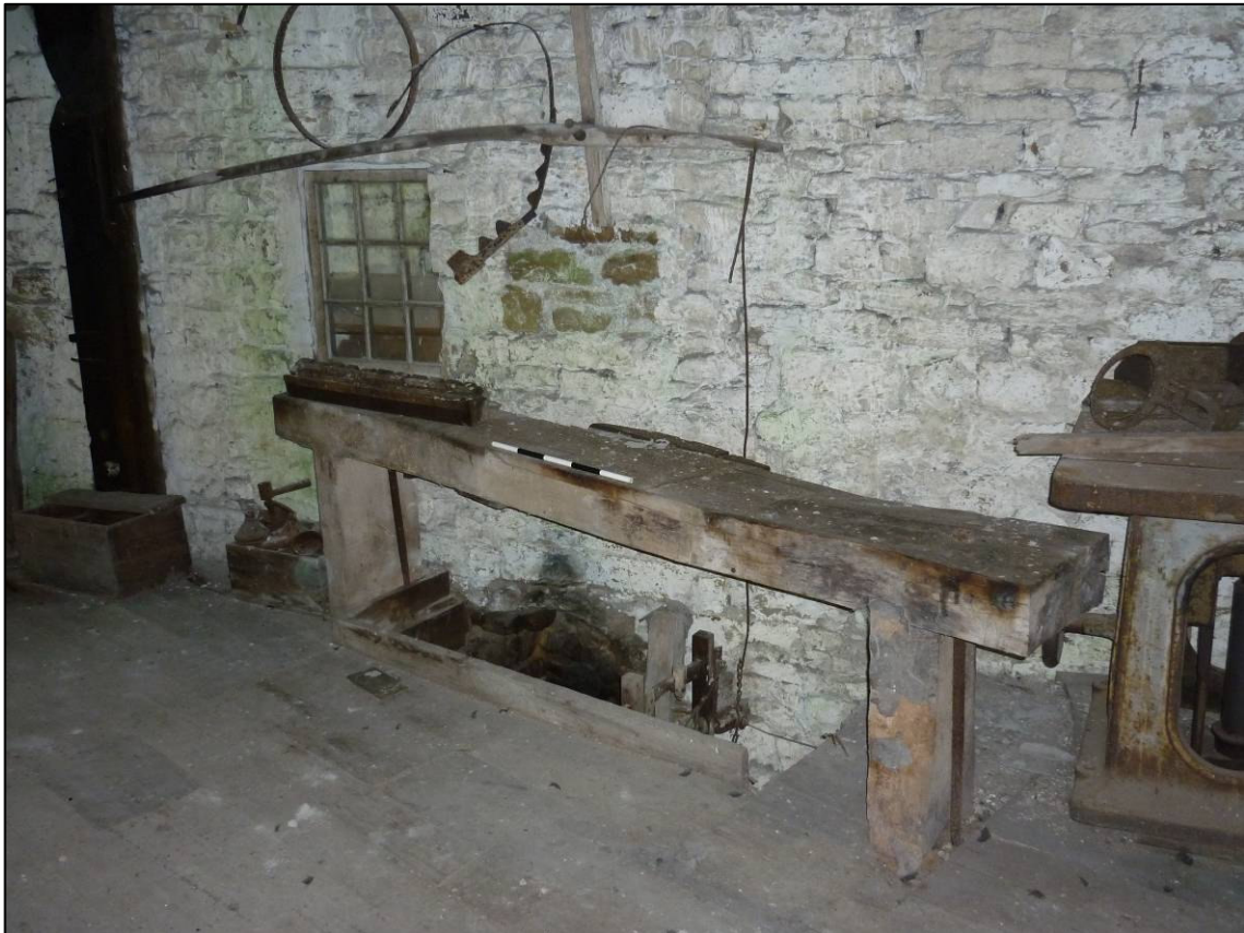
Plate 48: Garage (Site 36b), bench structure lever etc, north wall (elevation 19) of first floor room 1F12, looking N (photo 7/916).
