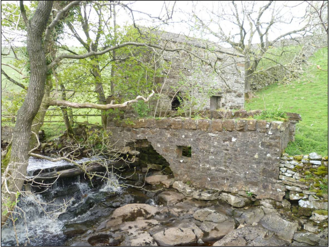
Plate 5: Leas House survey area, 1908-10 collecting chamber and weir (Sites 8a and 8c), looking N (photo 9/998).
