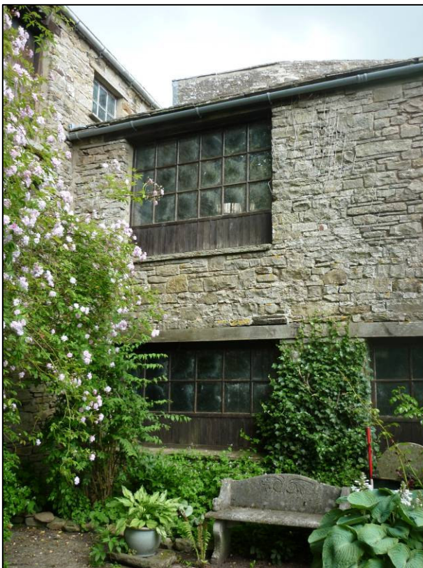
Plate 42: Garage (Site 36b), west end of south external elevation (10), looking N (photo 5/567).
