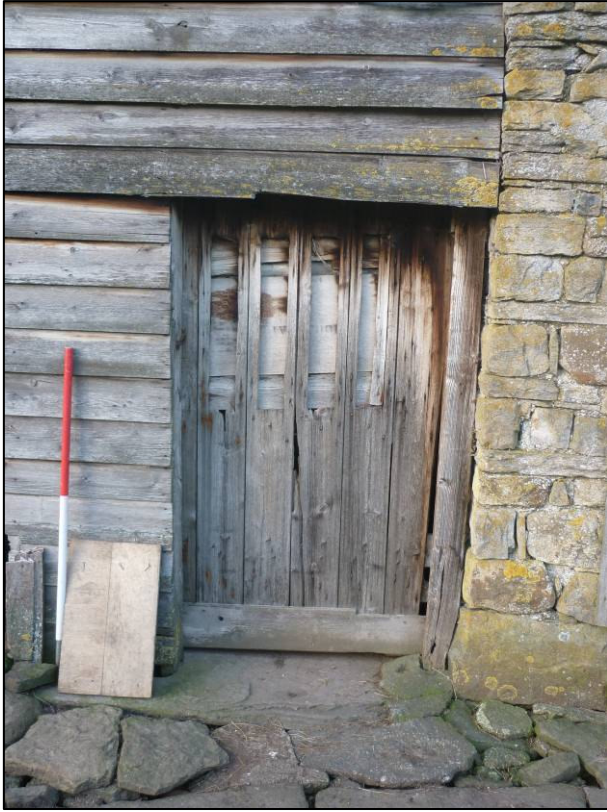
Plate 72: Poultry house (Site 33), doorway to central south, looking N (photo 3/724).
