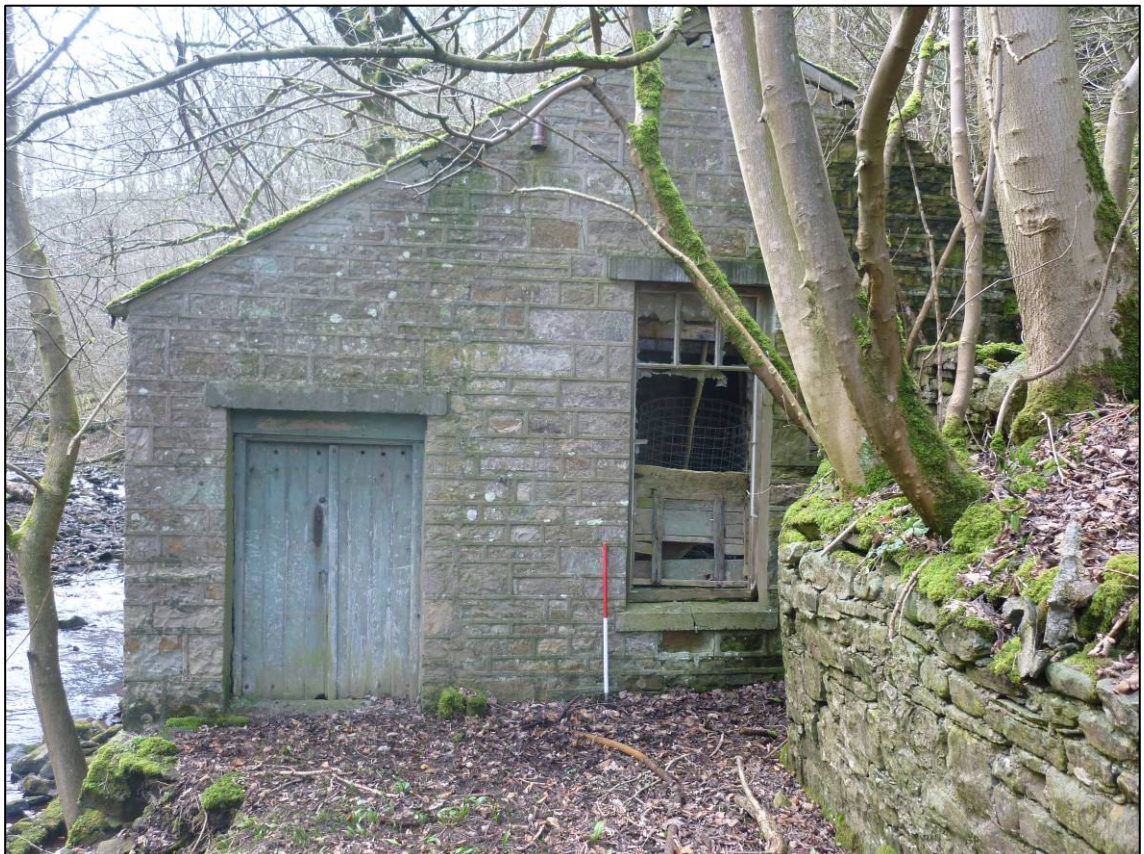
Plate 62: Power house (Site 32), east external elevation, looking W (photo 8/808).
