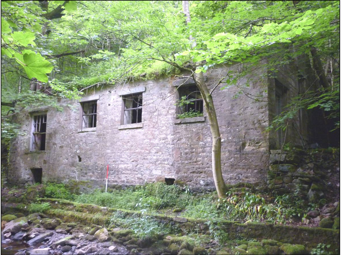
Plate 61: Power house (Site 32), south external elevation, looking NE (photo 6/800).
