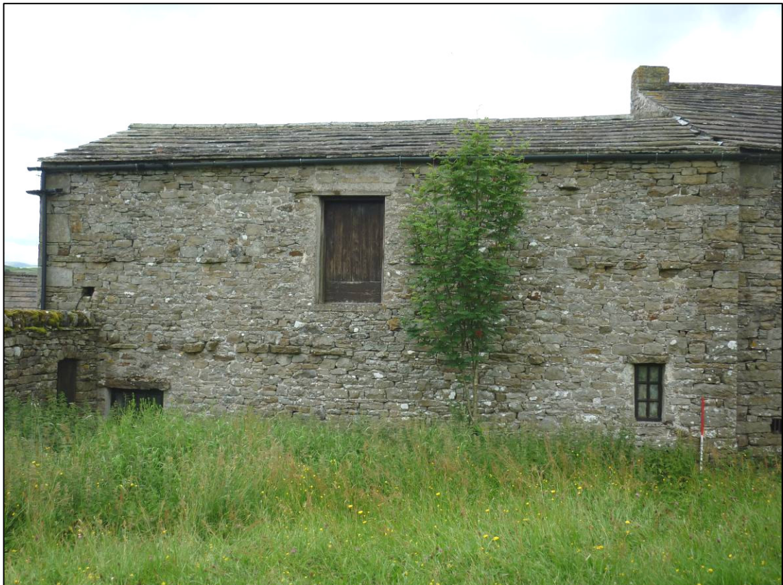
Plate 56: Barn range (Site 36d), north external elevation (6), looking S (photo 5/547).
