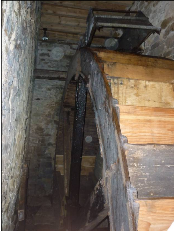
Plate 57: Mill (Site 36a), waterwheel and launder in wheelhouse (G1), looking N (photo 7/174).
