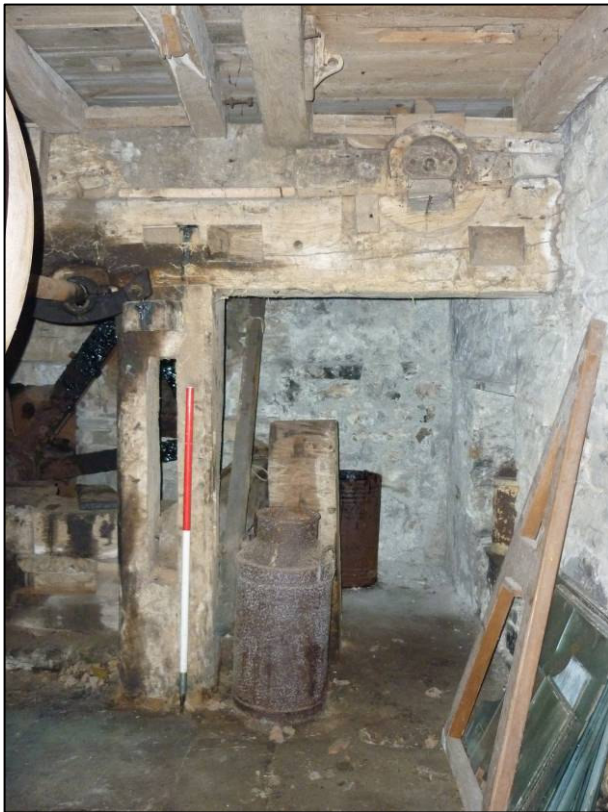
Plate 59: Mill (Site 36a), north post of frame and related beams in ground floor room G2, looking W (photo 7/039).
