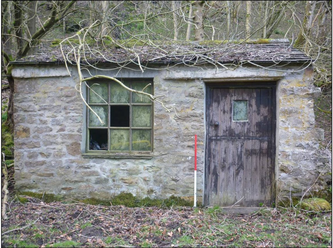
Plate 16: Mill Gill survey area, building east of the power house (Site 31), looking N (photo 8/815).
