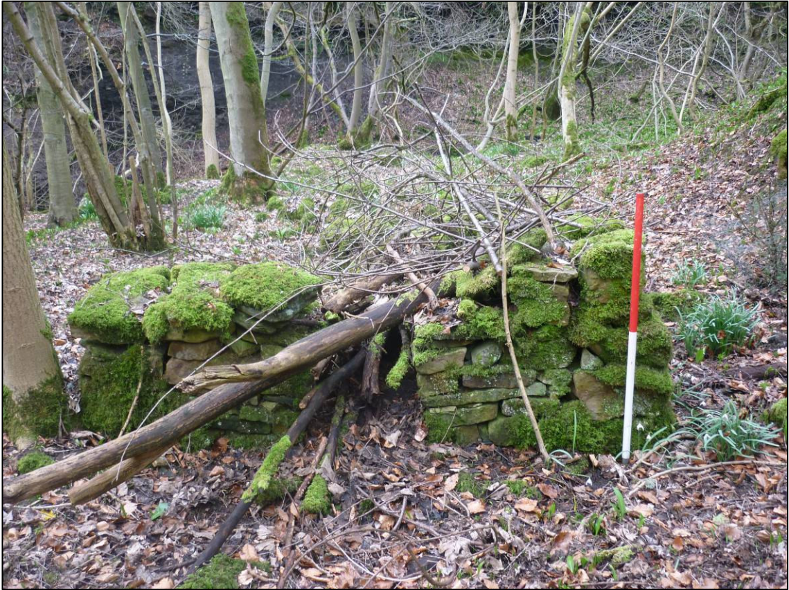
Plate 14: Mill Gill survey area, ruined structure (Site 21), looking W (photo 8/764).
