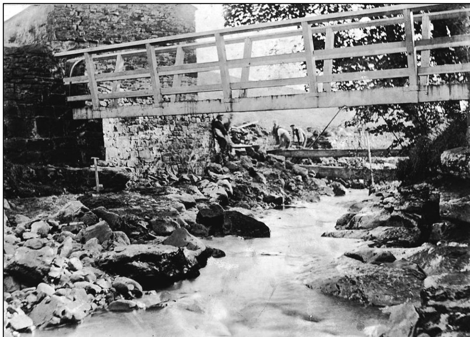
Top left: early photograph of original Mill Gill power house before 1913 expansion. Top right: pipeline to Mill Gill power house under construction. Bottom: collection chamber above Mill Gill Force under construction, c.1910. Source: Kershaw collection.
