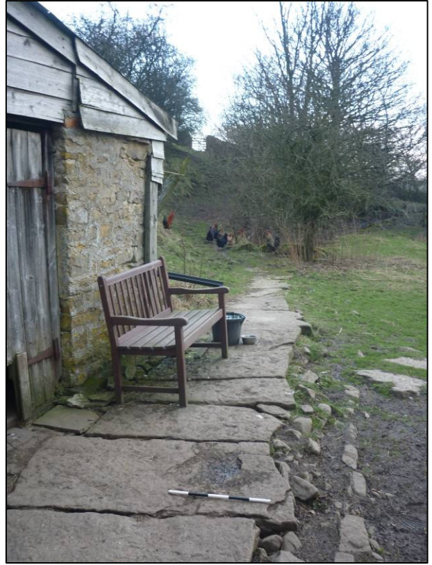
Plate 73: Poultry house (Site 33), flagged culvert of mill race, looking E (photo 8/836).
