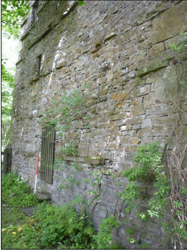
Plate 29: Mill (Site 36a), west external elevation (2), looking NE (photo 5/553).
