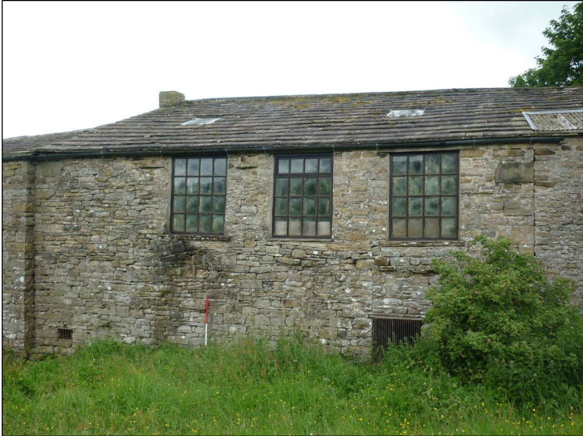
Plate 49: Kiln range (Site 36c), north external elevation (5), looking S (photo 5/544).
