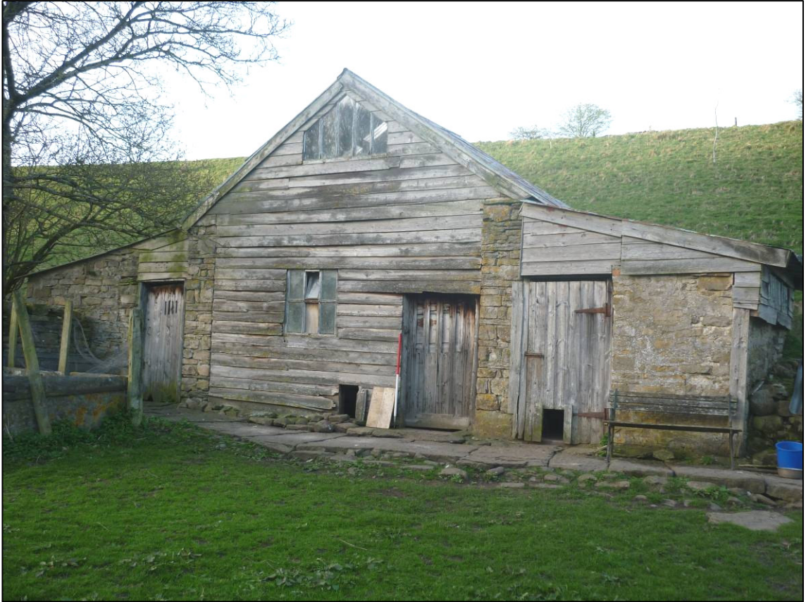
Plate 70: Poultry house (Site 33), south external elevation, looking N (photo 3/722).
