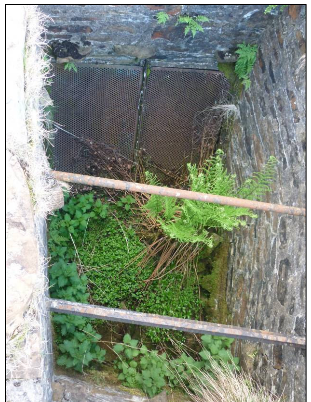
Plate 7: Leas House survey area, interior of 1913 collecting chamber (Site 12d) (photo 4/999).
