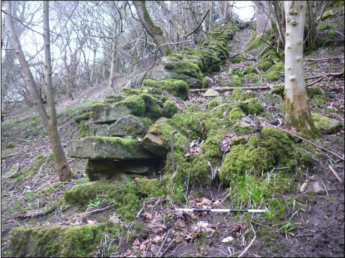
Plate 63: Mill Gill survey area, bolts on route of pipeline to power house (Site 30b), looking N (photo 8/776).
