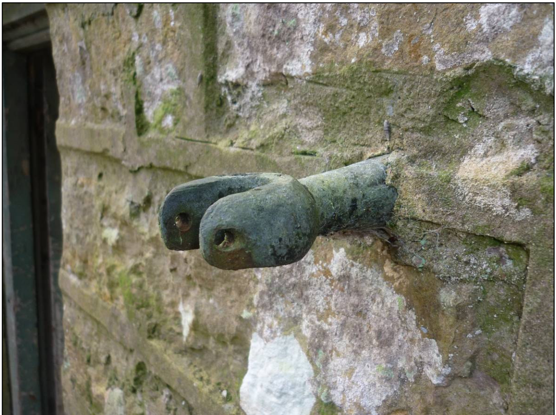
Plate 69: Power house (Site 32), fitting to external east gable (photo 8/803).
