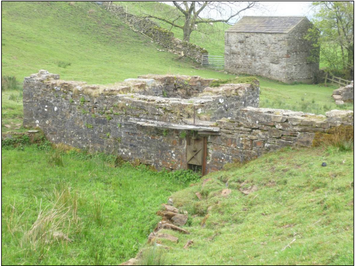
Plate 10: Leas House survey area, 1913 collecting chamber (Site 12d), looking E (photo 9/991).
