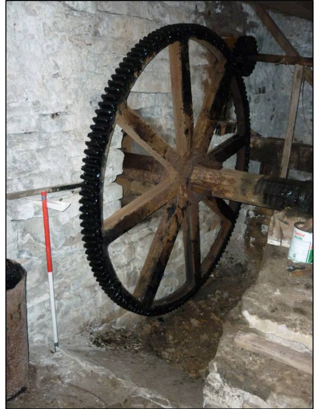
Plate 58: Mill (Site 36a), pit wheel in ground floor room G2, looking NW (photo 7/023).
