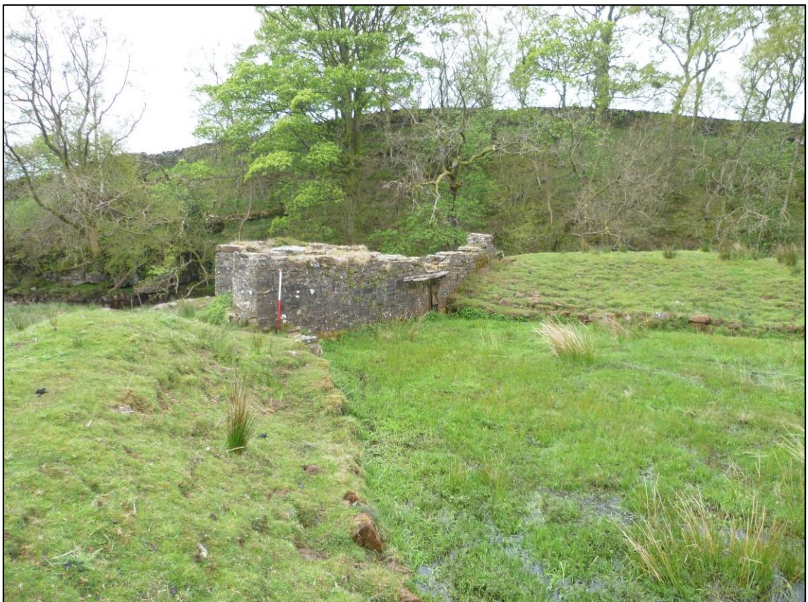
Plate 11: Leas House survey area, 1913 collecting chamber and pond (Sites 12c and 12d), looking S (photo 9/973).
