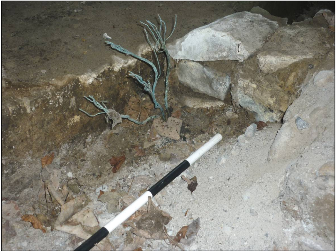
Plate 68: Power house (Site 32), 3-phase and neutral supply wiring to west of concrete base, looking E (photo 8/802).
