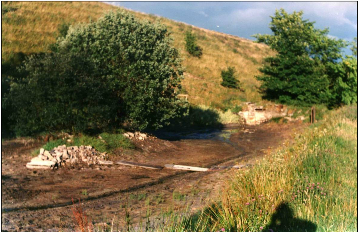
Top: Rebuilding leat adjacent to the power house in 1986.
