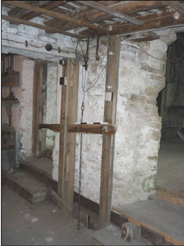
Plate 34: Mill (Site 36a), launder sluice control on south wall (elevation 11) of first floor room 1F10, looking S (photo 7/978).
