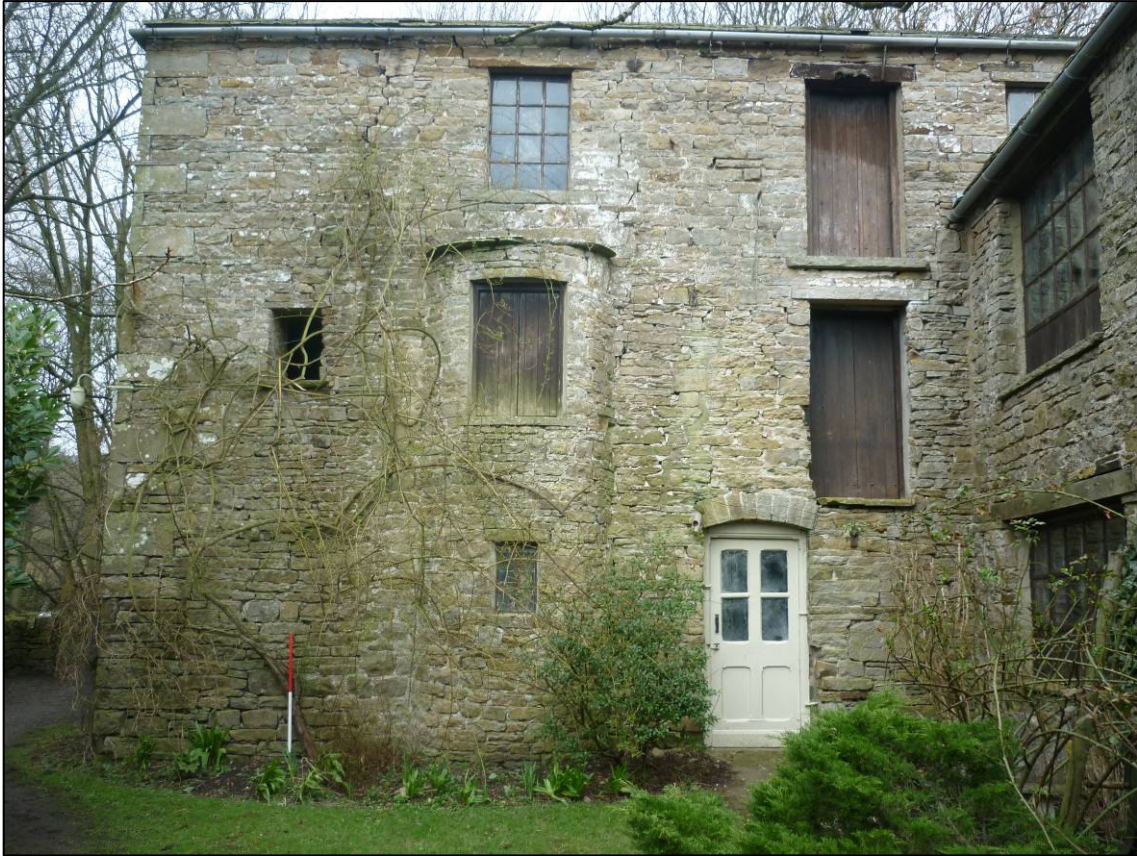
Plate 27: Mill (Site 36a), south external elevation (1), looking N (photo 8/745).
