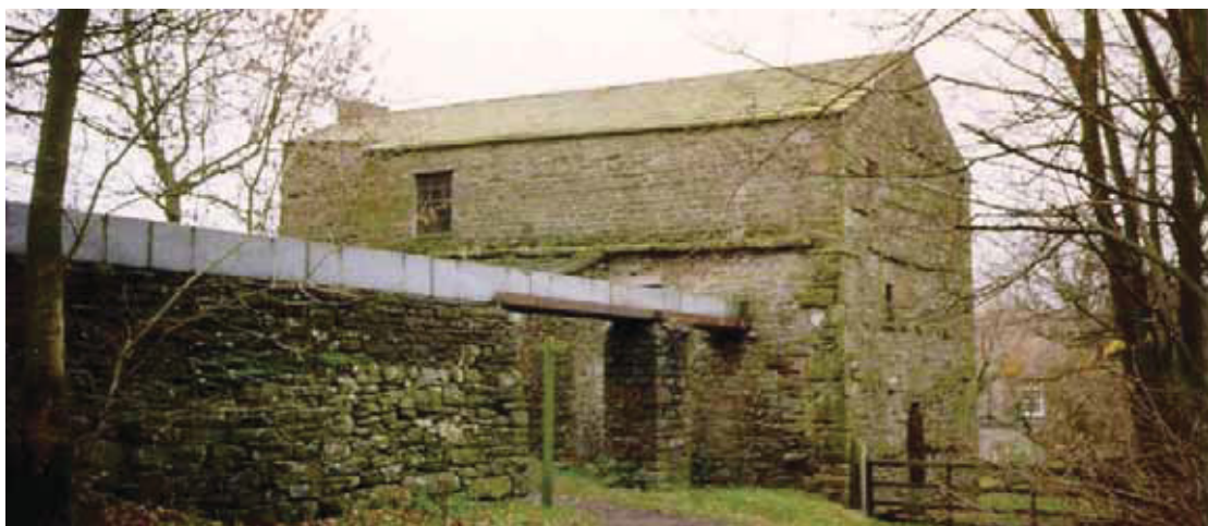
Mill building looking south east. 1997
