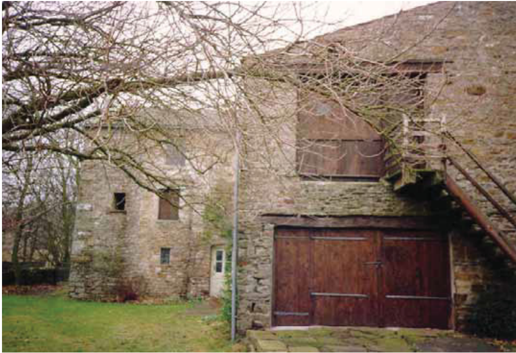
Mill building looking northwest. 1997
