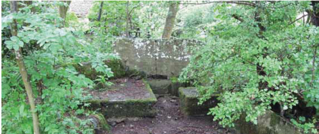
Sluice above overhead mill race. 2010
