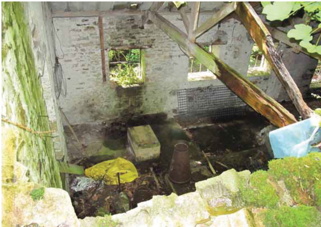
Turbine house interior. 2010
