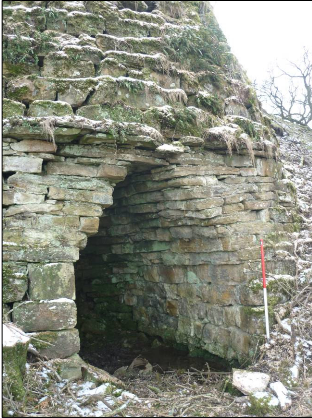
Plate 7: Draw-hole arch, looking SE (photo 1/608).
