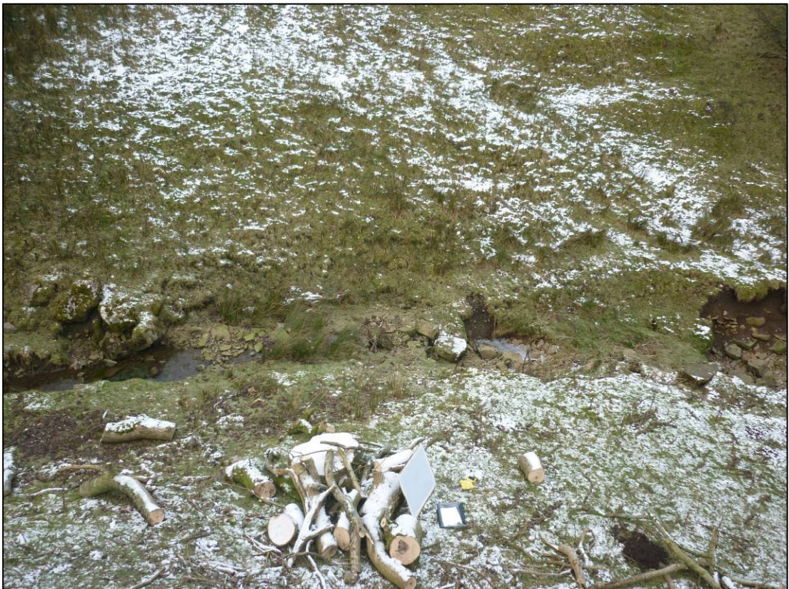
Plate 2: Ruined bridge or culvert, looking W (photo 1/641).
