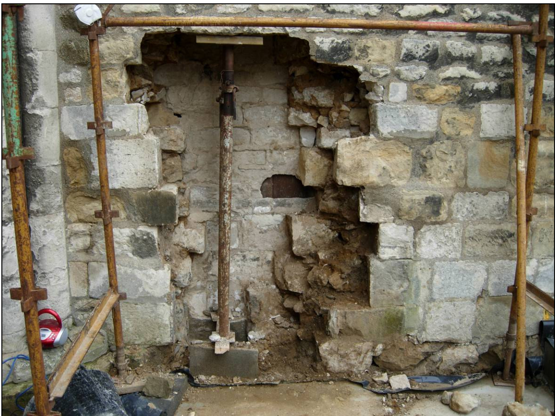
Plate 7: Cutting through infill of blocked arcade, looking north.
