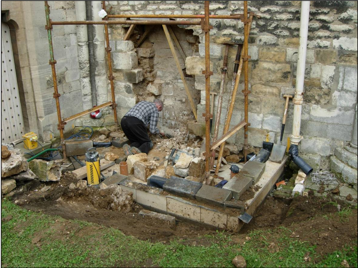
Plate 10: Construction work in progress, after additional landscaping, looking north-west.
