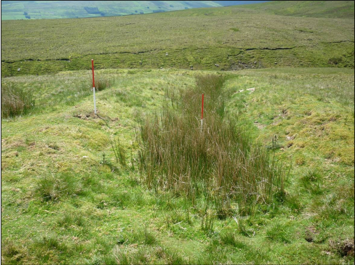
Plate 21: North end of zig-zag flue extension (SAR 01), looking S (photo 1/371).
