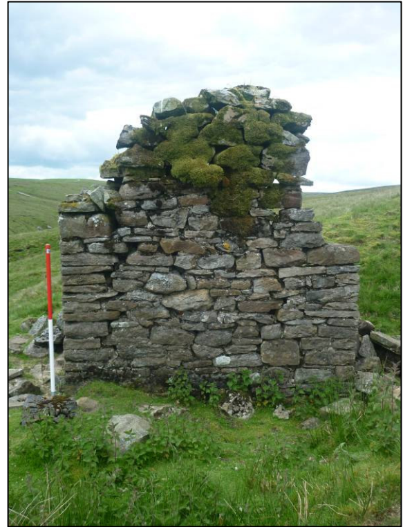
Plate 19: East side of chimney (SAR 04, elevation 2), looking W (photo 1/380).
