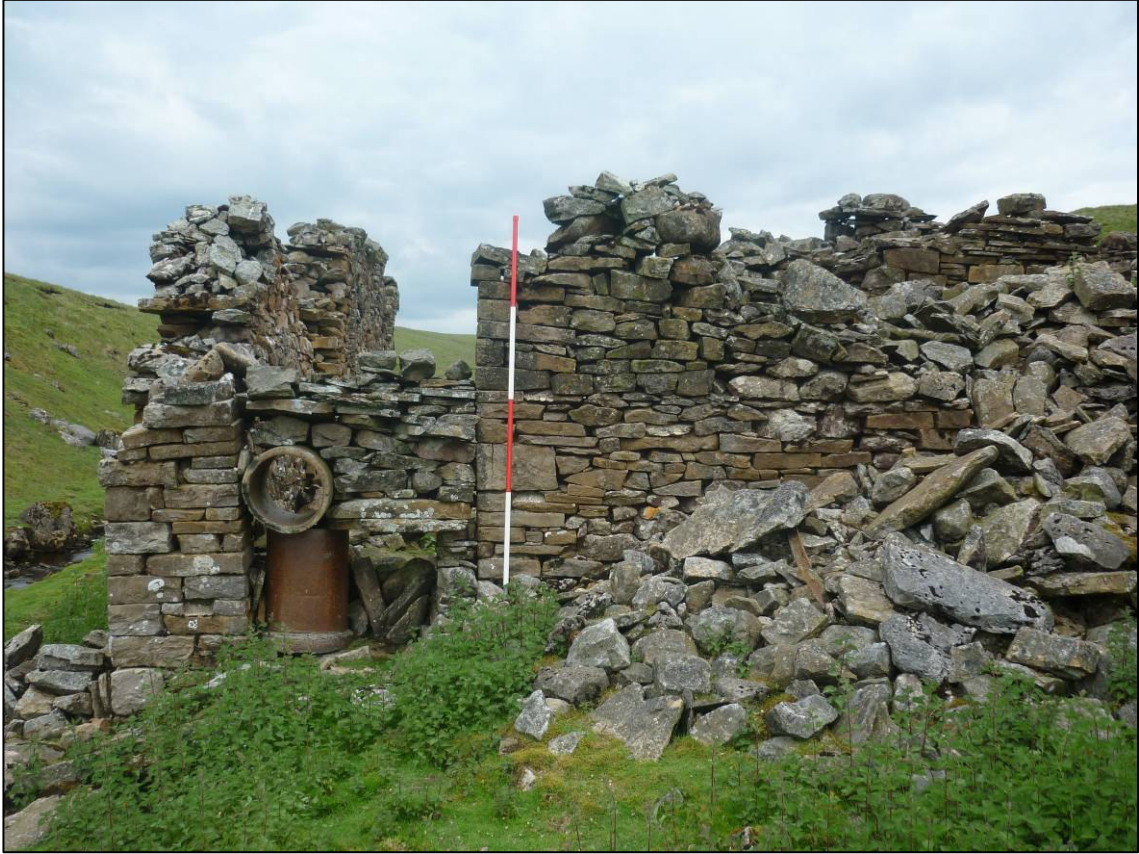
Plate 12: East external elevation of smelting mill (SAR 31.2, elevation 15), looking W (photo 1/430).
