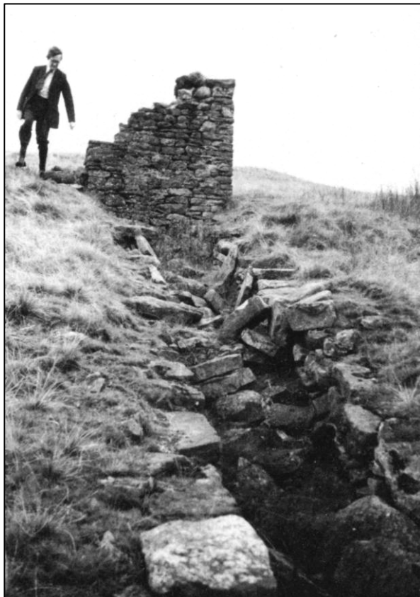
Top: View of smelt mill and chimney, looking NE, taken in 1905-06 by Backhouse (Raistrick 1975, 96).
