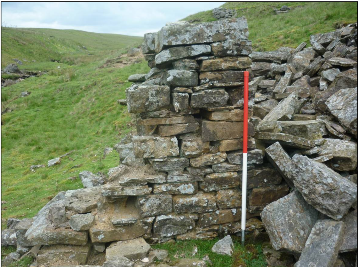
Plate 4: South end of west wall (internal face) of roasting house (SAR 43.2, elevation 8), looking W (photo 1/437).
