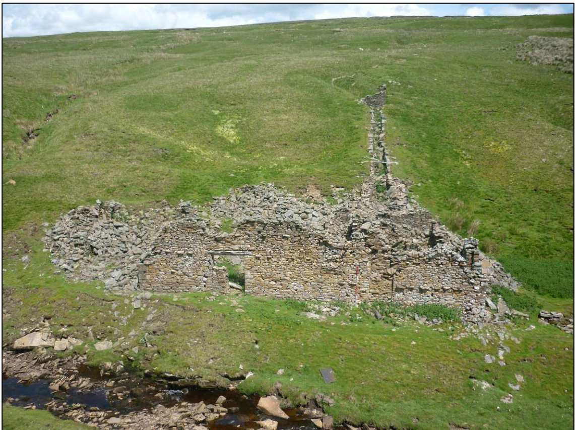
Plate 2: General view of Sargill smelt mill complex, looking N (photo 1/352).
