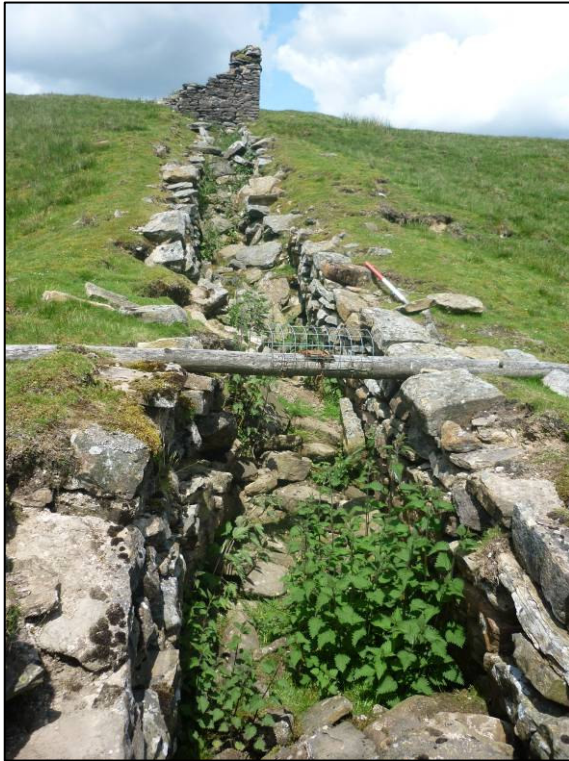
Plate 18: View up flue (SAR 9), looking N (photo 1/389).
