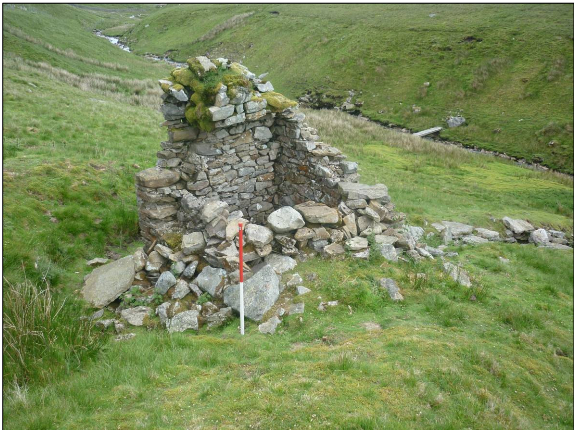
Plate 20: Chimney (SAR 04) at north end of flue (SAR 09), looking SE (photo 1/377).
