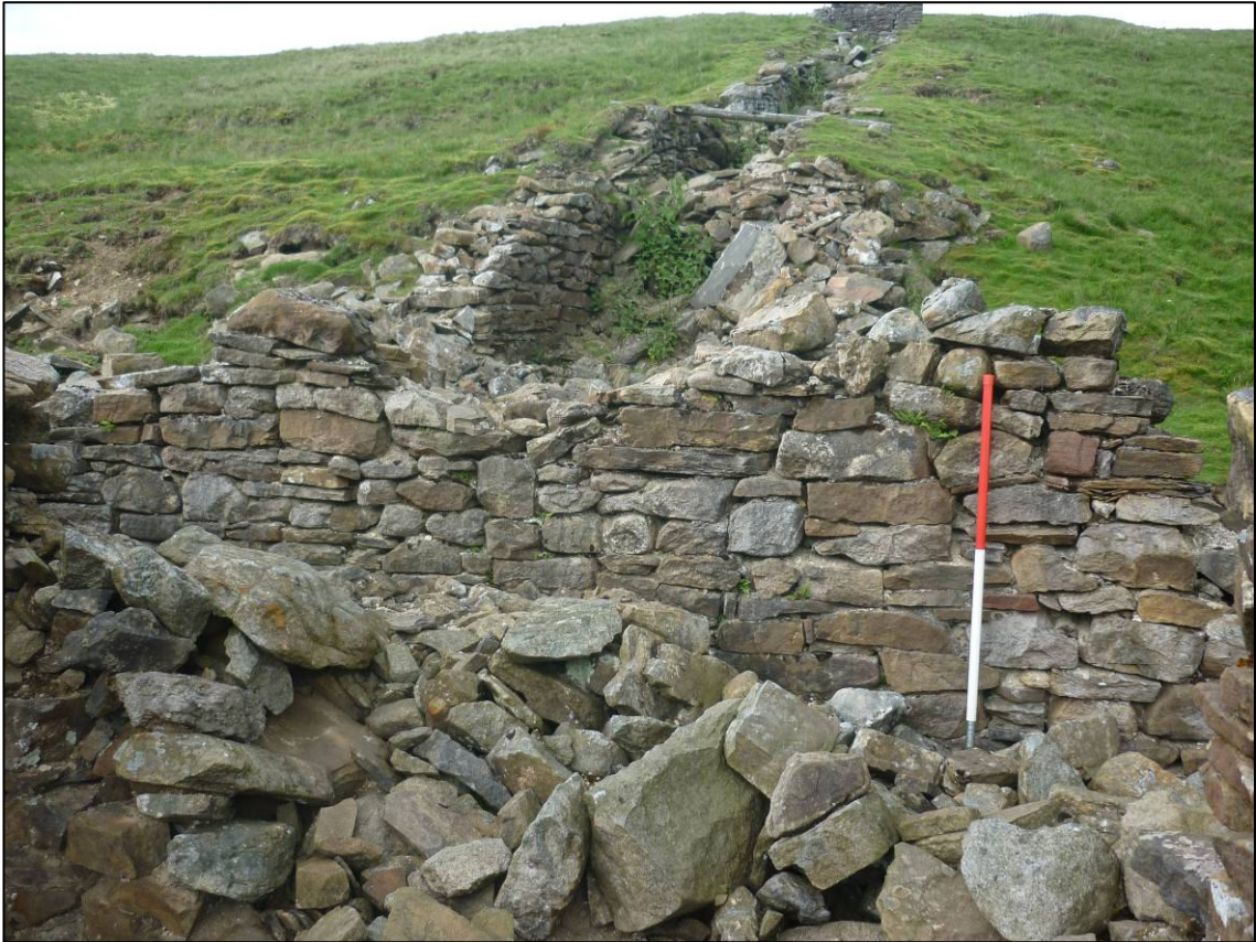
Plate 16: North wall of east-west passage (SAR 50.1, elevation 18), looking N (photo 1/465).
