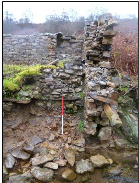
Plate 5: North end of Sir Francis mineshop, looking W (photo 1/205).
