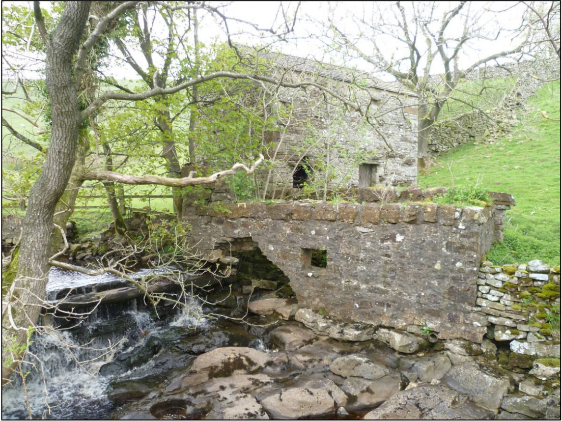
Plate 5: Leas House survey area, 1908-10 collecting chamber and weir (Sites 8a and 8c), looking N (photo 9/998).
