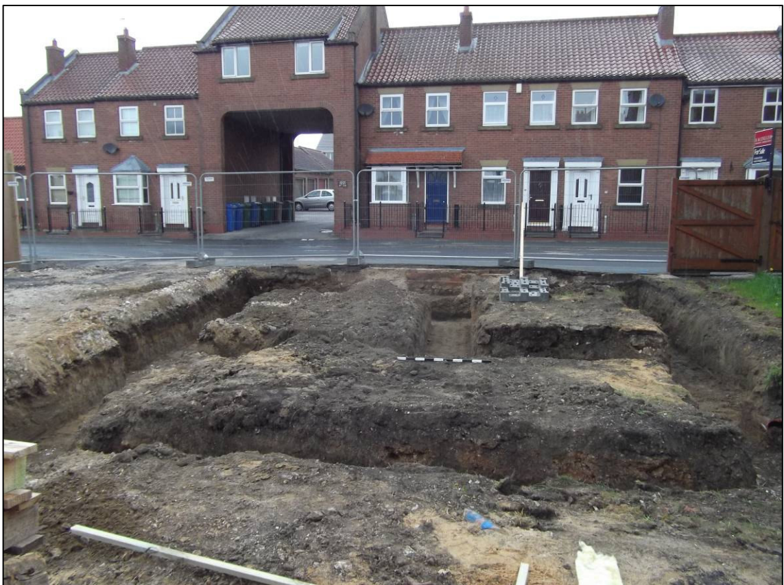
Plate 2: General view of excavated trenches, looking NW.
