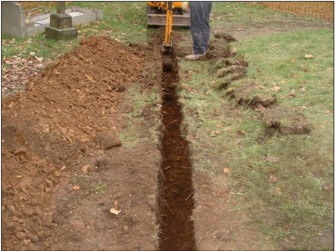
Plate 3: General view of east end of Trench 1, looking NE towards Trench 2.
