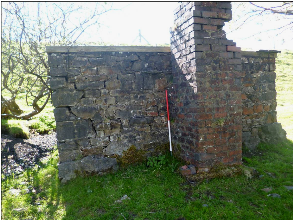
Plate 7: East elevation, looking W (photo 1/735).
