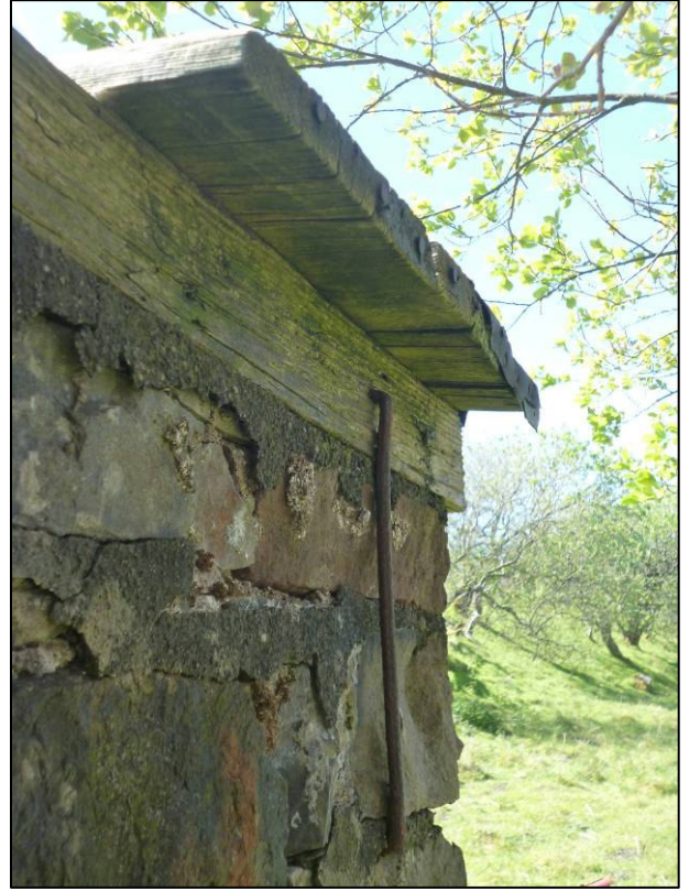
Plate 4: Roofing boards and clamp in north-east corner, looking NW (photo 1/746).
