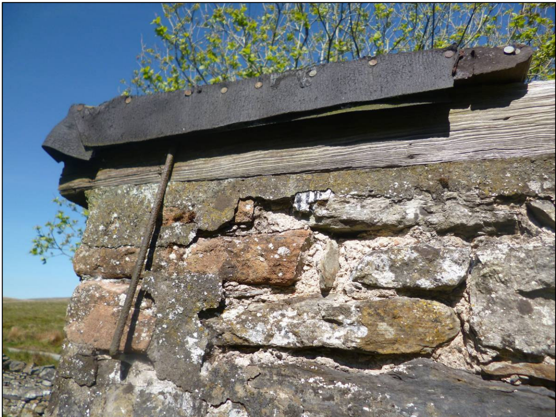
Plate 5: Roof structure in north-west corner, looking E (photo 1/743).
