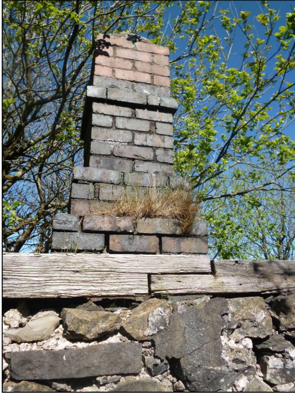
Plate 3: Scarf joint to east wall-plate, looking E (photo 1/750).
