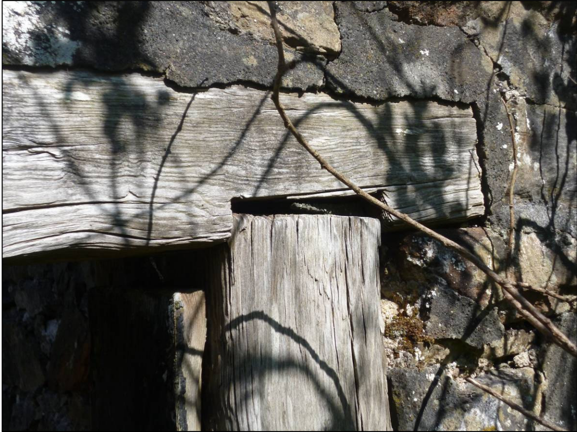
Plate 8: Detail to head of doorway in west elevation, looking E (photo 1/742).
