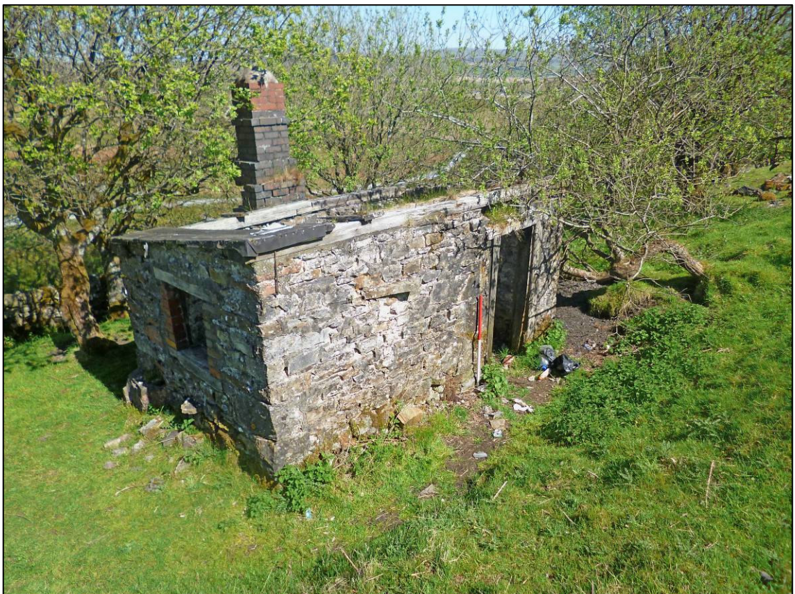
Plate 2: Platelayer's hut, looking SE (photo 1/738).
