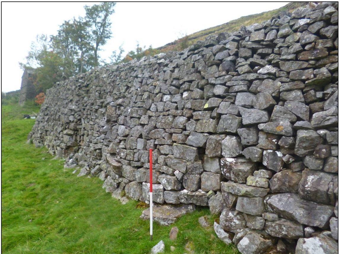
Plate 8: South face of east-west section of wall, looking W (photo 1/926).
