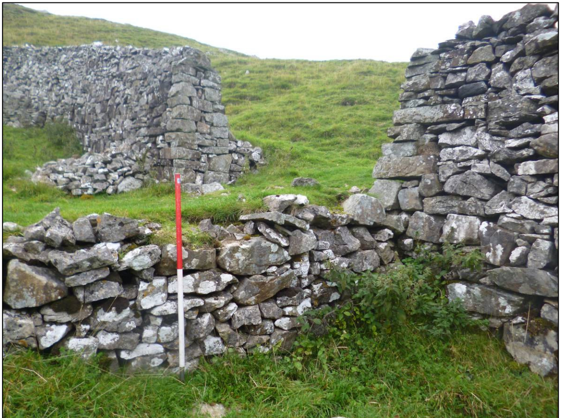
Plate 10: Revetted trackway through east gateway, looking N (photo 1/945).
