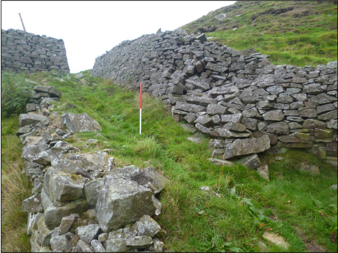
Plate 1: Revetted track at west end of wall, looking NW (photo 1/900).
