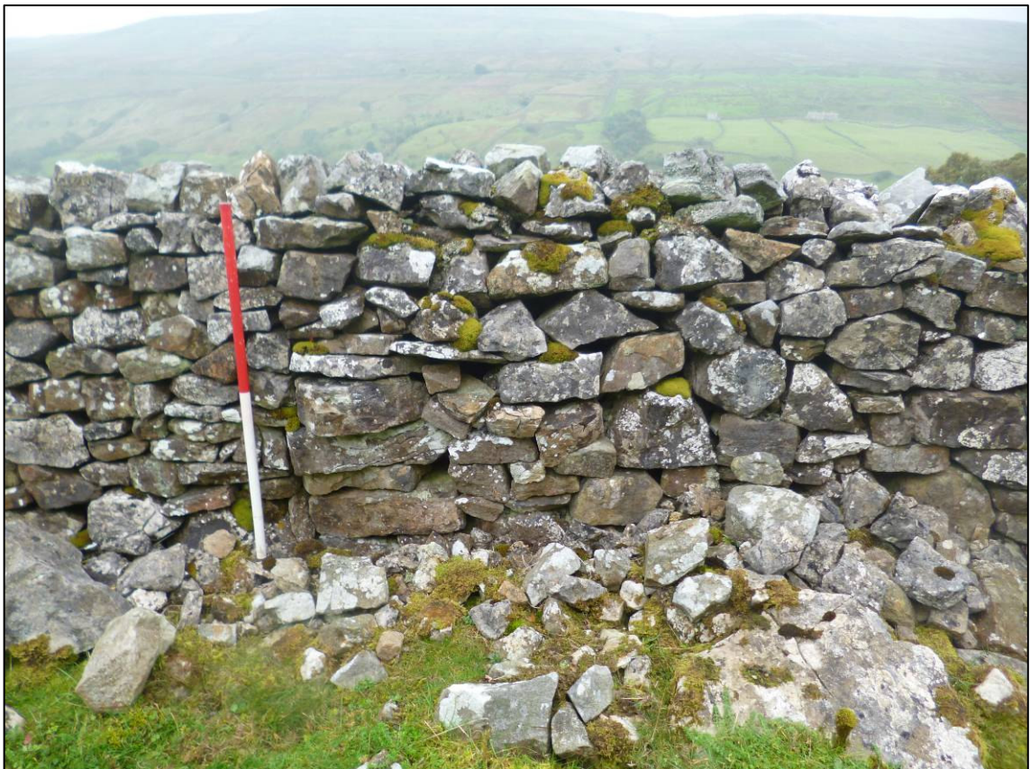
Plate 12: Blocked opening in north face of wall at change of angle, looking S (photo 1/964).
