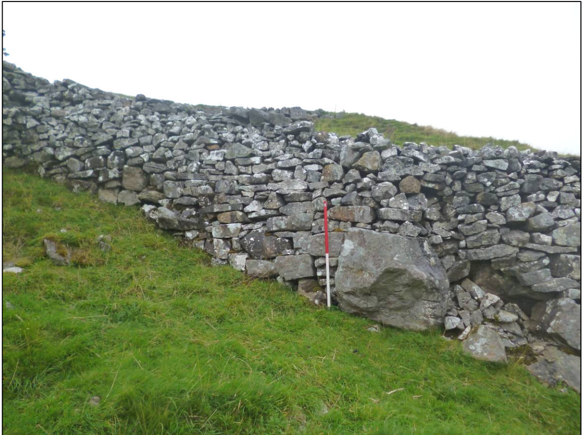
Plate 11: Orthostat in west face of wall, south of east gateway, looking E (photo 1/947).
