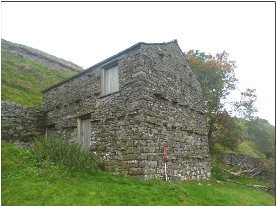
Plate 2: Field barn, looking NE (photo 1/906).
