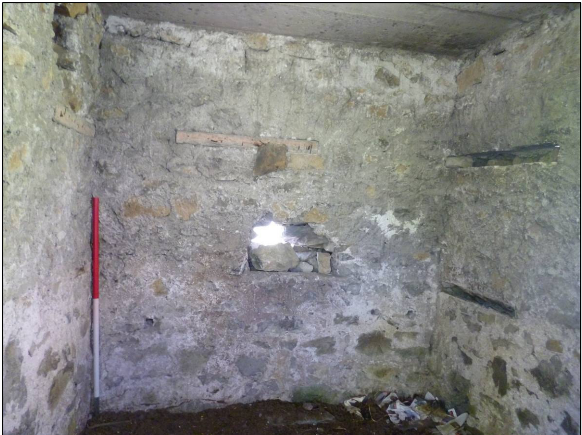
Plate 7: Internal west wall of west cell, showing battens, looking W (photo 1/707).
