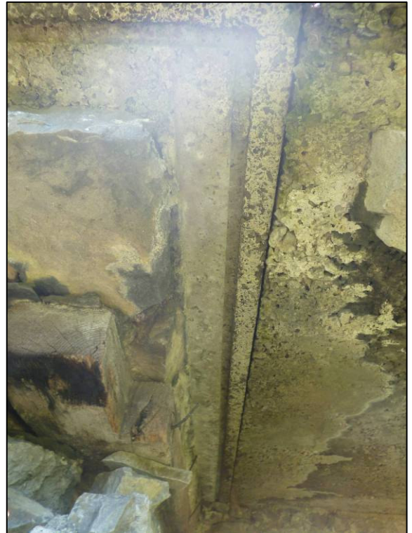
Plate 6: Roof drip line, east cell roof, looking N (photo 1/704).
