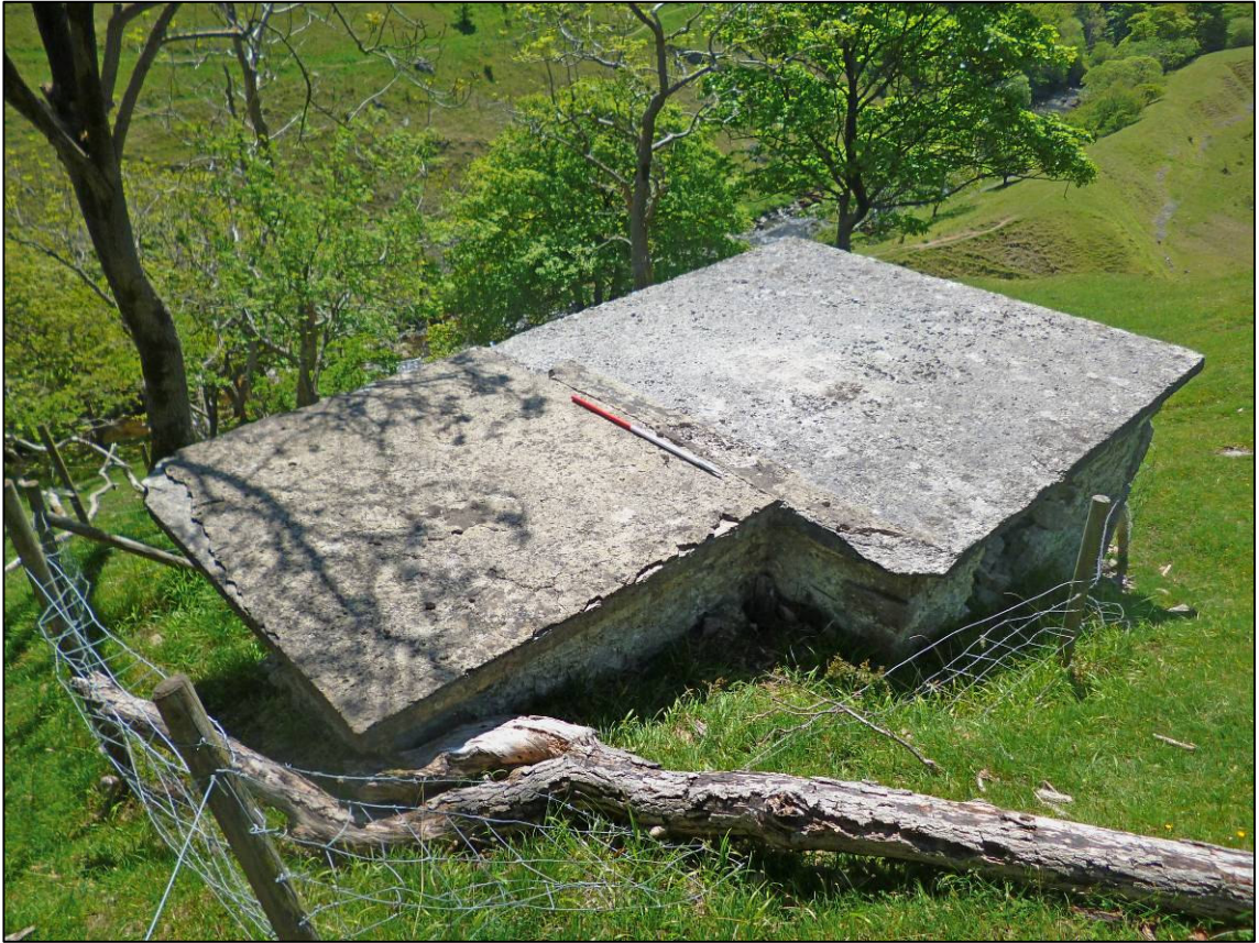
Plate 3: View of roof structure, looking SW (photo 1/691).
