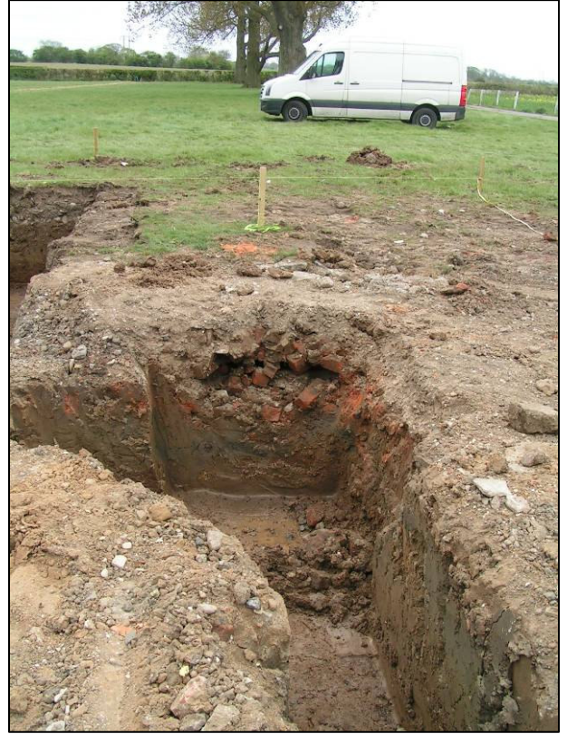
Plate 2: South central side of house foundation (Trench 1), looking E
