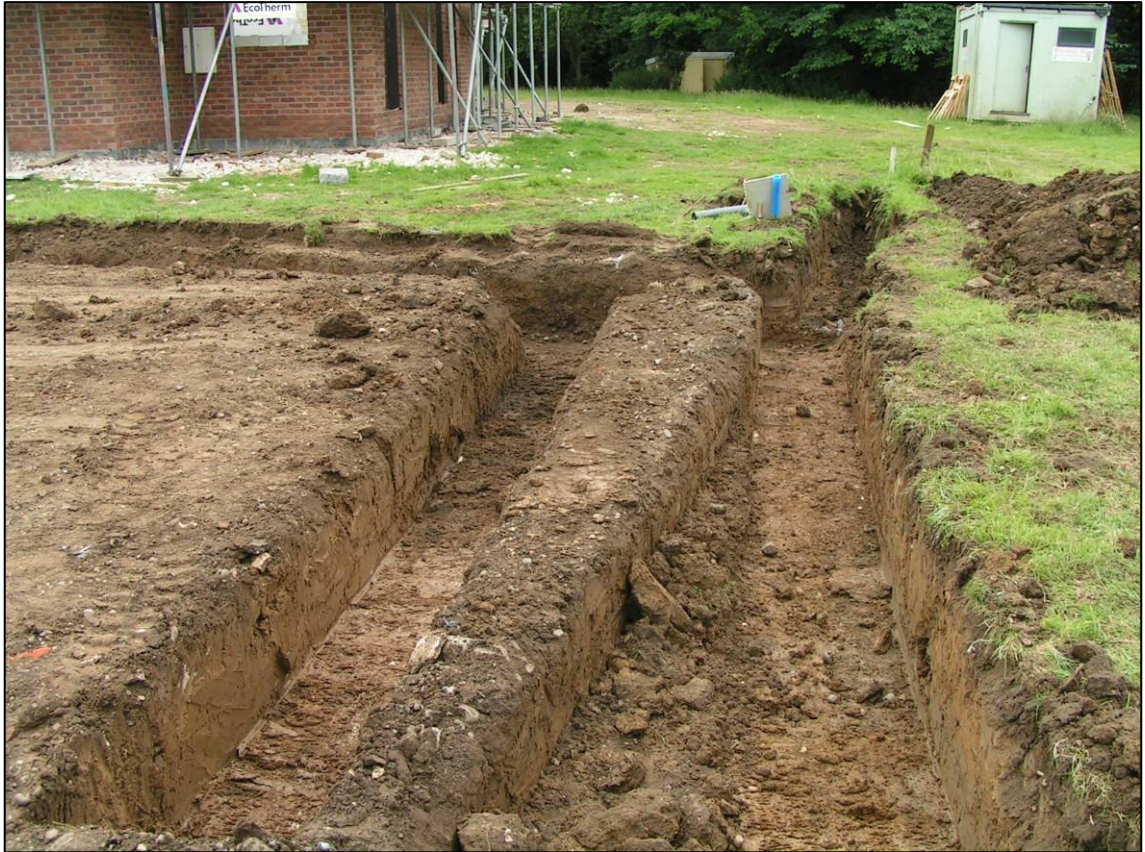
Plate 7: General view of north end of garage foundations (Trench 2), looking W.
