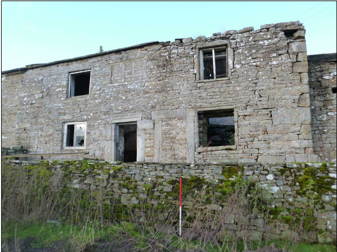
Plate 3: South elevation of house, looking NW (photo 3/281).
