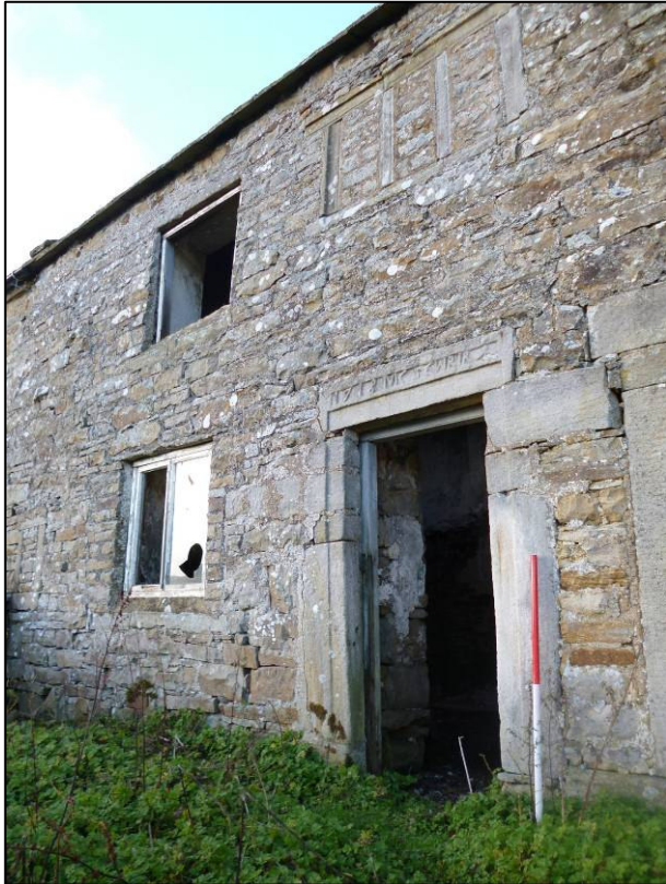
Plate 5: South elevation of west cell of house, looking W (photo 3/289).
