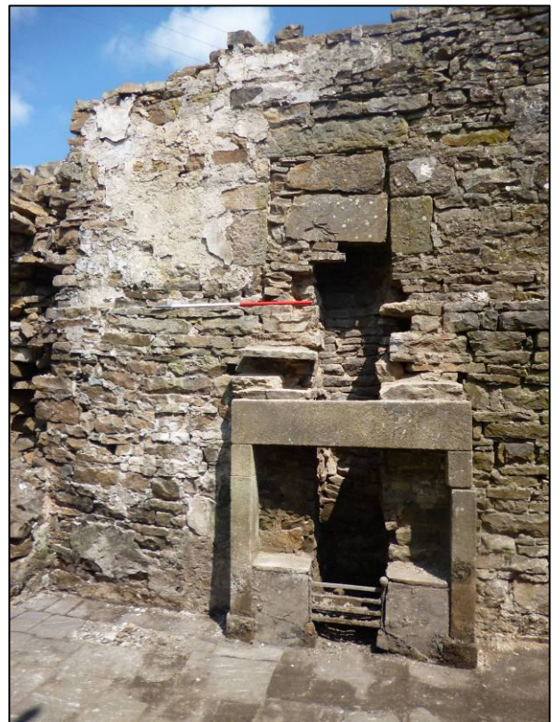
Plate 11: Fireplaces in east cell after clearance, looking NE (photo 4/066).
