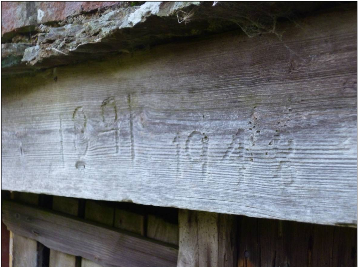
Plate 19: Dates in doorway in east gable of shed, looking S (photo 3/276).
