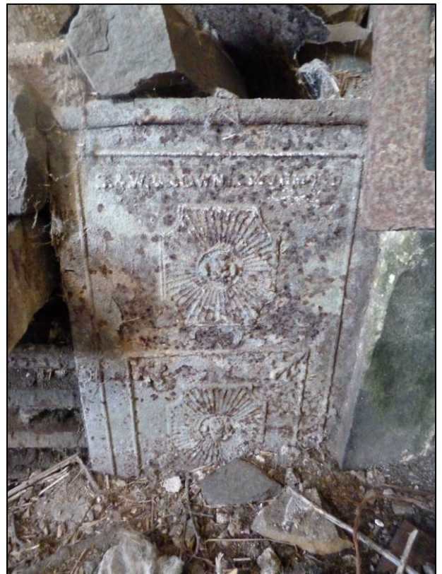
Plate 8: Boiler plate to fireplace in west cell of house, looking SW (photo 3/307).
