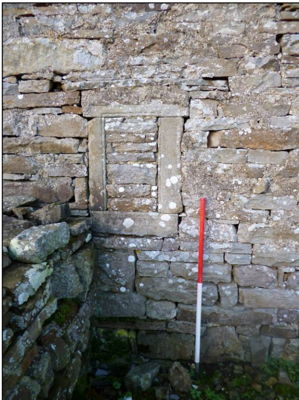
Plate 7: Fire window in south elevation of house, looking NW (photo 3/292).
