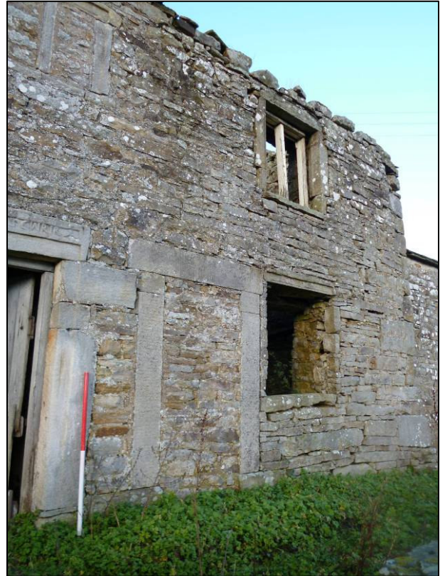
Plate 6: South elevation of east cell of house, looking N (photo 3/290).
