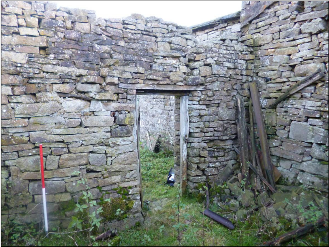
Plate 16: East internal wall of North Structure, looking E (photo 3/259).
