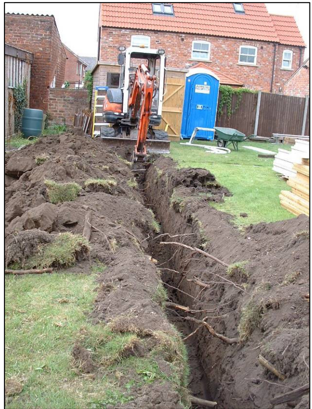
Plate 3: Excavation of west end of Trench 1, looking W.
