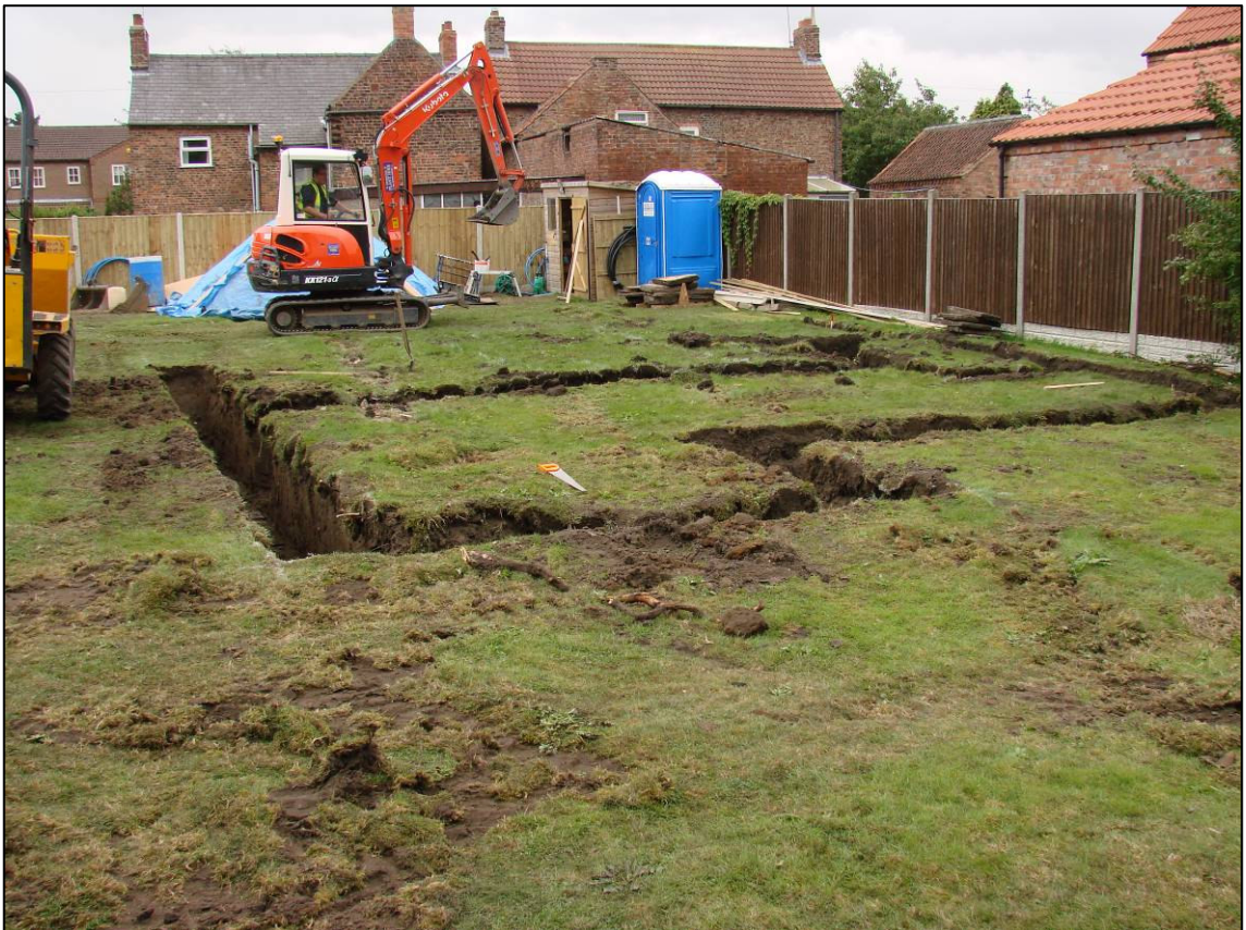
Plate 5: Foundations for Plot 2 (Trench 3) under excavation, looking SW.
