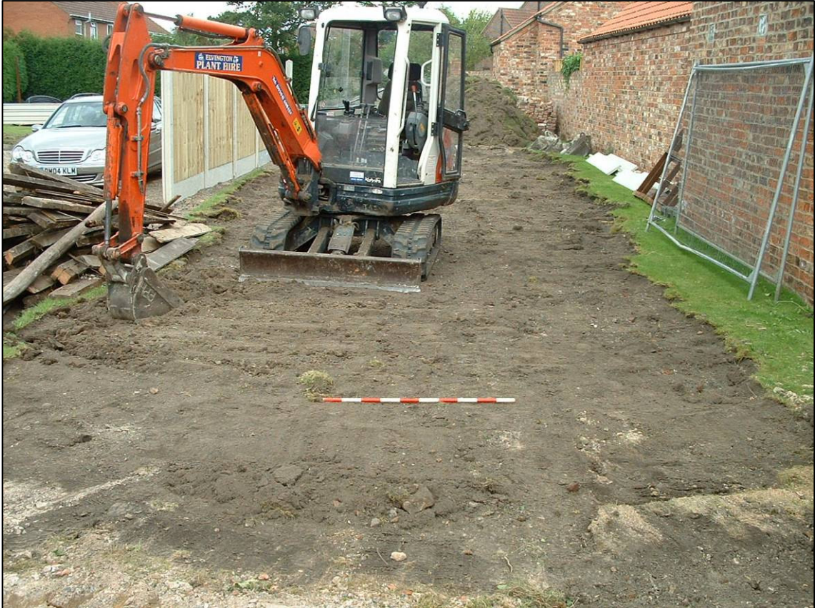
Plate 1: Topsoil strip for access road and drainage trench (Trench 1), looking N.
