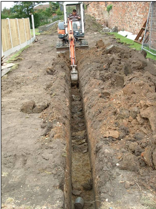
Plate 2: Excavation of south end of Trench 1, looking N.
