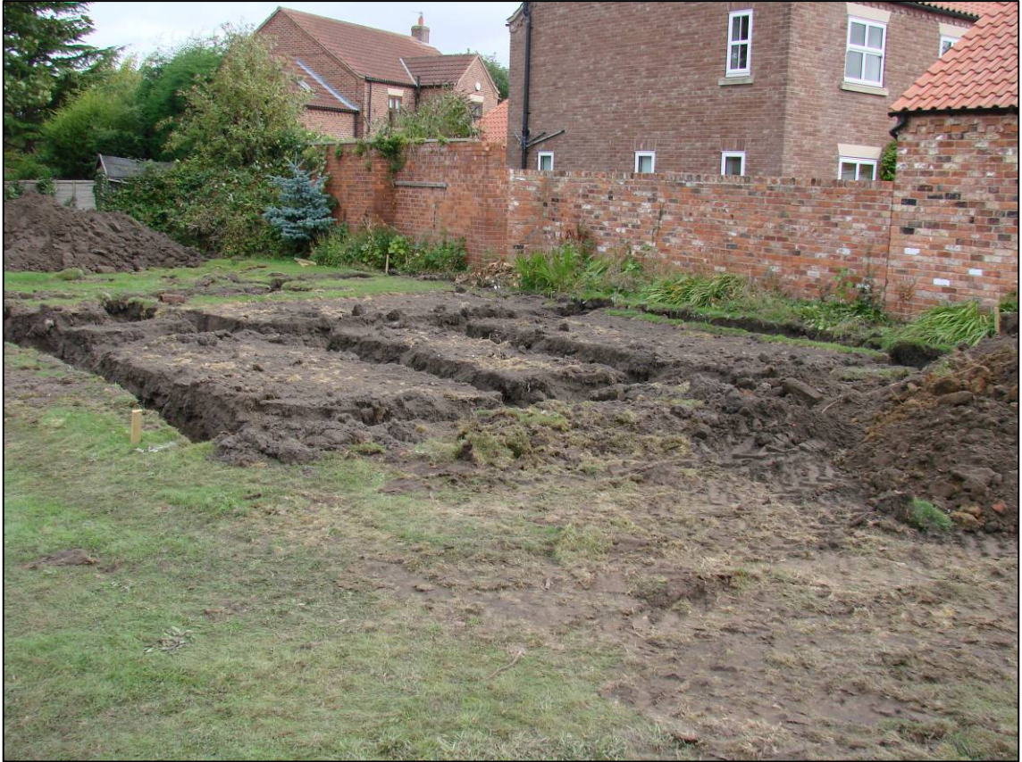
Plate 4: Foundation trenches for Plot 1 (Trench 2) completed, looking NE.
