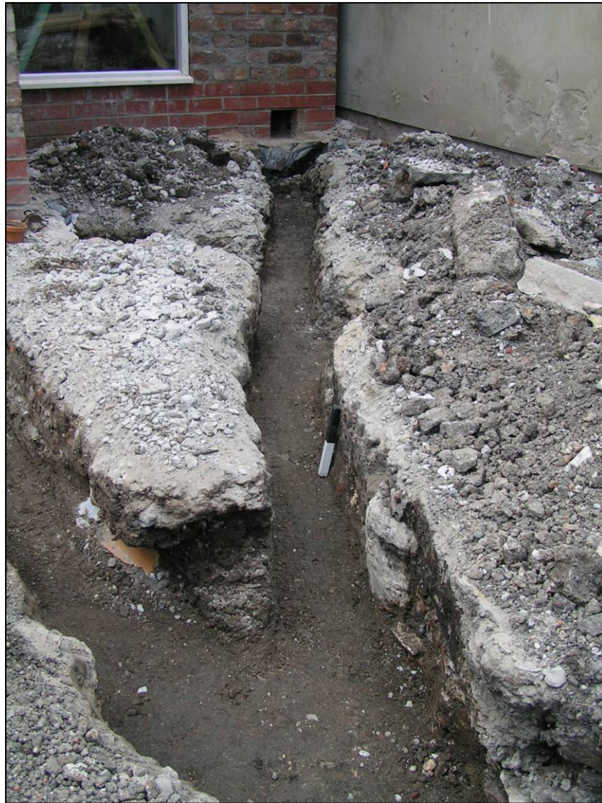
Plate 1: Excavated north trench, looking W.
