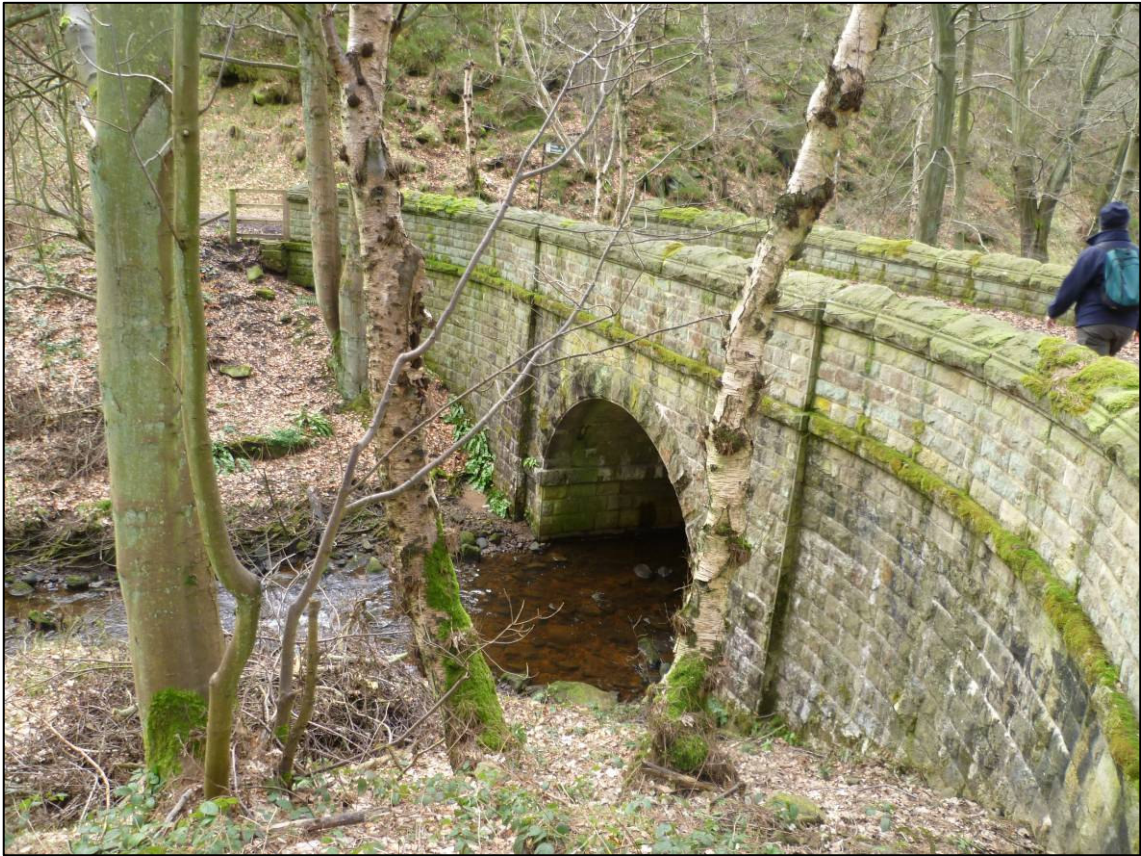
Plate 7: Rivelin Bridge (Site 5), looking SW (photo 3/889).
