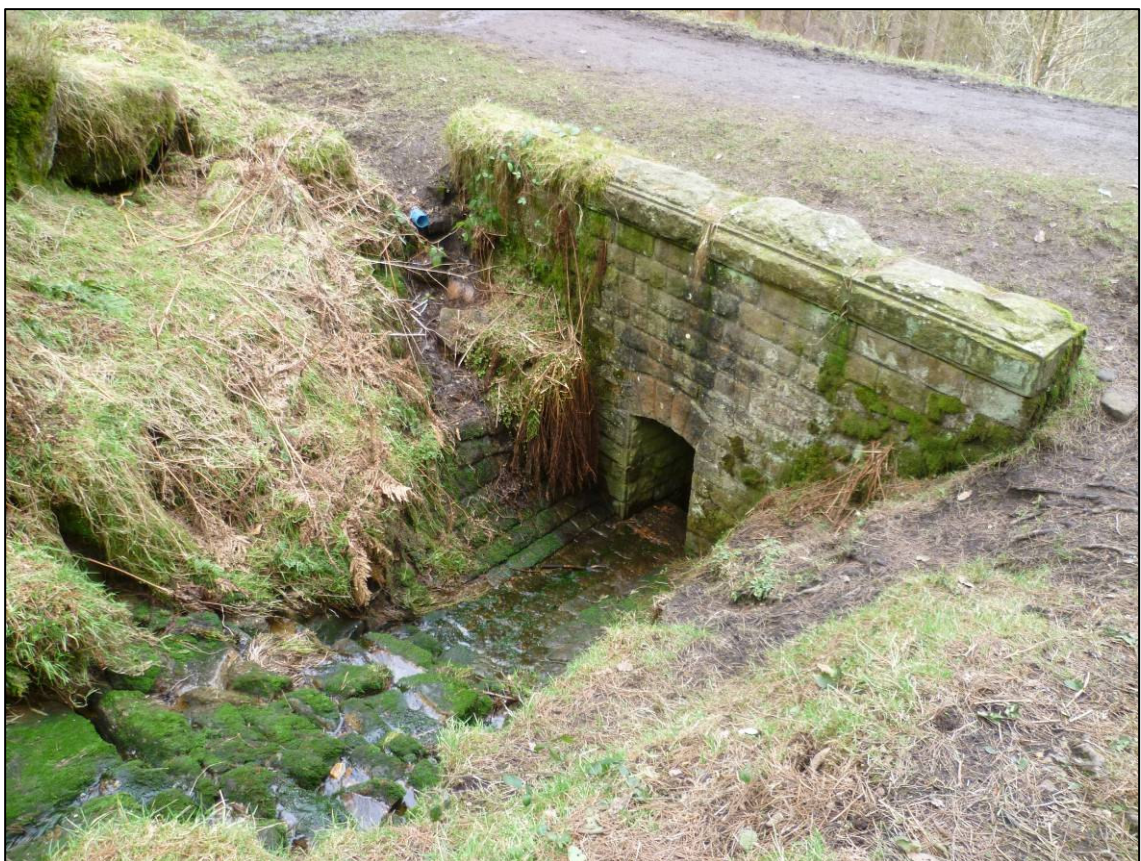
Plate 11: South side of Wyming Brook Drive culvert (Site 20), looking NW (photo 3/895).
