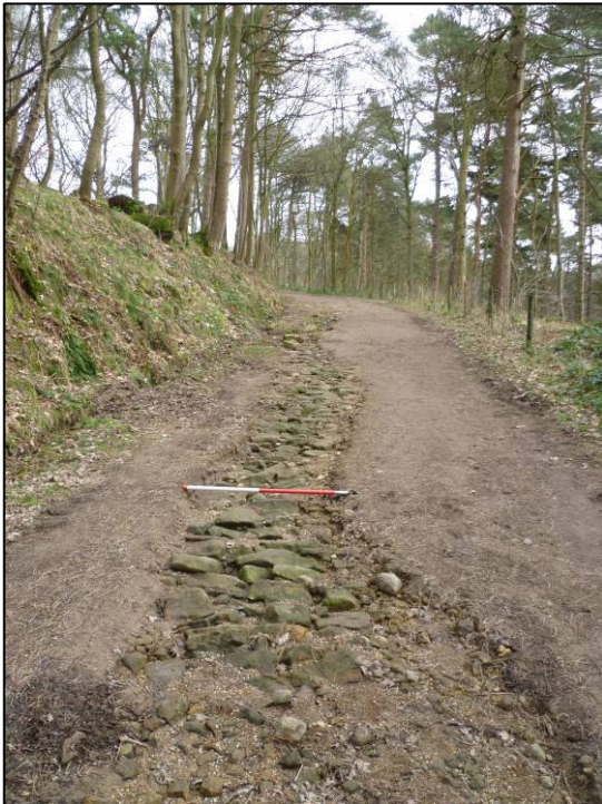
Plate 8: Water erosion on Wyming Brook Drive, on approach to A57, looking NE (photo 3/890).
