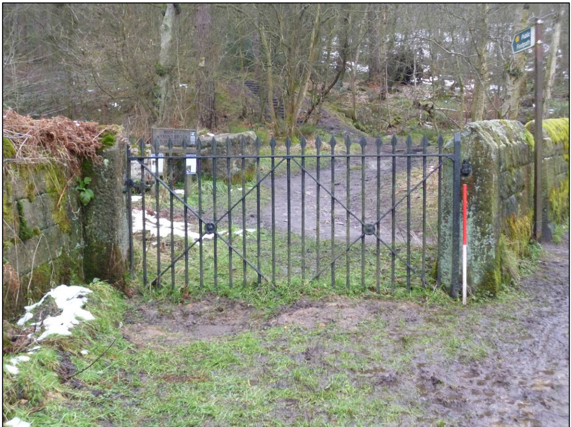
Plate 12: Gates in south side of Wyming Brook Drive (Site 17/8), looking W (photo 1/026).
