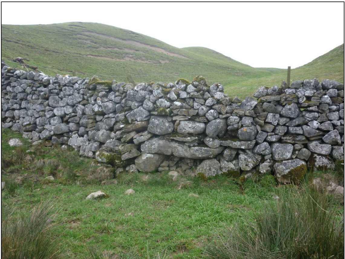
Plate 24: Blocked opening in field wall near Millstone Gill, looking N (photo 1/005).
