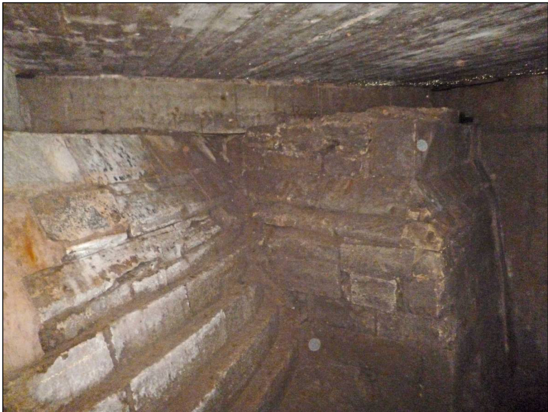
Plate 48: Remains of gate structures in underground chamber, November 2013 (photo 5/645).
