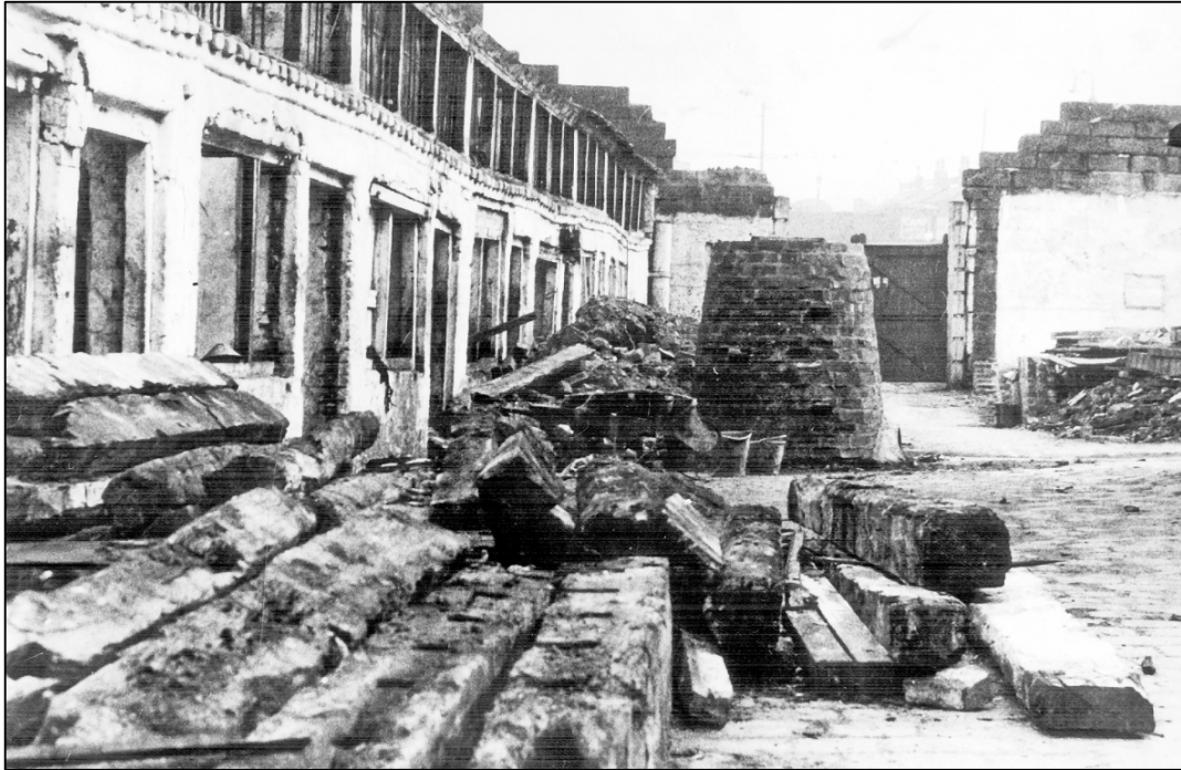
Plate 10: Remains of Shambles Slaughter House, showing ancient beams discovered in a horizontal position and newly built sewer manhole (for a new road for the continuation of Bridge Street) in background, taken by J B Himsworth, September 1929 ( www.picturesheffield.com , y00892).
