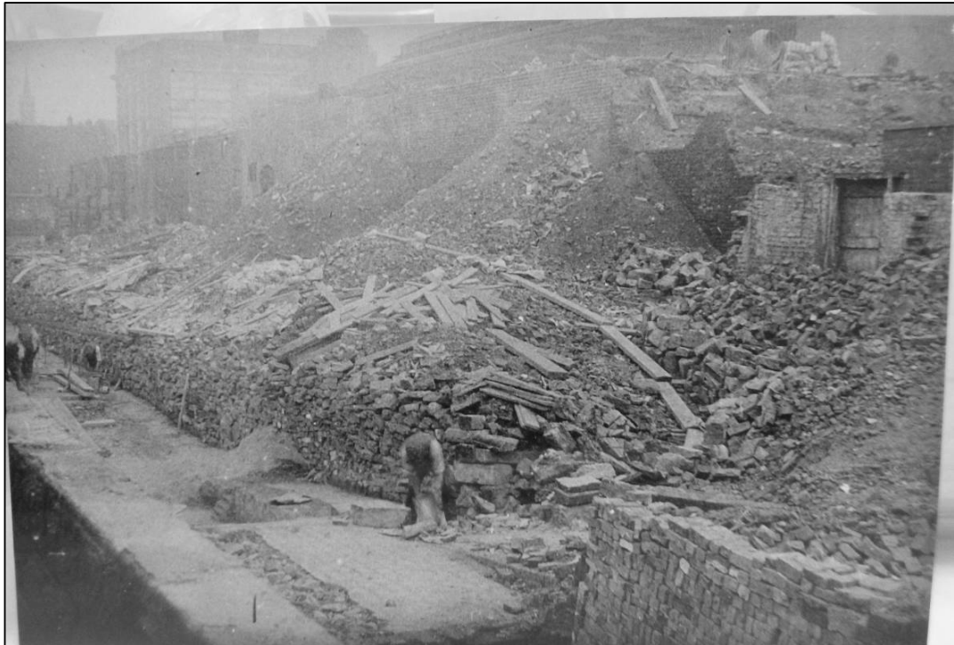
Plate 40: View taken after both Chandlers Row and Shambles Lane buildings had been demolished, leaving only the high south retaining wall to Chandlers Row still standing, looking W (photo 2/673).
