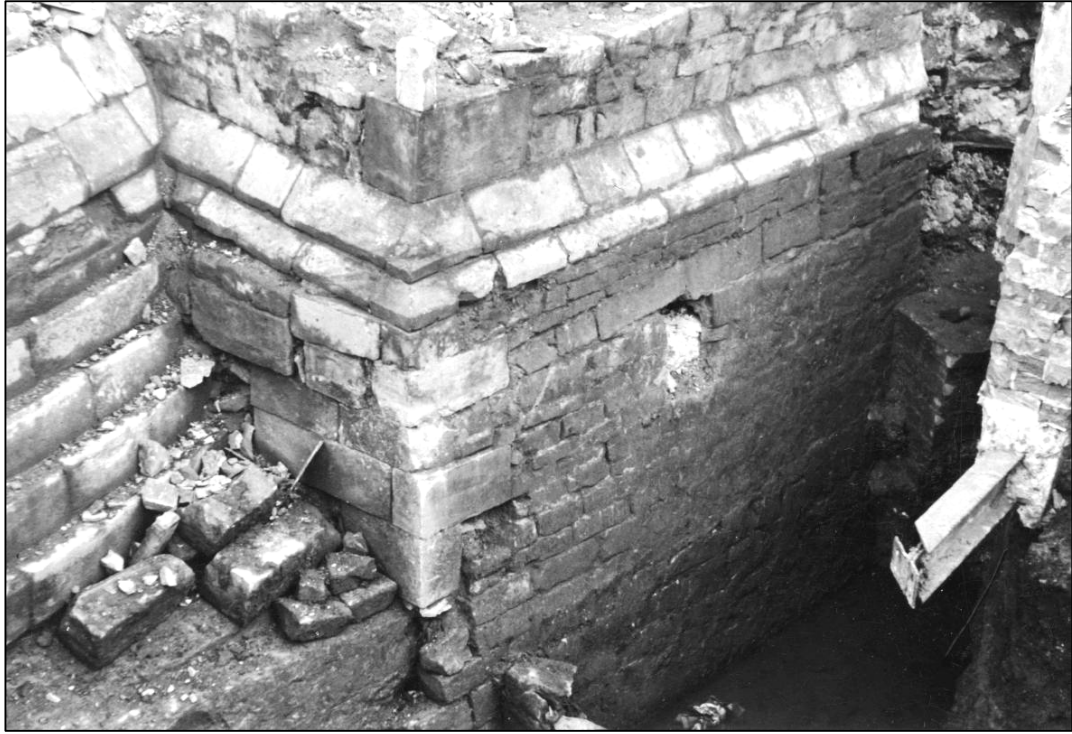
Plate 35: Detail of gatehouse structure (MSA Box file - Butcher 1976.1064 Sheffield Castle Notes/Photographs folder SC2/3).
