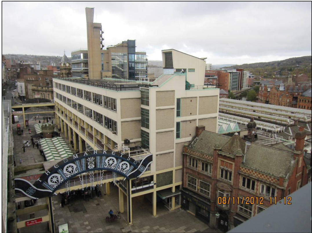
Plate 27: Low Block, part of the 1958-61 redevelopment works (photo IMG 5532 supplied by SCC).
