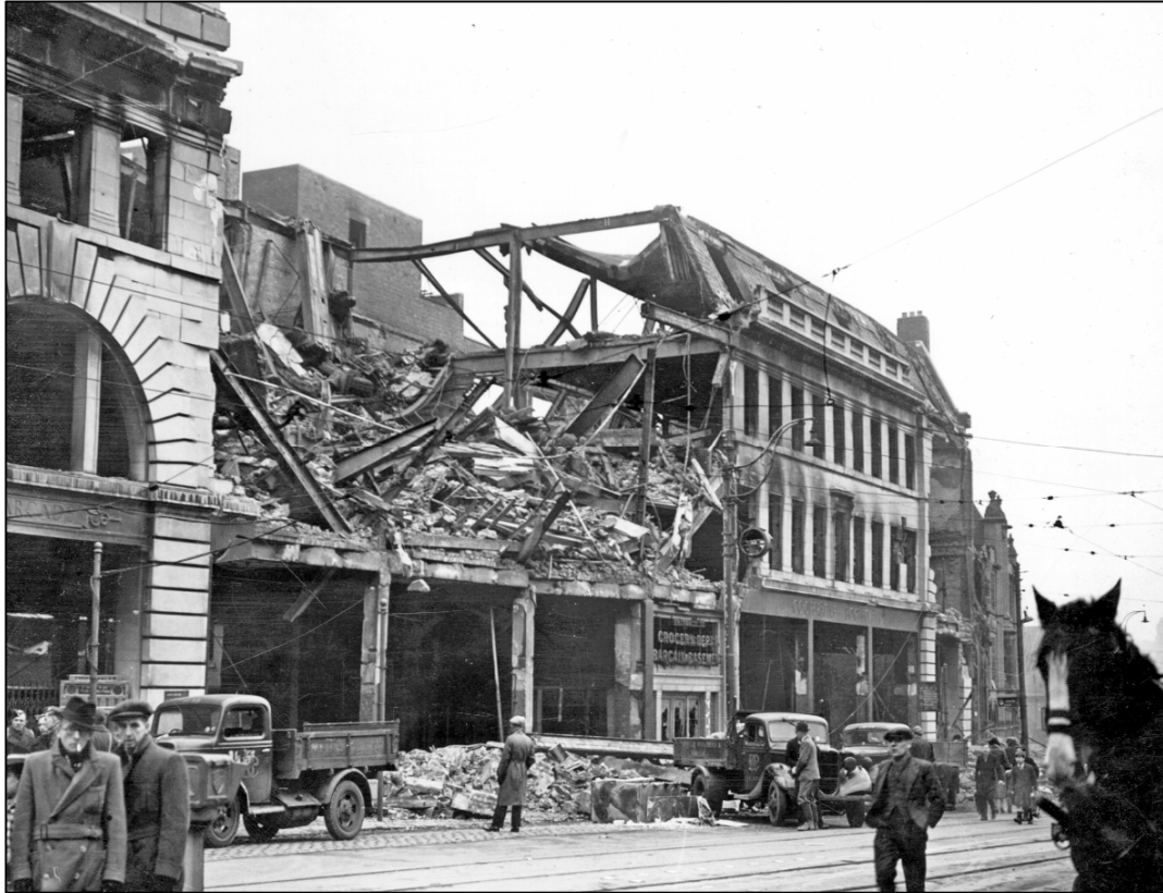
Plate 19: Brightside and Carbrook Co-operative Society building, Exchange Street frontage, after air raid on 12th/13th December 1940 ( www.picturesheffield.com , s01212 - © Sheffield Newspapers).
