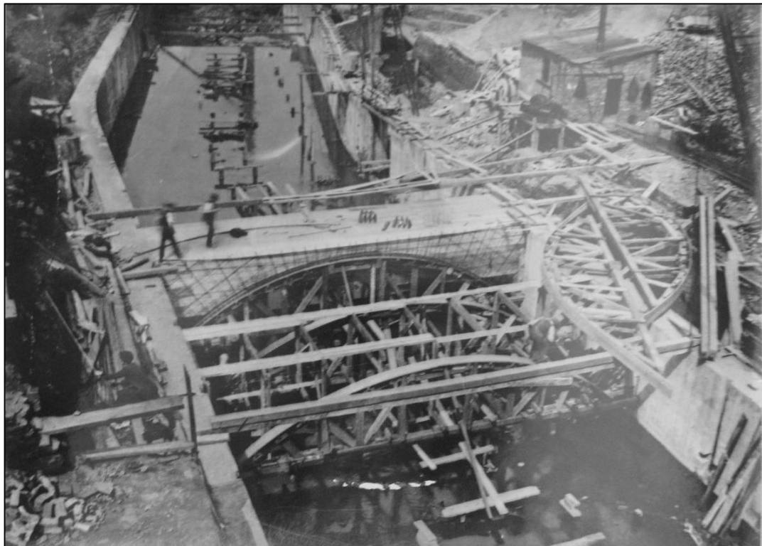
Plate 16: Construction of Sheaf culvert, 1915-16 (photo IMG 6025 supplied by SCC).
