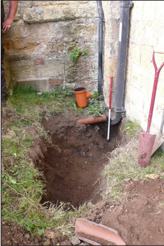
Plate 4: Excavation of Trench 3, looking W.
