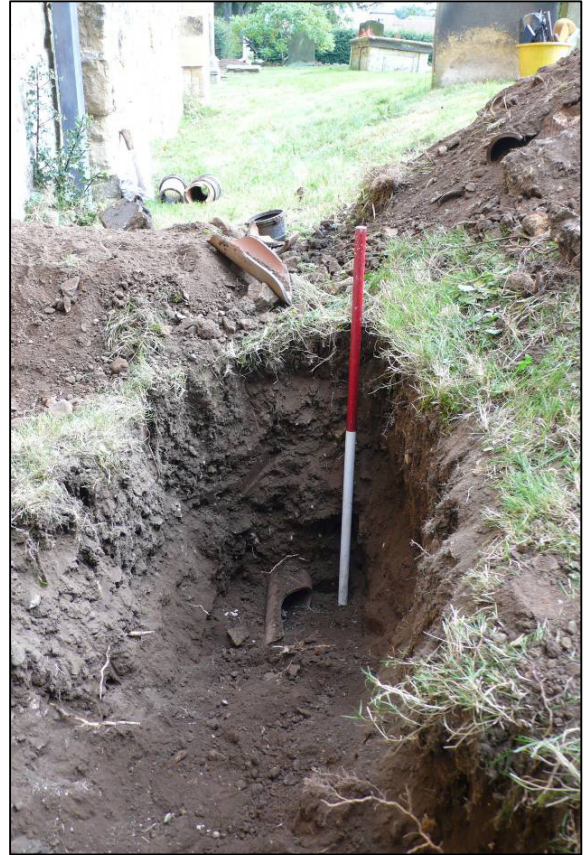
Plate 5: Excavation of Trench 3, showing drain pipe (021), looking E.
