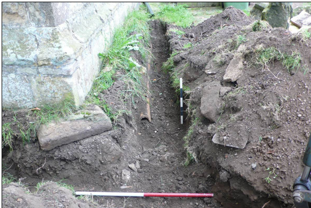
Plate 6: Old drain pipe (018) exposed in trench 5, looking W.
