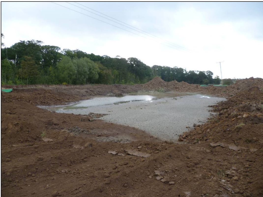
Plate 6: Infilling of northern pond, looking SE.
