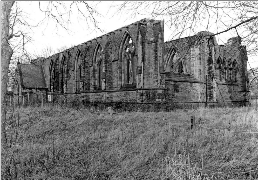
Plate 2: South and east elevations, looking NW (photo 2/13).
