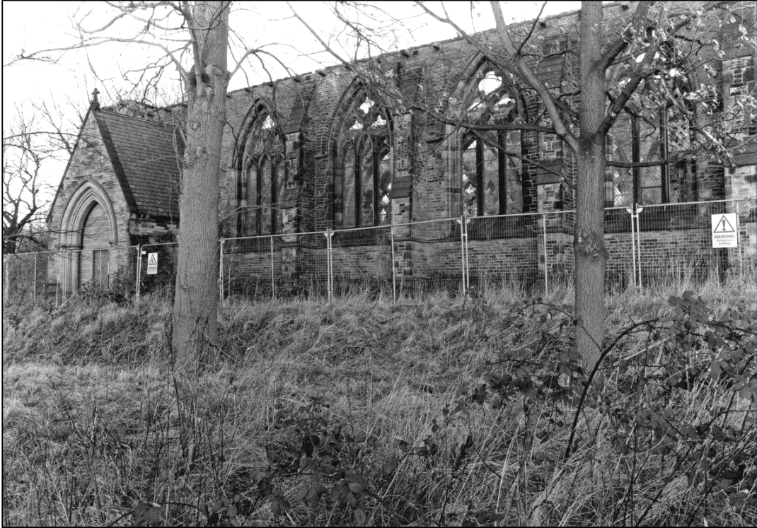
Plate 1: South porch and south elevation with platform scarp to foreground, looking NW (photo 1/4).
