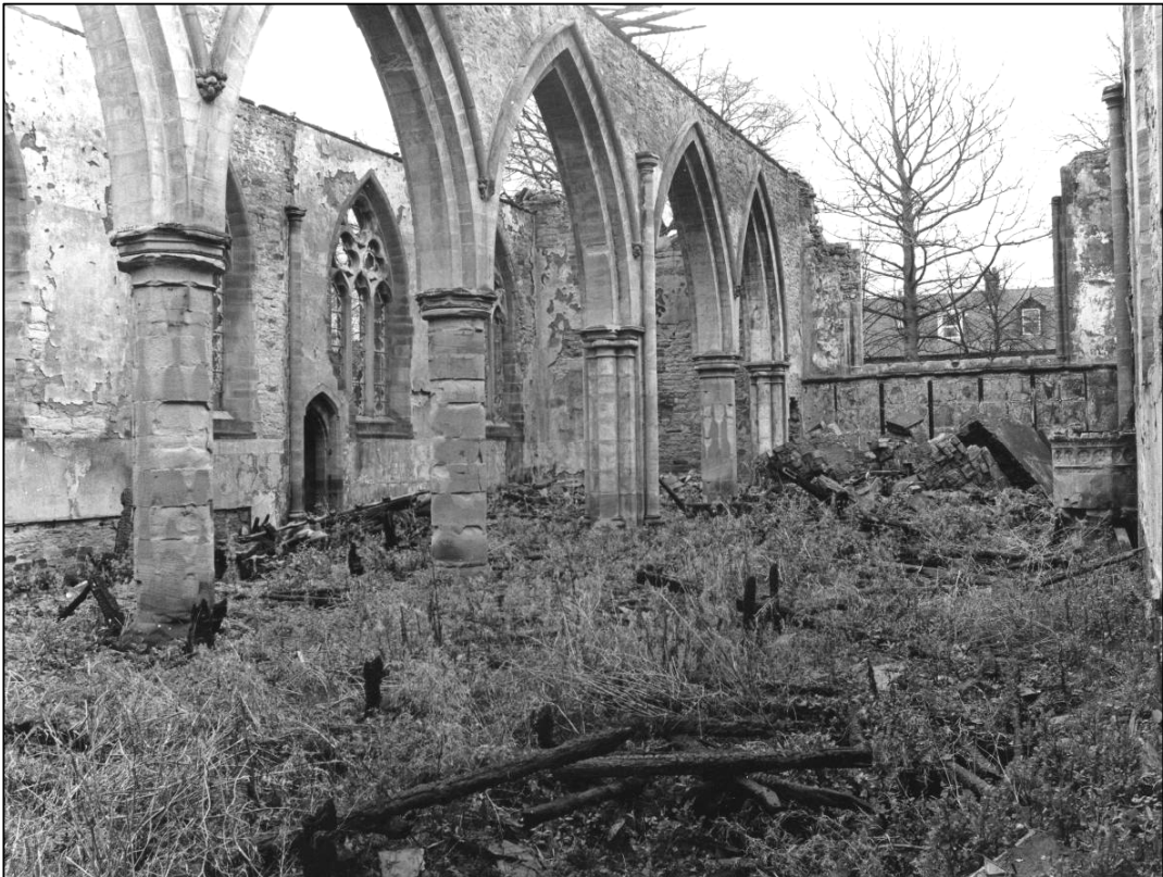
Plate 20: Interior from west end of nave, looking NE (photo 2/1).
