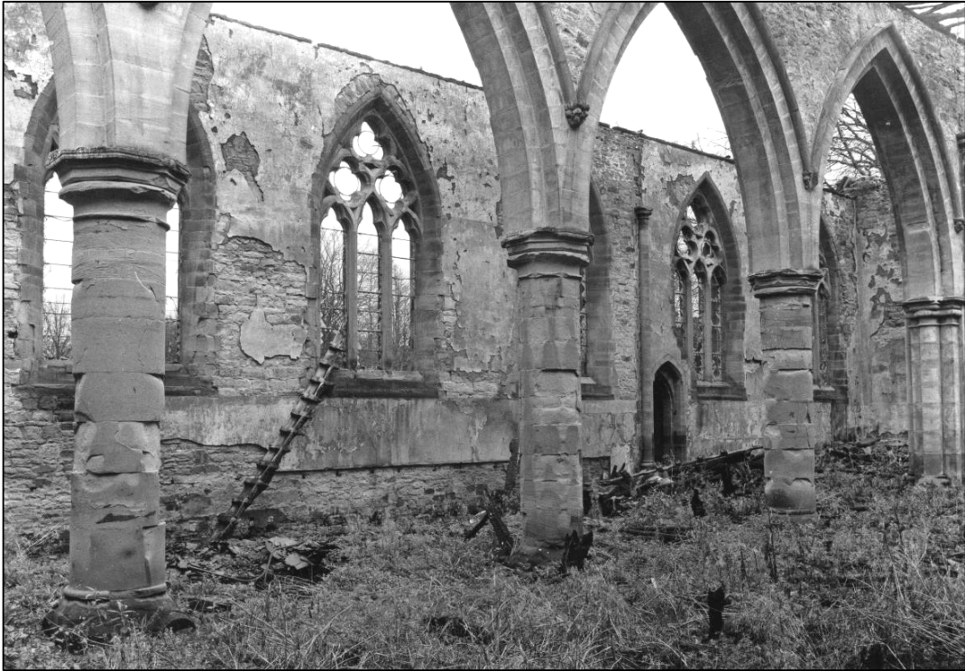
Plate 21: Interior from west end of nave, looking NE (photo 2/2).
