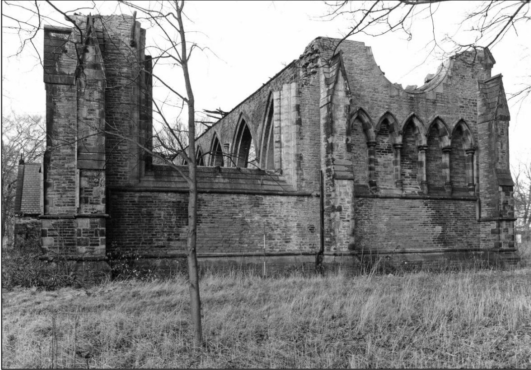
Plate 17: East elevation, looking NW (photo 2/15).
