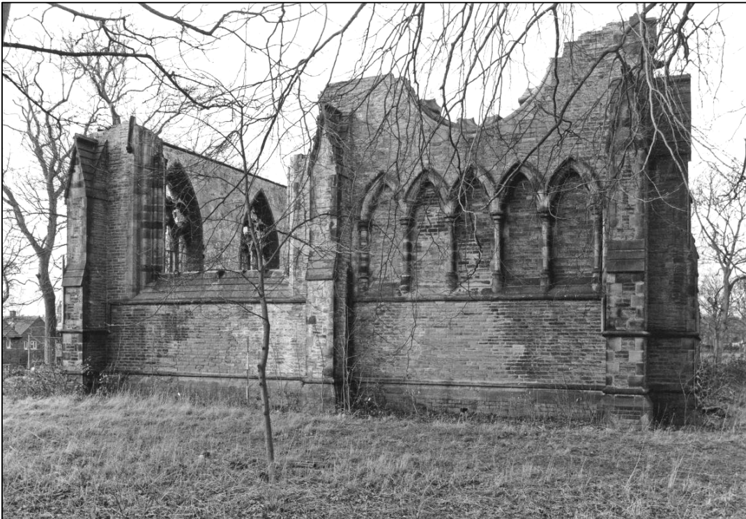
Plate 18: East elevation, looking SW (photo 2/16).
