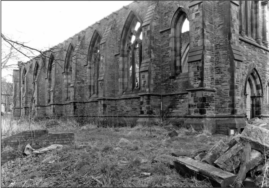
Plate 13: North elevation, looking SE (photo 1/15).
