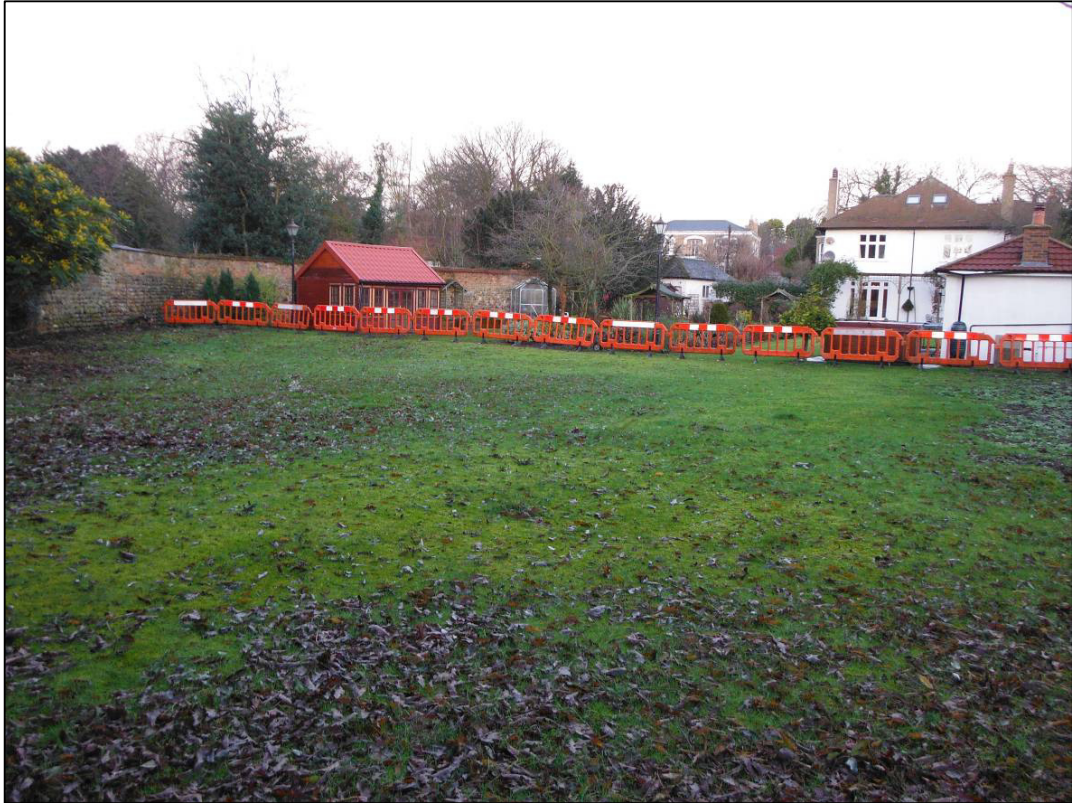
Plate 1: General view of development site prior to excavations, looking N.
