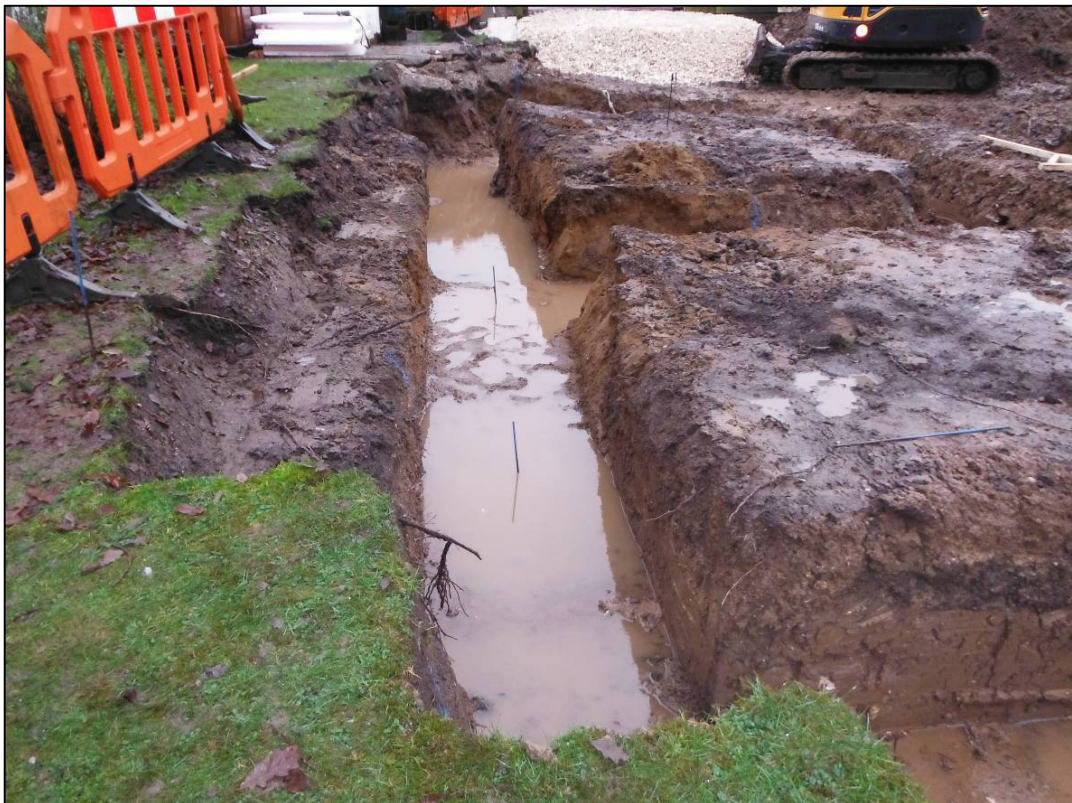
Plate 4: General view of north side of house foundations, looking E.
