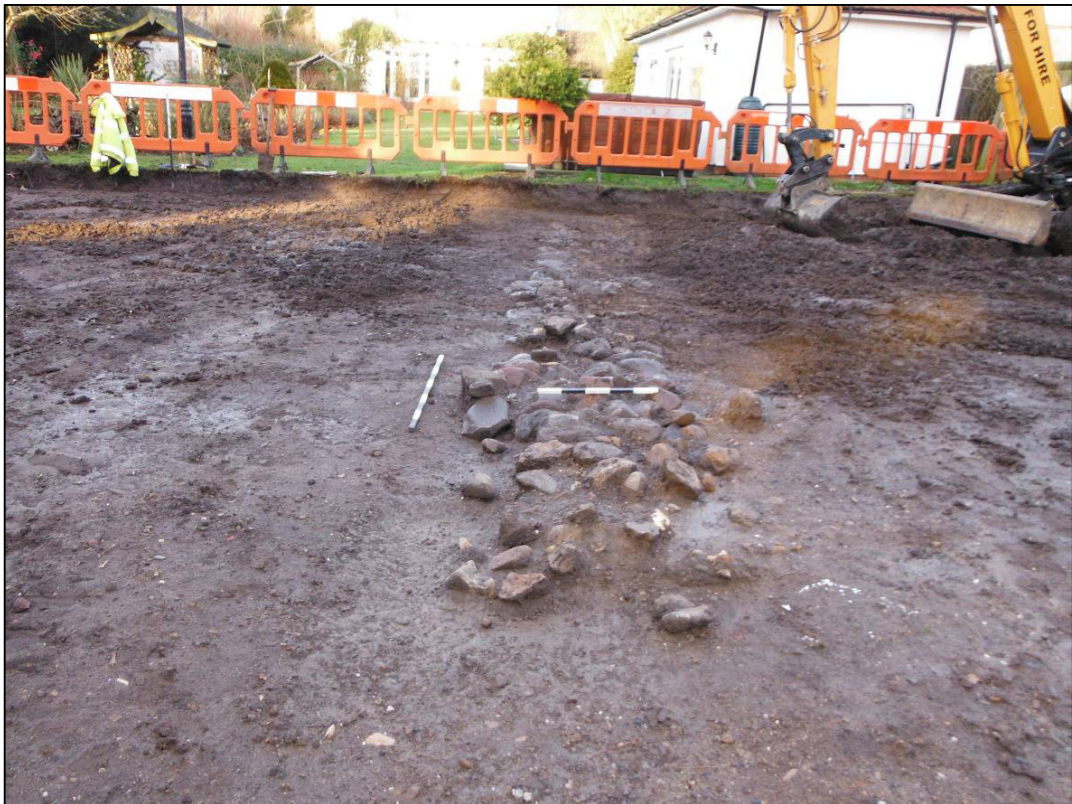
Plate 2: General view of cobble wall foundation (109), looking N.
