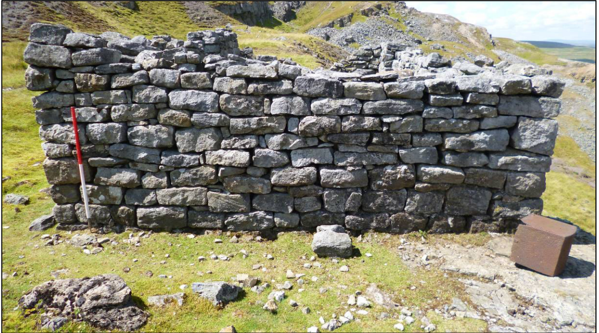
Plate 3: East elevation, looking W (photo 1/001).
