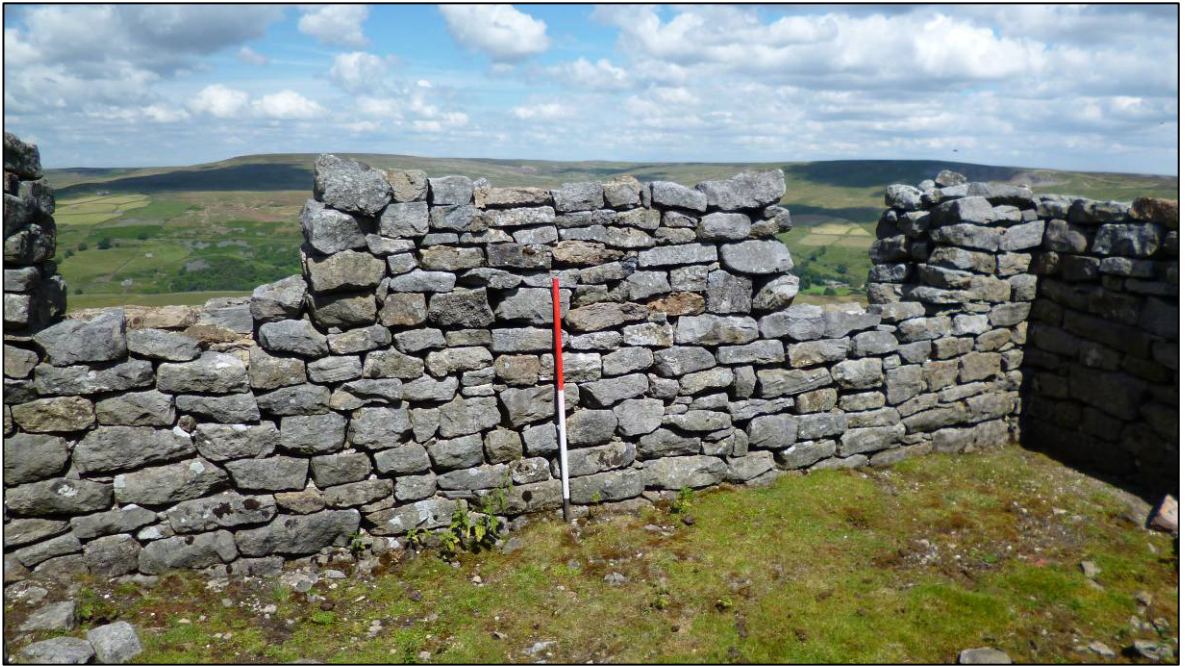
Plate 8: North internal wall, looking NE (photo 1/026).
