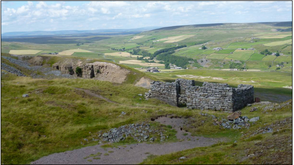
Plate 1: General view of smithy building within landscape context, looking NW (photo 1/033).
