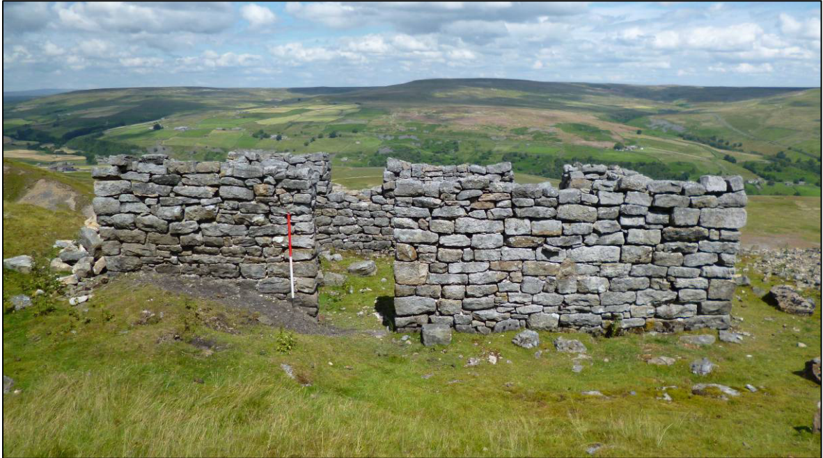
Plate 5: South elevation, looking N (photo 1/998).
