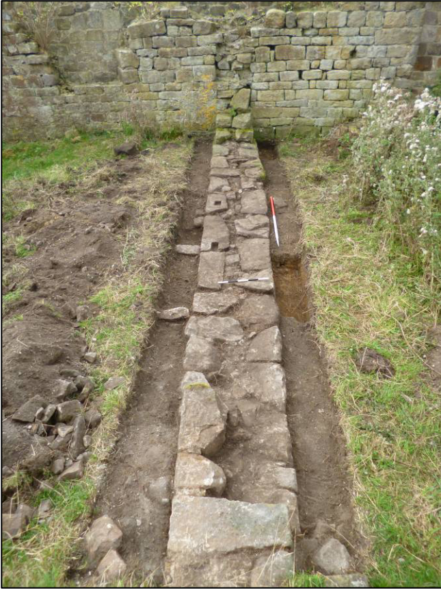
Plate 1: General view of Trench 1 after excavation, looking SW.
