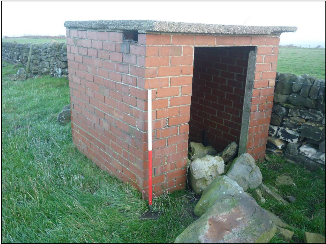
Plate 31: Building R5, looking E (photo 2/949, December 2011).
