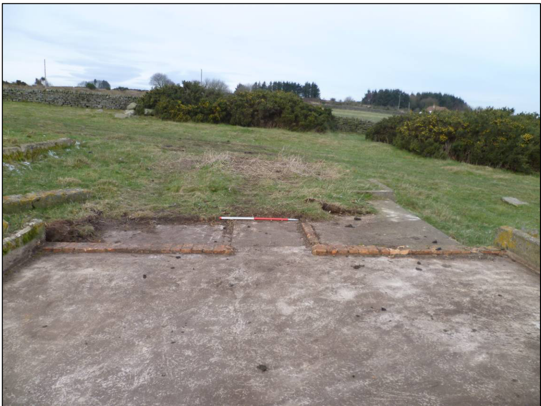
Plate 38: North end of southern part of Building A11 after clearance (photo 4/561, February 2012).
