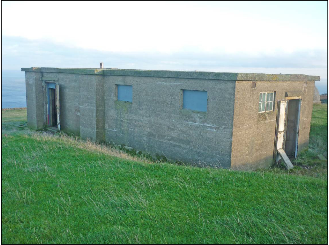
Plate 18: Building R4, north elevation, looking SE (photo 2/971, December 2011).
