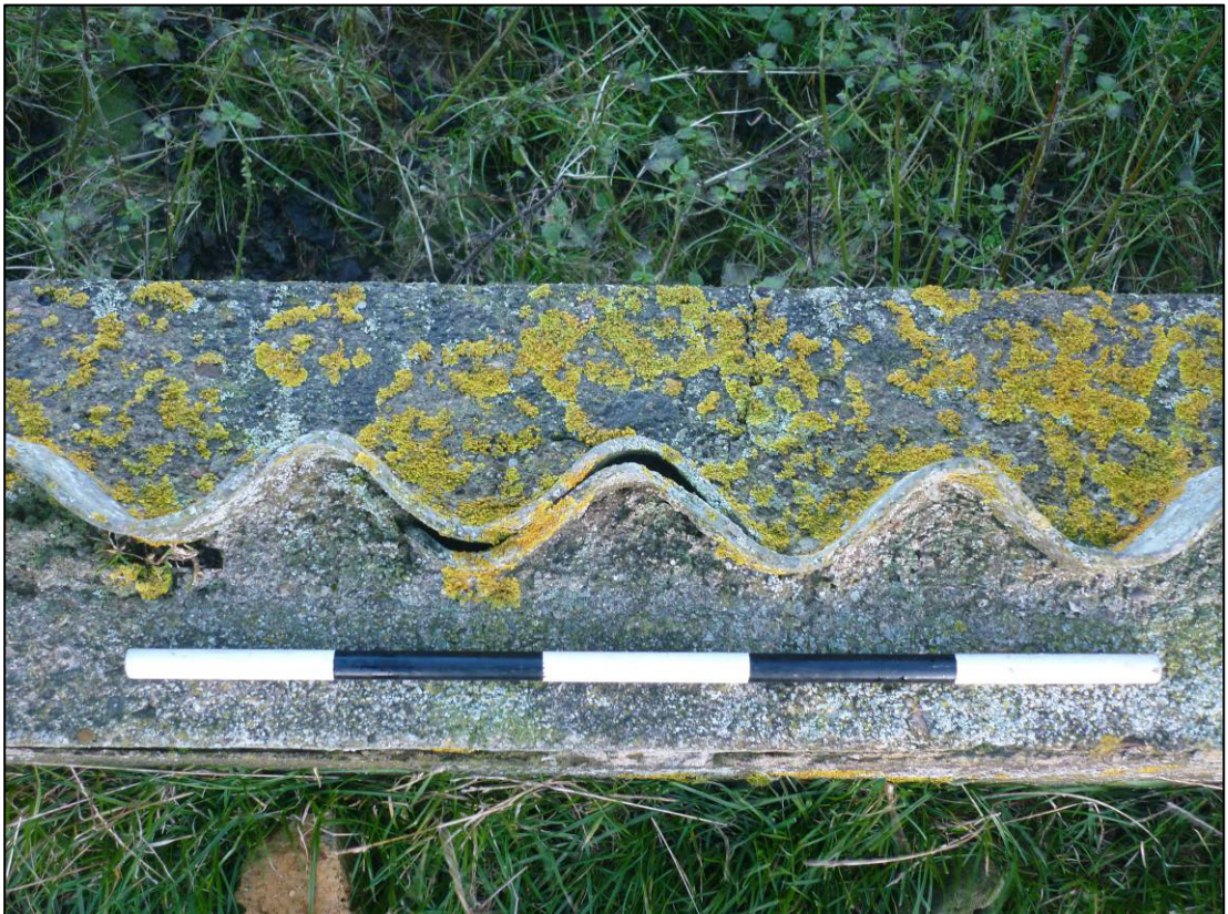
Plate 40: Building A11, detail of asbestos wall on east side (photo 2/940, December 2011).
