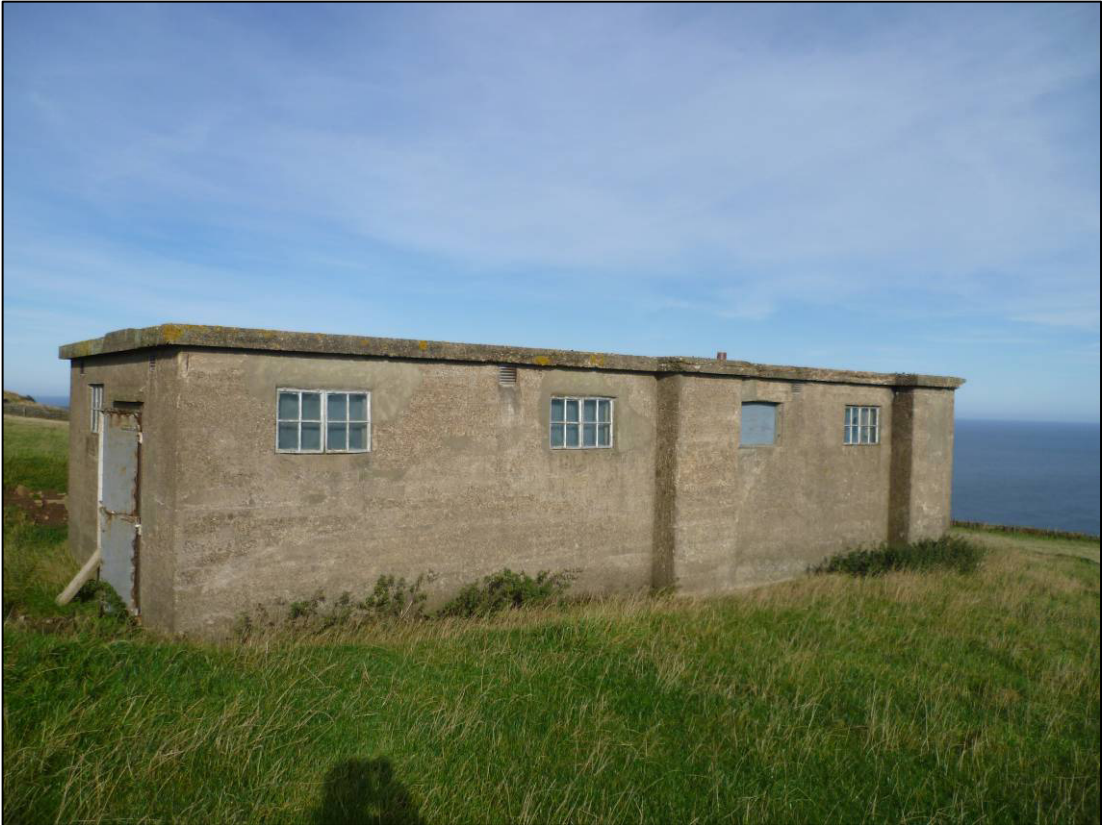
Plate 16: Building R4, south elevation, looking N (December 2011).
