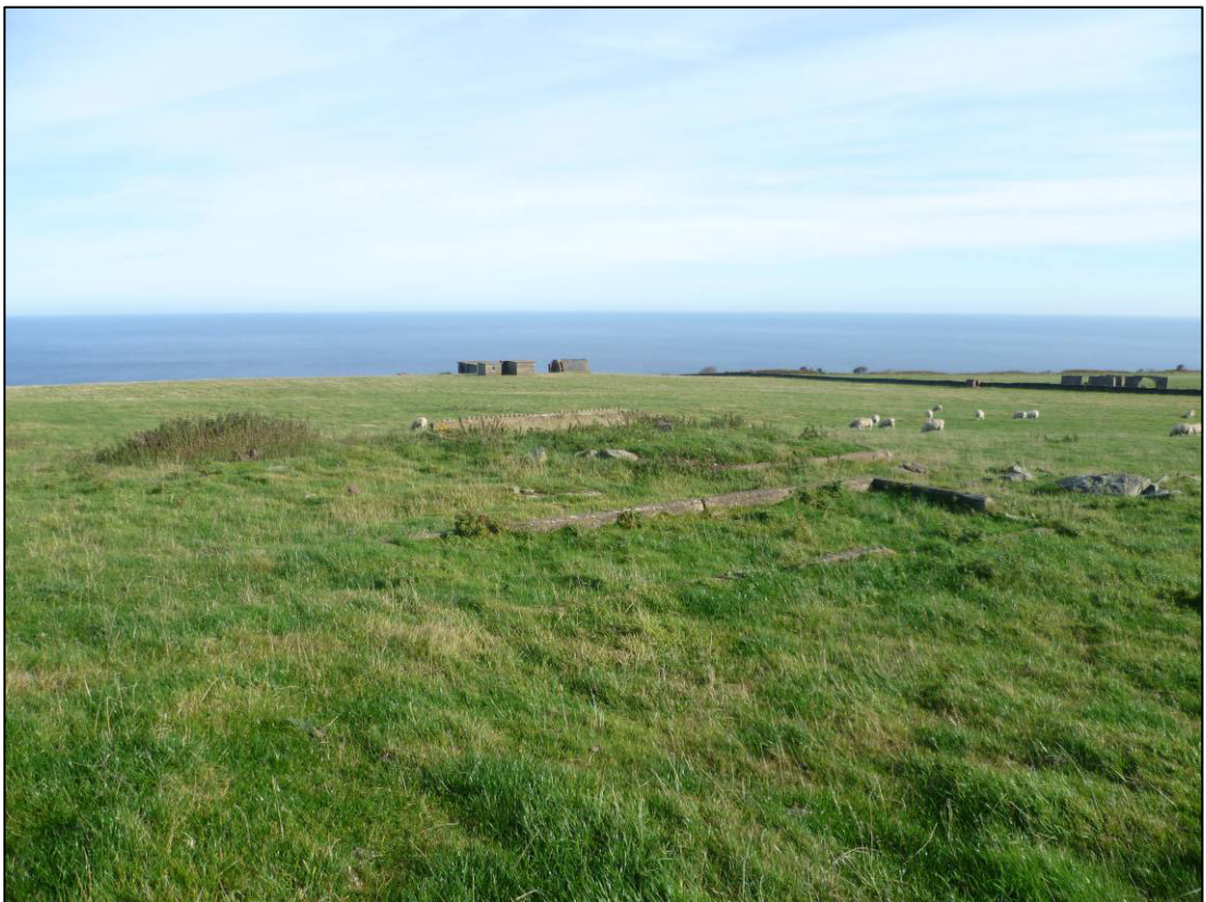
Plate 2: View from accommodation group (Buildings A8 to A11) towards radar buildings, looking E (December 2011).
