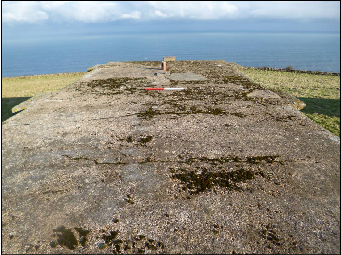
Plate 21: Roof of Building R4, looking E (photo 5/376, December 2012).
