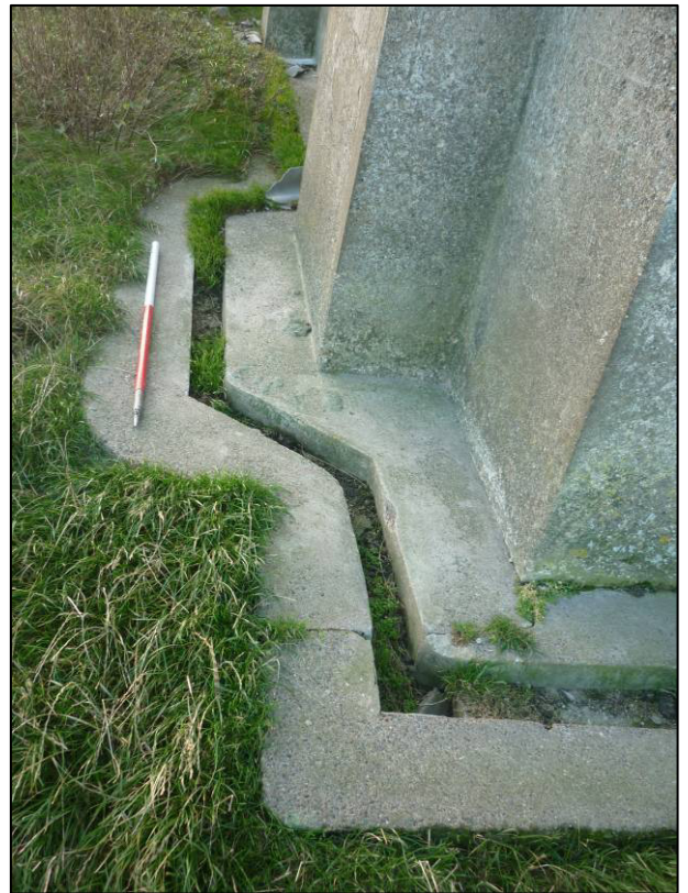
Plate 20: Building R4, external drain around NE corner, looking SW (photo 2/964, December 2011).
