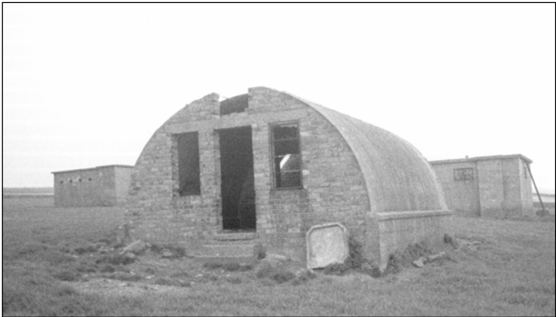
Plate 10: Building R3, looking NW (NT photo 100/9, February 1998).
