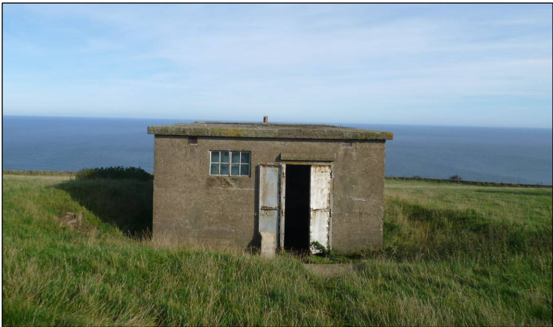
Plate 17: Building R4, west elevation, looking NE showing earthworks (December 2011).
