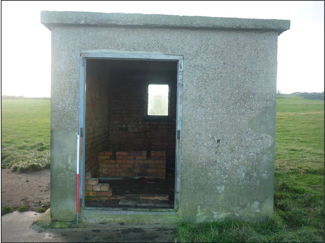
Plate 3: Building R1, east external elevation, looking SW (photo 2/954, December 2011).
