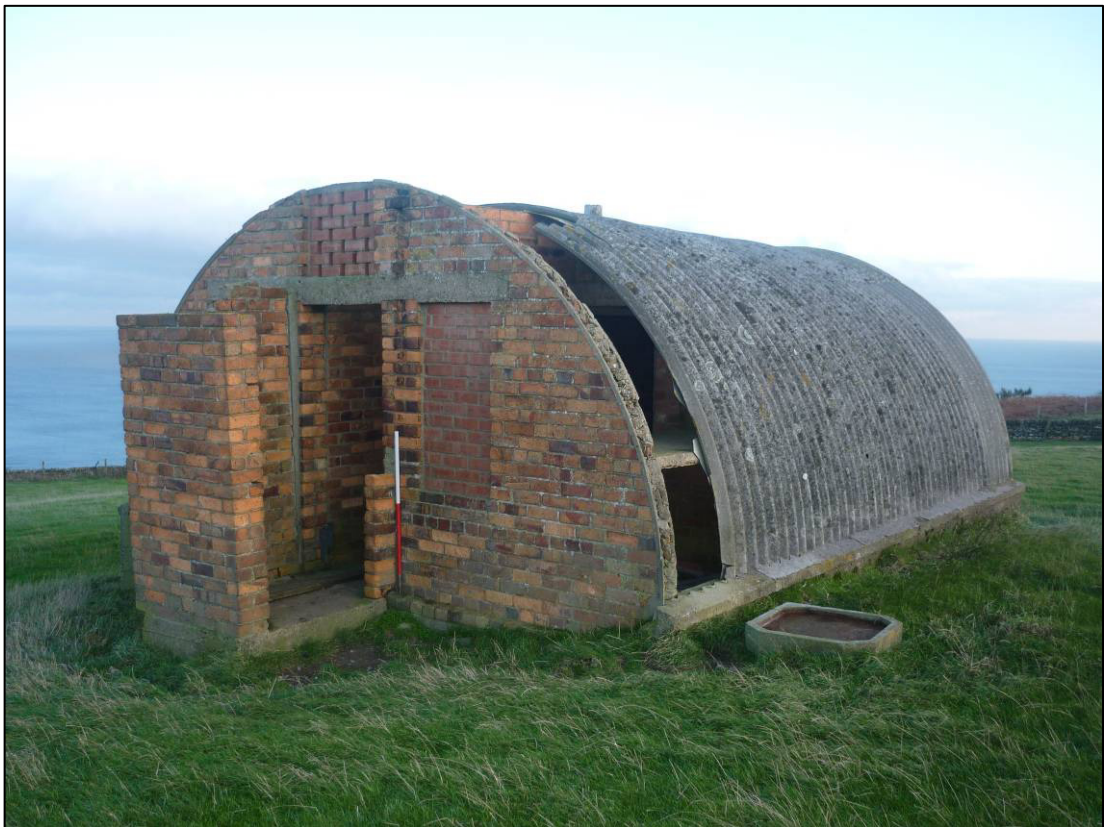
Plate 13: Building R3, looking SE (photo 2/002, December 2011).
