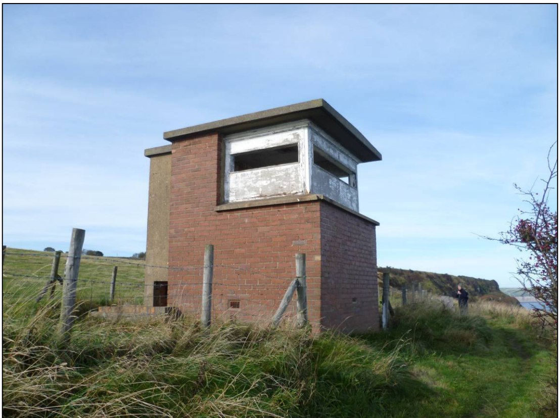
Plate 32: Coastguard station, looking NW (December 2011).
