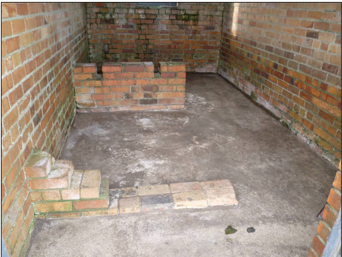
Plate 4: Interior of Building R1 after clearance, showing brick supports for fuel tank, looking SW (photo 4/566, February 2012).
