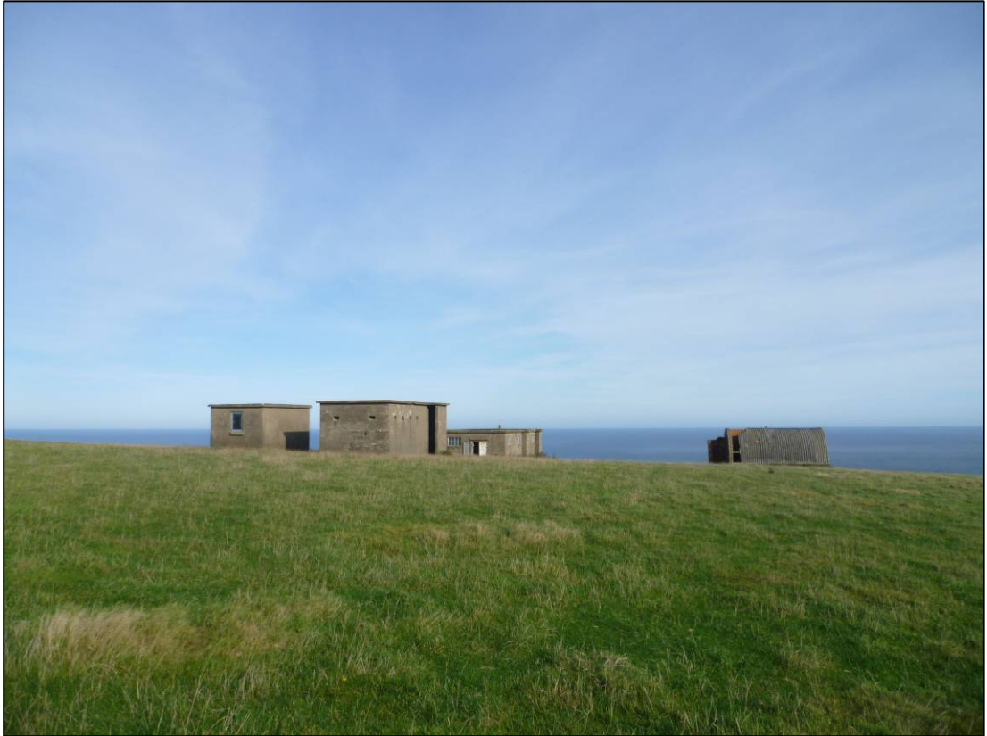
Plate 1: General view towards radar group of buildings, looking NE (December 2011).
