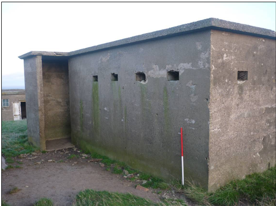
Plate 6: Building R2, north external elevation and porch, looking SE (photo 1/850, December 2011).
