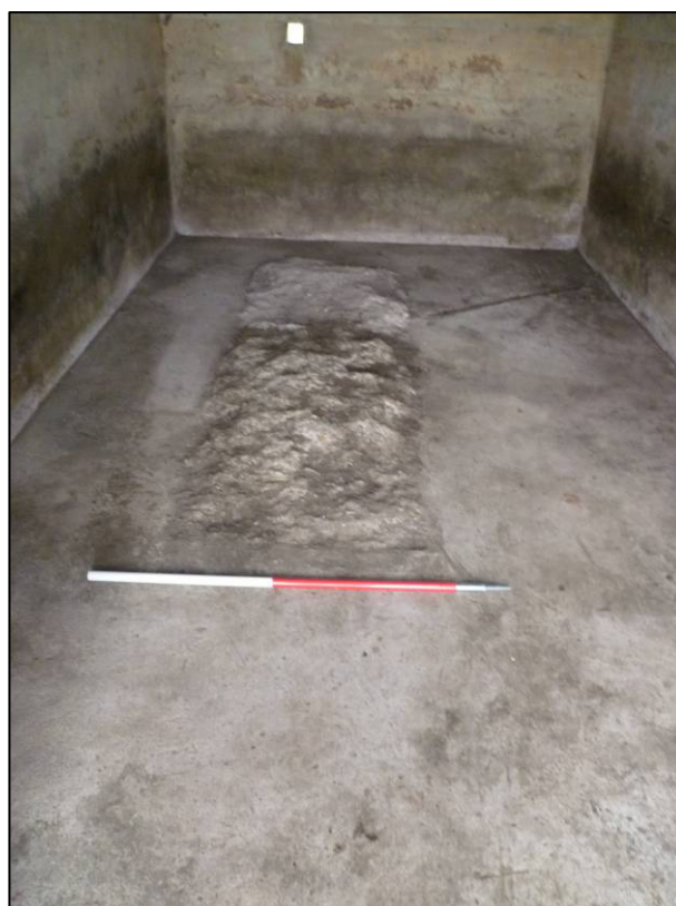
Plate 9: Building R2, remains of engine bed after clearance, looking SW (photo 4/573, February 2012).
