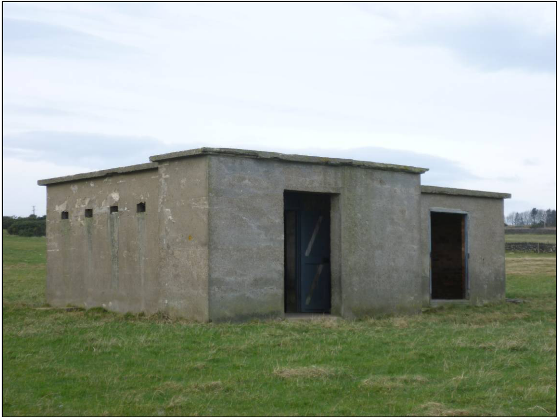
Plate 5: Building R2, south and east external elevations, looking NW (photo 4/575, February 2012).
