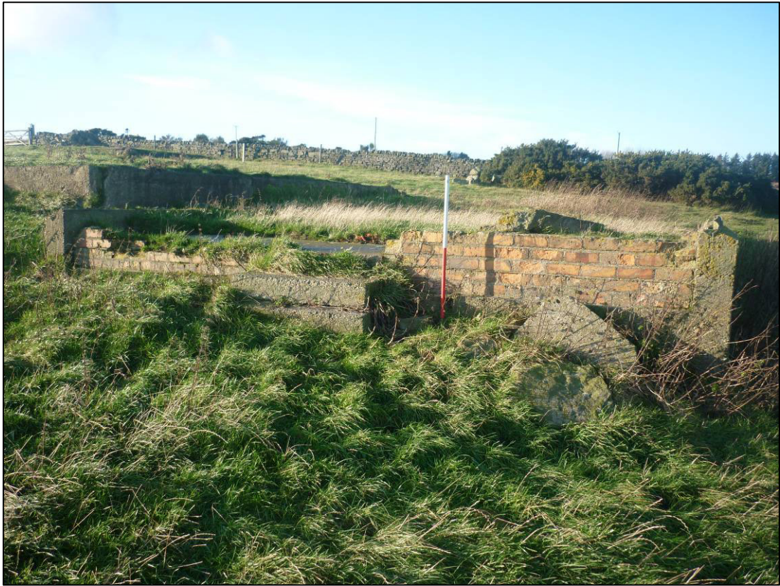
Plate 37: Building A11, looking NW (photo 2/935, December 2011).
