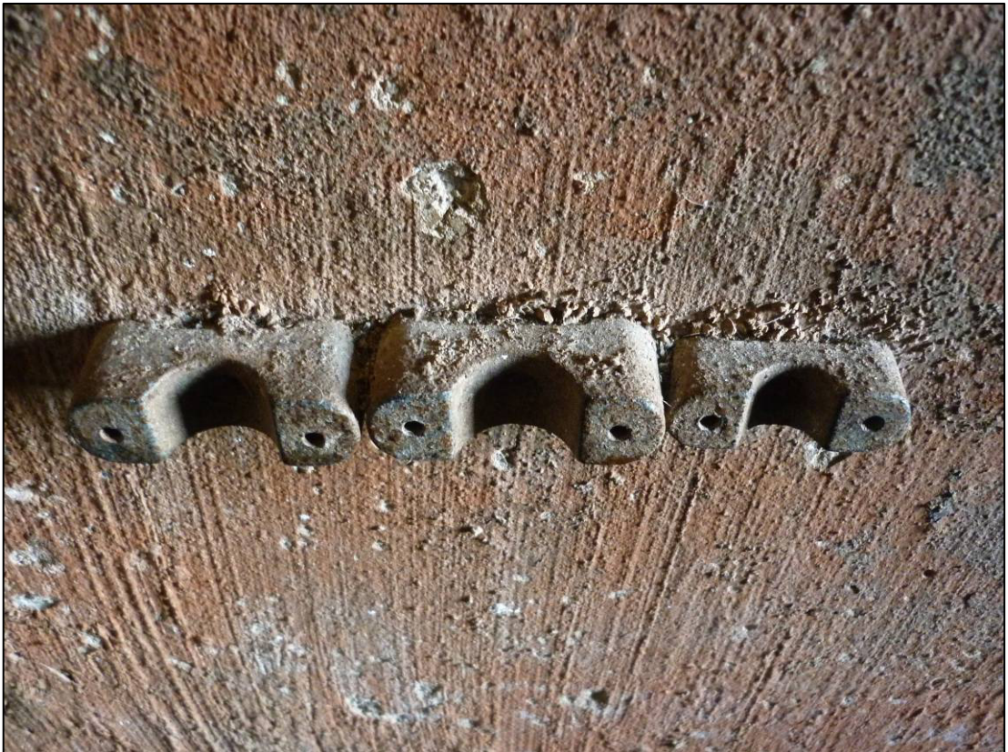
Plate 28: Building R4, west internal elevation of east room, showing bakelite clips, looking SW (photo 3/292, January 2012).
