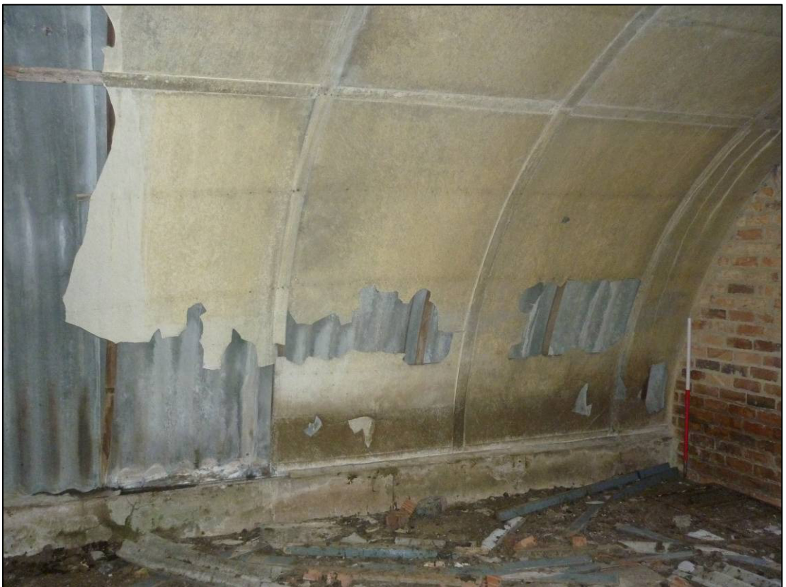
Plate 15: Building R3, interior showing construction, looking SW (photo 2/023, December 2011).
